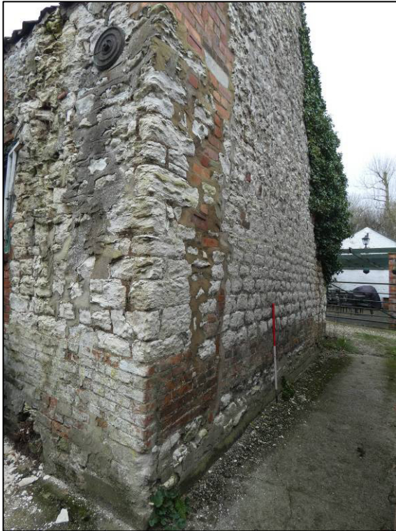
Photo 6: North gable, looking SW (photo 1/884).
