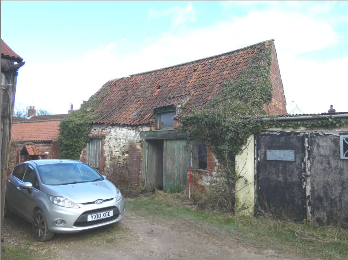
Plate 1: Recorded building, looking N (photo 1/893).
