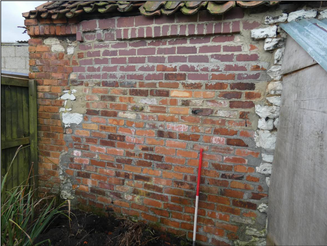
Plate 10: East elevation, south part, showing area of rebuild, looking SW (photo 1/878).
