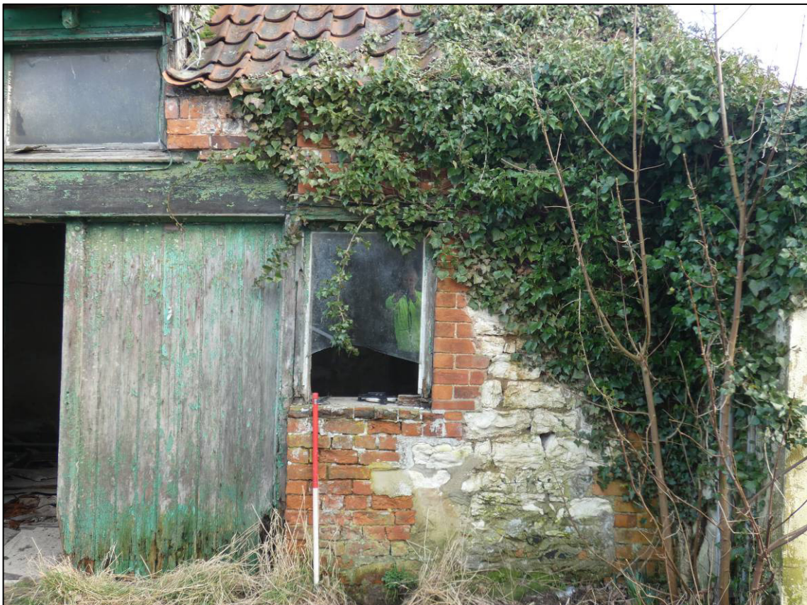
Plate 4: West elevation, southern part, looking NE (photo 1/894).
