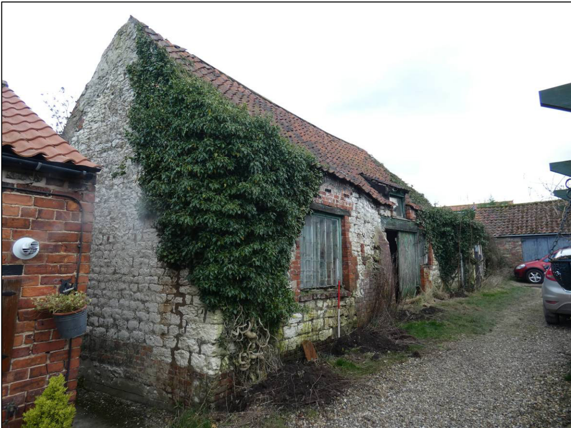
Plate 2: Recorded building, looking SE (photo 1/905).
