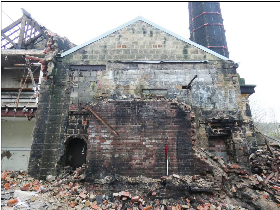
Plate 49: Economiser house after demolition, south wall, looking S (photo 3621).
