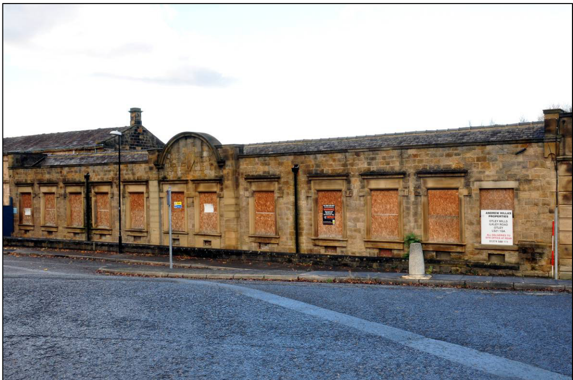
Plate 45: Ilkley Road frontage, 1891-1908 extension (Unit D), looking NW (photo 11716).
