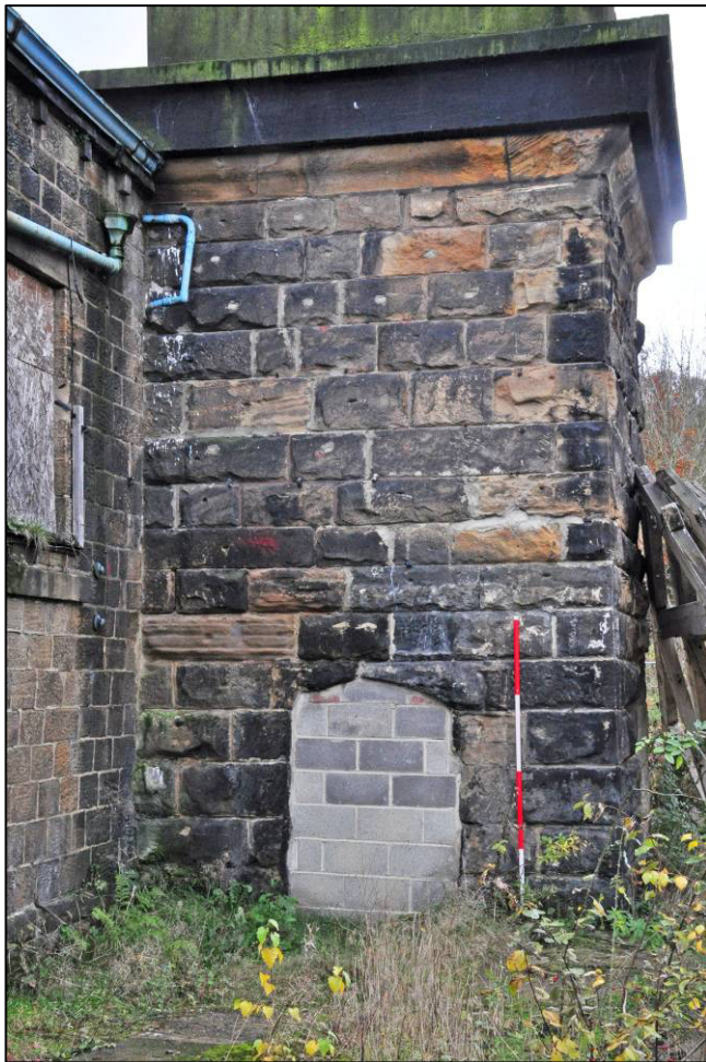
Plate 5: Chimney, north side of base, looking S (photo 11789).
