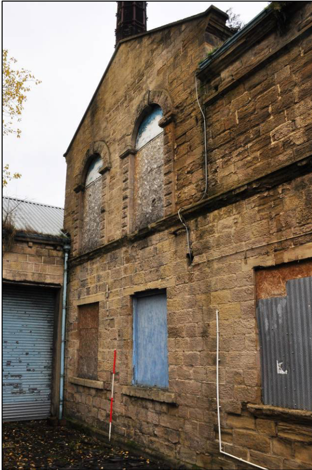
Plate 8: Southern engine house, south gable, looking NW (photo 11749).
