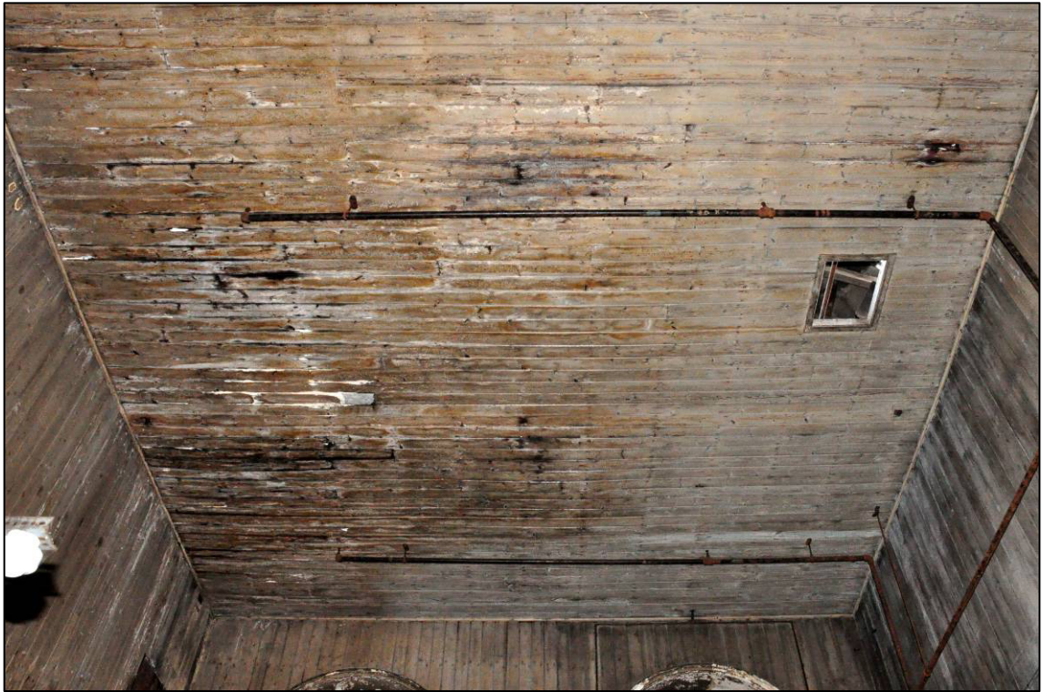
Plate 24: Southern engine house, ground floor, match boarding to ceiling, looking S (photo 11849).
