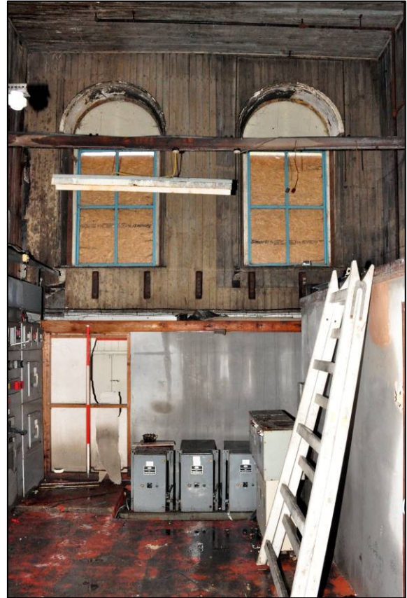
Plate 21: Southern engine house, ground floor, south wall, looking S (photo 11838).
