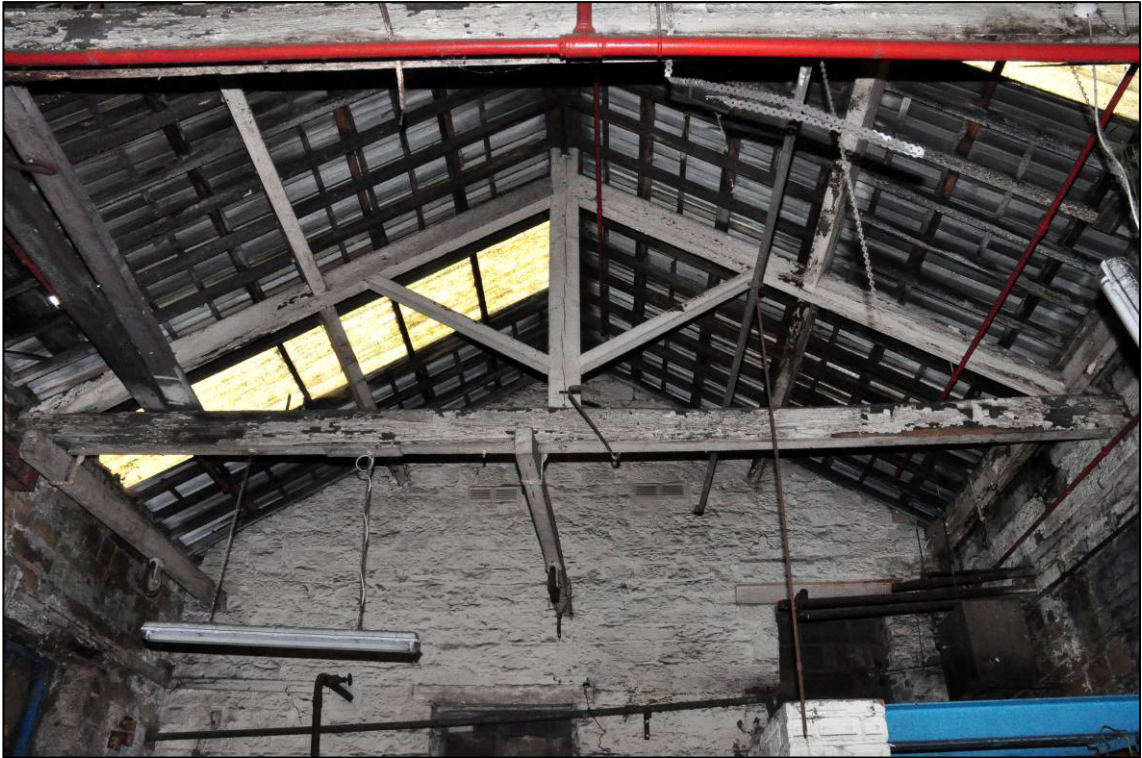
Plate 17: Boiler house, northernmost roof truss, looking N (photo 11831).
