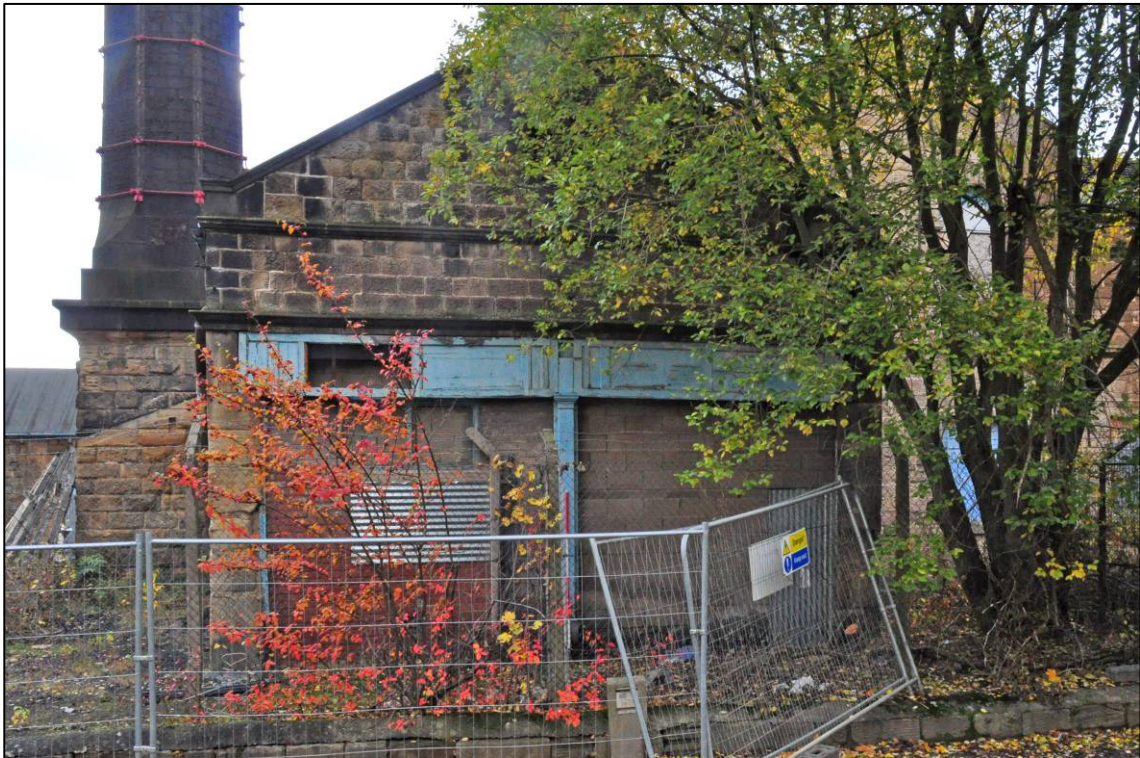
Plate 2: Boiler house, south gable, looking N (photo 11759).
