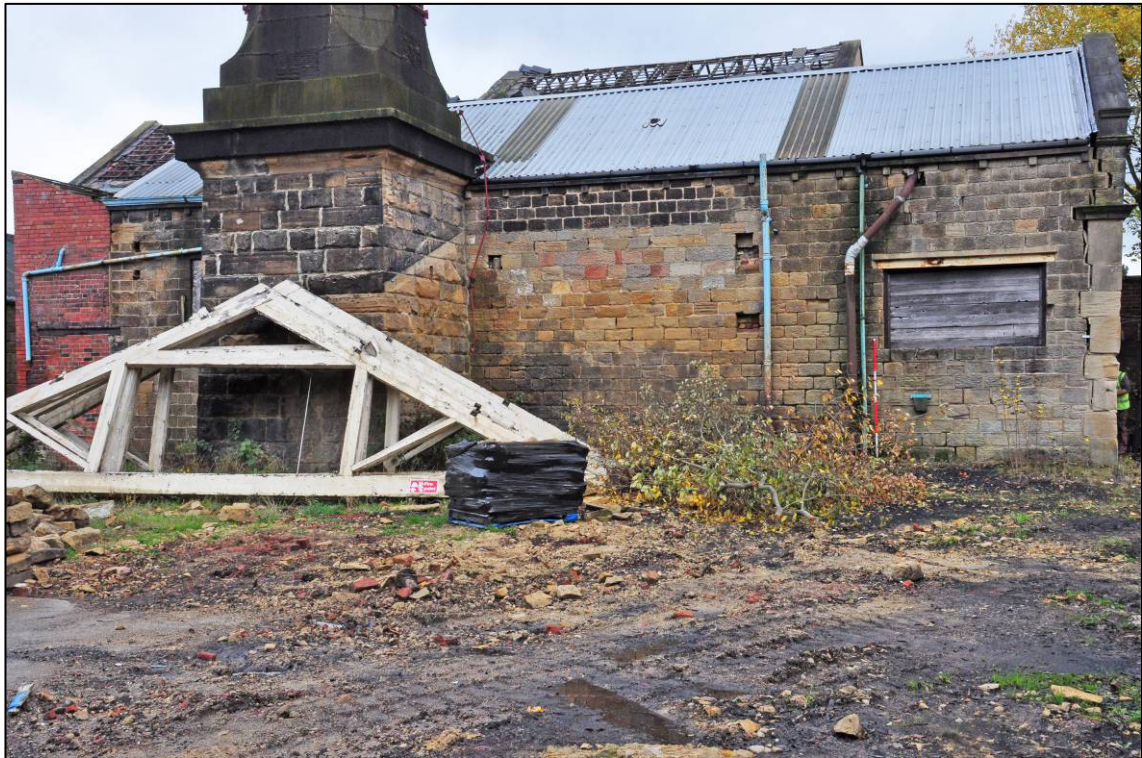
Plate 4: Boiler house, west elevation and chimney, looking NE (photo 11775).
