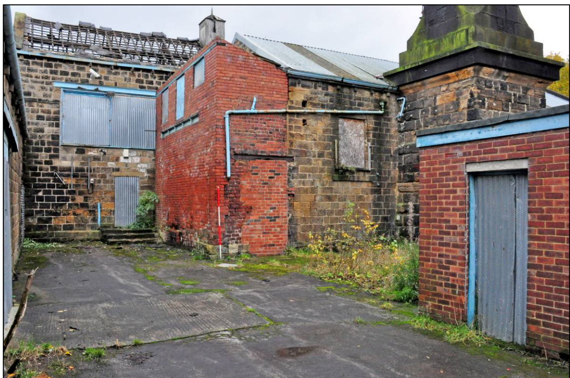
Plate 7: Economiser house, west and north elevations, looking NE (photo 11787).
