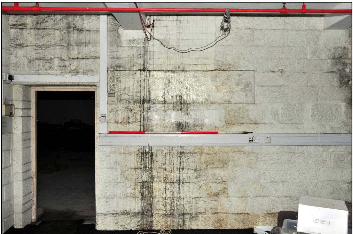
Plate 33: Northern engine house, ground floor, bearing box at north end of east wall, looking E (photo 11803).
