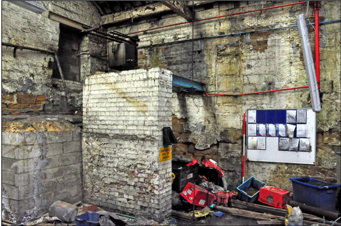
Plate 15: Boiler house, north end of east wall, looking E (photo 11825).
