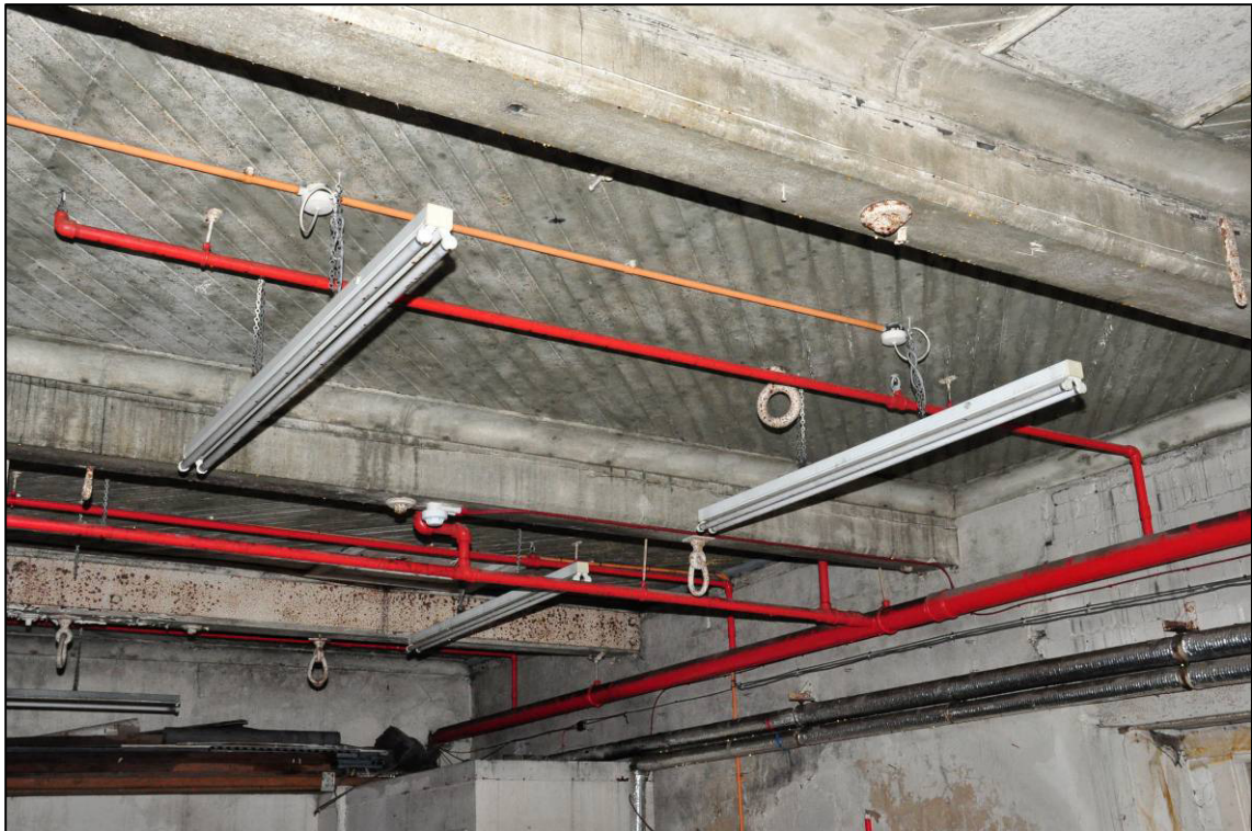
Plate 36: Northern engine house, first floor, ceiling beams with lifting rings, looking NE (photo 11855).
