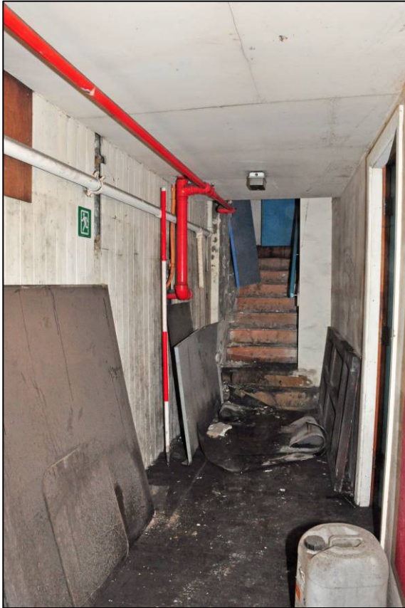
Plate 20: Southern engine house, ground floor, modern north-south corridor, looking N (photo 11836).
