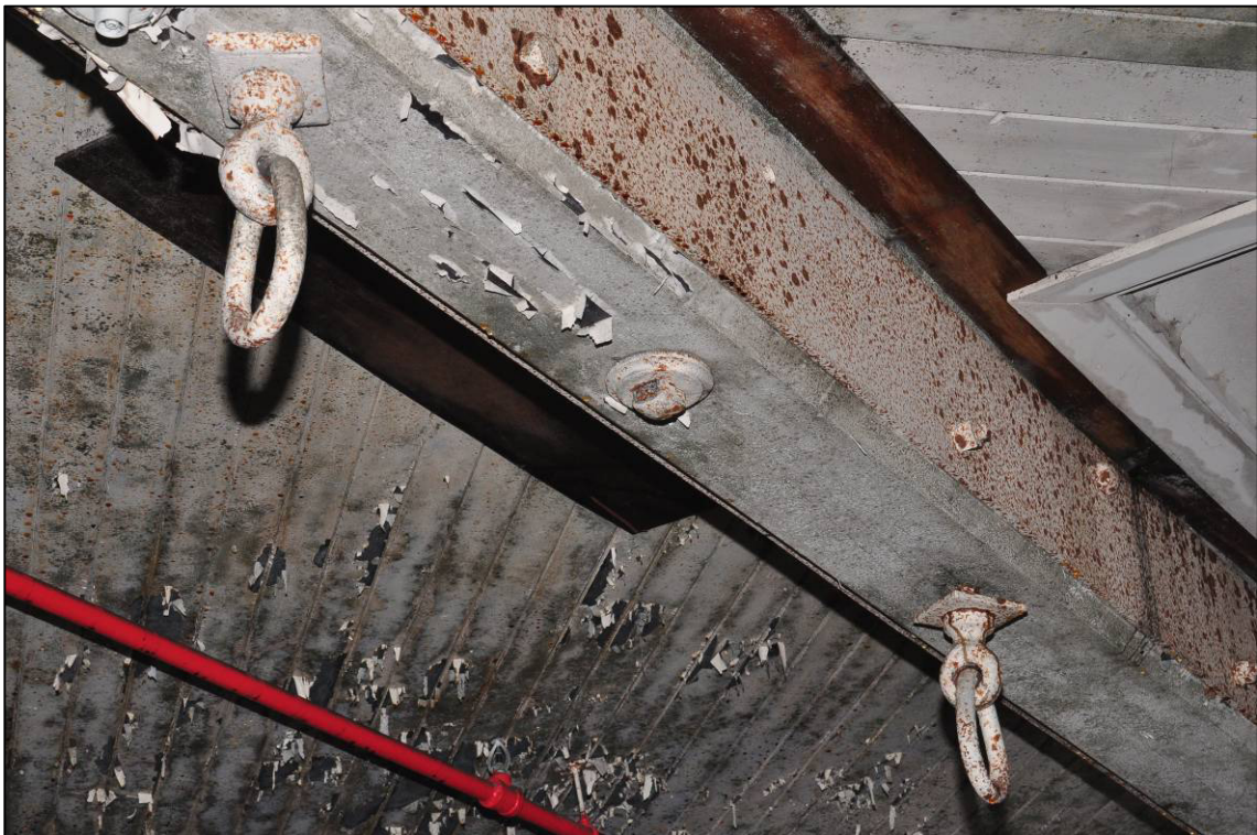
Plate 37: Northern engine house, first floor, lifting rings, looking SW (photo 11858).
