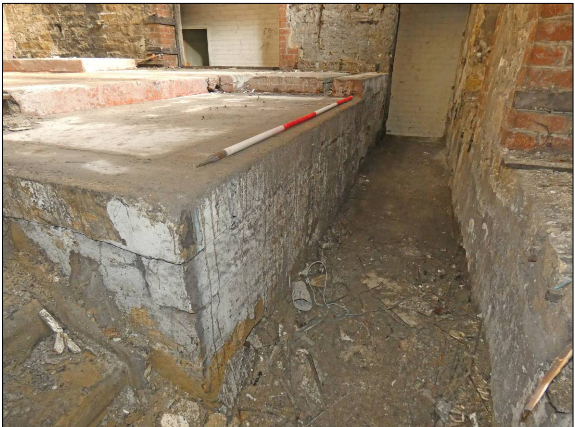
Plate 25: Southern engine house, ground floor after stripping out, original engine bed, looking E (photo 2387).
