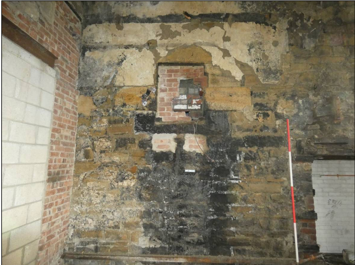
Plate 28: Southern engine house, ground floor after stripping out, bearing box at north end of east wall, looking E (photo 2378).
