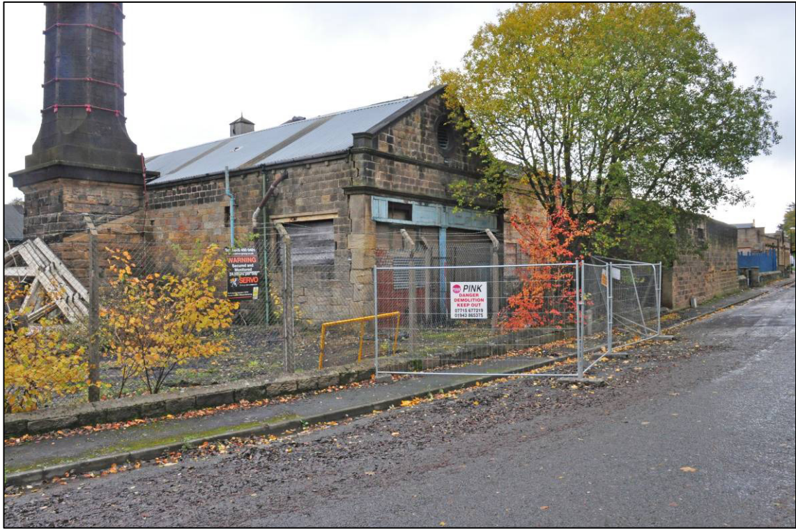
Plate 1: Boiler house, south gable and south end of west elevation, looking NE (photo 11765).
