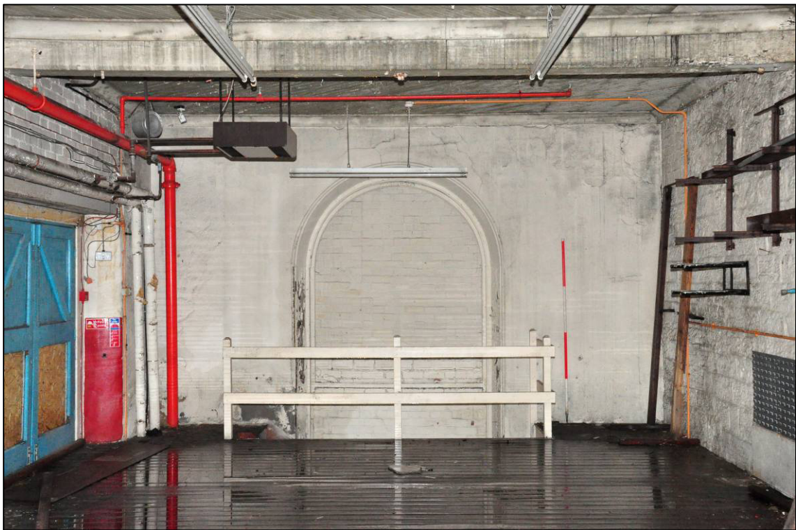
Plate 35: Northern engine house, first floor, north wall, looking N (photo 11851).
