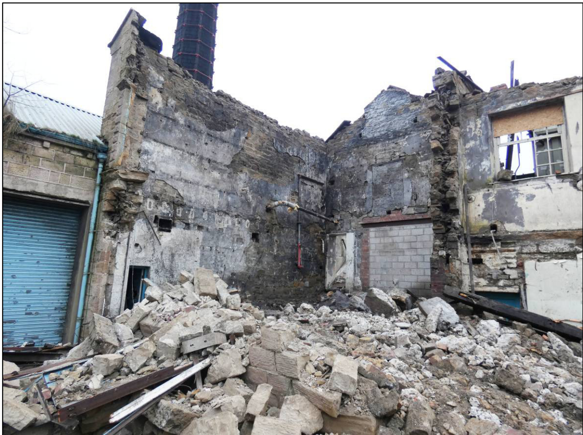
Plate 54: Southern engine house engine bed during demolition, looking NW (photo 4663).
