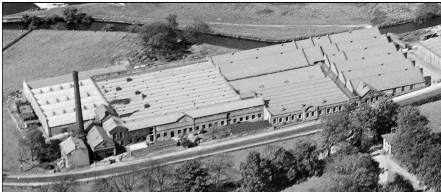
A) 1926 Aerial photograph of the Otley Worsted Mills, Otley, detailed view (Source: Historic Environment Scotland, EPW015692 © Historic England).
