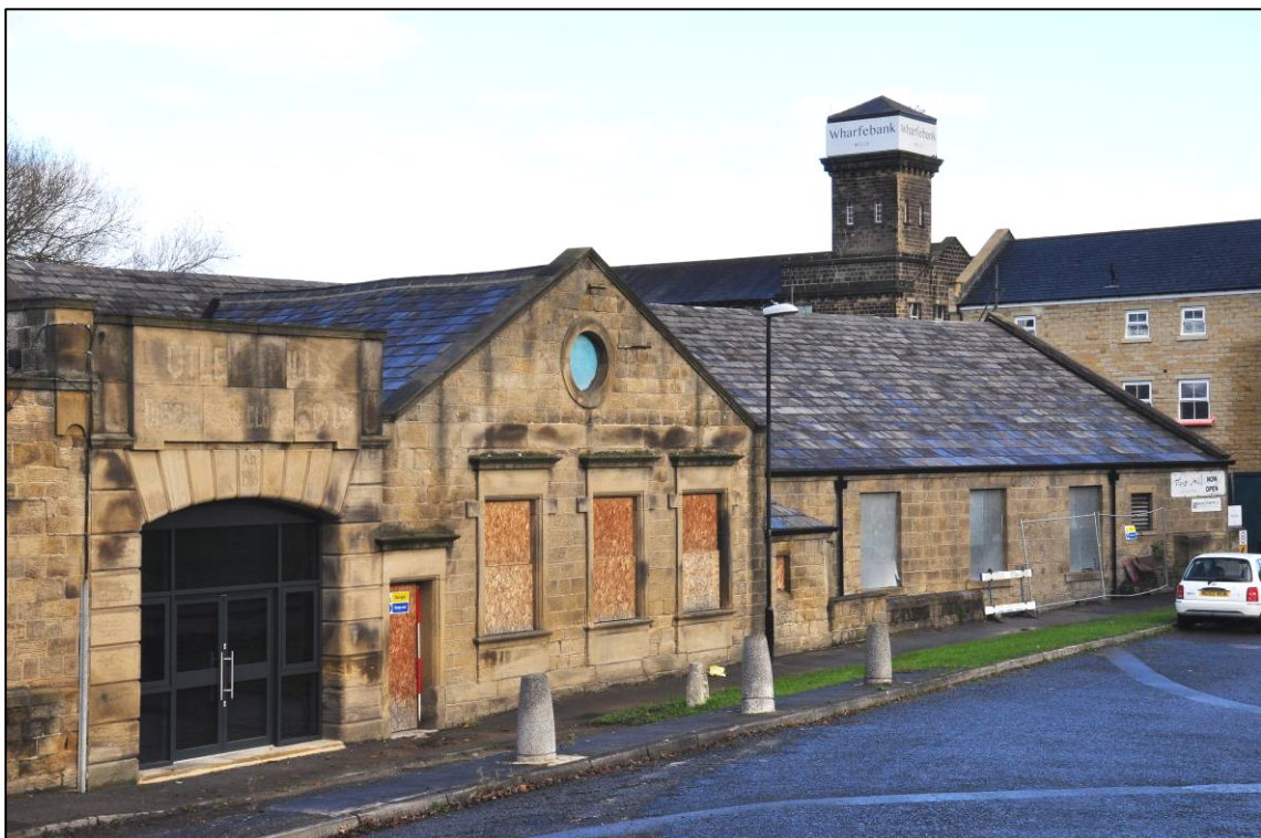
Plate 47: Ilkley Road frontage, 1908-21 extension (Unit E), looking NE (photo 11705).
