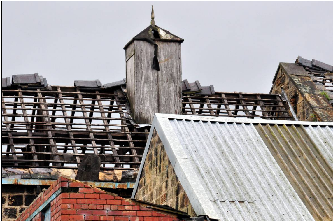
Plate 13: Northern engine house, roof with wooden vent, looking E (photo 11786).
