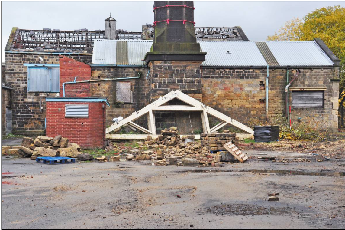
Plate 3: Boiler house, west elevation and chimney, looking E (photo 11772).
