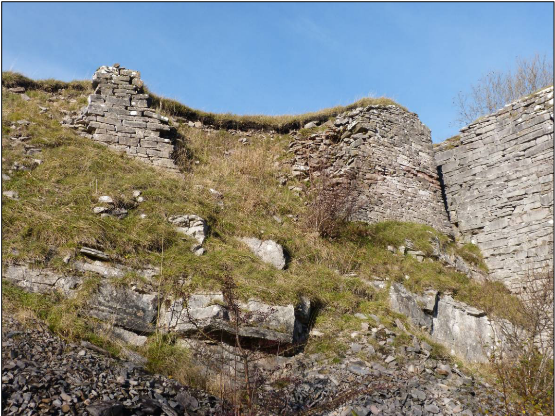
Plate 16: Smardale quarry, upper level of retaining wall (Site 101/1), looking NW (photo 2/108).
