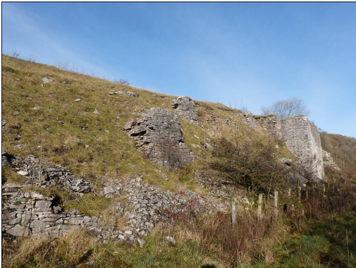
Plate 15: Smardale quarry, retaining walls (Sites 101/1 and 101/2), looking NW (photo 2/111).
