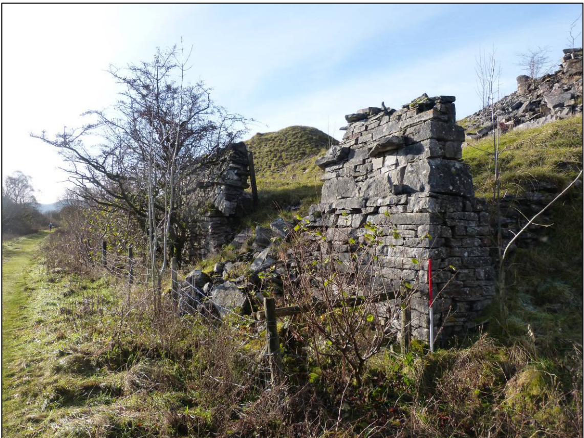
Plate 17: Smardale quarry, north end of trackside structure (Site 102), looking SW (photo 2/113).
