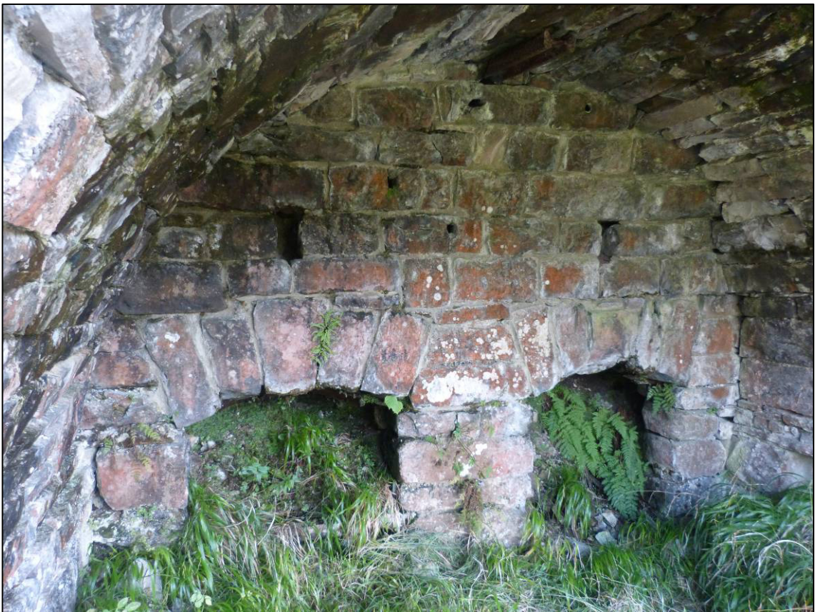
Plate 7: Smardale kilns, west wall of north draw arch, looking W (photo 1/016).
