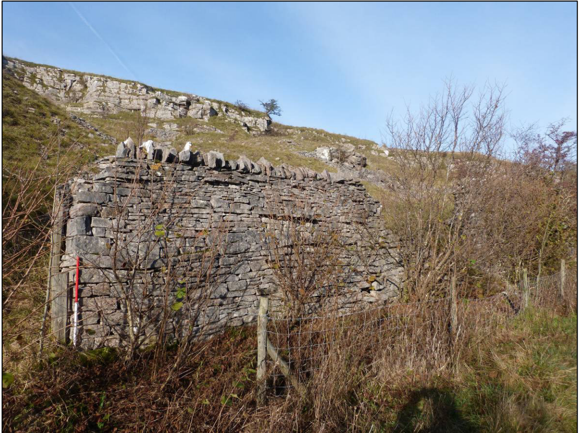
Plate 18: Smardale quarry, south end of trackside structure (Site 102), looking NW (photo 2/117).
