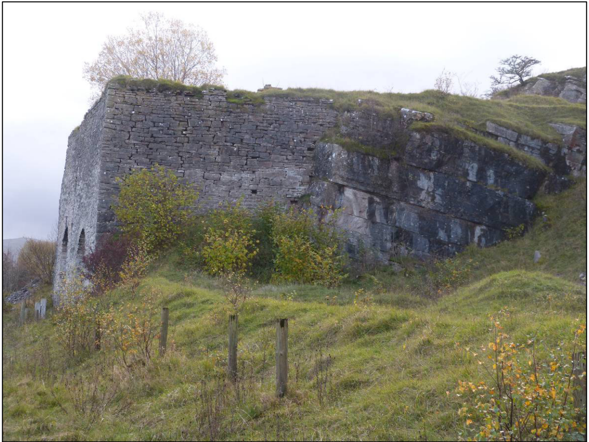
Plate 3: Smardale kilns, north elevation, looking S (photo 1/060).
