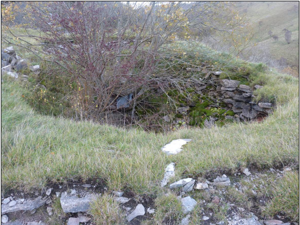
Plate 13: Smardale kilns, top of south charge bowl, looking N (photo 1/054).
