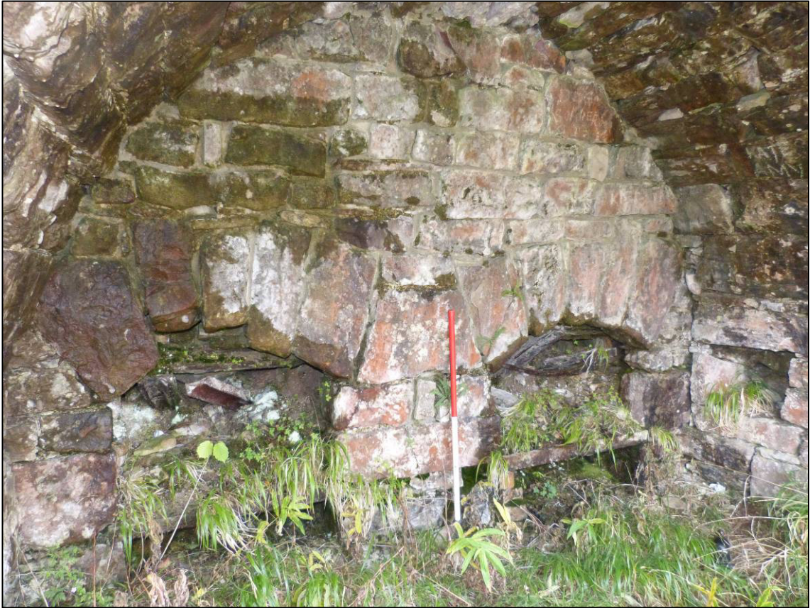
Plate 6: Smardale kilns, west wall of south draw arch, looking W (photo 1/028).
