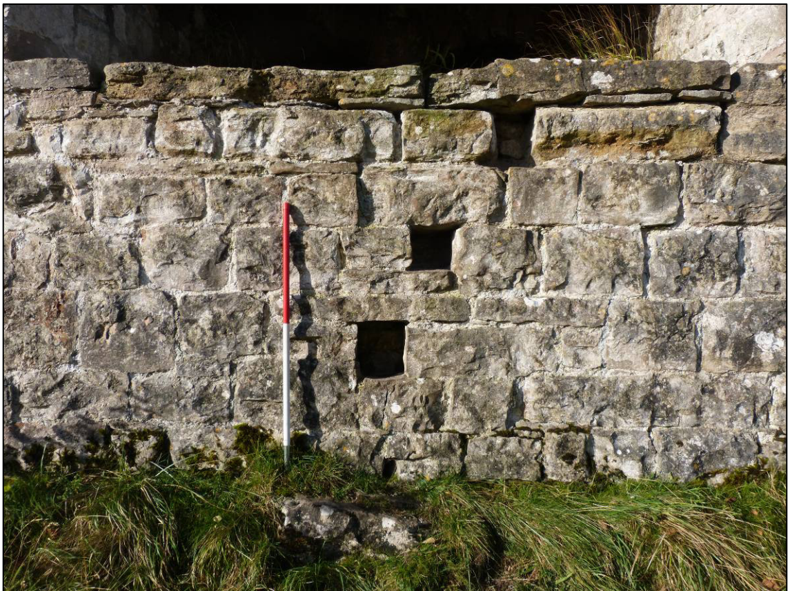
Plate 2: Smardale kilns, sockets beneath south draw arch in east elevation, looking W (photo 1/008).
