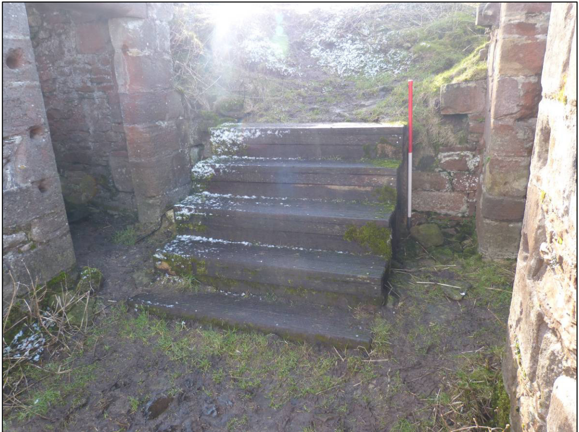
Plate 80: Pendragon Castle, entrance passage, modern wooden steps, looking S (photo 9/546).
