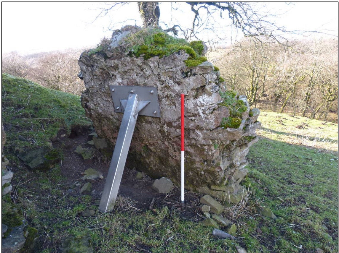
Plate 47: Pendragon Castle, propped masonry at north-west corner of castle, looking SW (photo 9/574).
