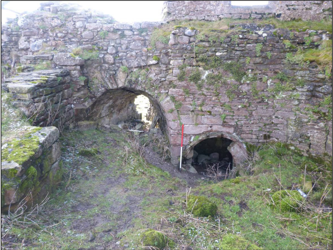
Plate 84: Pendragon Castle, west end of south internal wall, looking S (photo 9/553).
