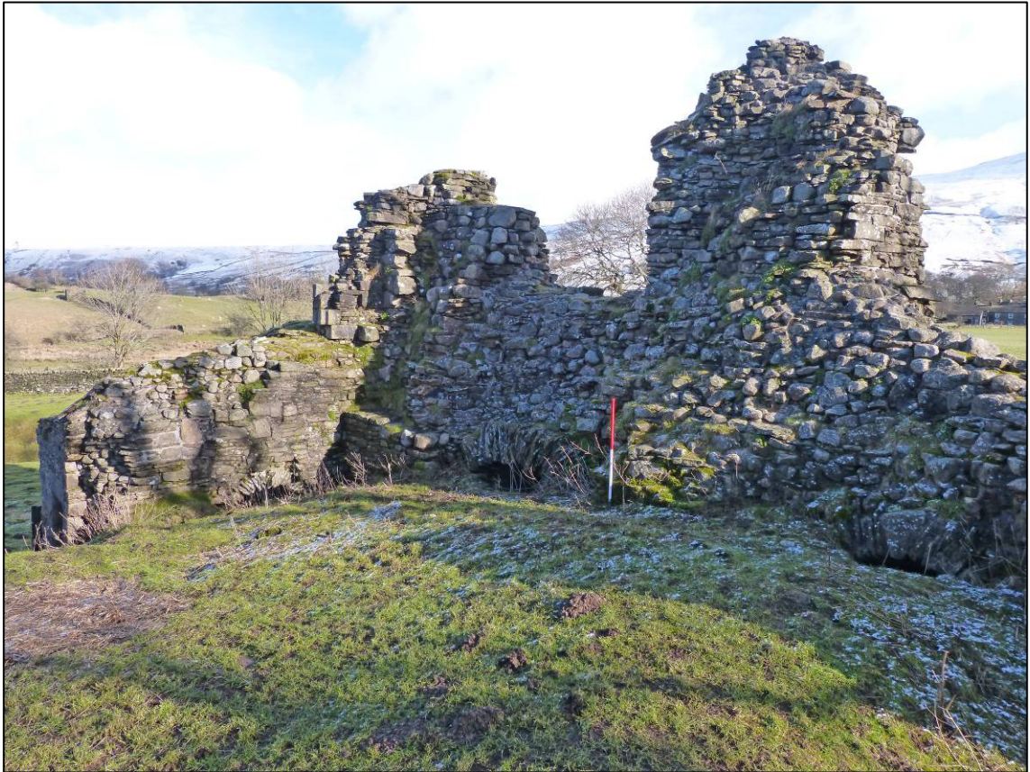
Plate 63: Pendragon Castle, interior, looking NE (photo 9/558).
