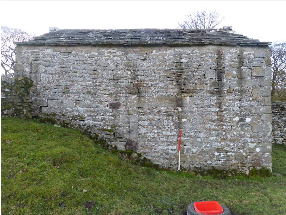
Plate 69: Pendragon Castle barn, east elevation, looking W (photo 3/191).
