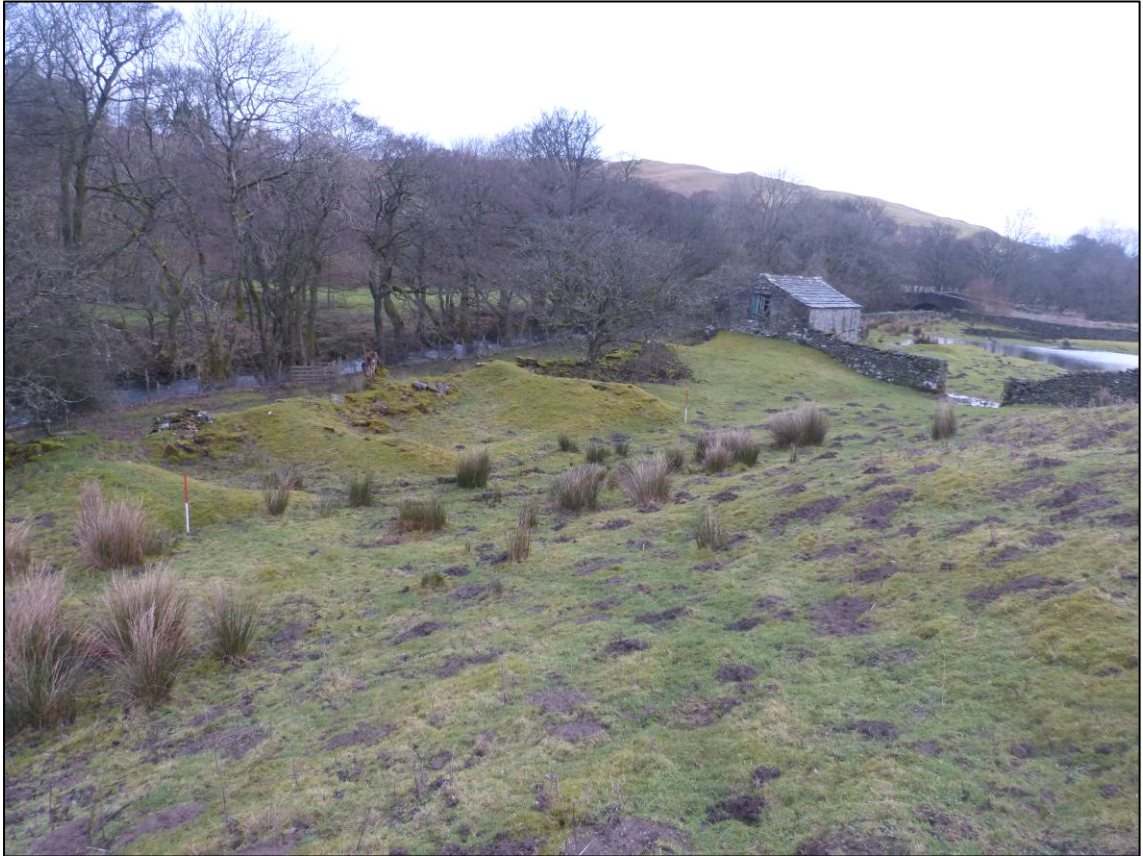
Plate 40: Pendragon Castle, south part of building range (Site 204/2), looking NW (photo 7/473).
