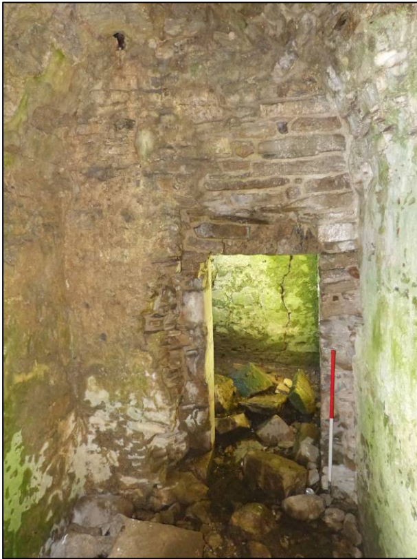
Plate 60: Pendragon Castle, interior of south-east chamber, garderobe doorway, looking W (photo 9/593).
