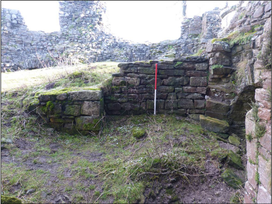
Plate 56: Pendragon Castle, cross wall to south side of interior, looking E (photo 9/554).
