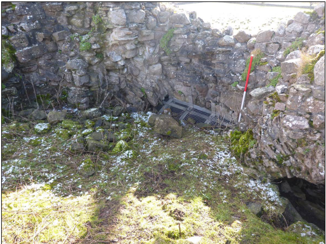
Plate 83: Pendragon Castle, interior, repaired roof of SE chamber, looking SE (photo 9/555).
