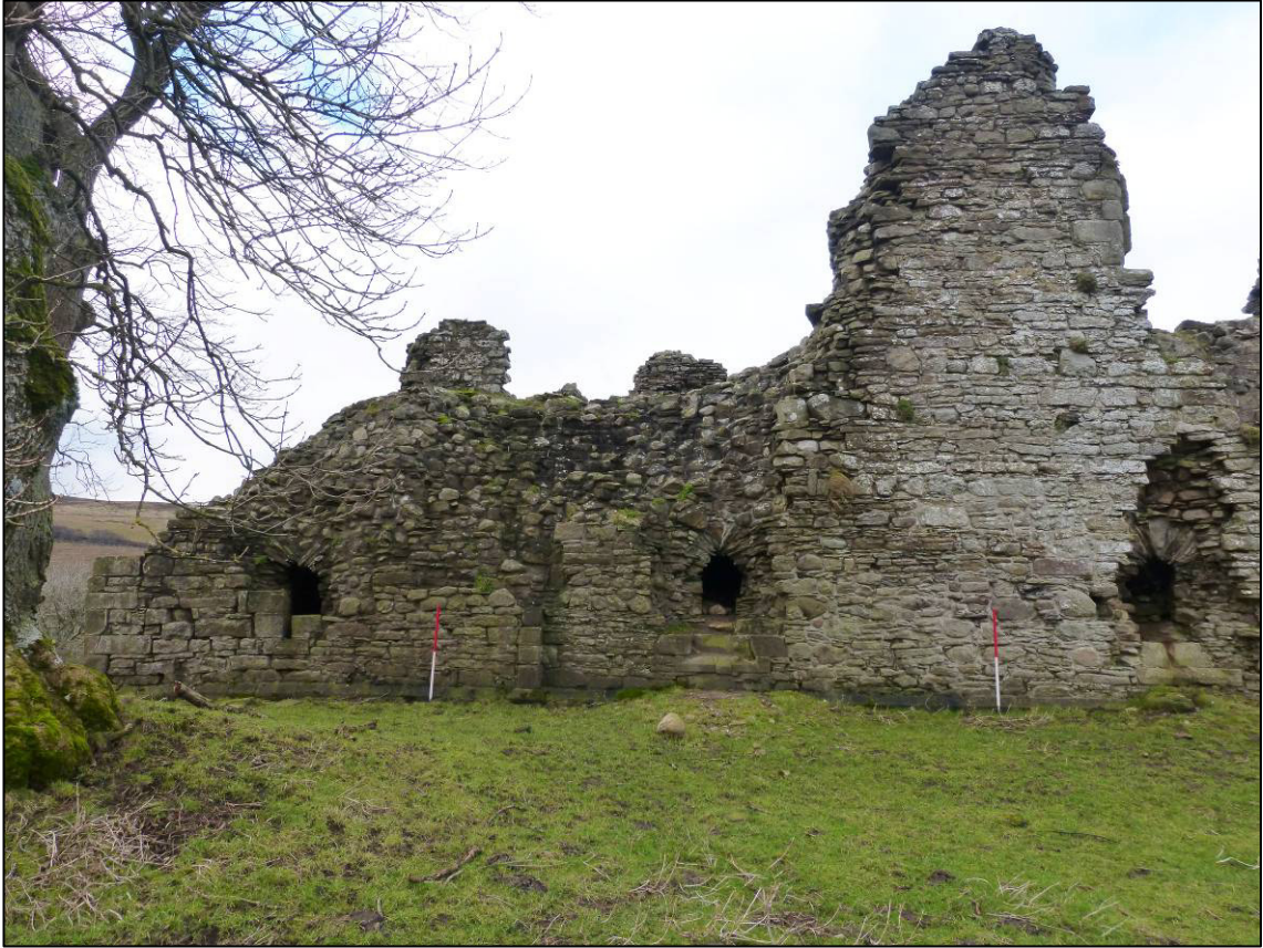
Plate 48: Pendragon Castle, east external elevation, looking W (photo 7/512).
