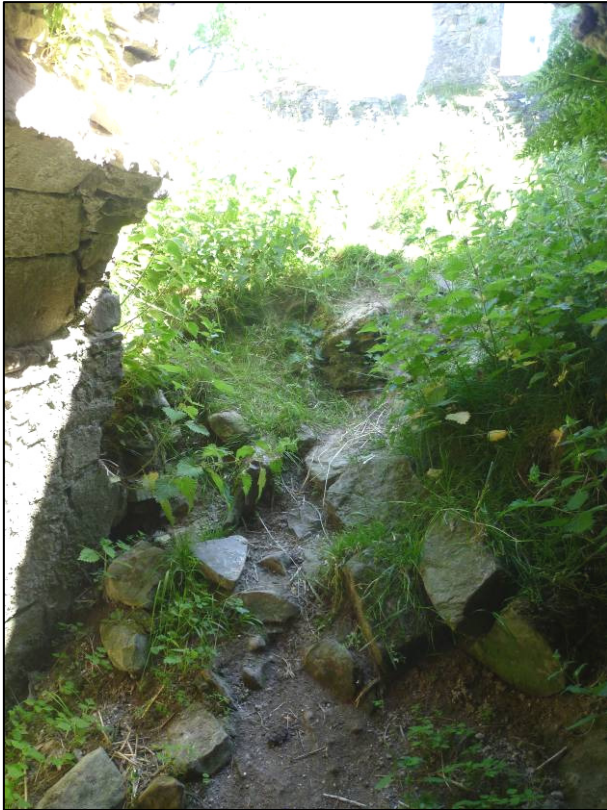
Plate 81: Pendragon Castle, interior, entrance to north-west chamber, looking S (photo 10/183).
