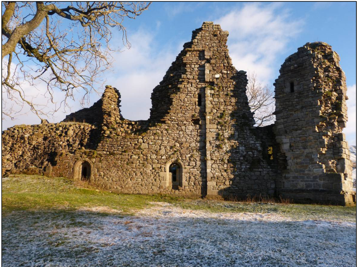
Plate 52: Pendragon Castle, west external elevation, looking E (photo 6/314).
