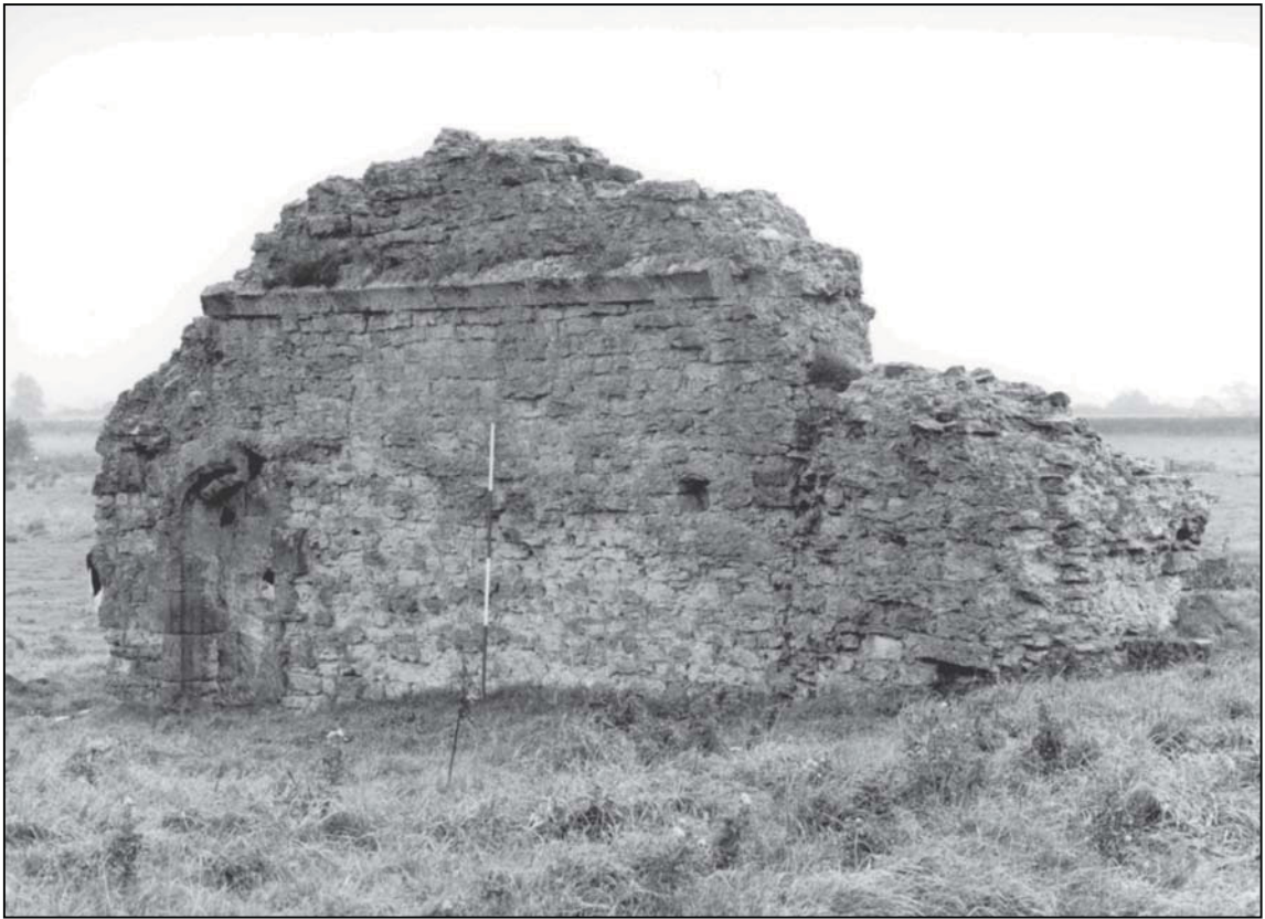
Plate 1: East elevation prior to consolidation, looking SW (photo 1/17).
