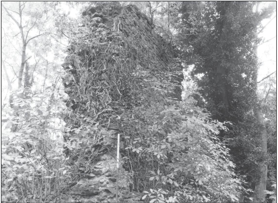
Plate 2: West elevation prior to vegetation clearance and consolidation, looking S (photo 1/13).
