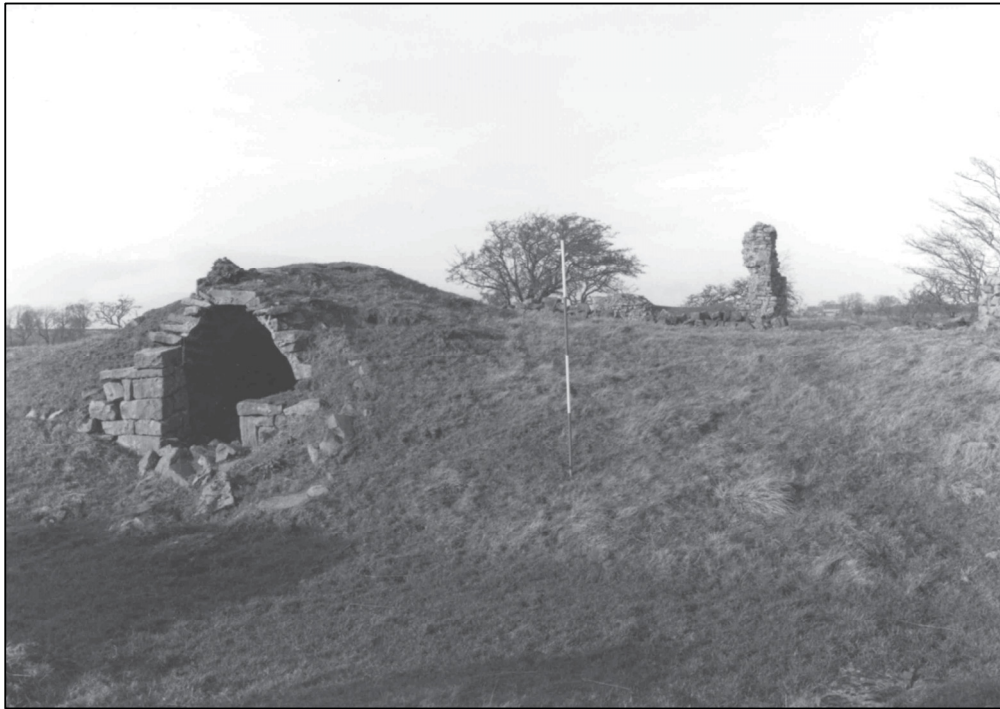
Plate 4: West turnip house before consolidation, looking N (photo 2/14).
