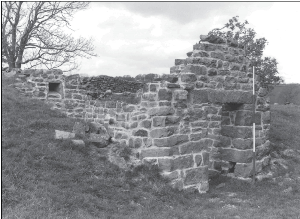
Plate 6: East turnip house after consolidation, looking NE (photo 4/12).
