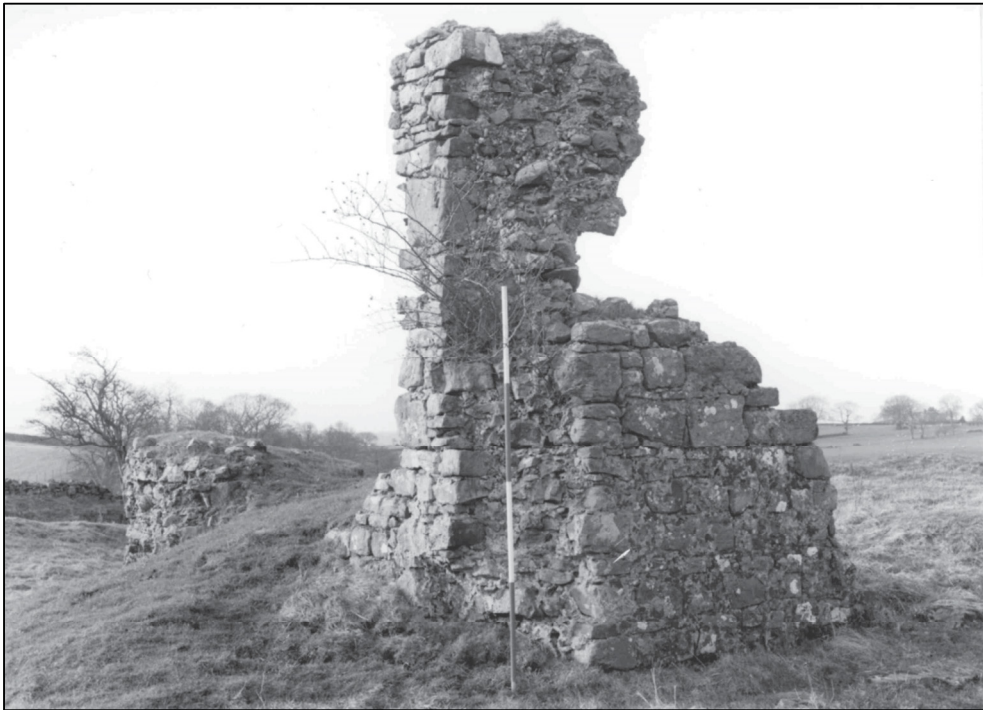
Plate 2: Standing masonry before consolidation, looking NW (photo 1/15).
