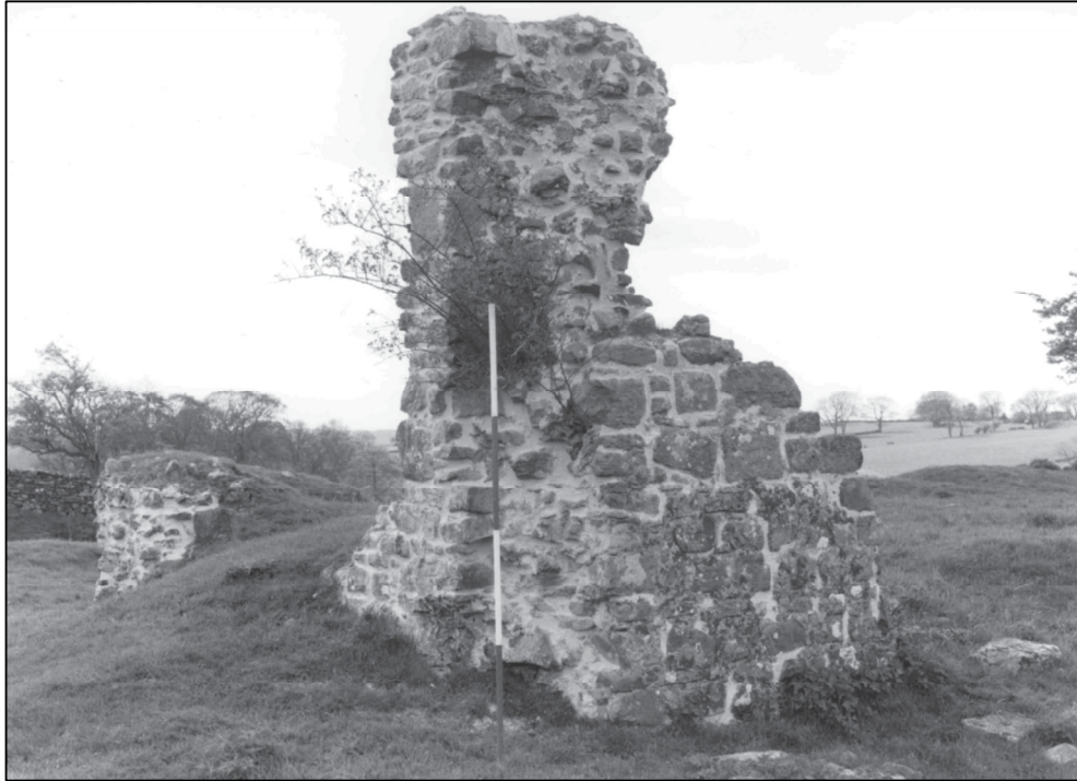
Plate 5: Standing masonry after consolidation, looking NW (photo 4/6).
