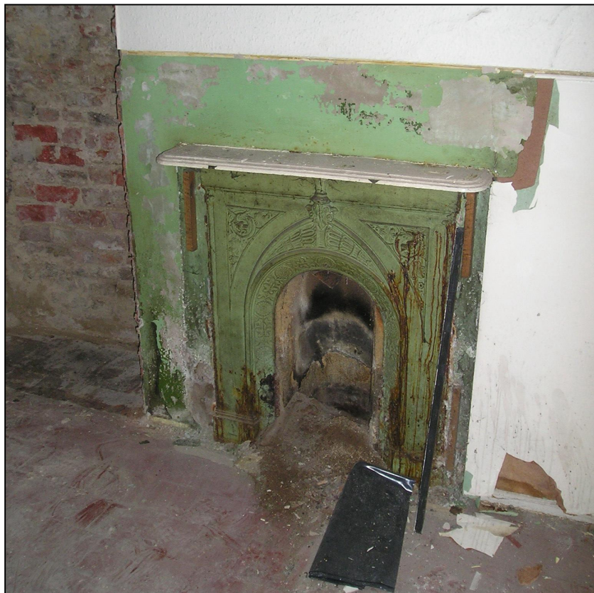
Plate 7: Fireplace in ground floor of Building A, looking NE (photo 1/23).
