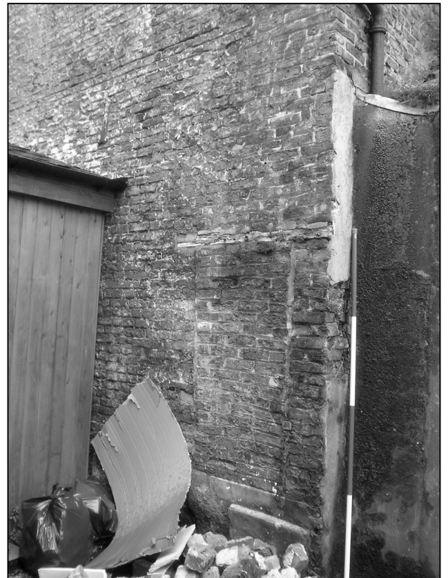
Plate 3: North elevation of Building B, showing blocked doorway, looking SE (photo 1/4).
