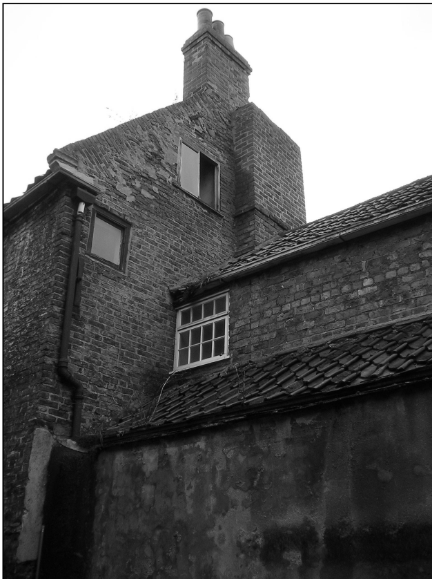
Plate 2: East gable of Building B, looking E (photo 1/2).
