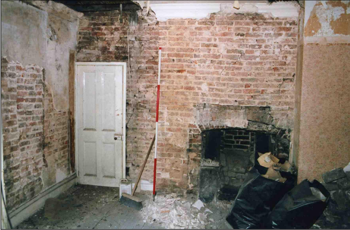
Plate 6: First floor of Building B, looking S (photo 4/10).
