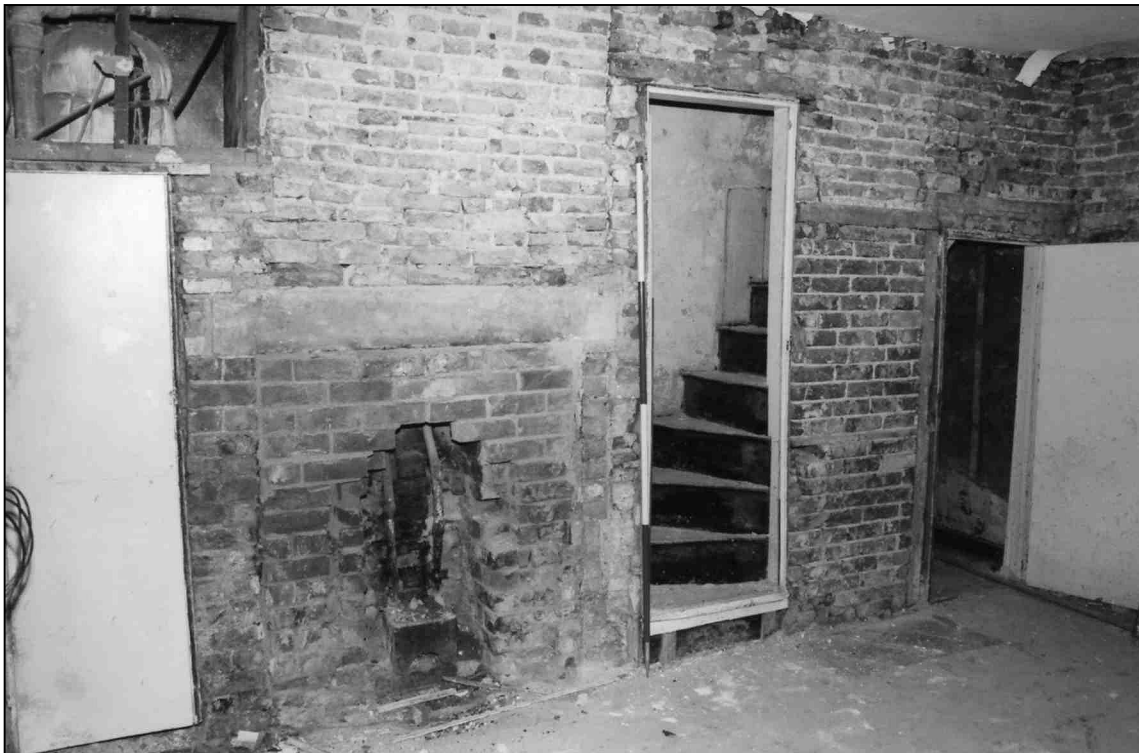
Plate 5: Ground floor of Building B, looking NW (photo 3/10).
