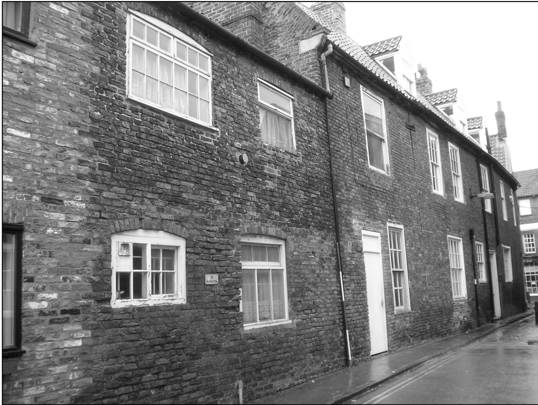
Plate 1: South elevation, looking N (photo 1/1).
