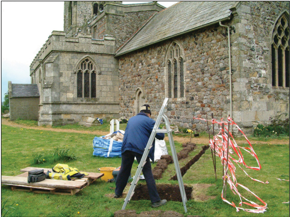
Plate 1: General view of work in progress, looking NW.
