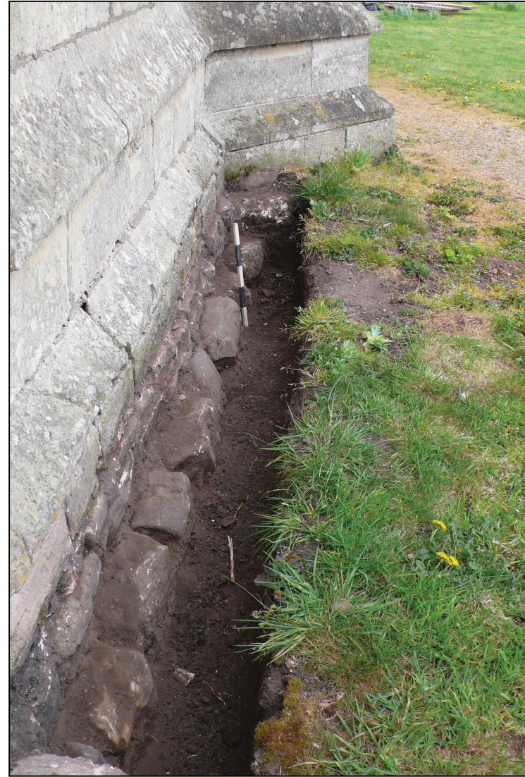
Plate 4: Exposed foundations (016) of south aisle wall, looking E.
