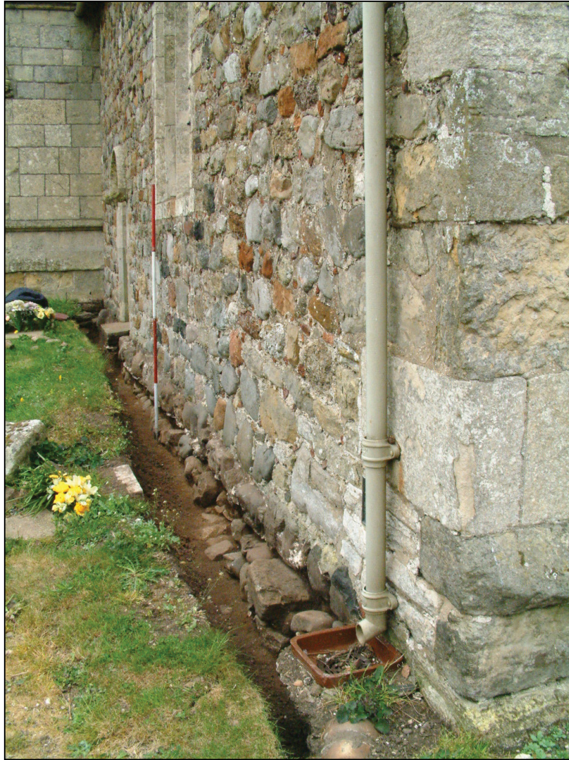
Plate 3: Exposed foundations (021) of south chancel wall, looking W.
