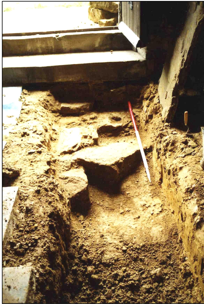
Plate 1: Foundations (004) exposed beneath west wall of tower in initial trench, looking west.
