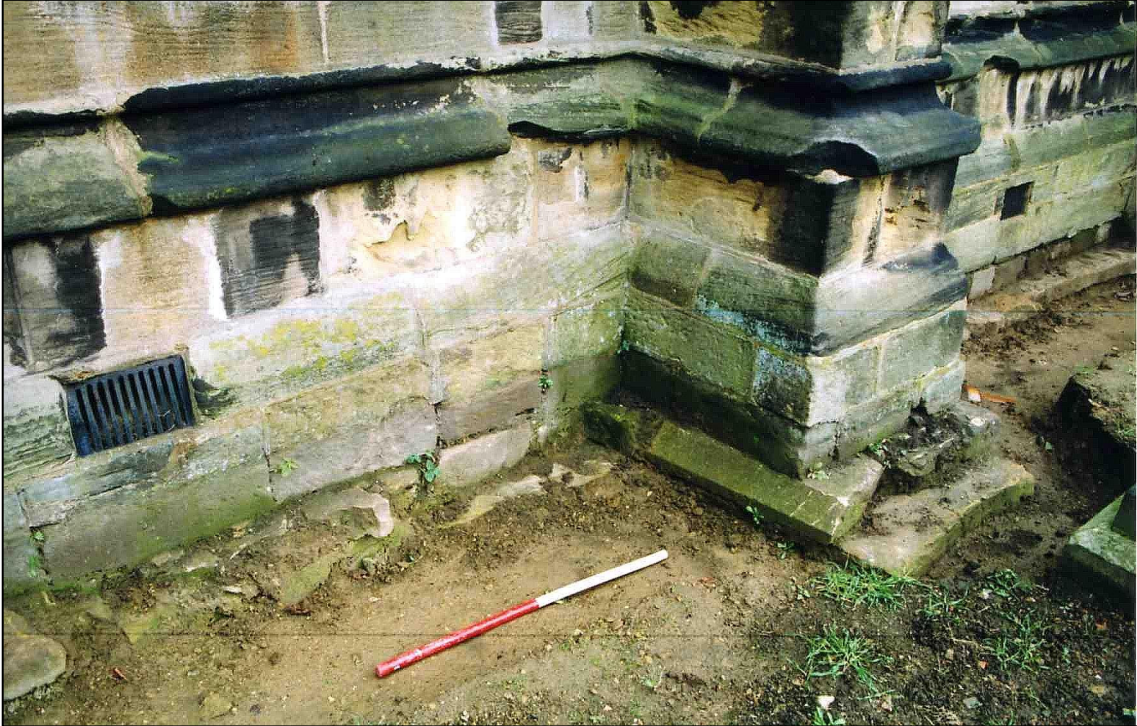
Plate 3: Footings beneath buttress C of south aisle, looking north-east.
