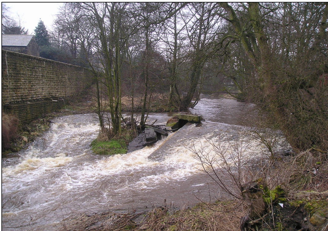
Plate 2: View of weir and overflow channel, looking west
