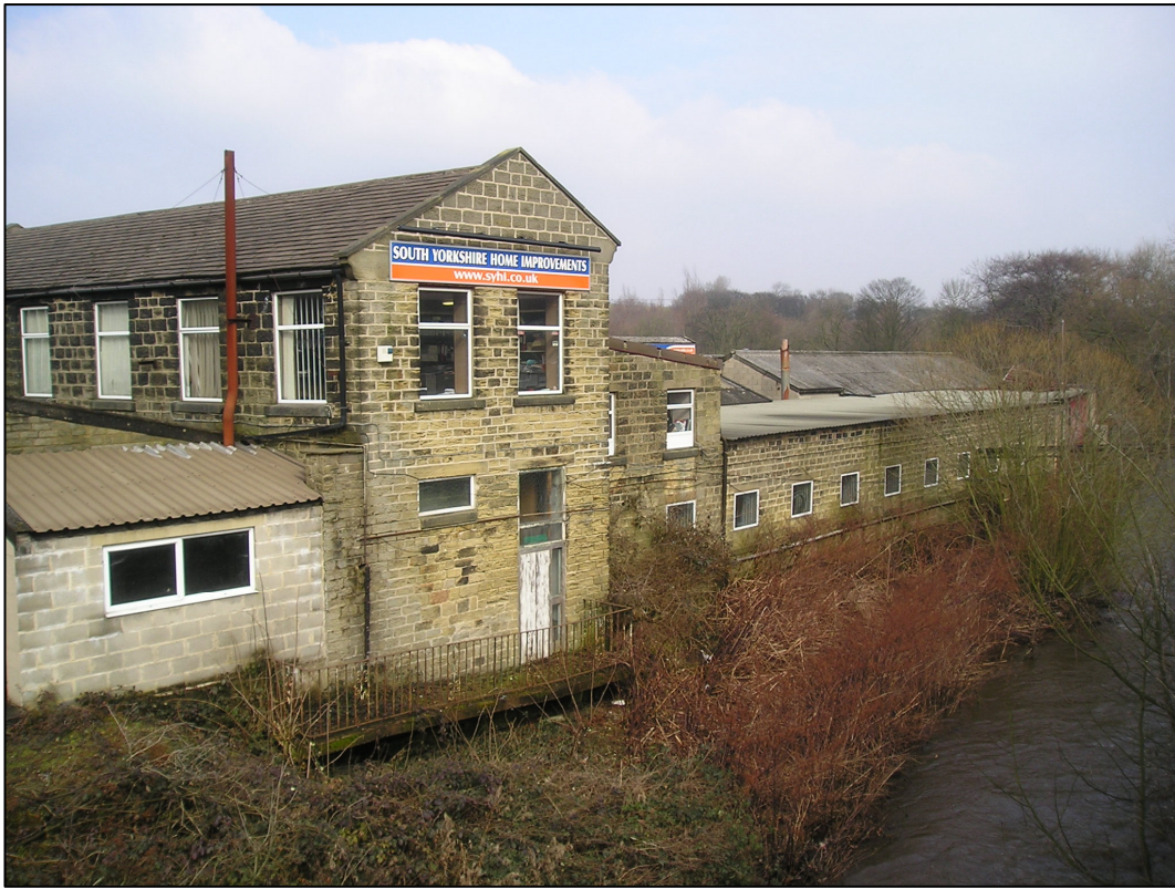
Plate 3: South side of mill complex, Buildings B, C and D, looking north-east
