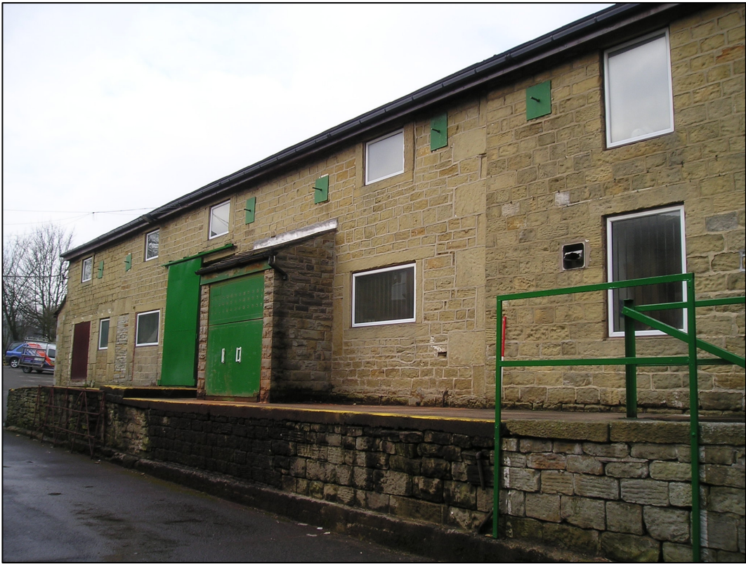
Plate 5: South side of former cottages (Building H), looking north-west
