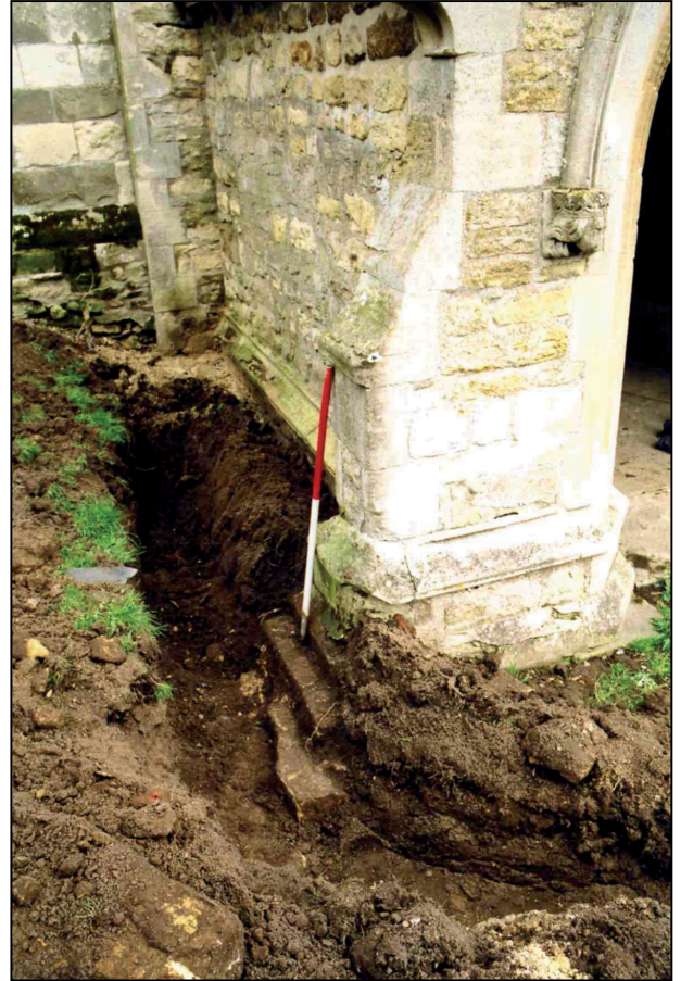
Plate 2: Trench 7 on west side of south porch, looking north.
