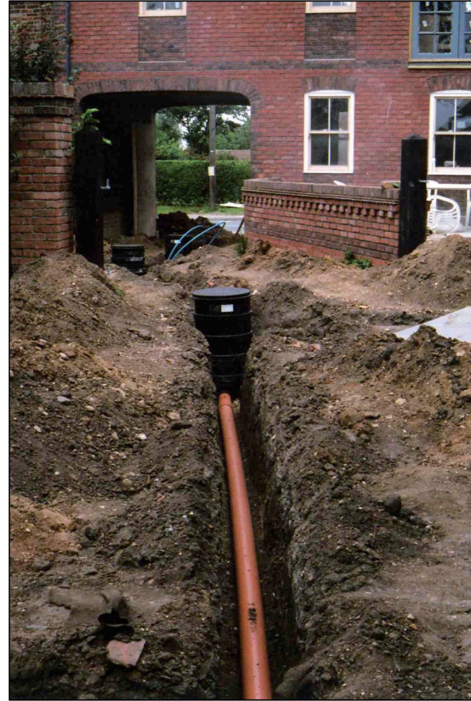
Plate 2: General view of drainage trenches, west side of site, looking north.
