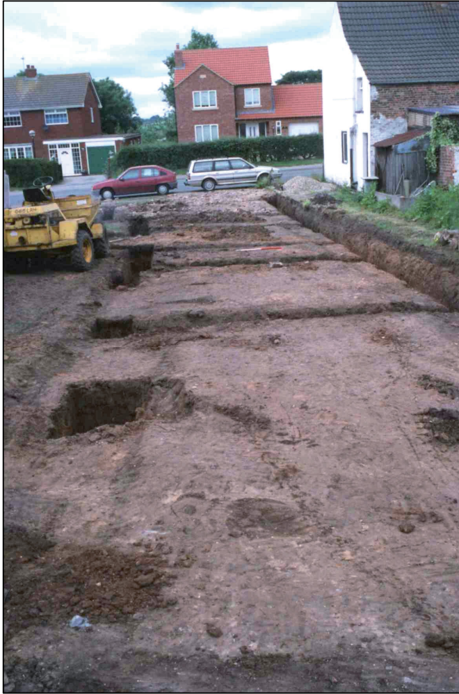
Plate 1: General view of foundation trenches, looking north.
