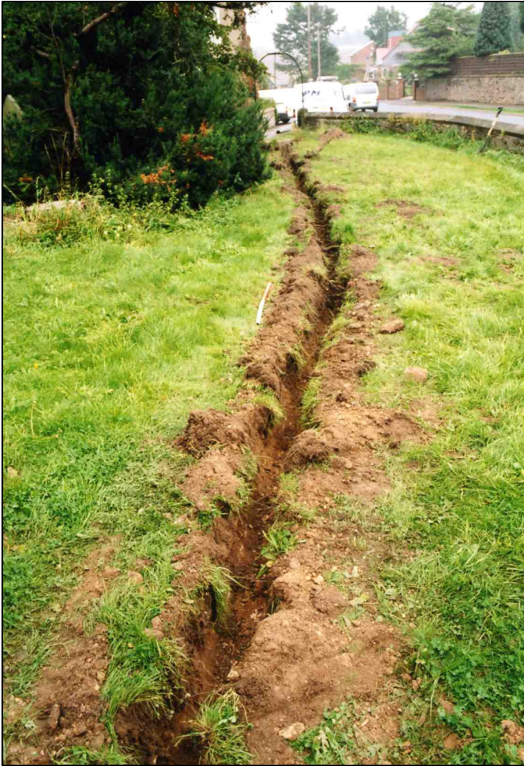
Plate 1: General view of service trench, looking north-east.
