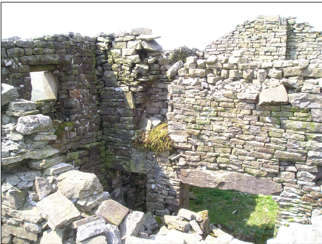
Plate 8: North side of internal wall of house (A3), looking north-west.
