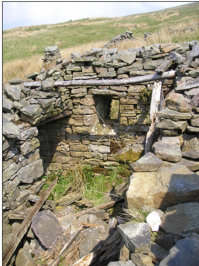
Plate 4: North cell (B2) of outshut to rear of barn, looking east.
