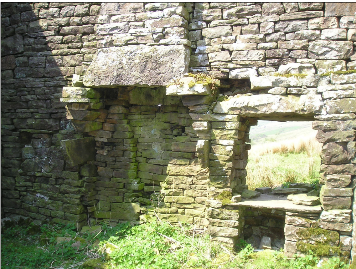
Plate 6: Fireplace and recess in north wall of house (A1), looking north-west.
