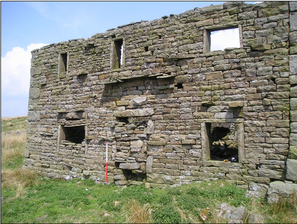
Plate 5: West (main) elevation of house (Building A), looking north-east.
