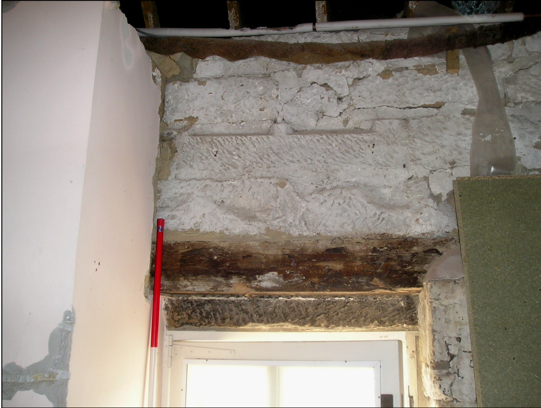
Plate 7: Reused base of 2-light mullioned window over west door in south range (B1) (photo 57).
