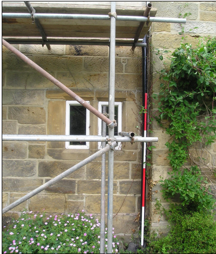
Plate 5: Later 17th century mullioned window at north end of east elevation of south range (B1) (photo 70).
