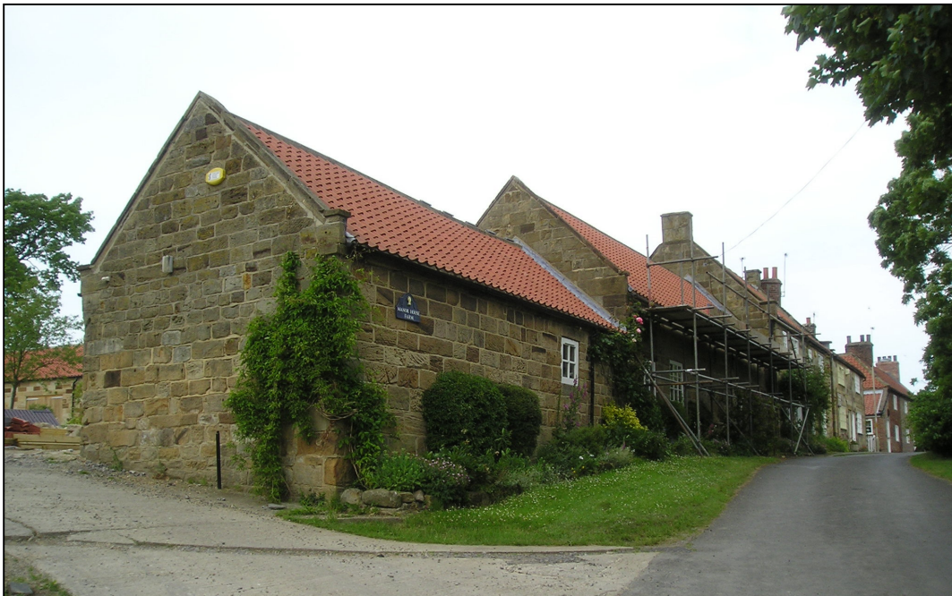
Plate 4: South gable and east side of south range (B3 and B4), looking west (photo 67).
