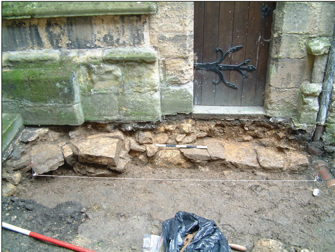
Plate 2: Exposed foundations of west wall of south chapel (006), looking E.
