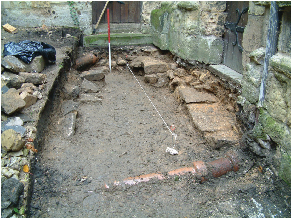
Plate 3: General view of Trench 1, looking N.
