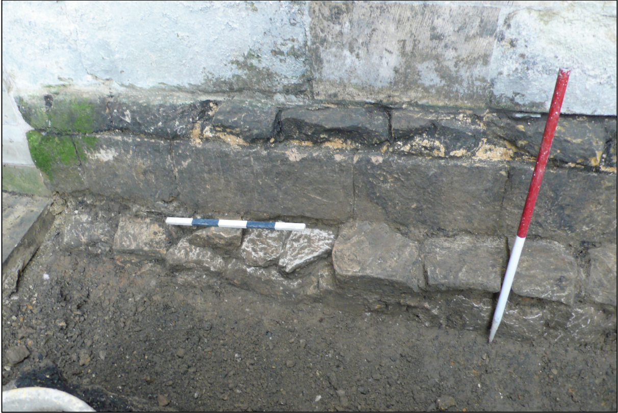
Plate 1: Exposed foundations of south chancel wall (017), looking N.
