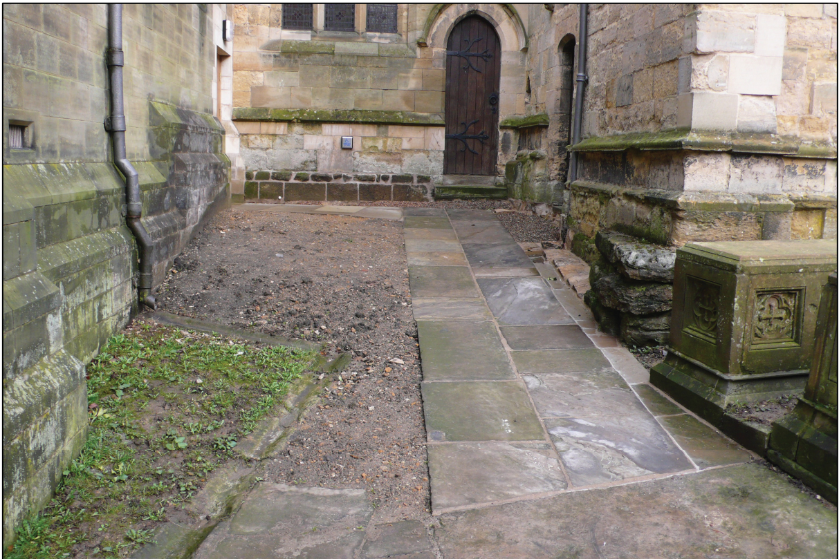
Plate 4: Completed works, looking N.
