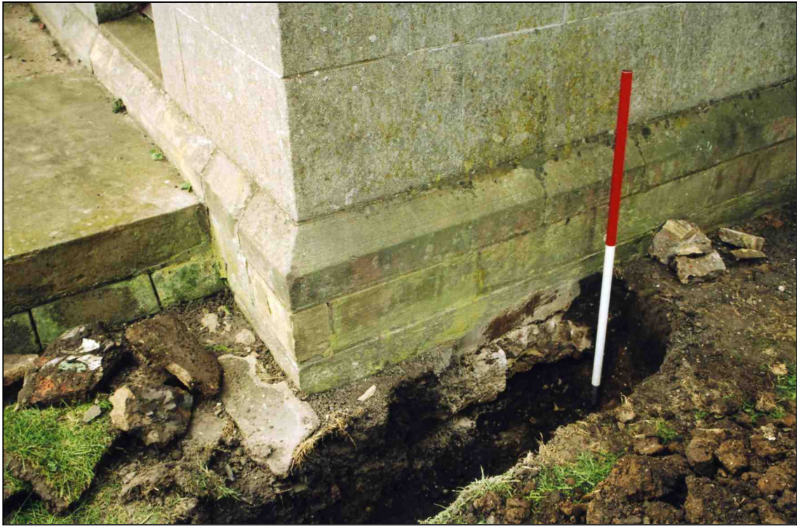
Plate 1: Footings of NE corner of vestry, looking SW.
