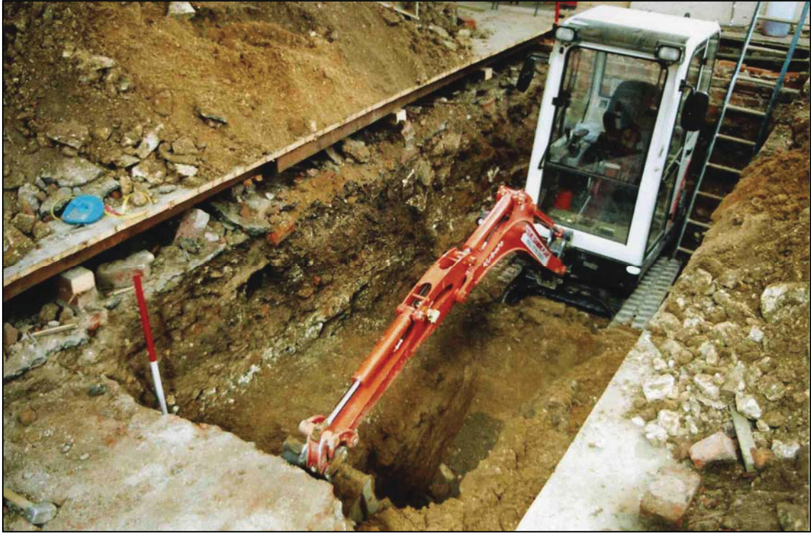
Plate 7: Test Pit 2, south facing section, looking north-east.
