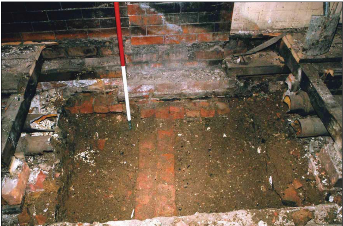
Plate 8: Test Pit 5 – brick wall (037) before removal, looking east.
