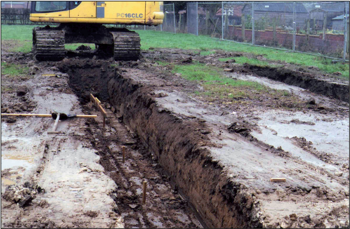
Plate 3: Plot 3, foundations under excavation, looking N.
