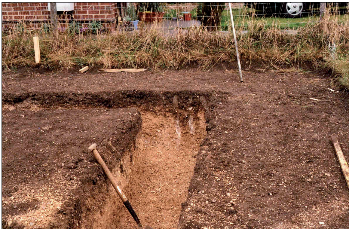
Plate 2: Plot 2, foundations under excavation, looking NNE.
