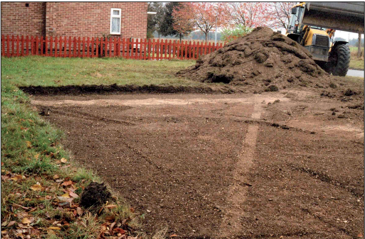
Plate 4: Plot 4, service trench (403) running through stripped area, looking S.
