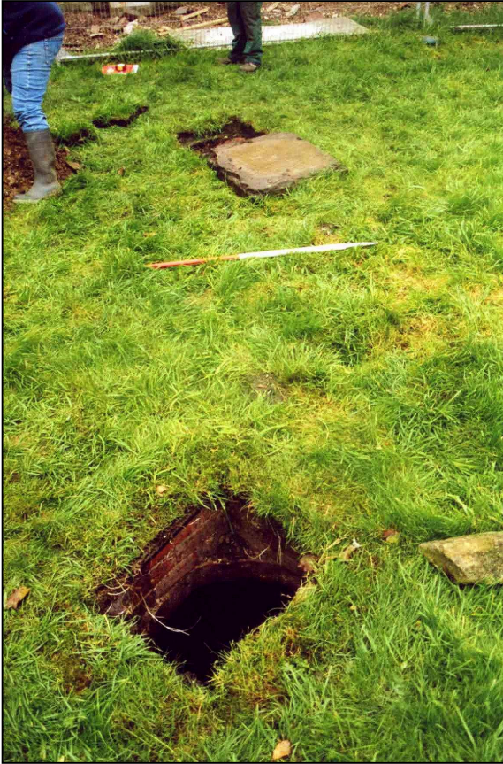
Plate 1: Openings of both underground water storage tanks, looking S.
