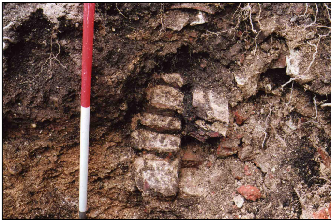
Plate 3: Wall foundation (016) with rubble infill (017) on right, looking W.
