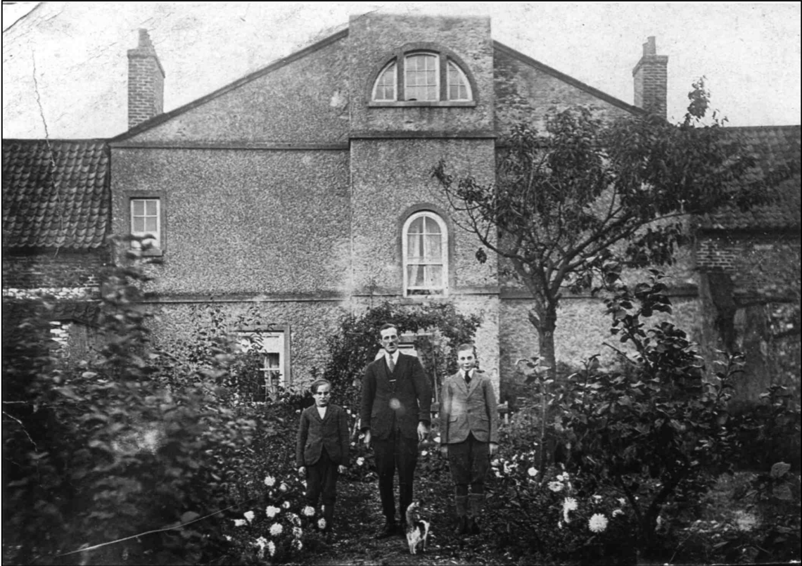
Plate 5: Early photograph (c.1900) showing south elevation of Hall Farm house.
