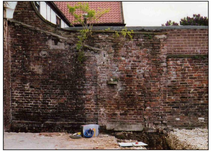
Plate 2: East garden wall (023) following demolition of coal shed, looking E.
