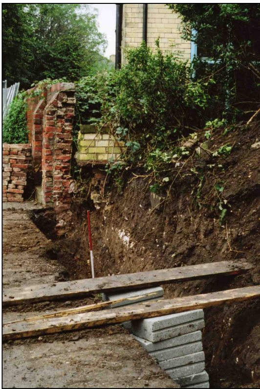
Plate 2: Work in progress, looking west.
