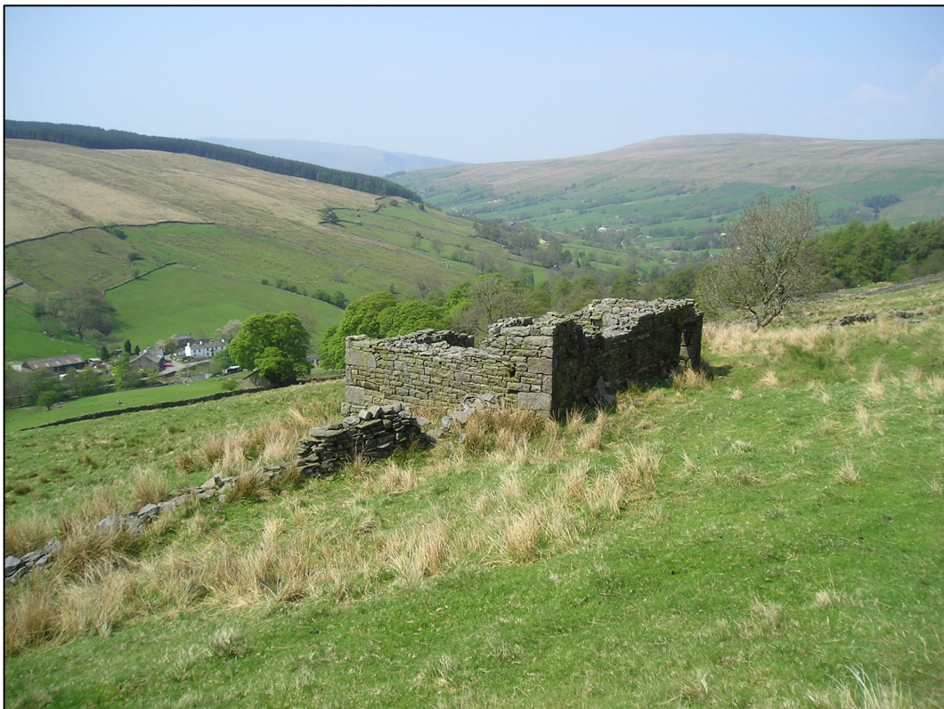
Plate 20: Ruined field barn in Jean Fields (Site 25), looking north-west.
