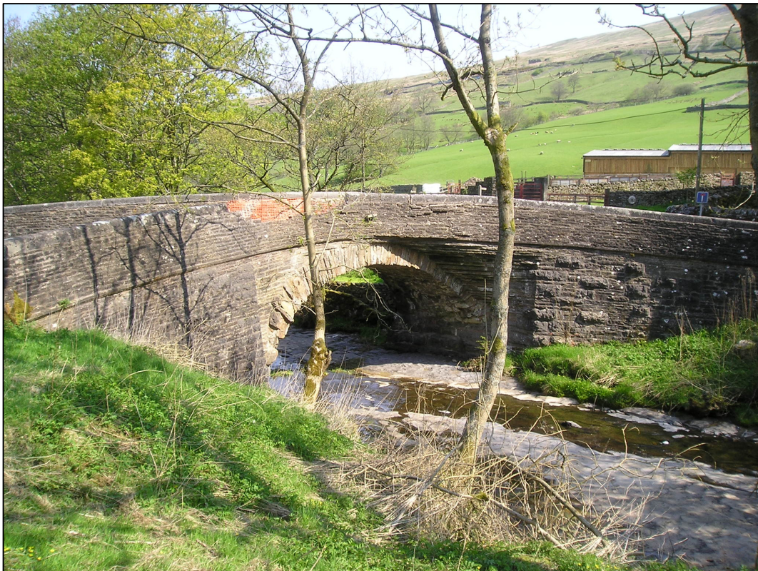
Plate 18: Stonehouse Bridge (Site 18), looking south-east.
