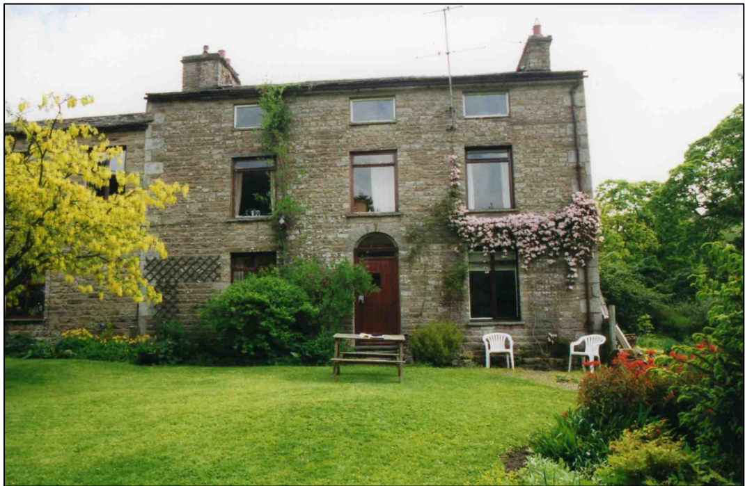
Plate 14: West elevation of Stonehouse (Site 9), looking east.
