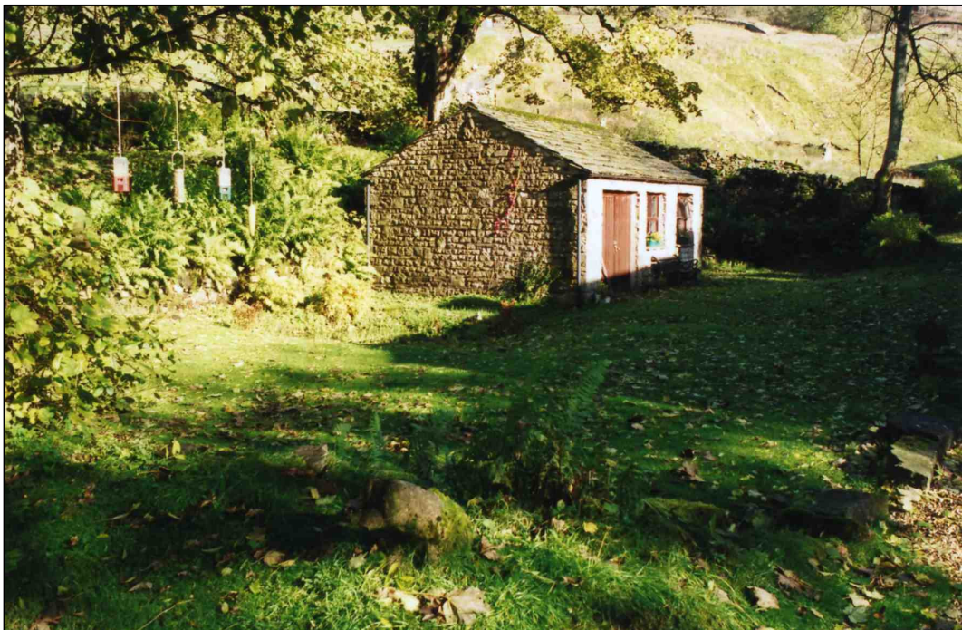
Plate 12: General view of the marble works reservoir (Site 8), looking north-east.
