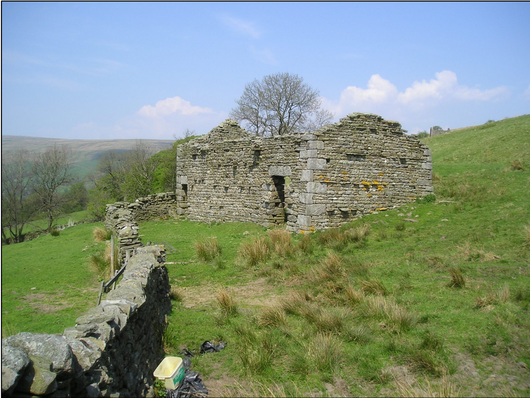
Plate 19: Ruined field barn in Jean Fields (Site 24), looking north-west.
