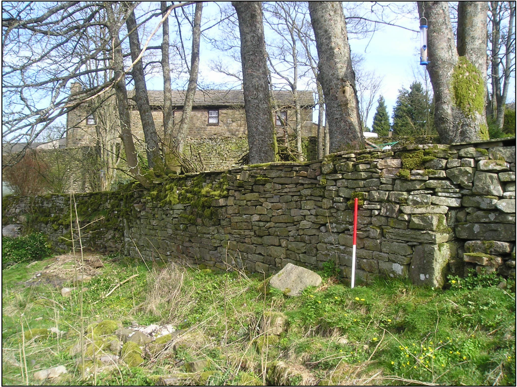
Plate 13: Remains of the west gable of High Mill (Site 7), looking north.
