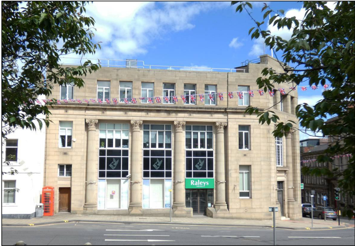
Plate 3: West elevation, looking E across Church Street (photo 662).
