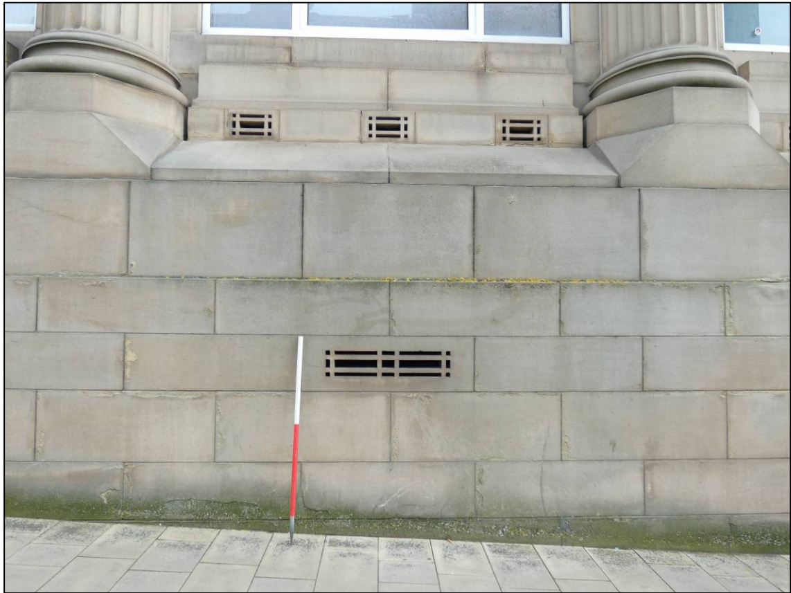
Plate 15: South elevation, vent, looking N (photo 695).
