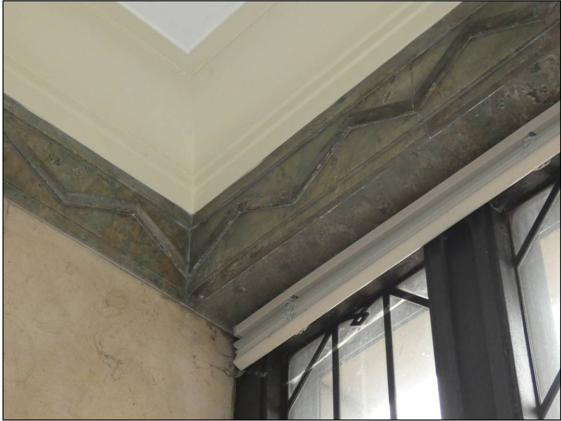
Plate 21: Lobby (GF17), original frieze and coving, looking S (photo 789).
