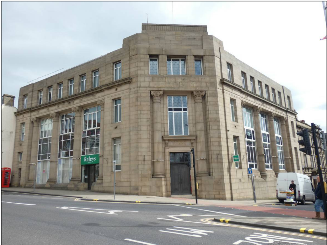
Plate 1: General view of building, looking NE (photo 677).
