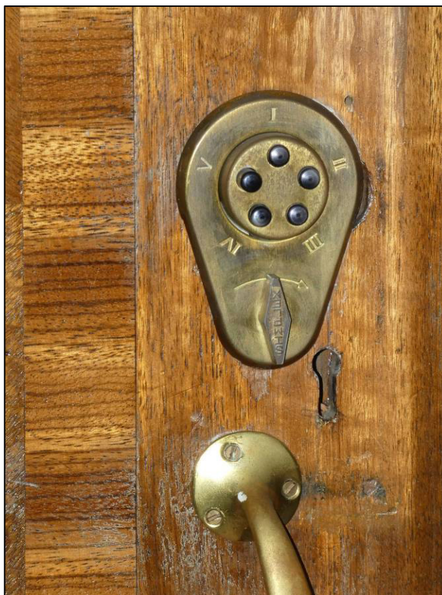
Plate 48: Machine and typists' room (GF11), combination lock on doorway, looking E (photo 845).
