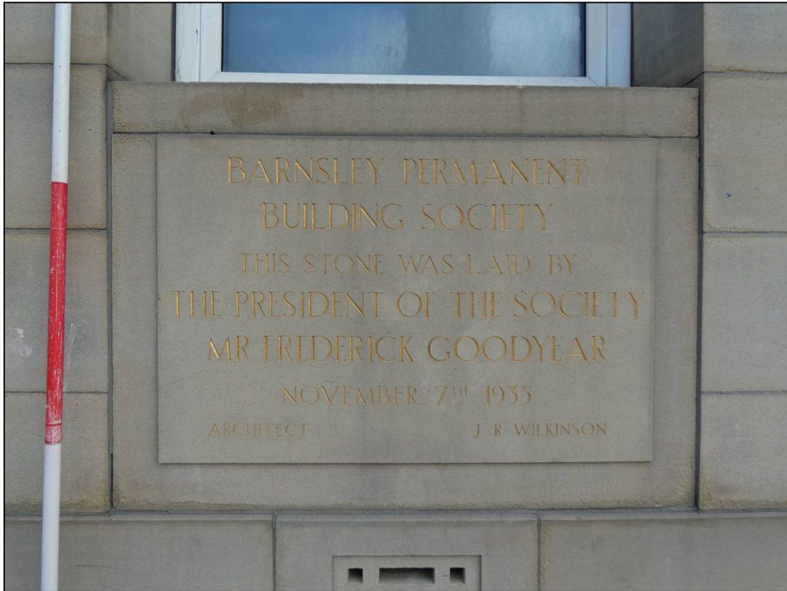
Plate 6: West elevation, foundation stone, looking E (photo 714).
