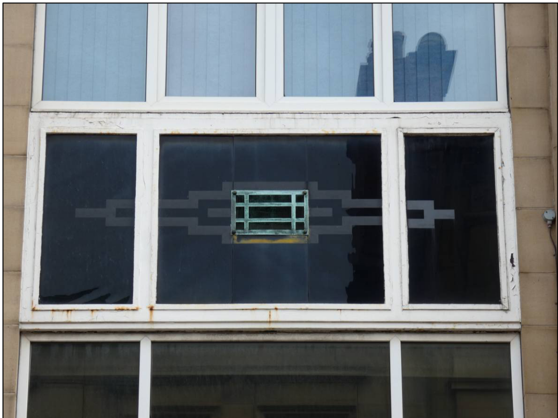
Plate 18: South elevation, window and vent detail, looking N (photo 699).
