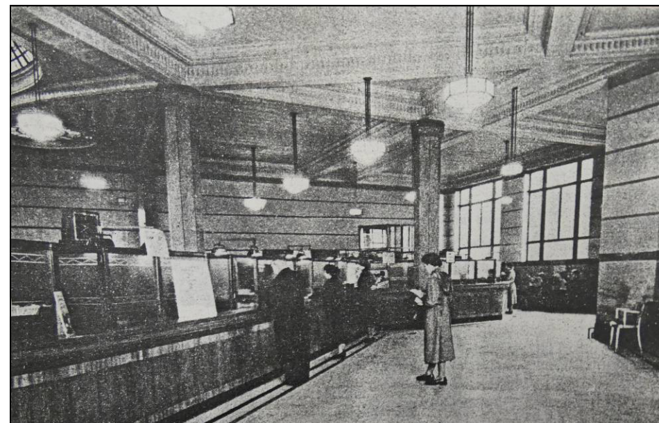
E) View of the Banking Hall (GF2), looking N.
