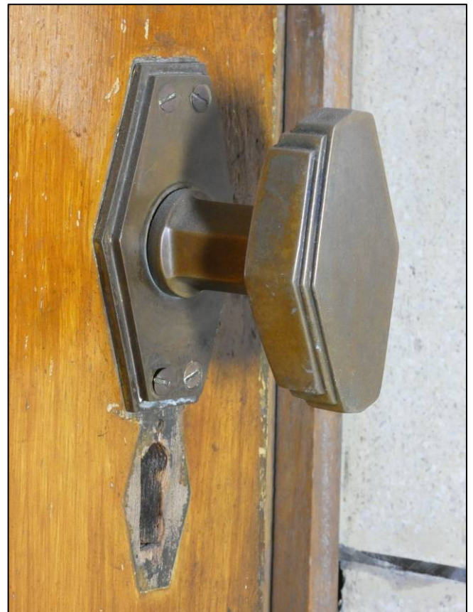
Plate 45: Staff entrance (GF6), door knob on ex-situ original door, looking SE (photo 933).
