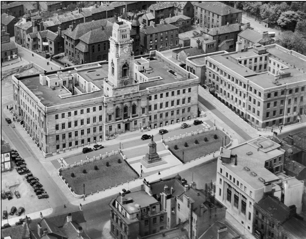
Section of aerial photograph of Barnsley town centre, taken 25th May 1938 (© Historic England Image EPW057294).
