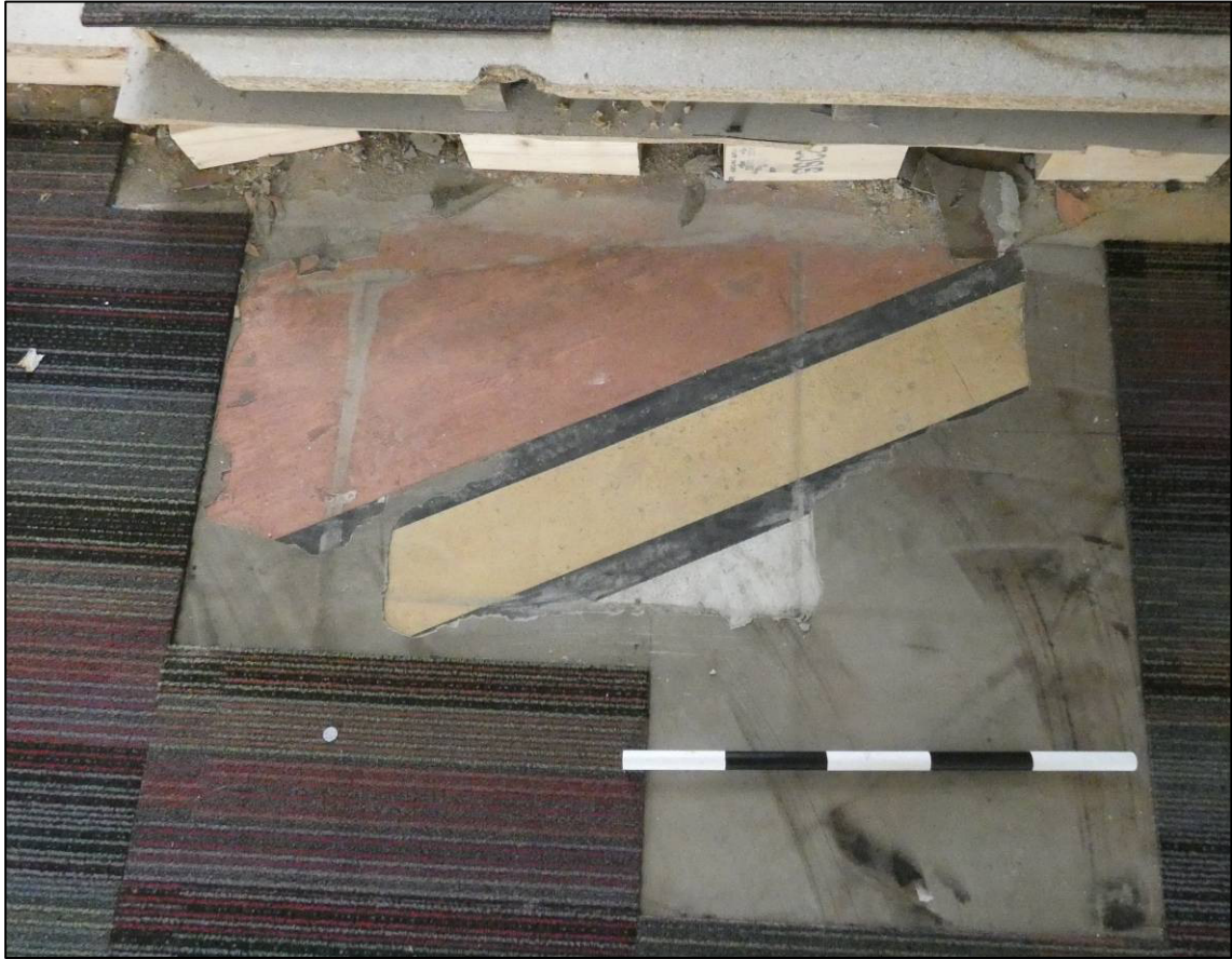
Plate 29: Modern office (GF4), detail of original terrazzo floor, looking NE (photo 913).
