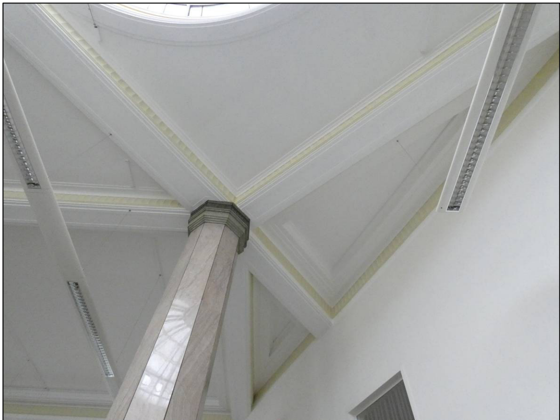
Plate 34: Banking hall and general office (GF2), ceiling panels, looking NW (photo 889).
