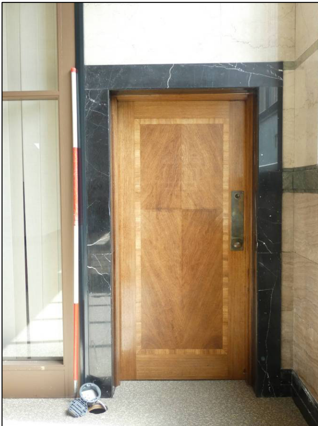
Plate 54: Assistant manager's office (GF13), doorway, looking E (photo 869).
