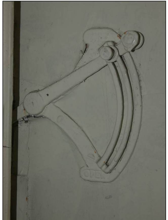
Plate 39: North-west waiting room (GF3), vent opening mechanism to west wall, looking W (photo 941).
