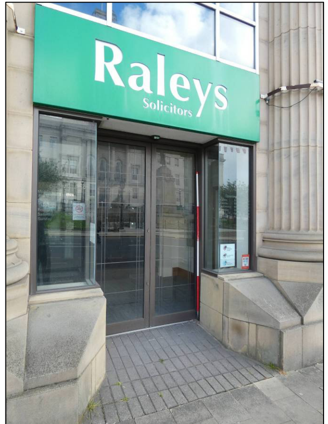
Plate 5: West elevation, inserted entrance, looking SE (photo 716).
