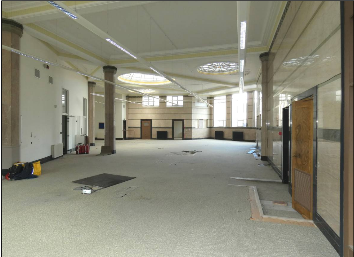
Plate 31: Banking hall and general office (GF2), looking N (photo 803).
