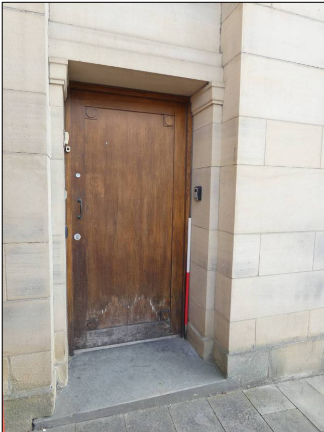
Plate 4: West elevation, staff entrance at north end, looking SE (photo 719).
