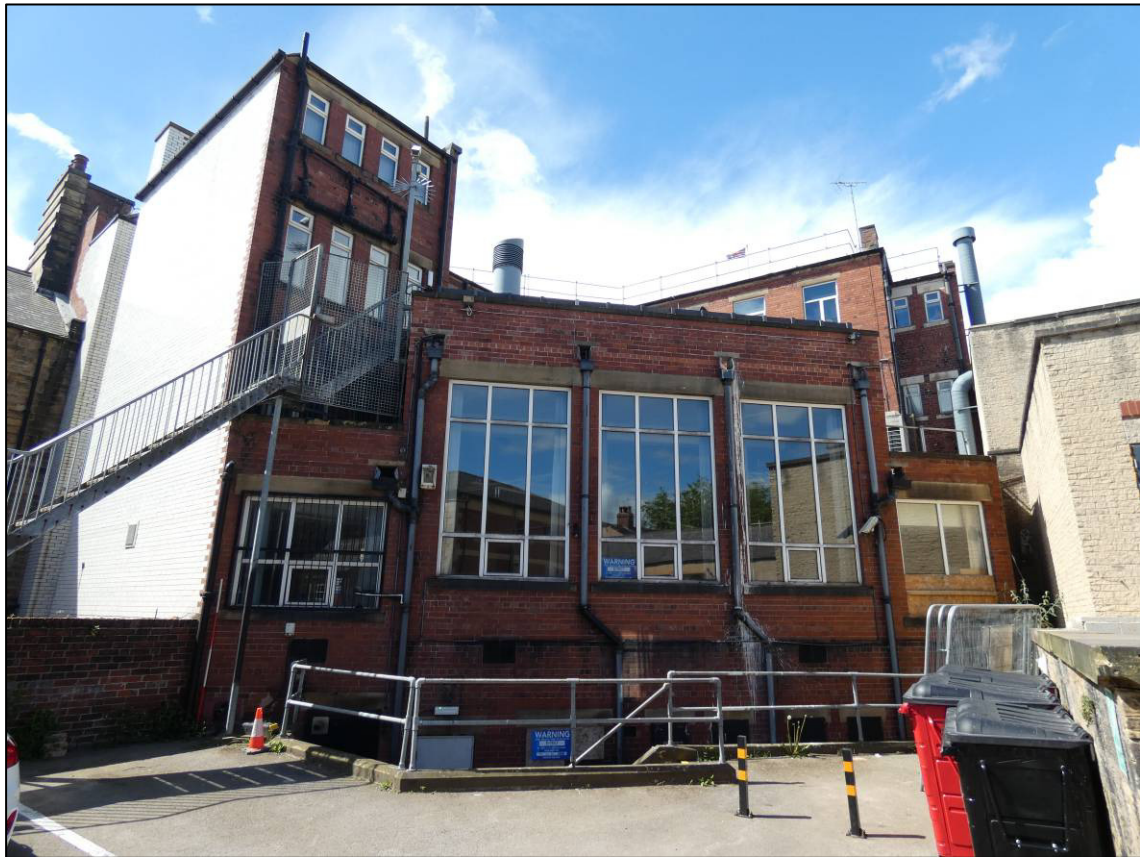
Plate 19: Rear elevation, main part, looking SW (photo 726).
