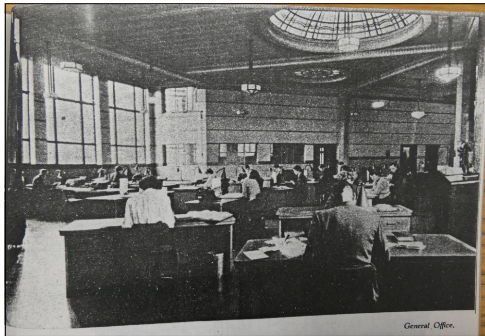
D) View of general office (GF2), looking SE.
