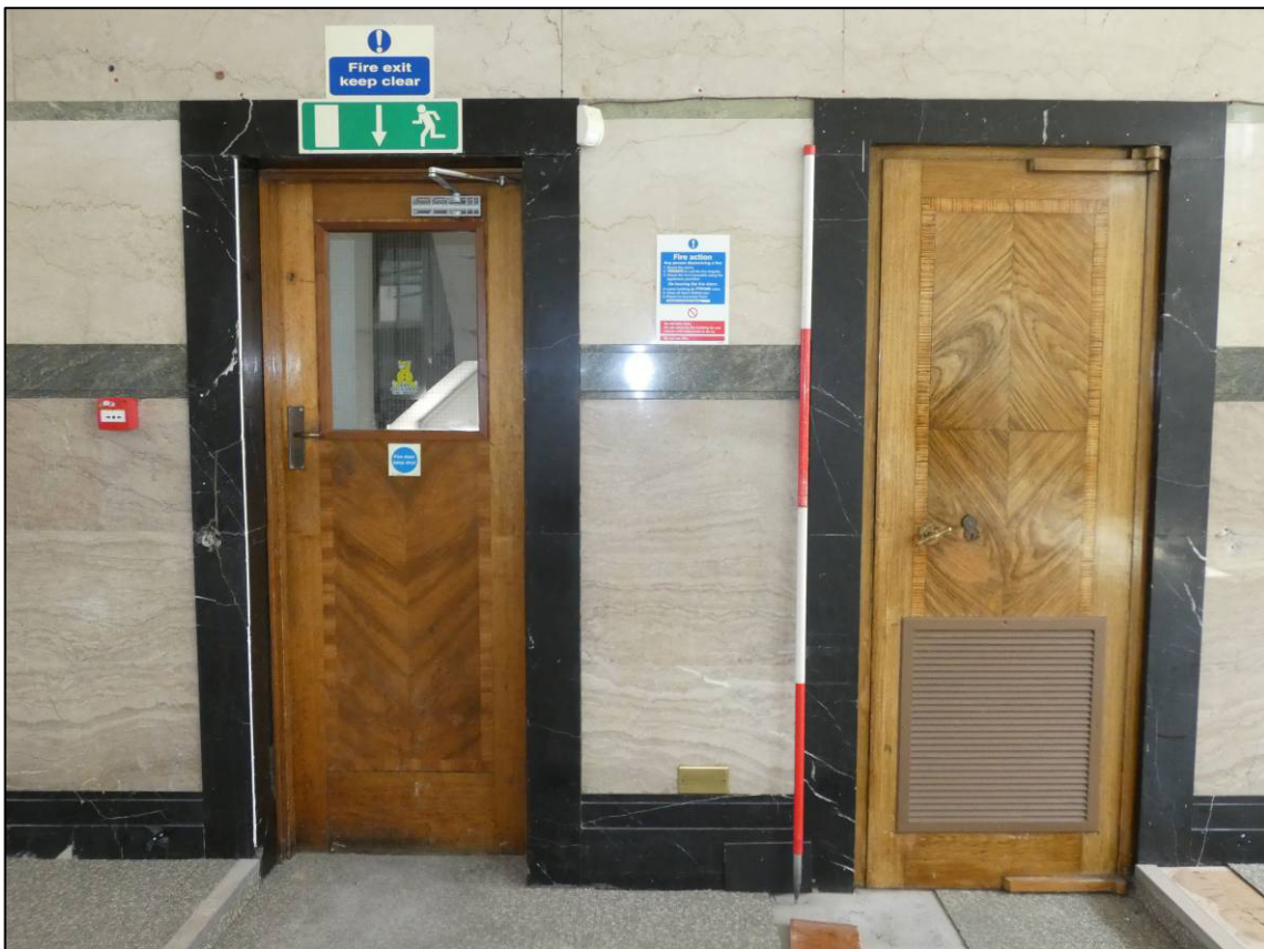
Plate 50: Banking hall and general office (GF2), south part of east wall, doorways to basement stairs (GF19 - left) and strong room (GF12 - right), looking E (photo 862).
