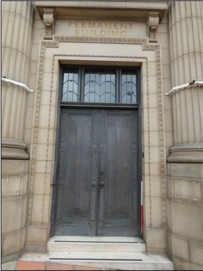
Plate 8: South-west corner, doorway to main entrance, looking NE (photo 703).
