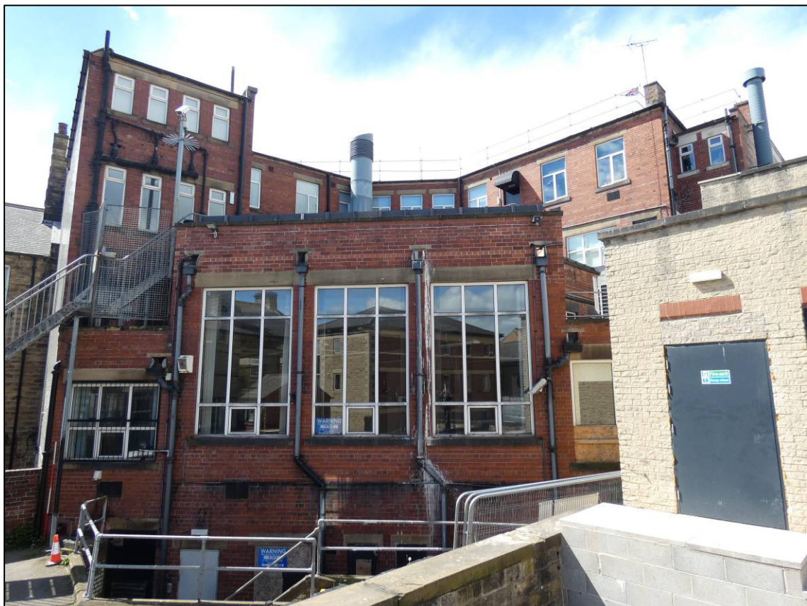
Plate 20: Rear elevation, central section, looking SW (photo 731).
