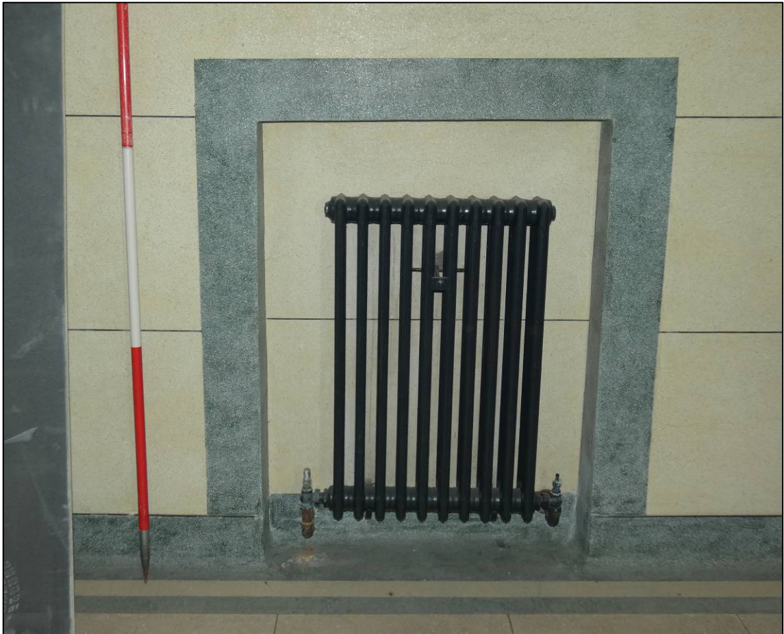
Plate 43: Staff entrance (GF6), east wall recess, looking E (photo 929).
