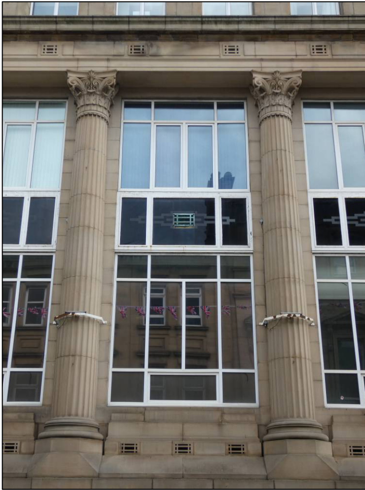
Plate 17: South elevation, window detail, looking N (photo 700).
