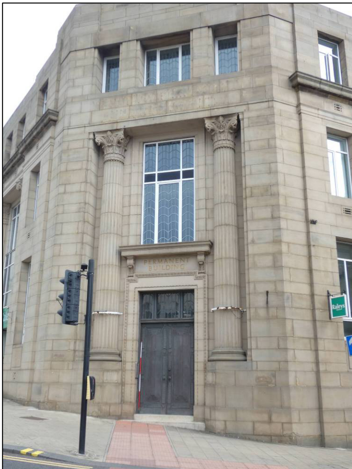
Plate 12: South-west corner, general view of main entrance, looking NE (photo 681).
