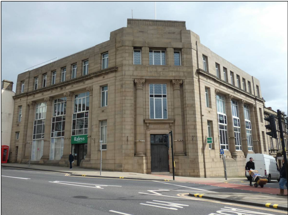
Plate 7: South-west corner, main entrance, looking NE (photo 678).
