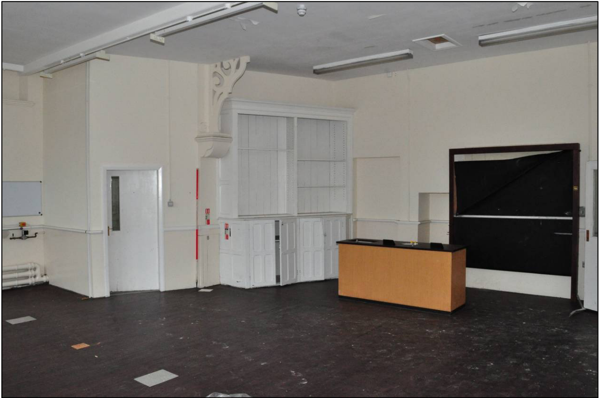
Plate 41: 1879 Board School, science classroom (1F6), showing original corbel, bracket, cupboard and recesses, looking SE (photo 2475).
