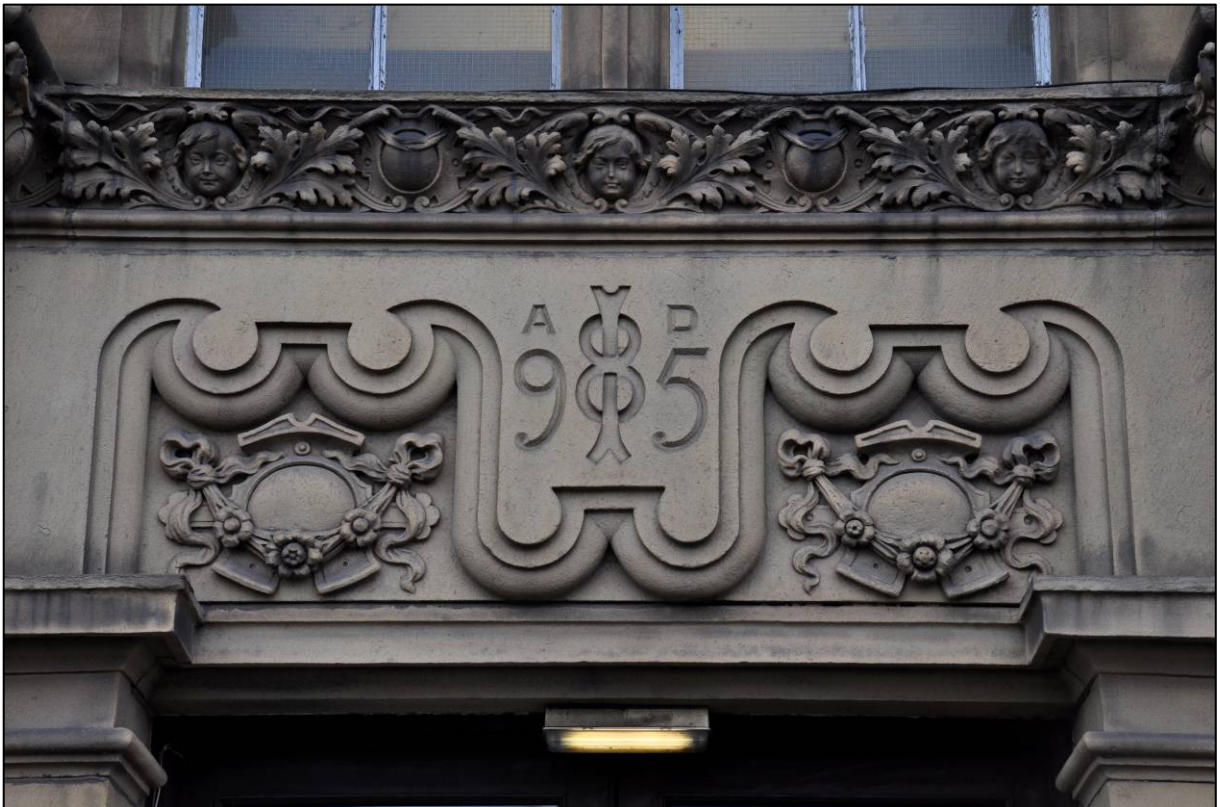
Plate 51: 1895 Higher Grade Boys' School, east elevation, ground floor entrance detail, looking W (photo 2131).
