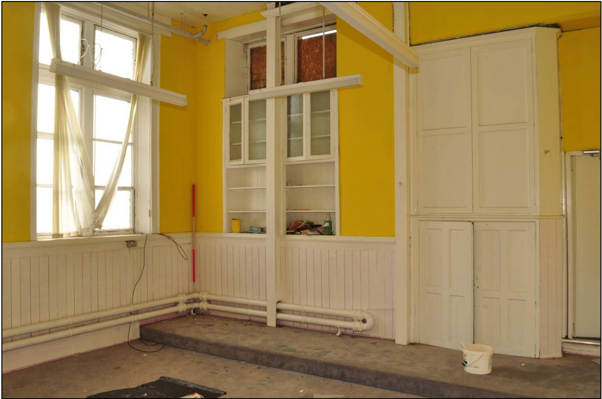
Plate 25: 1879 Board School, girls' classroom (GF12), showing original features, looking SW (photo 2415).
