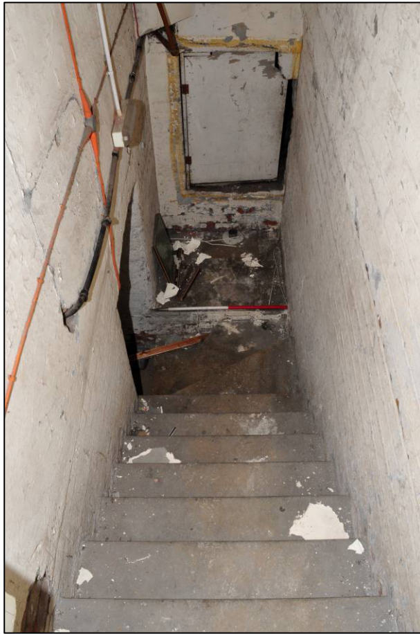
Plate 14: 1879 Board School, basement stairs (B1), looking W (photo 2382).
