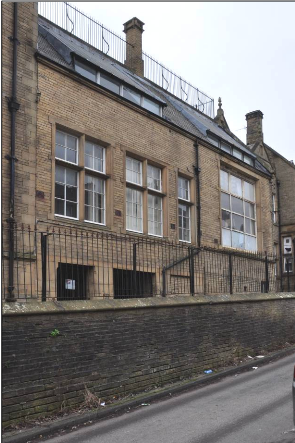
Plate 101: c.1897-99/1908 Higher Grade Girls' School, north elevation, looking SW (photo 2144).
