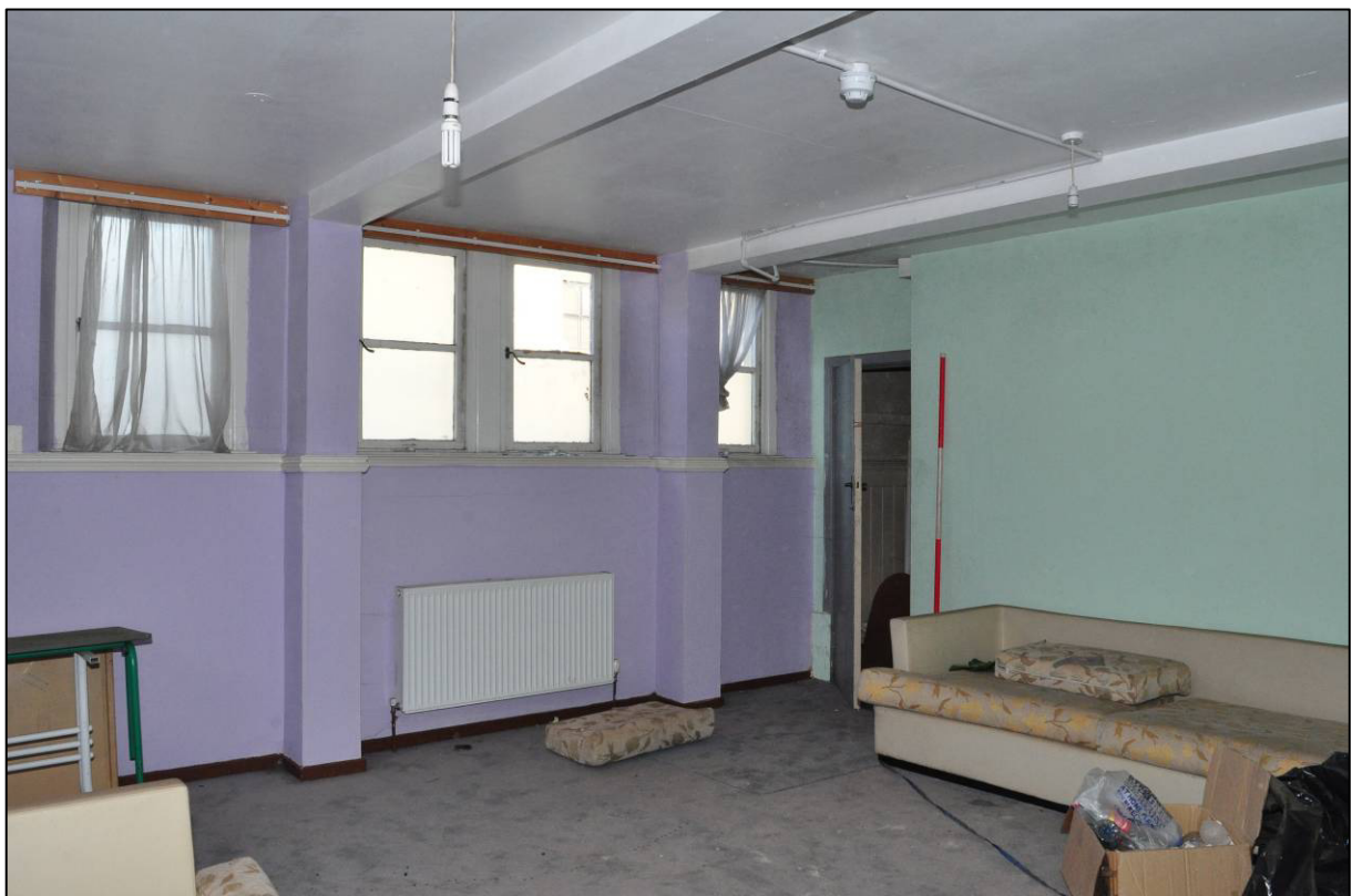
Plate 38: 1879 Board School, girls' classroom (GF1), looking NE (photo 2459).
