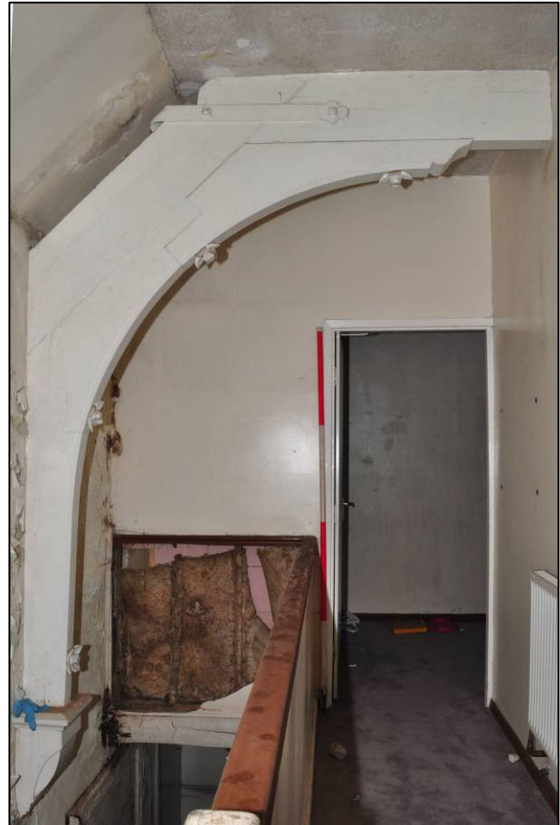
Plate 47: 1879 Board School, girls' block (1F1), truss, looking S (photo 2464).
