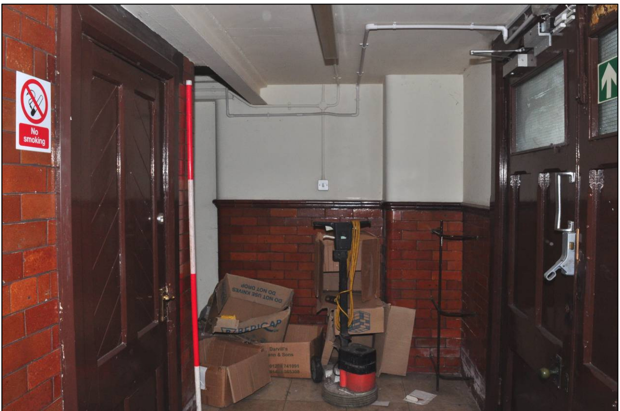
Plate 61: 1895 Higher Grade Boys' School, entrance lobby (GF14), looking N (photo 2201).
