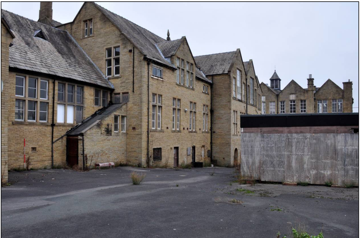
Plate 13: 1879 Board School, south elevation, and modern unit, looking E (photo 2181).
