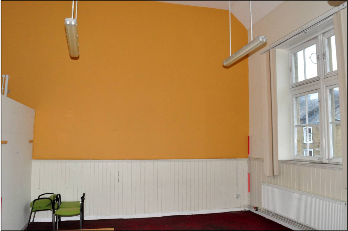
Plate 96: 1895 Higher Grade Boys' School, classroom (2F13), looking W (photo 2353).
