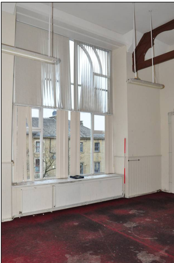
Plate 99: 1895 Higher Grade Boys' School, classroom (2F14), window to north wall, looking NE (photo 2360).
