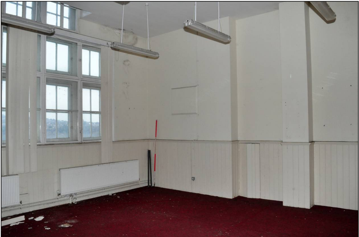
Plate 85: 1895 Higher Grade Boys' School, classroom (2F4), tongue and groove panelling and wall vents, and access to space under seating, looking SE (photo 2322).
