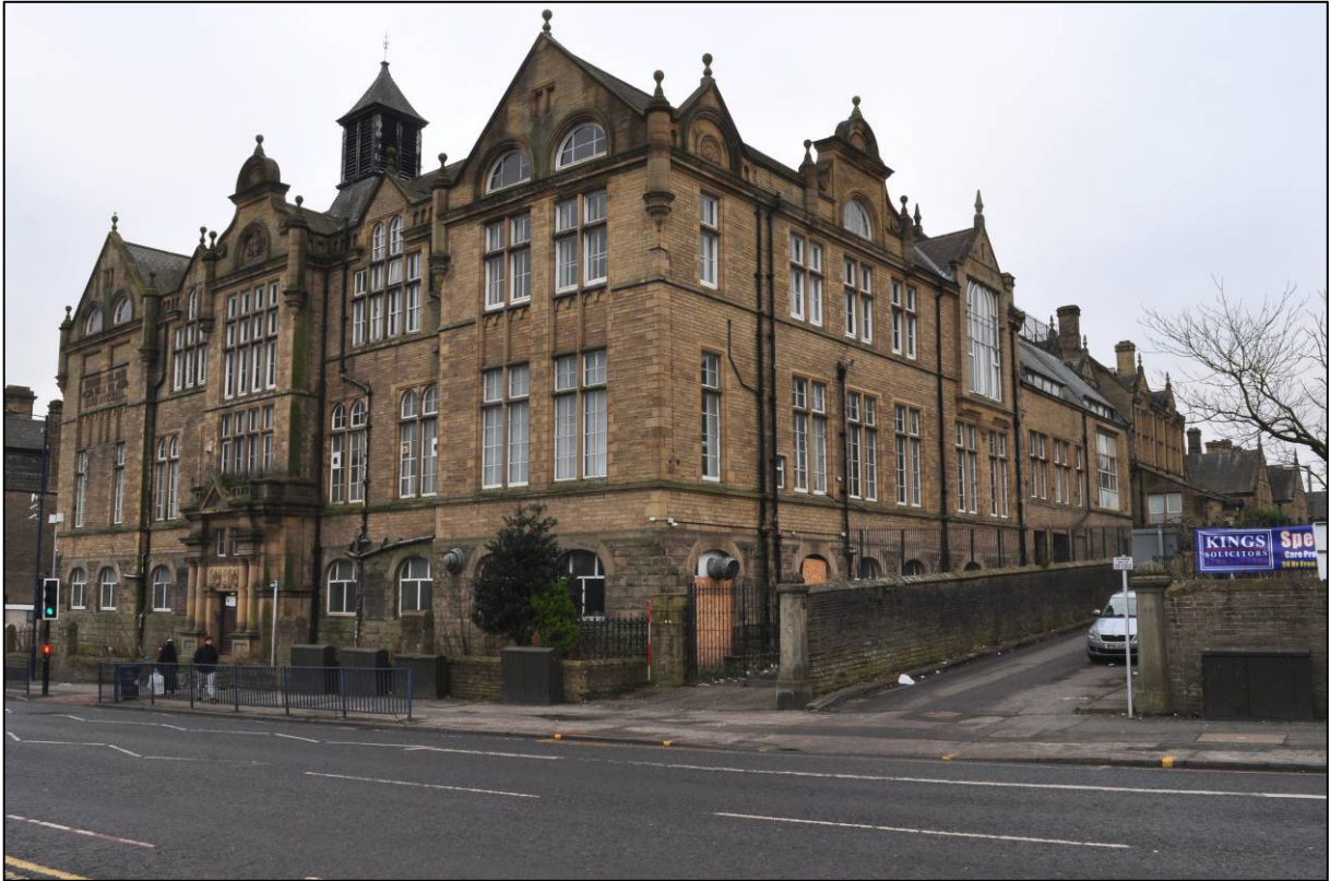
Plate 1: 1895 Higher Grade Boys' School, general view from Manningham Lane, looking SW (photo 2103).
