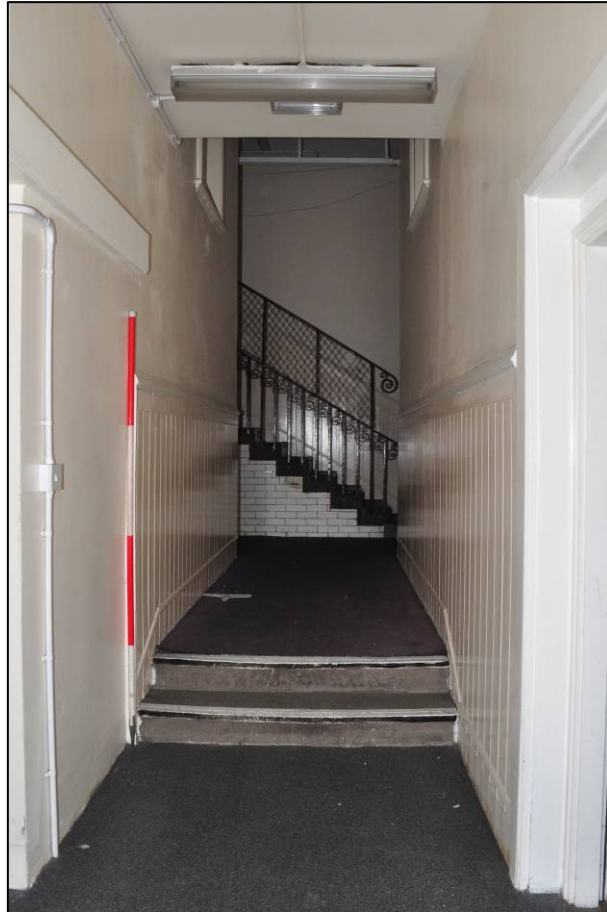
Plate 30: 1879 Board School, entrance corridor (GF9), looking S (photo 2430).
