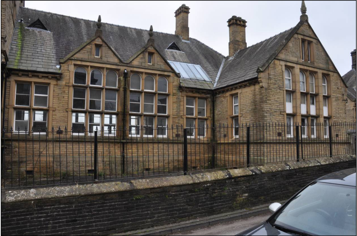
Plate 7: 1879 Board School, north elevation of girls' block, looking S (photo 2155).
