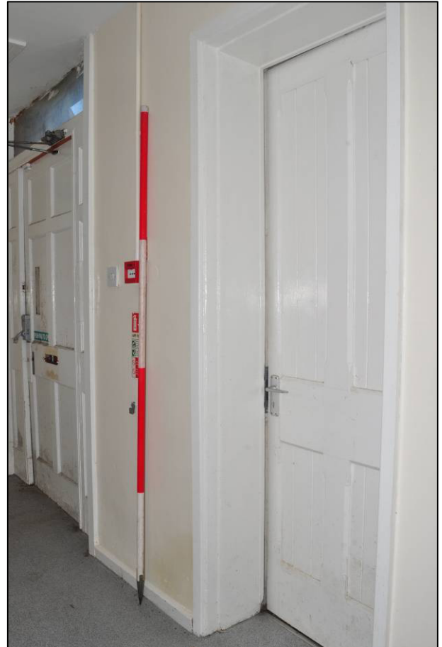
Plate 37: 1879 Board School, girls' entrance lobby (GF2), original doors, looking W (photo 2458).
