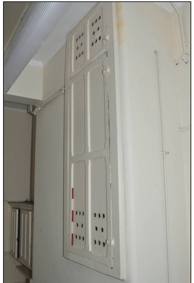
Plate 114: c.1897-99 Higher Grade Girls' School, classroom/dining room (1F28), possible vent cover to chimney breast to west wall, looking SW (photo 2274).
