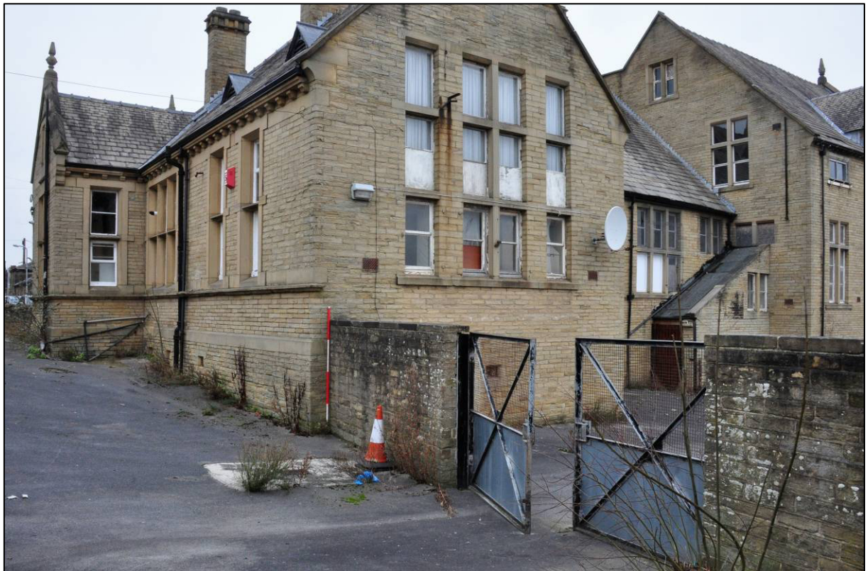
Plate 11: 1879 Board School, south elevation of girls' block, looking NE (photo 2184).
