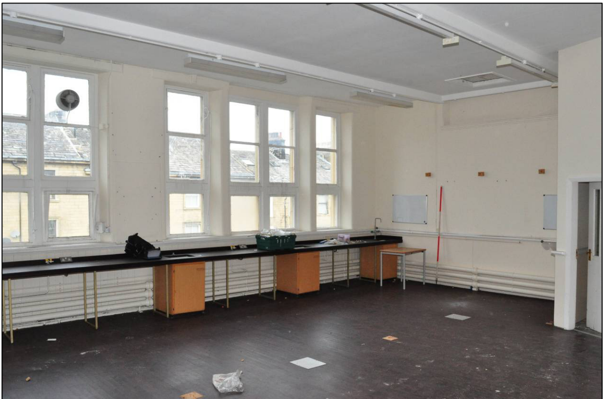
Plate 40: 1879 Board School, science classroom (1F6), looking NE (photo 2476).
