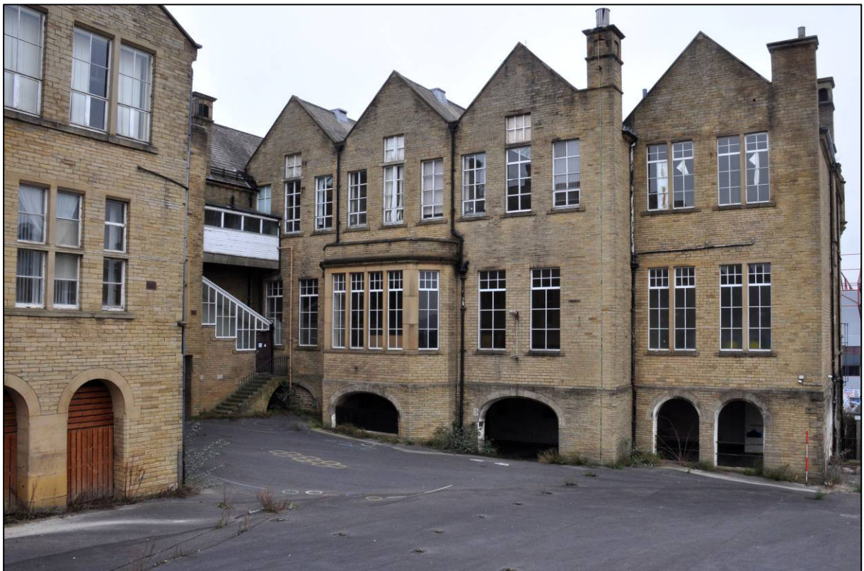
Plate 59: 1895 Higher Grade Boys' School, west elevation, looking E (photo 2167).
