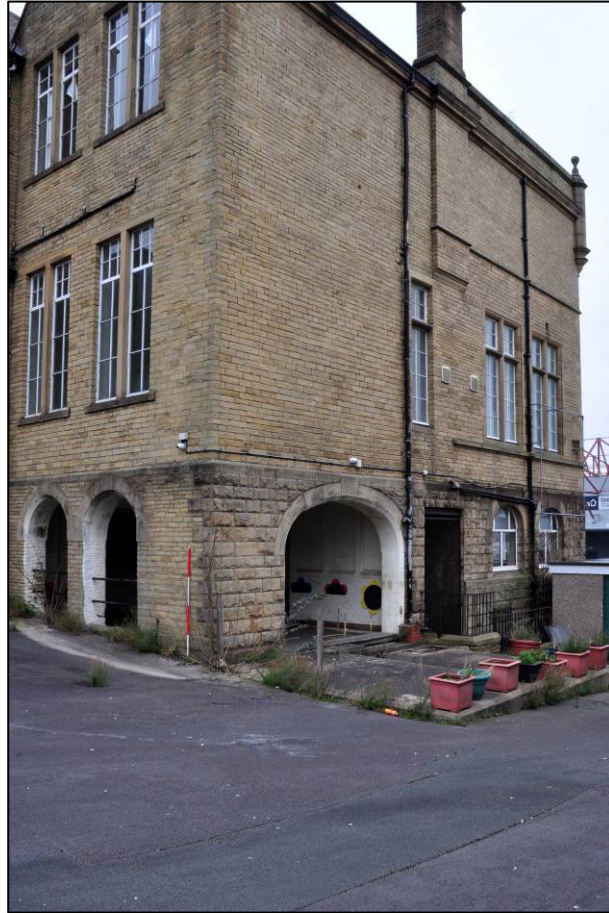
Plate 58: 1895 Higher Grade Boys' School, south elevation, looking NE (photo 2162).
