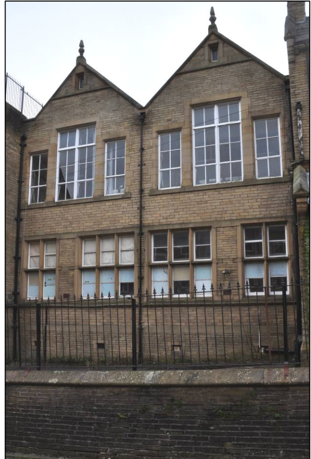
Plate 102: 1879 Board School (boys' block) with 1908 Higher Grade Girls' School extension, north elevation, looking S (photo 2149).
