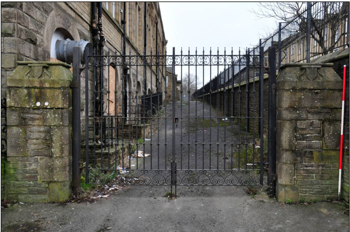
Plate 2: 1895 Higher Grade Boys' School, east elevation, replacement north yard gates on Manningham Lane, looking W (photo 2138).
