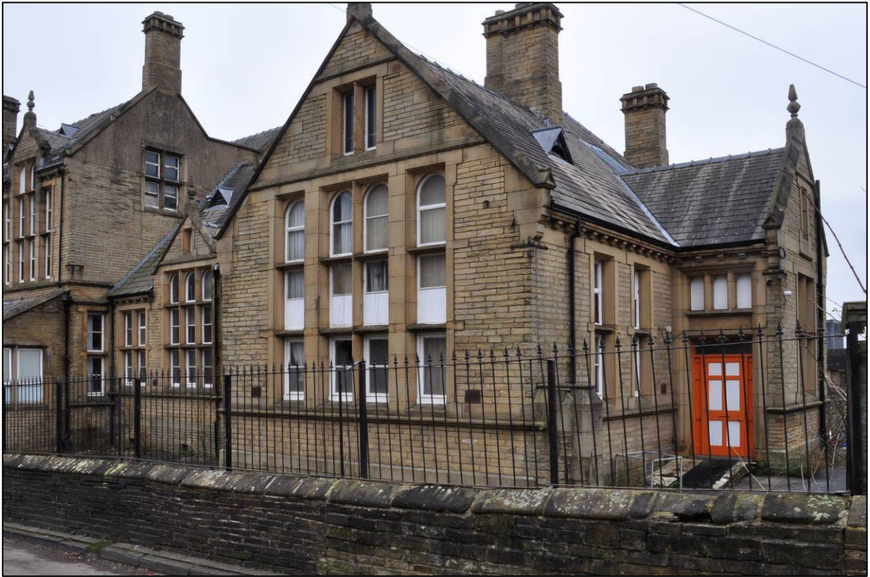
Plate 10: 1879 Board School, north elevation of girls' block, looking SE (photo 2157).
