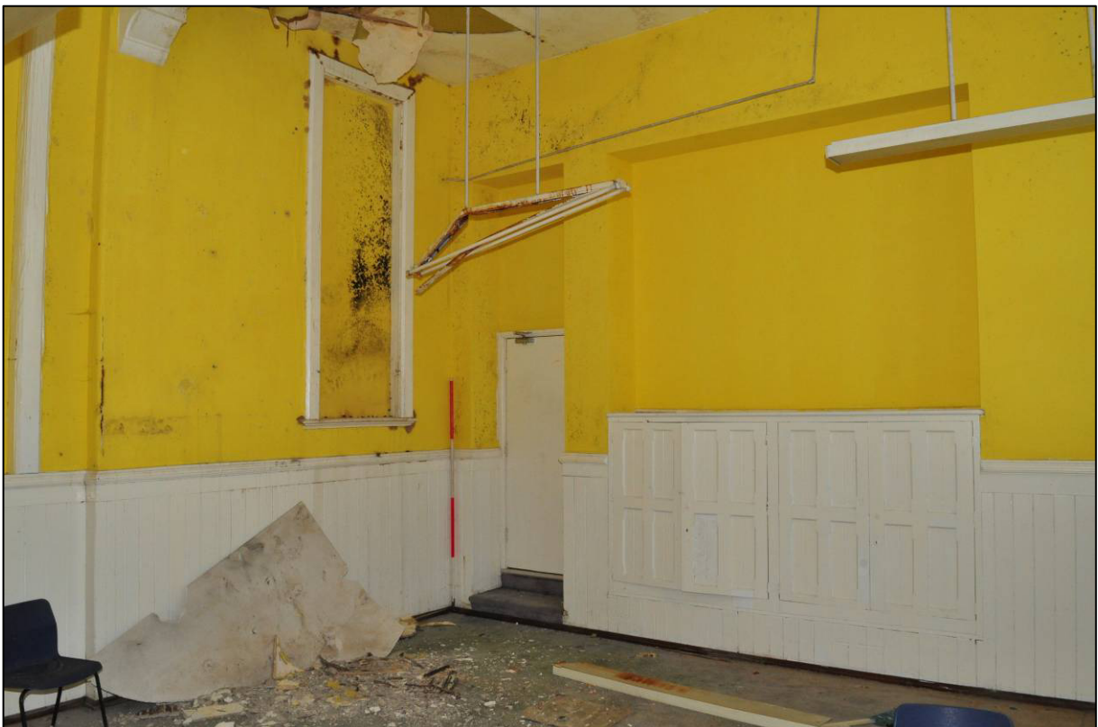
Plate 31: 1879 Board School, girls' classroom (GF8), showing original features, looking SW (photo 2433).
