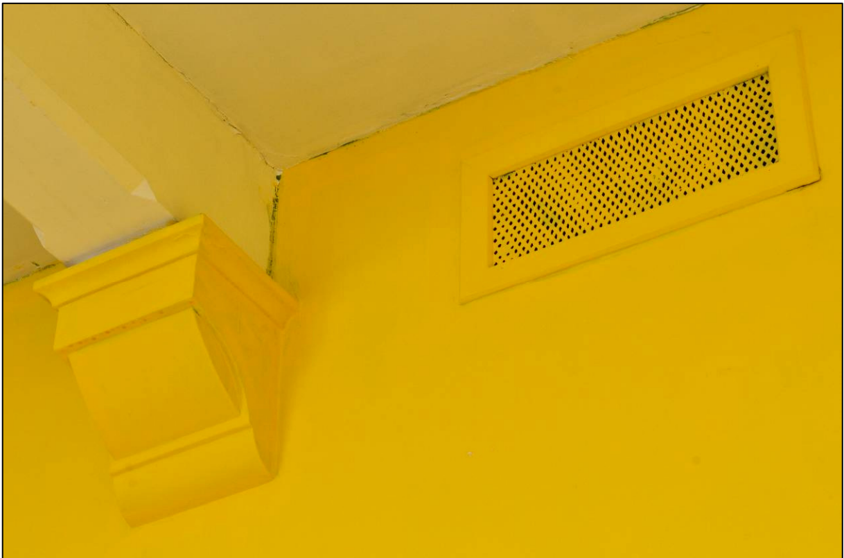
Plate 26: 1879 Board School, girls' classroom (GF12), corbel and vent, looking NE (photo 2426).
