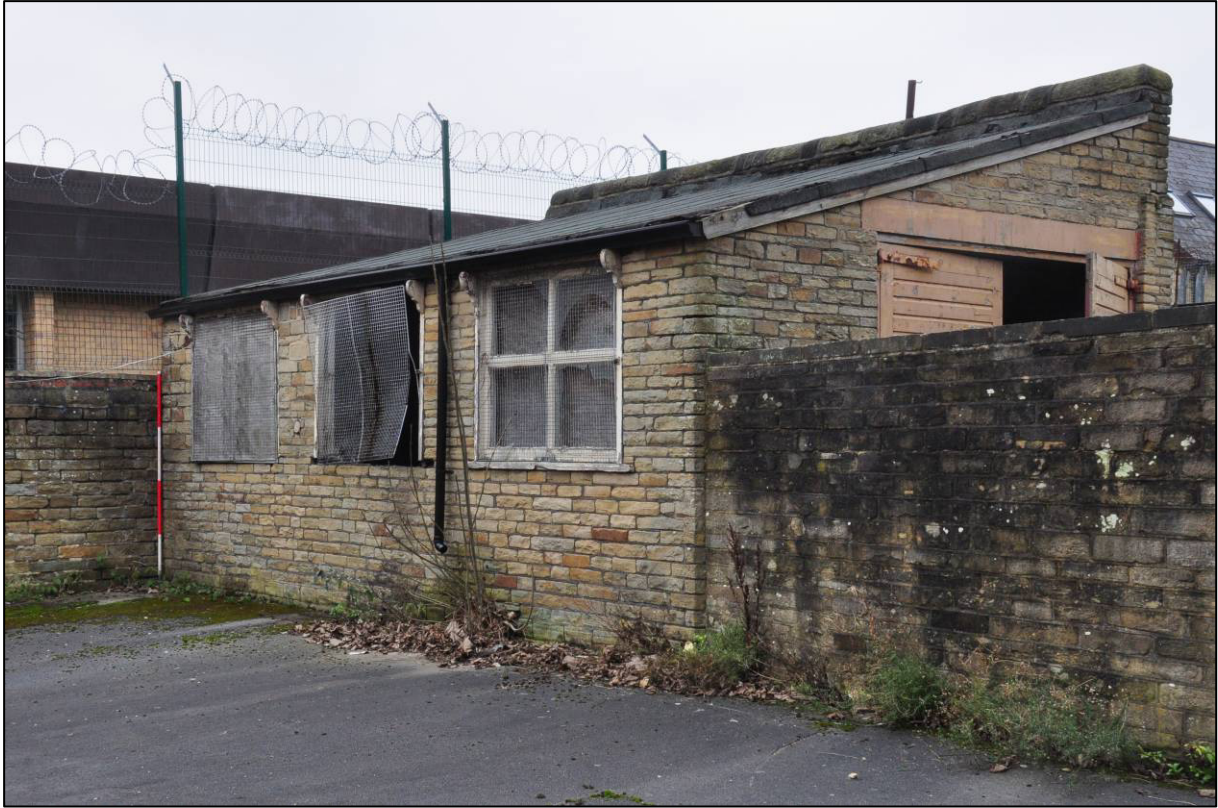
Plate 5: 1922-34 shed to south-west corner of yard, looking SW (photo 2182).
