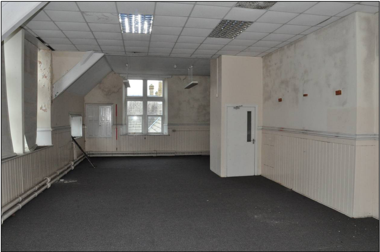
Plate 45: 1879 Board School, laboratory (1F7), showing original features, looking W (photo 2484).
