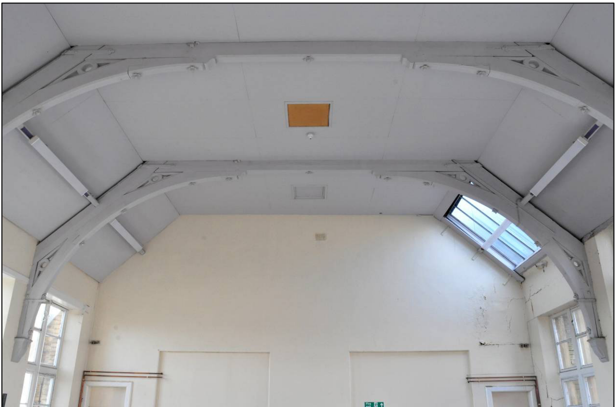
Plate 35: 1879 Board School, girls' hall (GF4), roof trusses, looking W (photo 2439).
