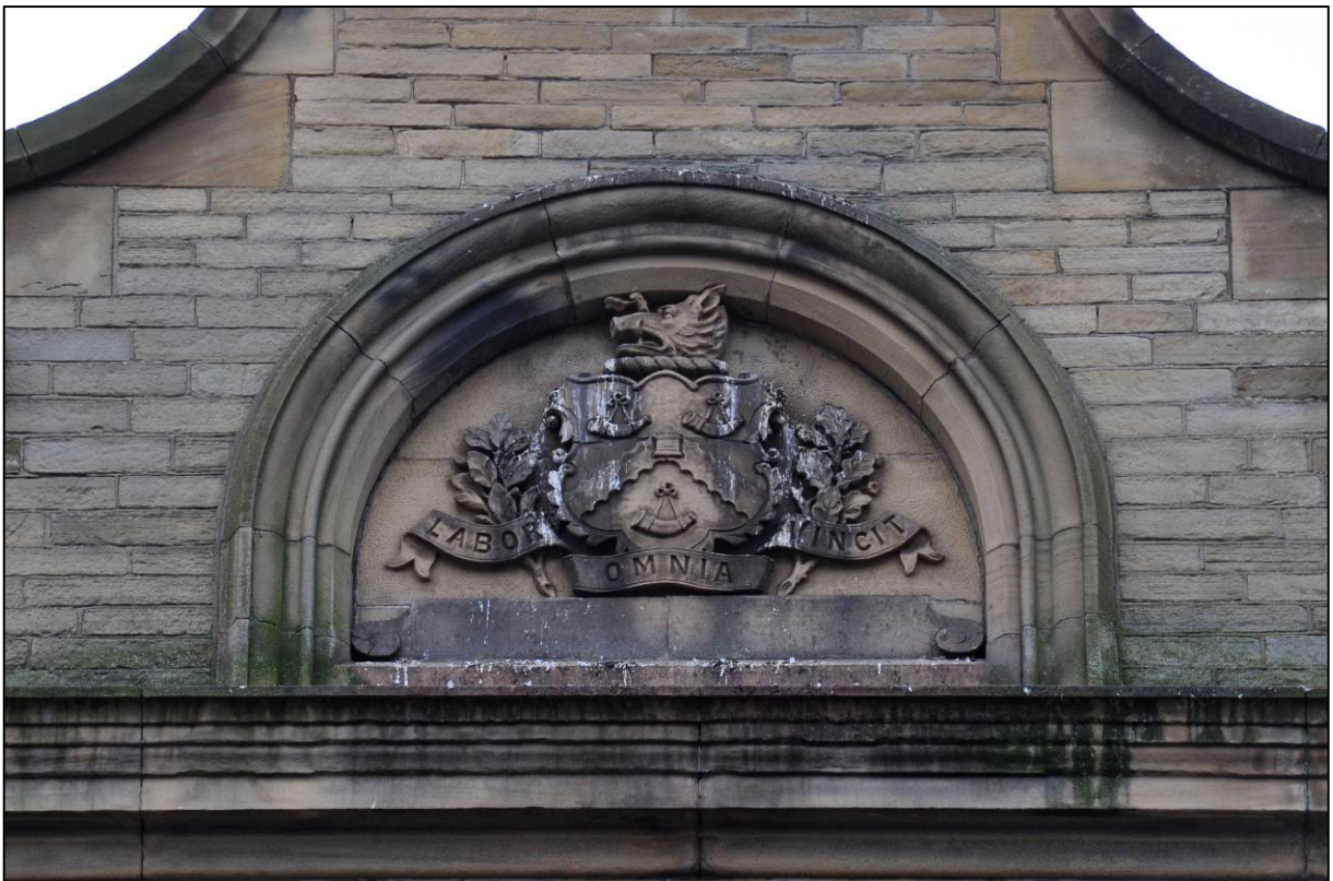
Plate 53: 1895 Higher Grade Boys' School, east elevation, Bradford coat of arms to central bay, looking W (photo 2121).
