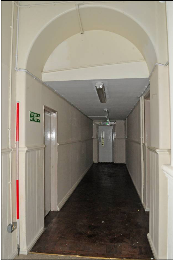
Plate 76: 1895 Higher Board Boys' School, east-west corridor (1F14), looking W (photo 2252).
