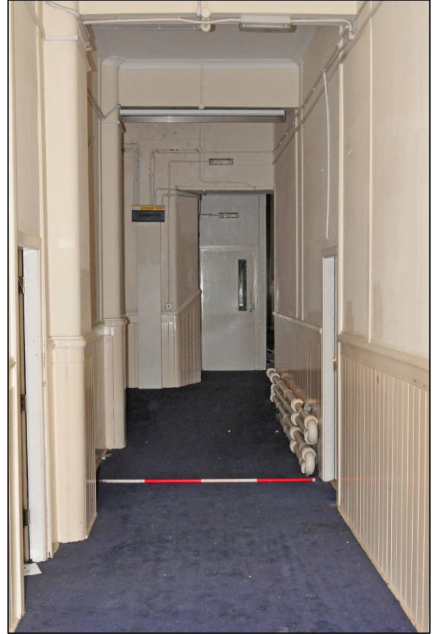
Plate 105: c.1897-99 Higher Grade Girls' School, corridor (1F18), showing misalignment with 1879 Board School corridor (GF11), looking W (photo 2391).
