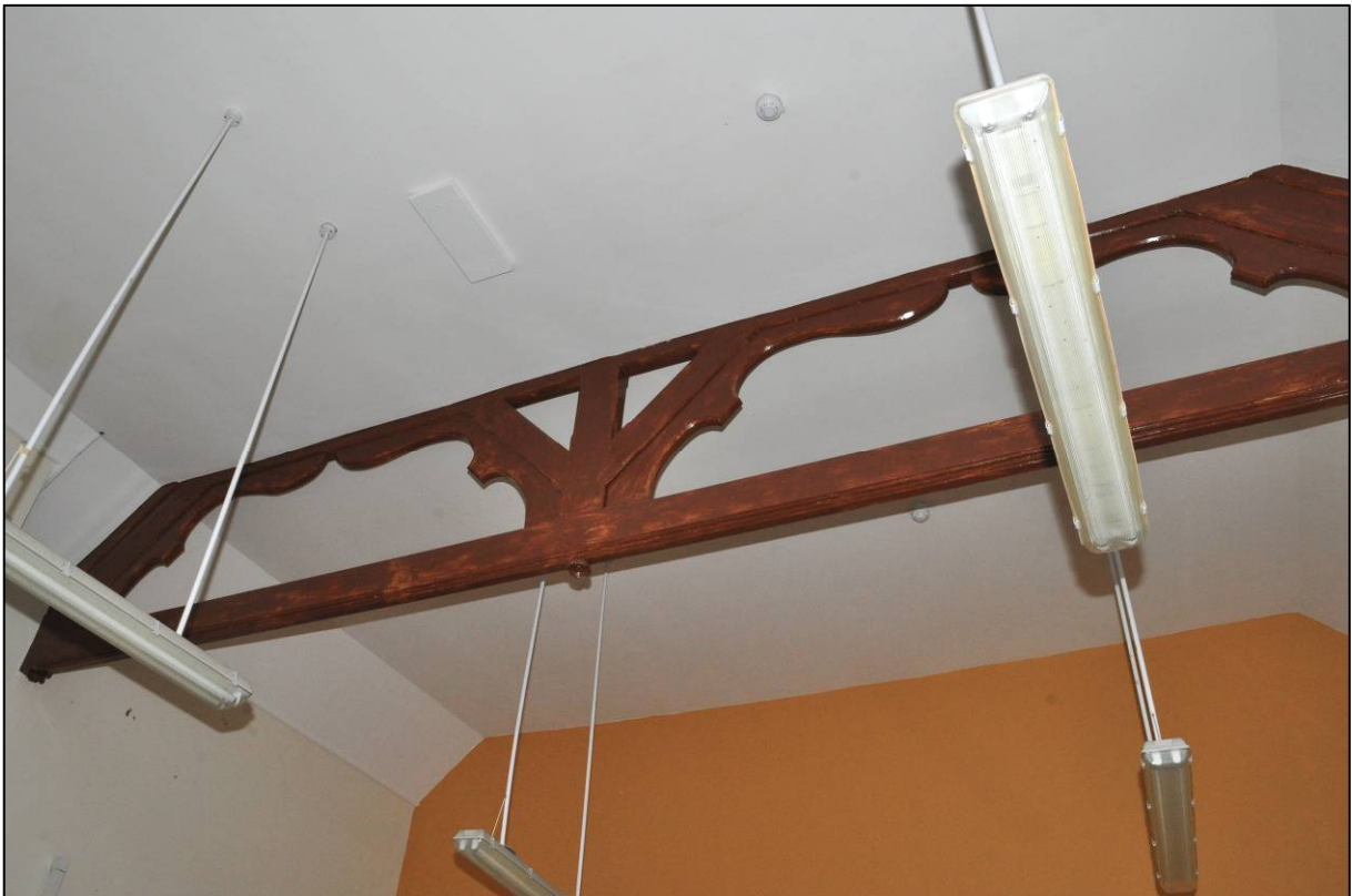
Plate 98: 1895 Higher Grade Boys' School, classroom (2F13), roof truss, looking E (photo 2352).
