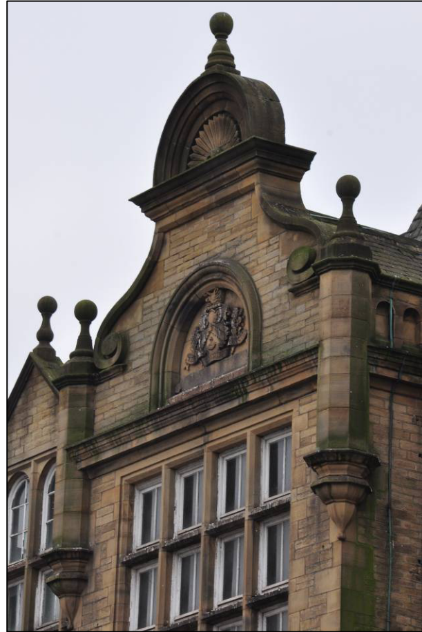
Plate 52: 1895 Higher Grade Boys' School, east elevation, gable and parapet to central bay, looking SW (photo 2127).
