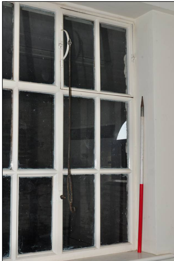
Plate 66: 1895 Higher Grade Boys' School, dining room (GF18), opening mechanism to window in south wall, looking SW (photo 2216).
