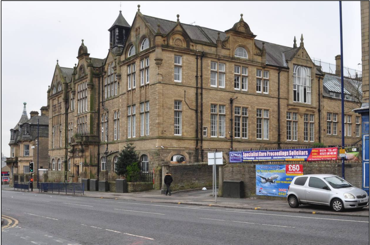
Plate 56: 1895 Higher Grade Boys' School, general view from Manningham Lane, looking SW (photo 2105).
