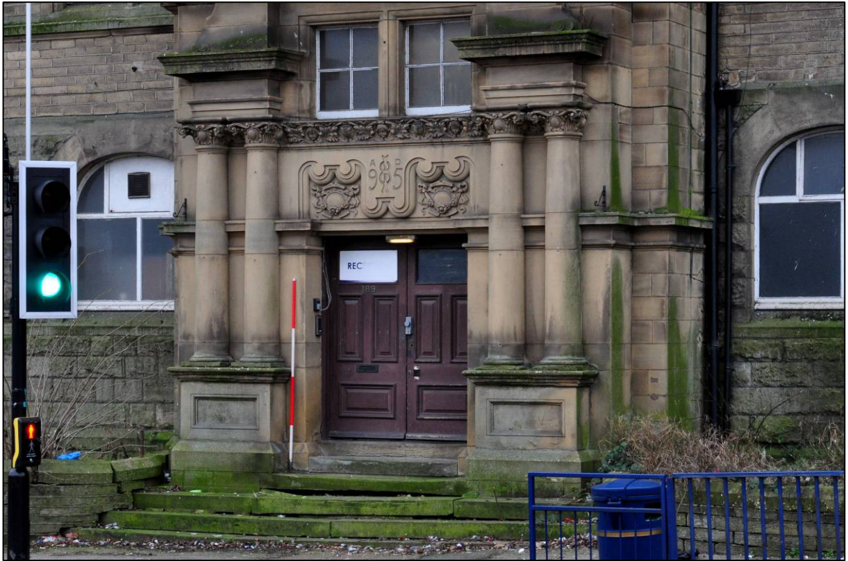
Plate 50: 1895 Higher Grade Boys' School, east elevation, ground floor entrance, looking W (photo 2109).
