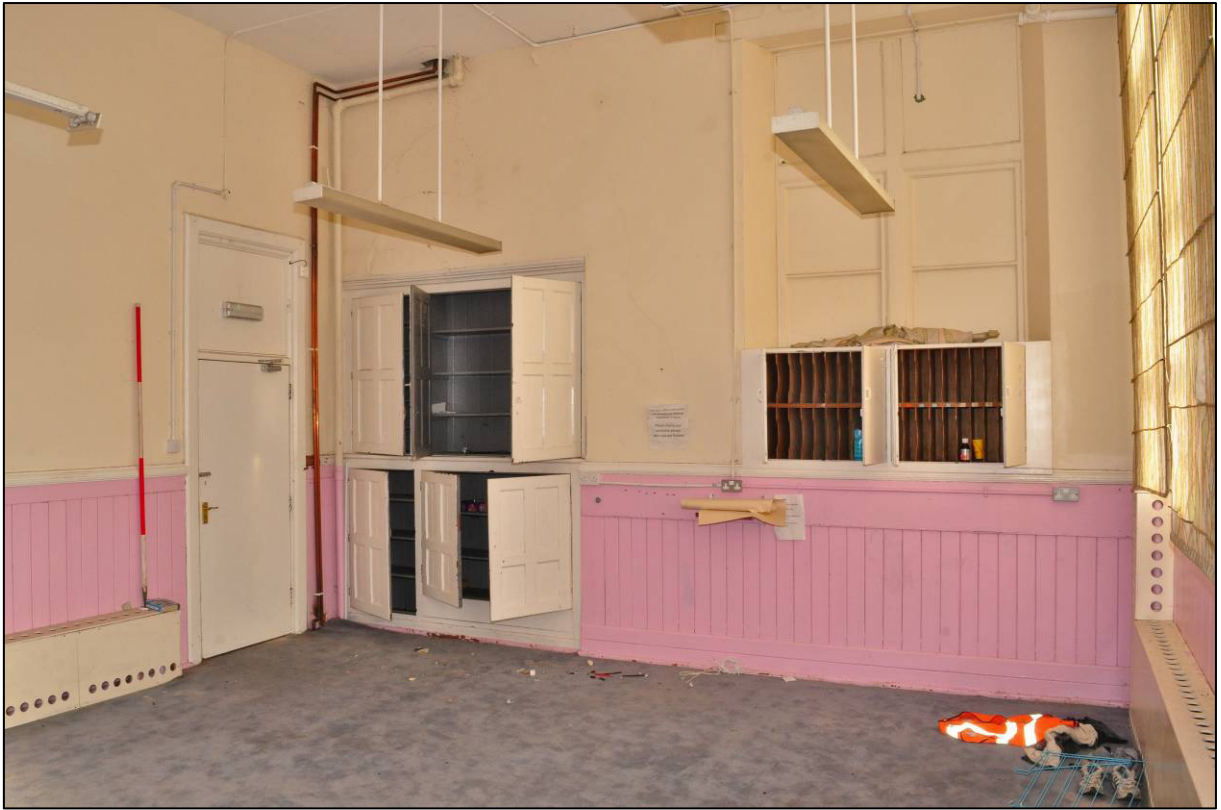
Plate 27: 1879 Board School, boys' classroom (GF13), original features to E wall, looking E (photo 2409).
