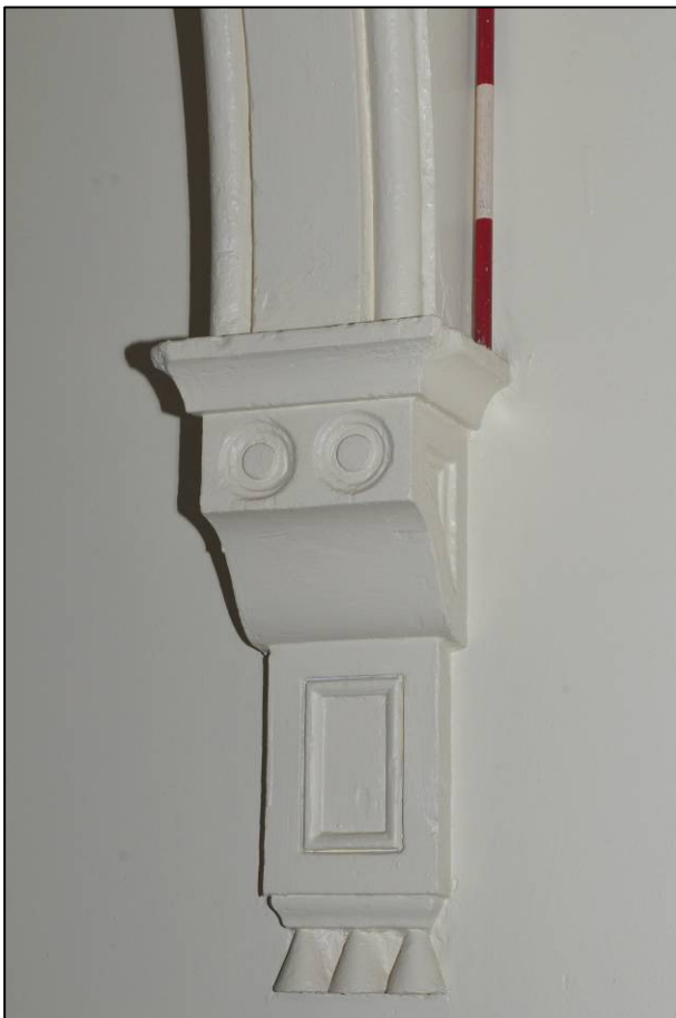
Plate 82: 1895 Higher Grade Boys' School, circulation space (2F2), corbel to arch, looking W (photo 2338).
