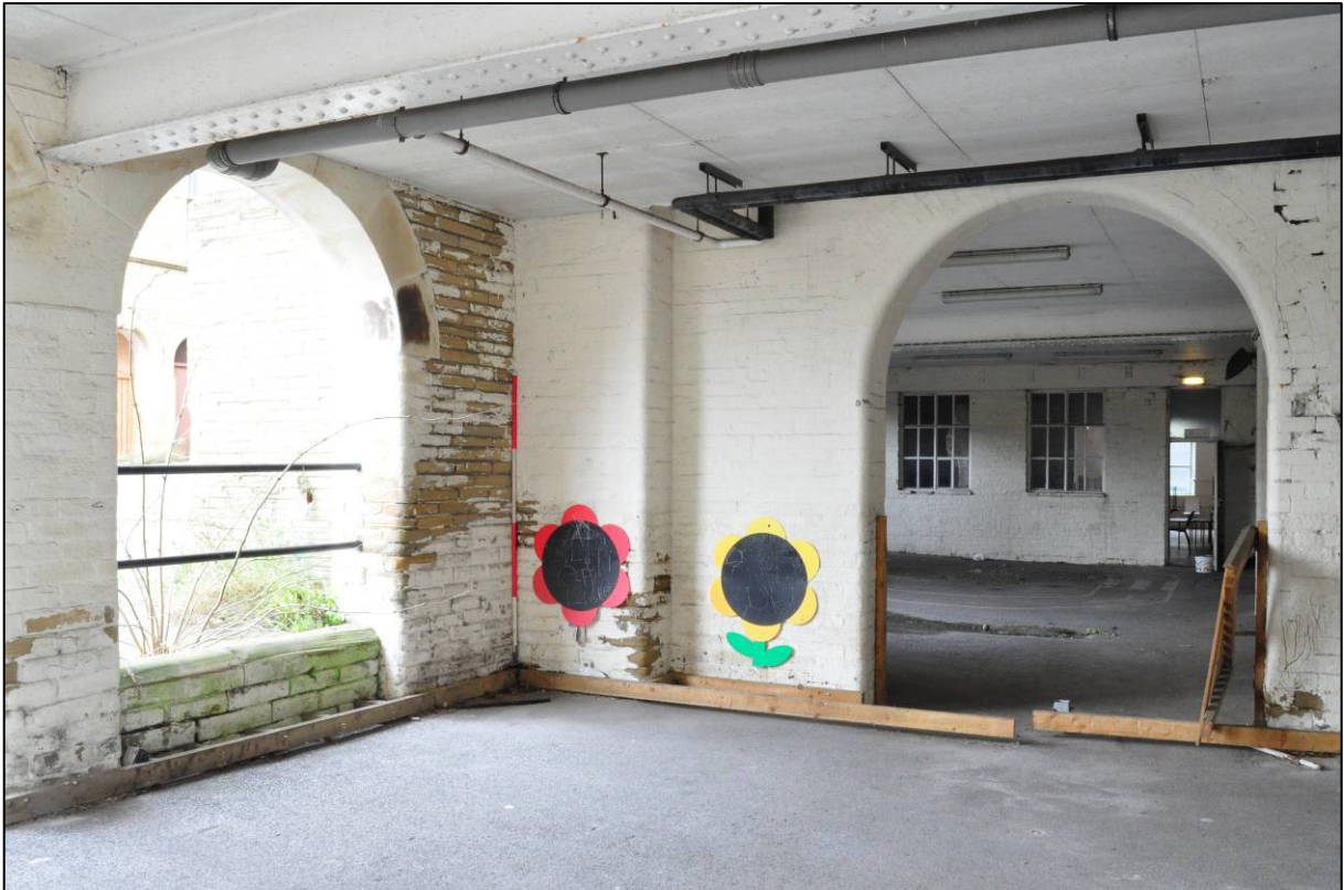
Plate 69: 1895 Higher Board Boys' School, south covered playground (GF24), looking NW (photo 2229).
