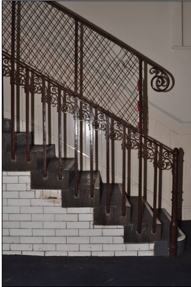
Plate 23: 1879 Board School, corridor (GF11), stairs, looking S (photo 2408).
