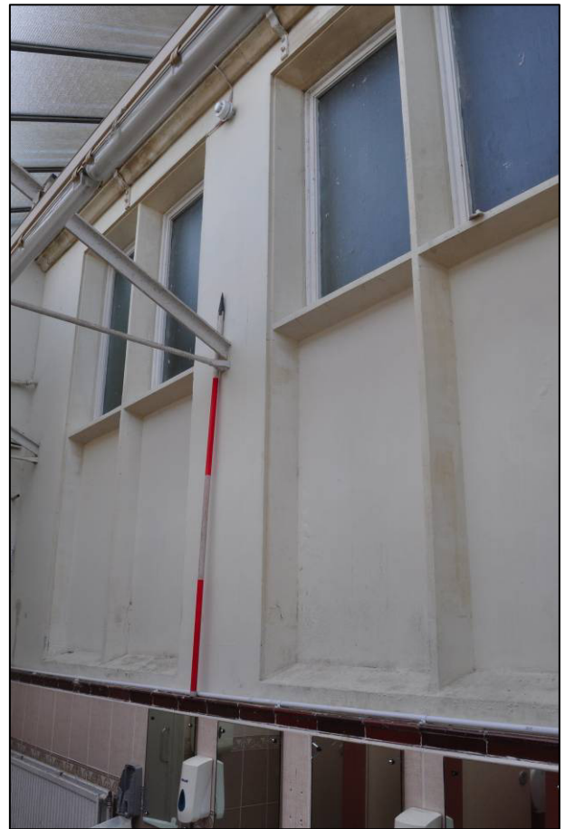
Plate 29: 1879 Board School, former girls' classroom (GF8), original external windows inside Higher Grade Girls' School 1908 extension (GF6), looking SW (photo 2429).
