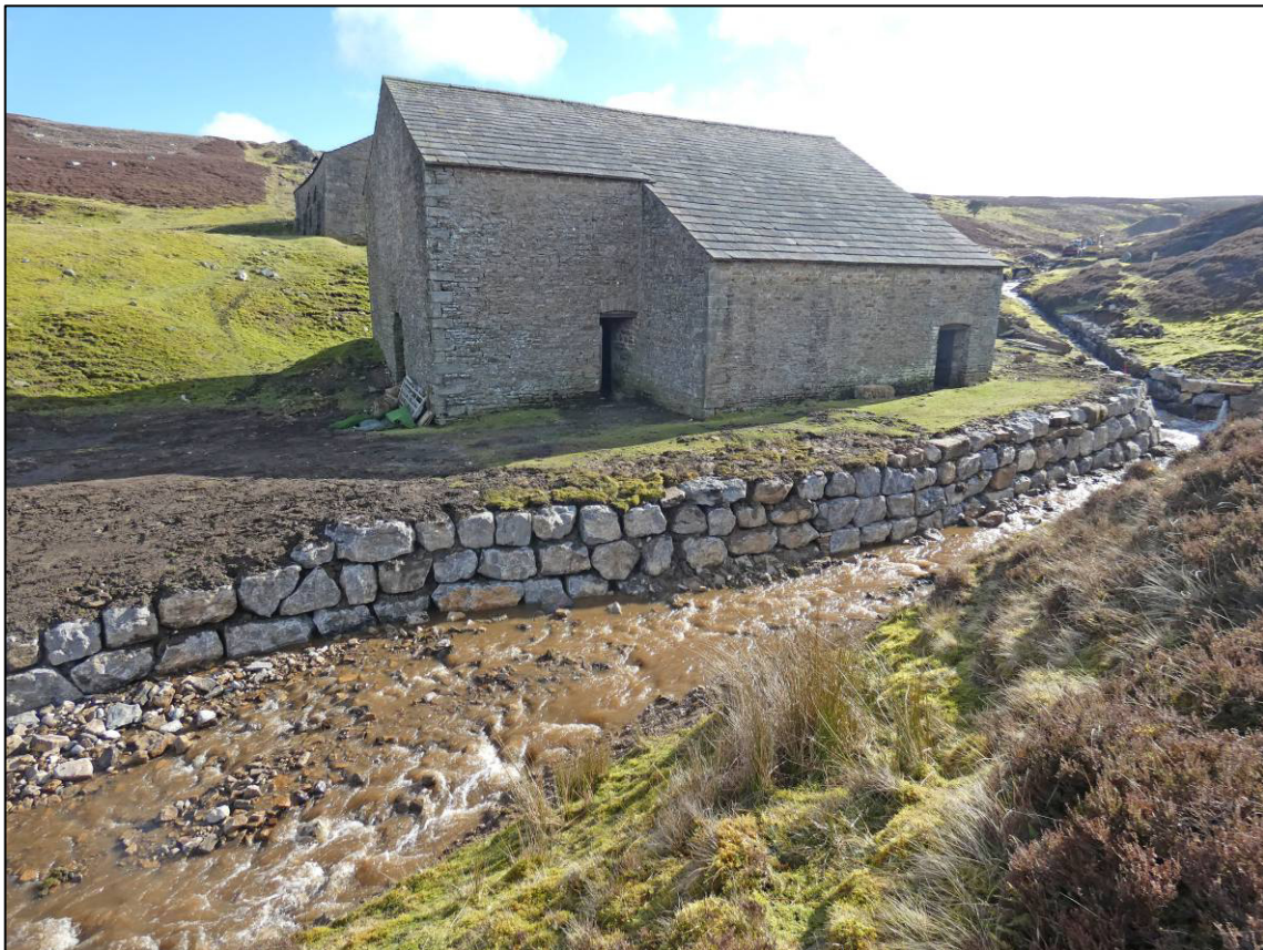
Plate 43: Completed rock-armoured wall to east side of beck, adjacent to smelt mill, looking SE (photo 4/155).
