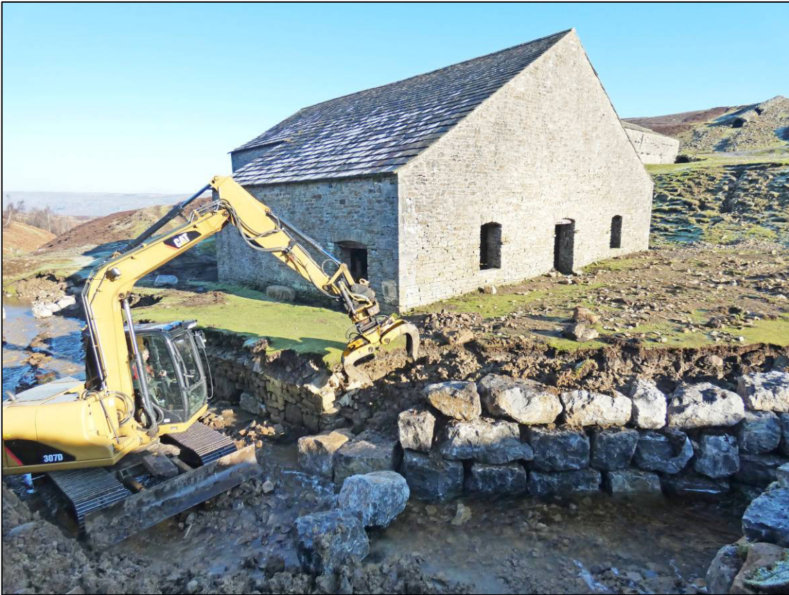
Plate 40: Rock-armoured wall under construction, adjacent to smelt mill, looking NE (photo 3/814).
