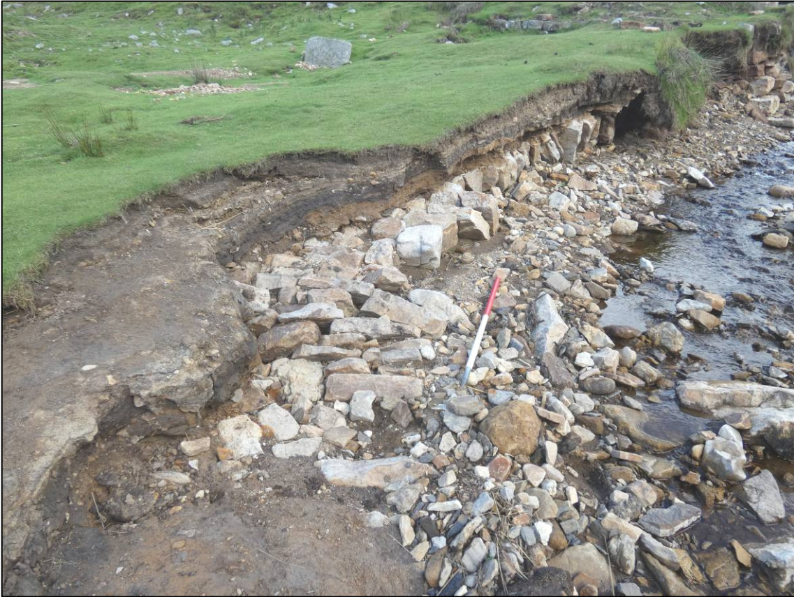
Plate 5: Exposed section of pitched stone surface in east side of beck/spillway, looking S (photo 2/896).
