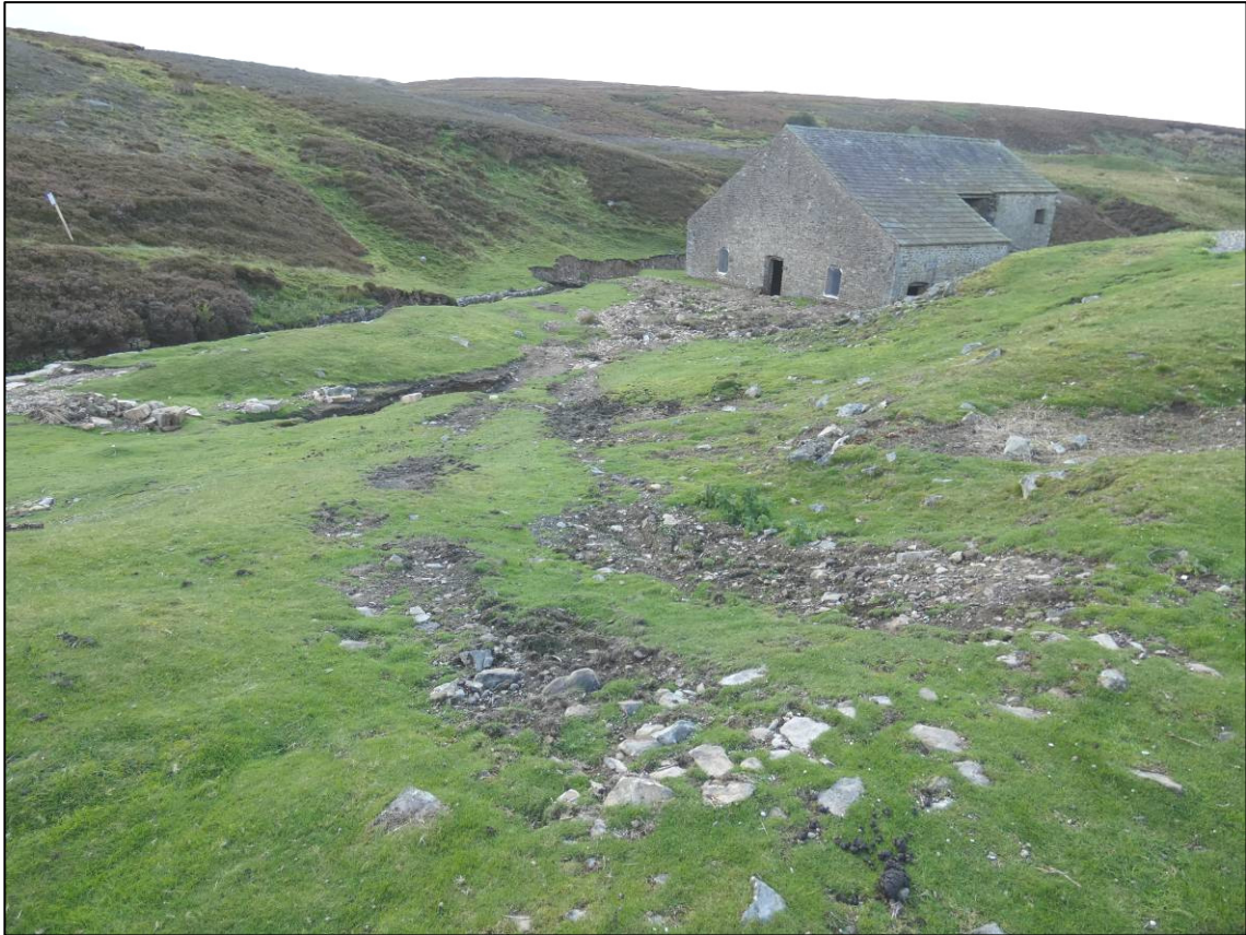
Plate 7: Erosion scars following vehicle tracks off north-west corner of smithy range, looking NW (photo 2/890).
