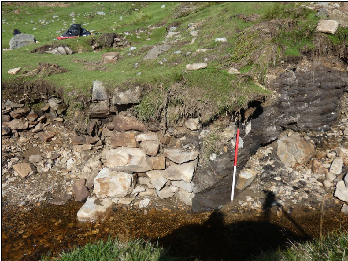
Plate 33: Reservoir dam, west facing section (S2), detail of front wall (024) and peat infill (026), looking E (photo 1/533).
