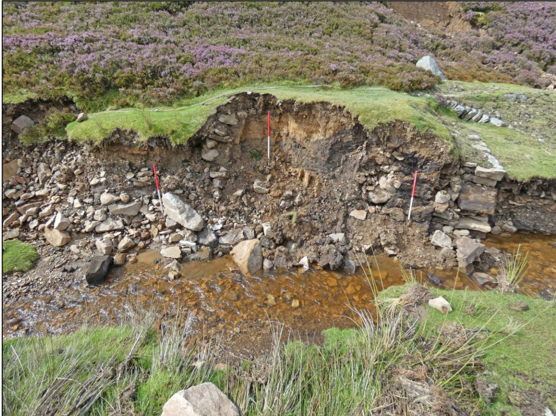
Plate 26: Reservoir dam, east facing section (S1), looking W (photo 1/516).
