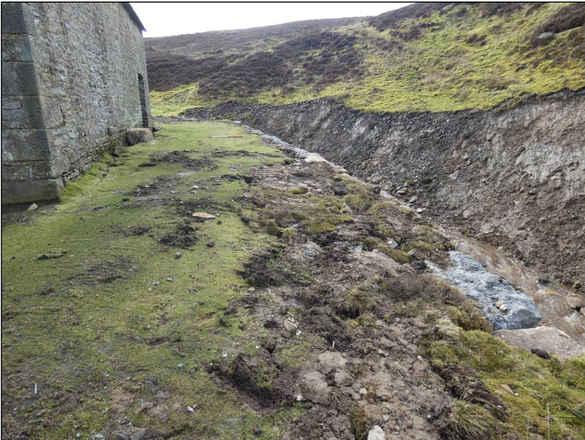
Plate 41: Repaired area to west of smelt mill, looking S (photo 4/146).
