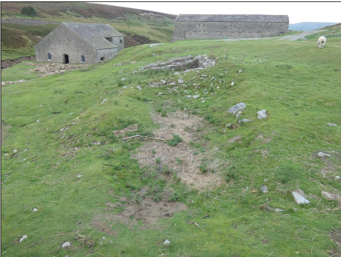
Plate 6: Flood debris in south cell of smithy range, looking N (photo 2/904).
