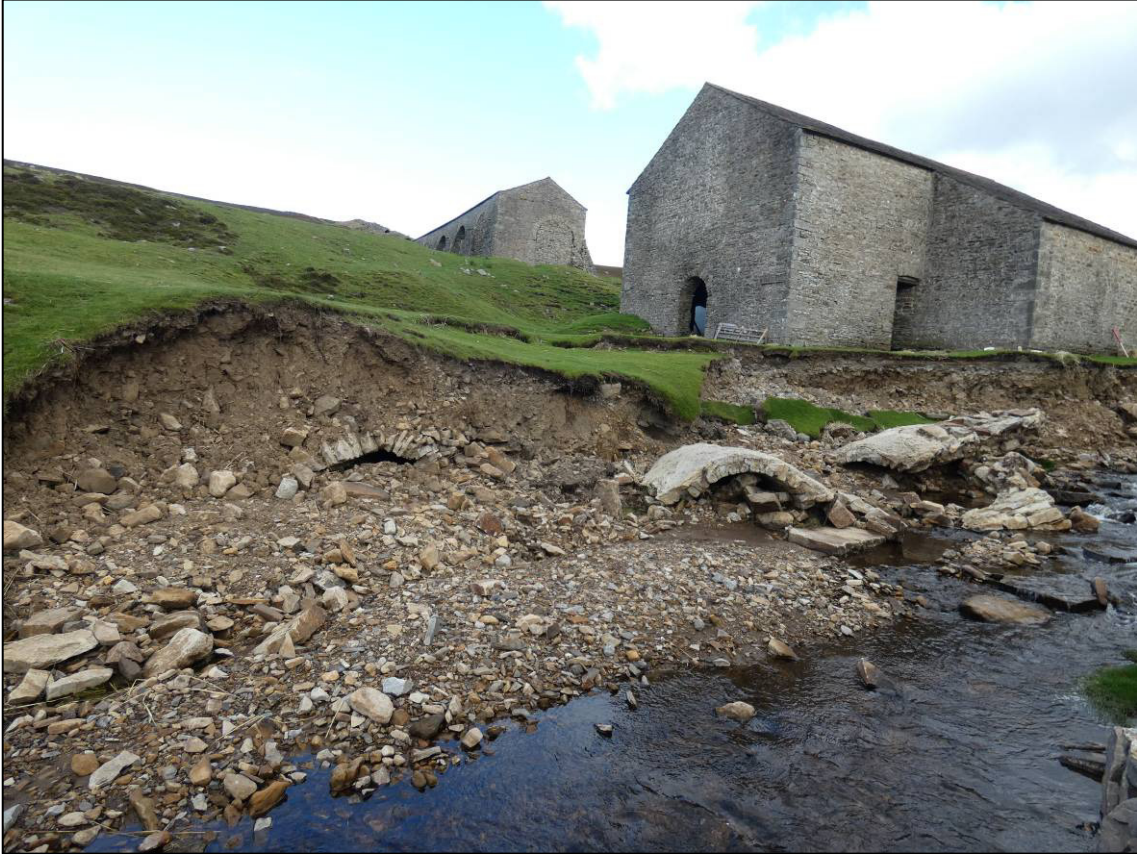
Plate 22: Remains of culvert roof and smelt mill tailrace, east side of beck, looking SE (photo 2/870).
