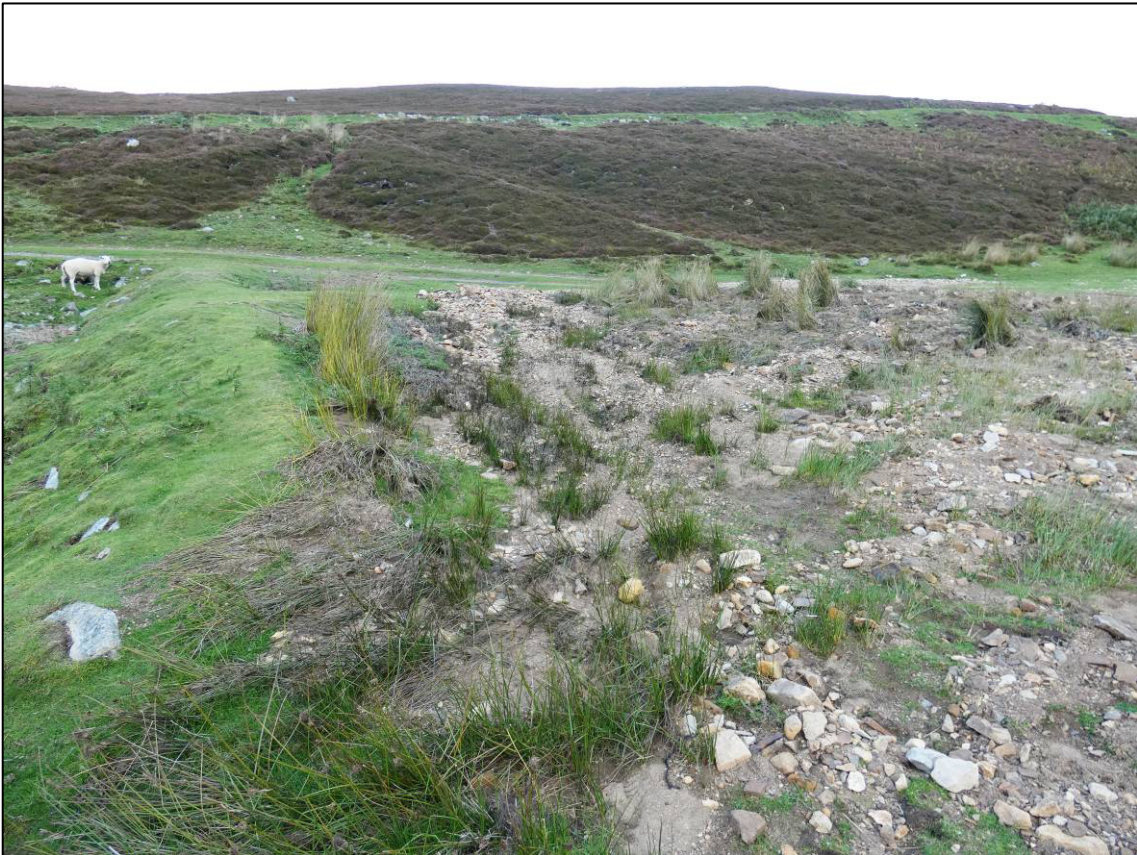
Plate 4: Flood debris in reservoir, looking E (photo 2/901).
