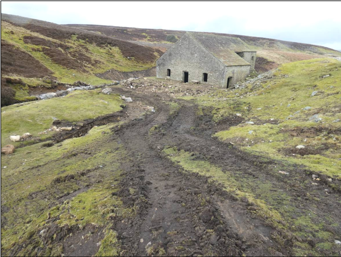
Plate 38: Vehicle tracks to area between reservoir dam and smelt mill, looking NW (photo 4/138).
