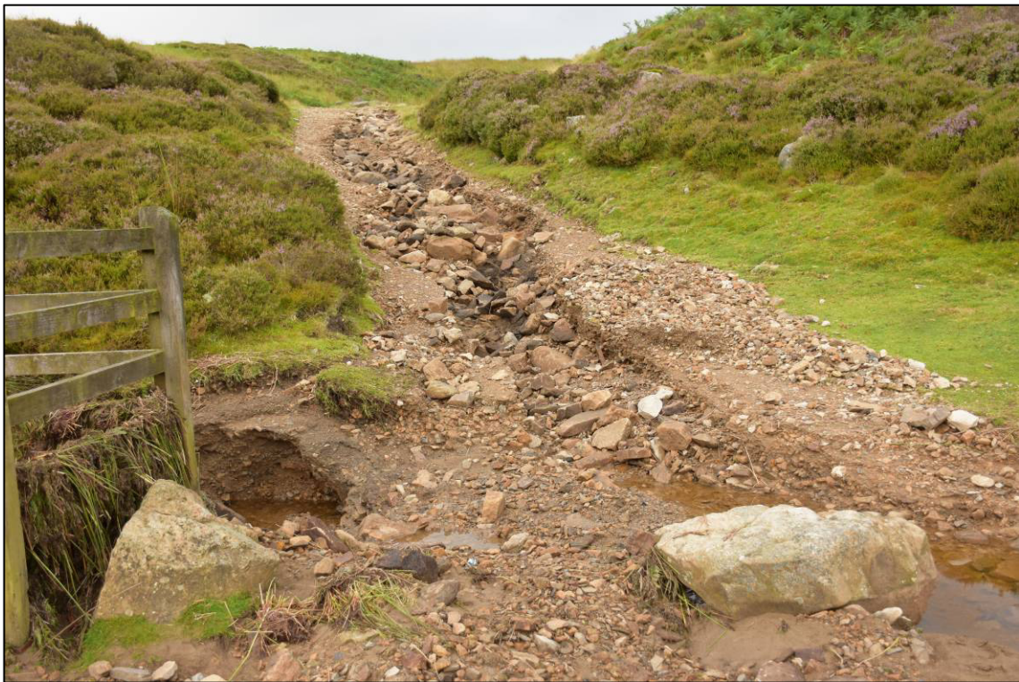
Plate 2: Eroded track running west from beck crossing point, looking S (photo courtesy Miles Johnson, YDNPA).
