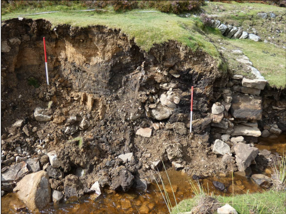
Plate 28: Reservoir dam, east facing section (S1), north part showing earliest phase of dam, looking W (photo 1/518).
