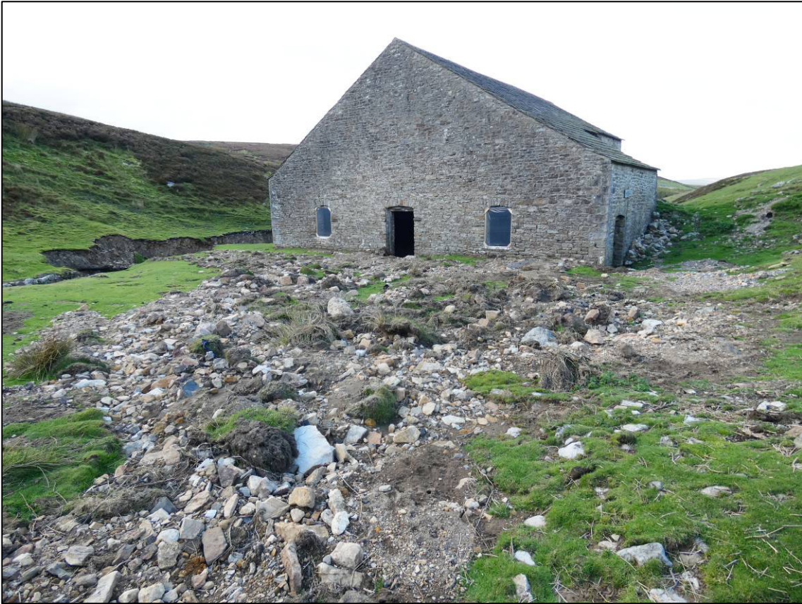
Plate 11: Flood debris to south of smelt mill, looking N (photo 2/891).
