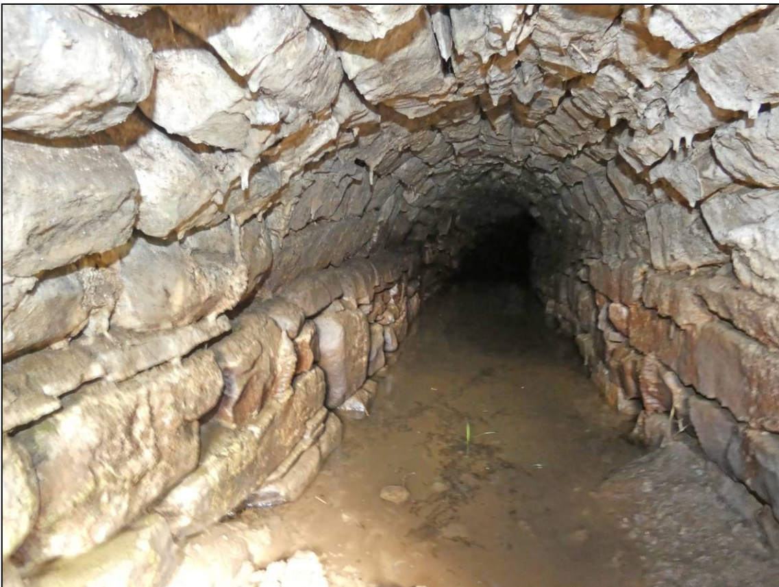
Plate 23: Inside of smelt mill tail race, looking SE (photo 2/885).
