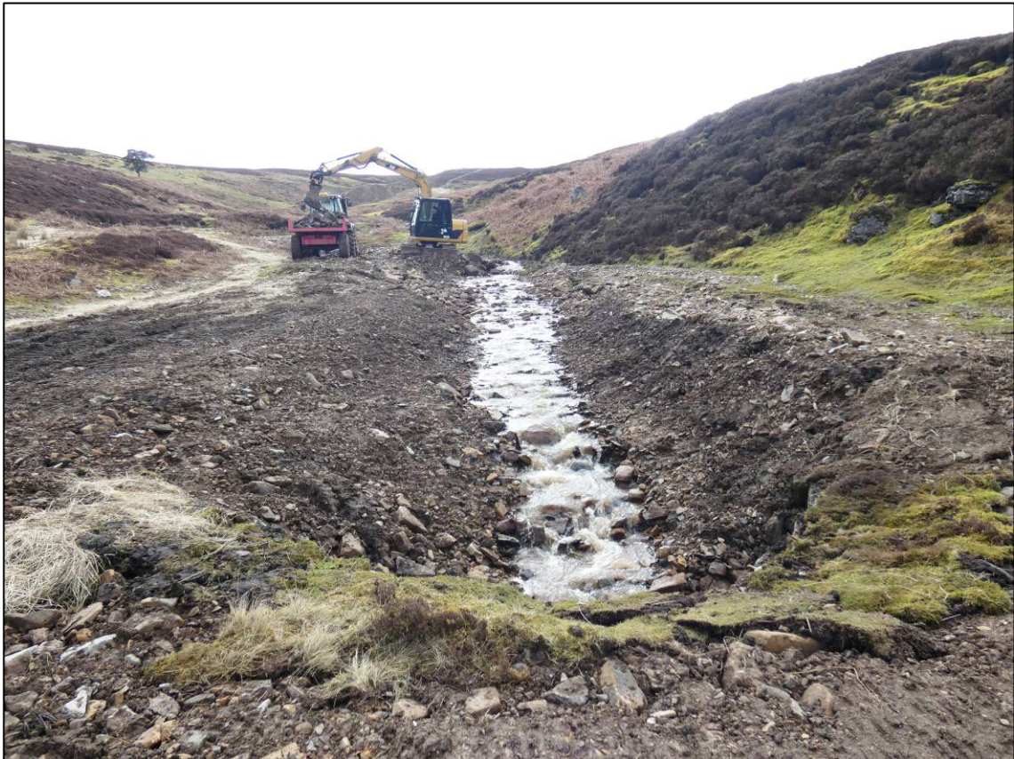
Plate 35: Regraded sides to beck, south of track, looking S (photo 4/129).
