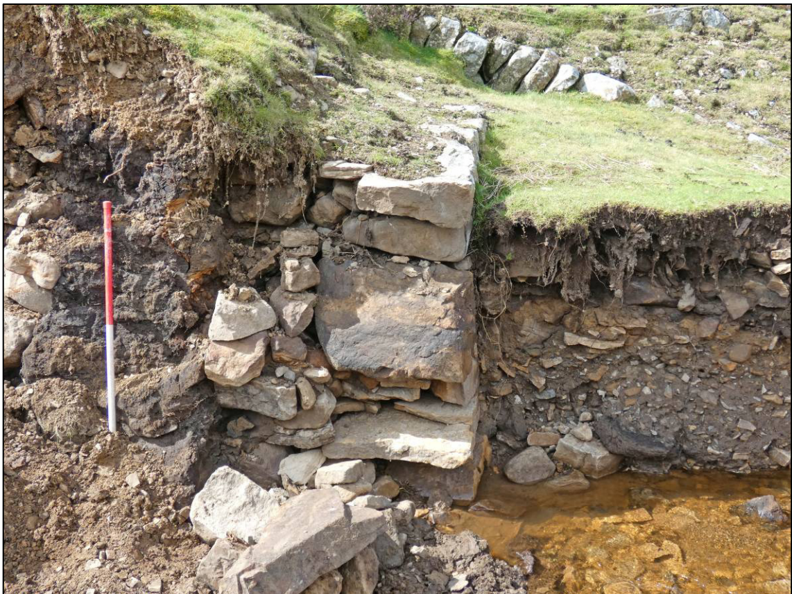
Plate 29: Reservoir dam, east facing section (S1), detail of front north wall (005), looking W (photo 1/520).
