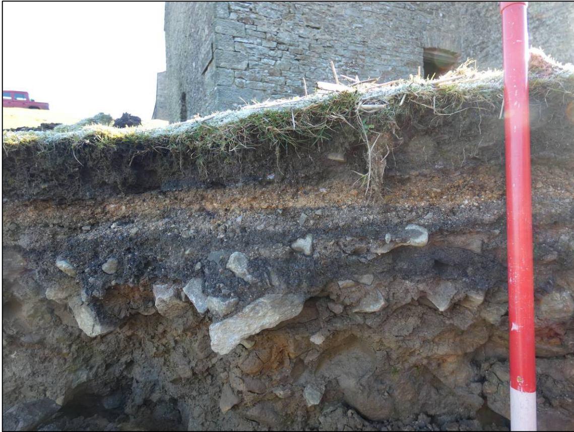
Plate 42: Compacted surfaces exposed in west facing section to west of smelt mill, looking E (photo 3/832).
