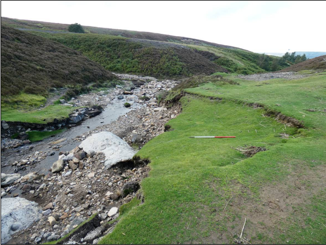
Plate 24: Slumped ground, east side of beck, north-west of smelt mill, looking N (photo 2/866).
