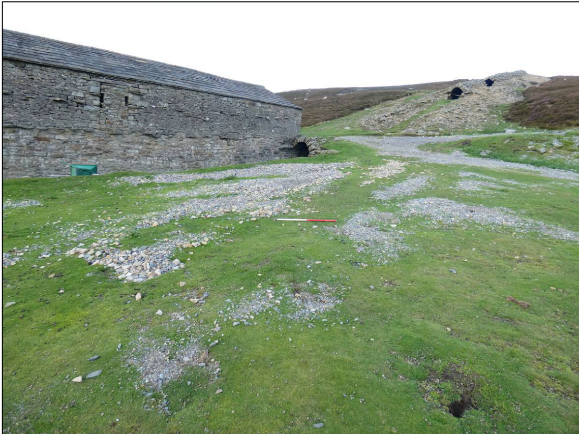
Plate 8: Abraded gravels washed into area to south of peat house, looking E (photo 2/889).
