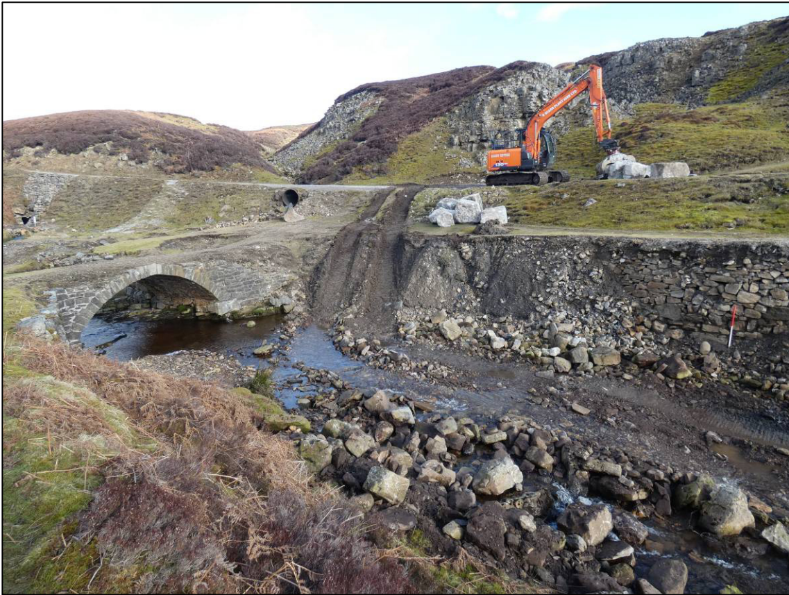
Plate 5: Area 1N, works in progress, looking N (photo 1/836).
