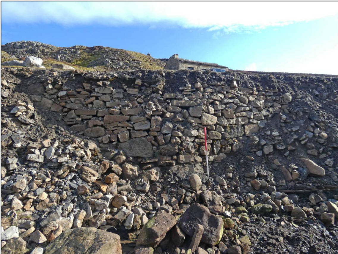
Plate 4: Area 1N, exposed revetment wall, looking NE (photo 1/832).
