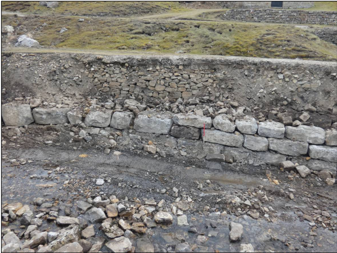
Plate 7: Area 1N, exposed revetment wall behind rock armour, looking NE (photo 2/882).
