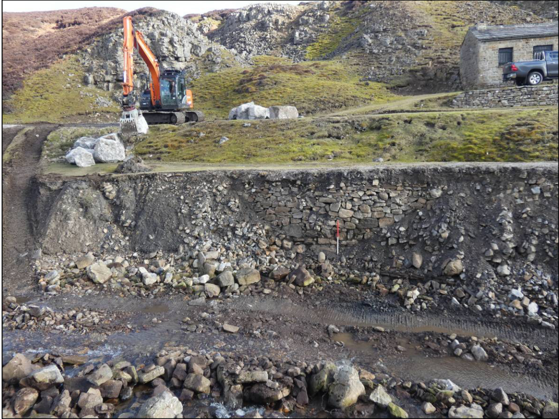
Plate 3: Area 1N, exposed revetment wall, looking NE (photo 1/835).
