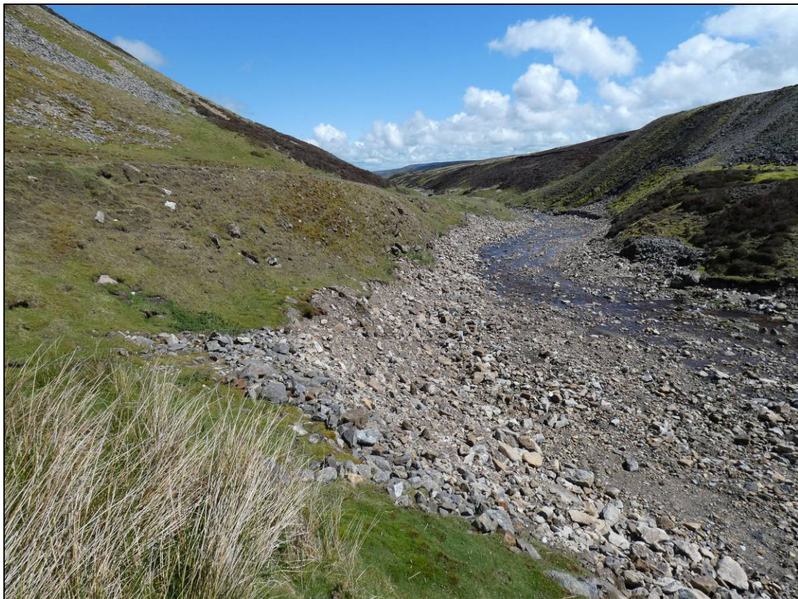
Plate 22: Area 3N, works complete and bedded-in, looking S (photo 3/305).
