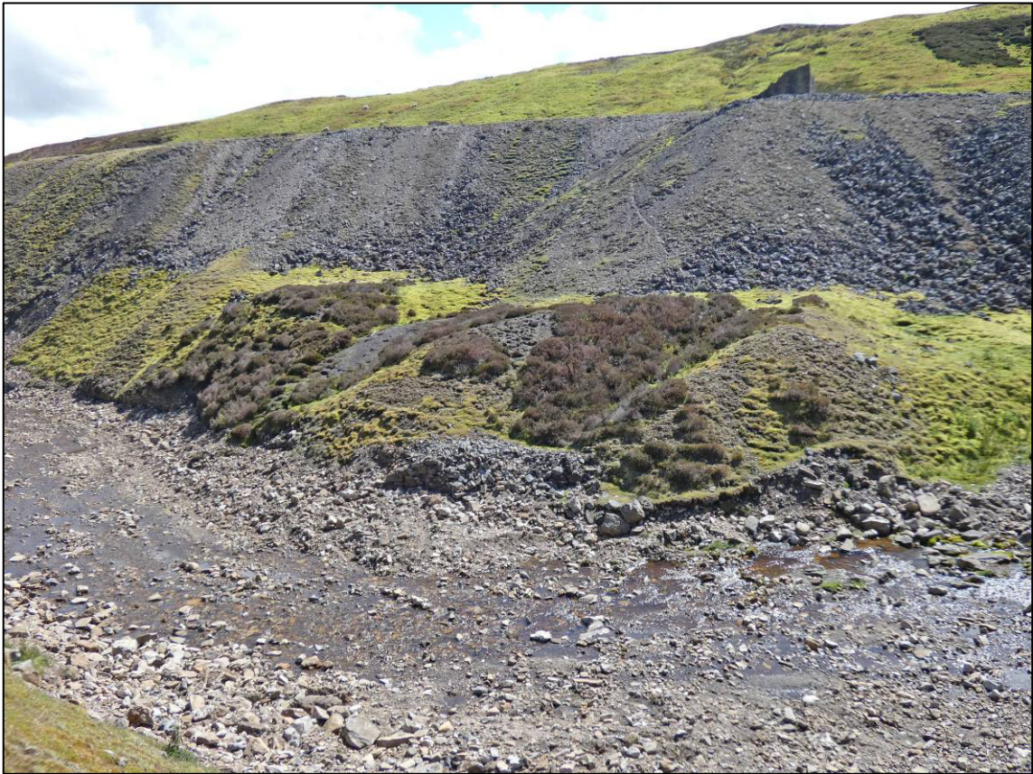
Plate 19: Area 3W, works complete and bedded-in, looking S (photo 3/311).
