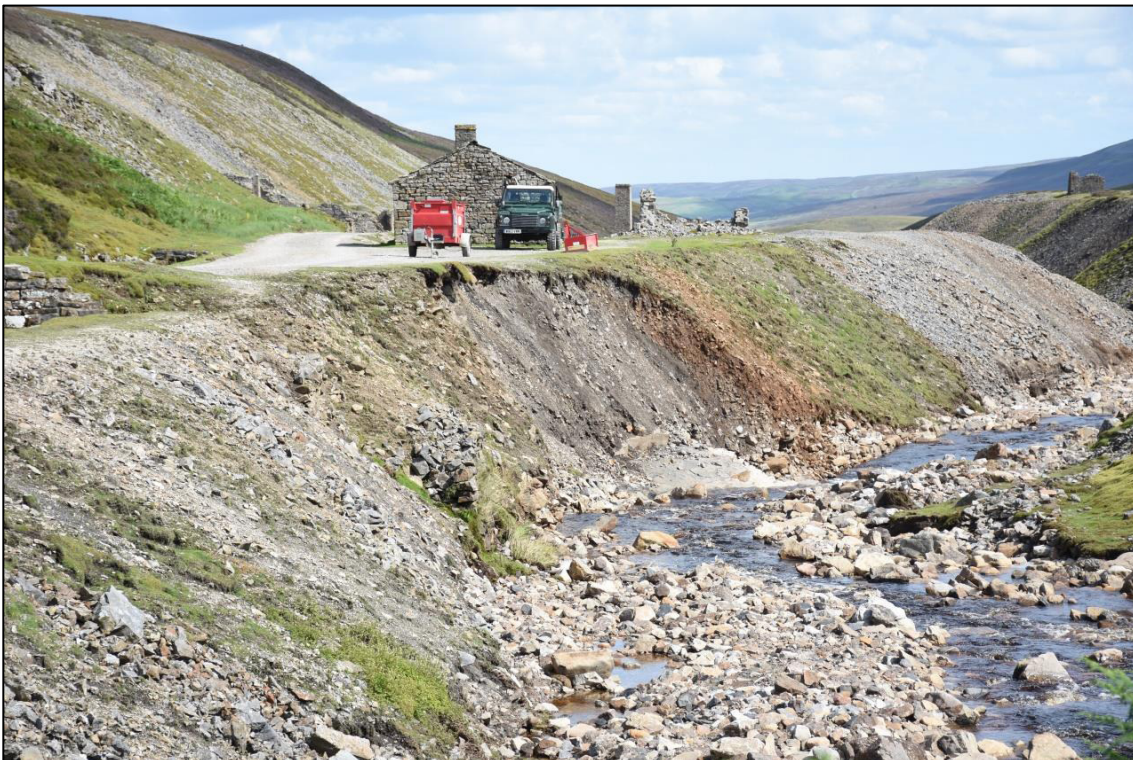
Plate 10: Area 2, prior to start of works, looking E (photo courtesy YDNPA).
