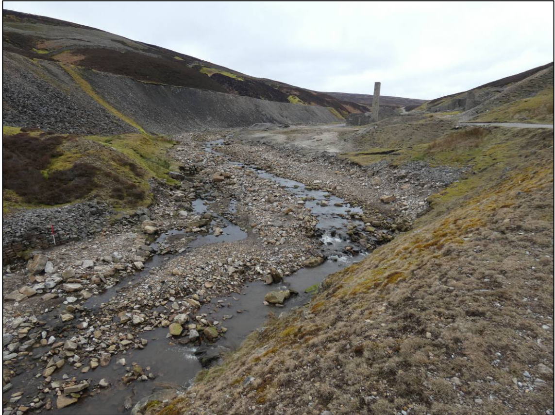
Plate 20: Area 3N, prior to start of works, looking NW (photo 1/870).
