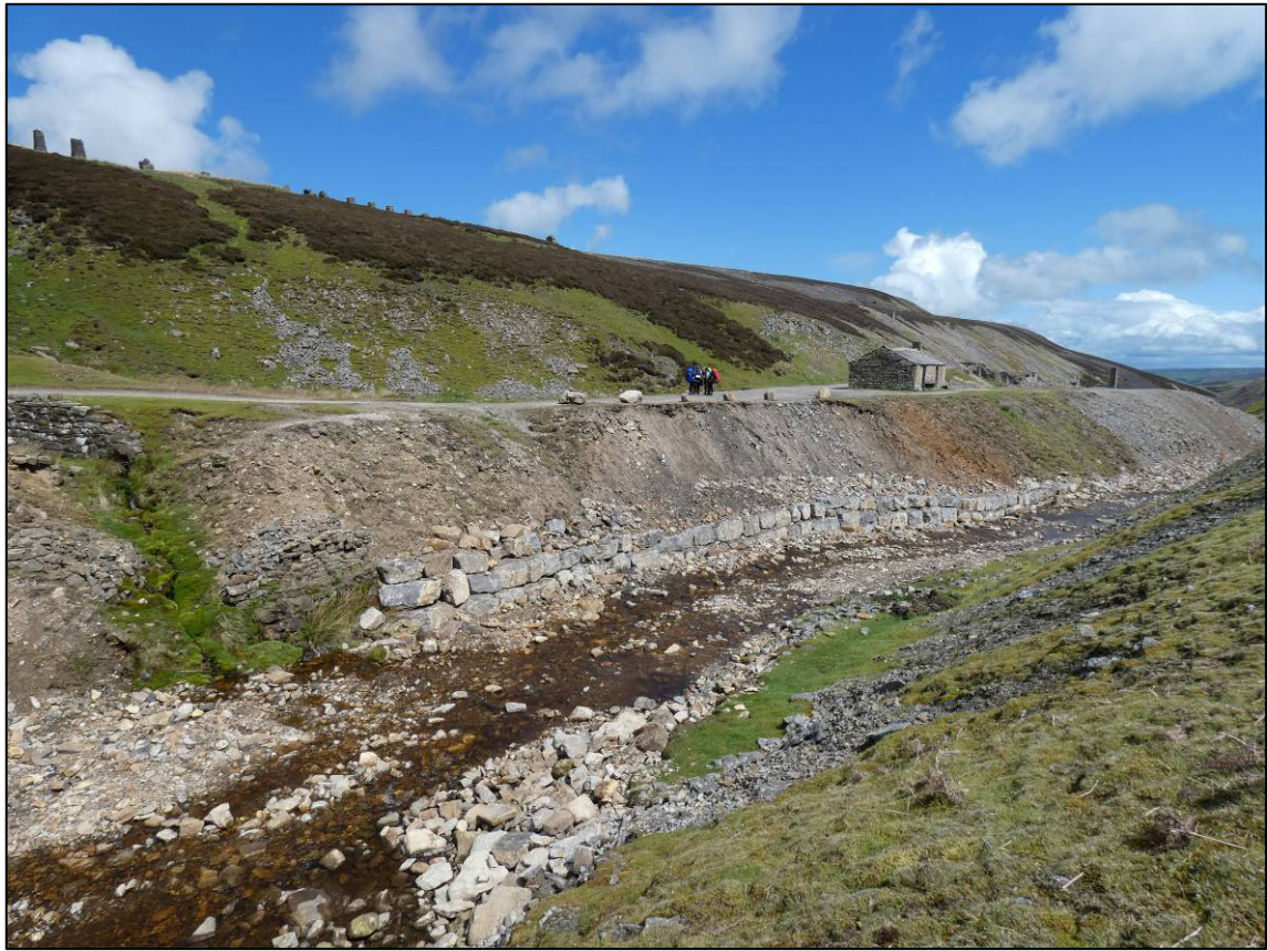
Plate 15: Area 2, works complete and bedded-in, looking E (photo 3/253).
