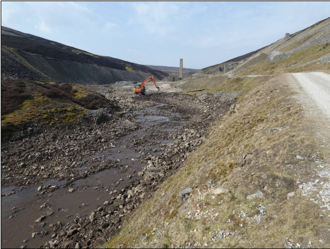
Plate 21: Area 3N, works in progress, looking NW (photo 2/905).
