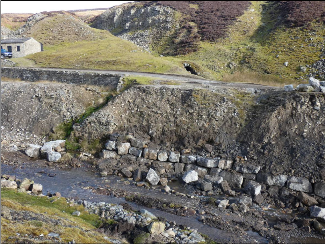
Plate 11: Area 2, west end, works complete, looking NE (photo 1/844).
