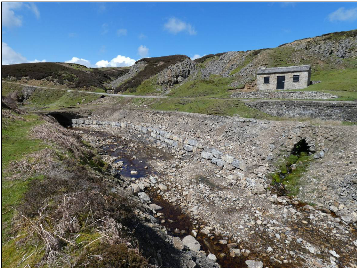
Plate 8: Area 1N, works complete and bedded-in, looking N (photo 3/280).
