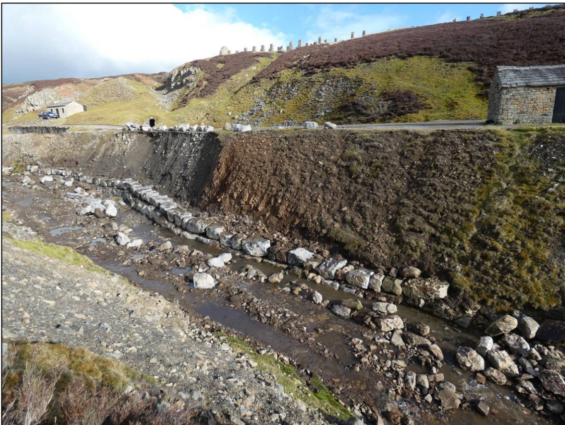
Plate 14: Area 2, works complete, looking N (photo 1/848).
