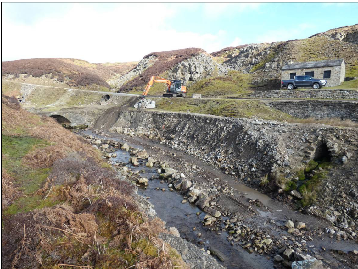
Plate 2: Area 1N, works in progress, looking N (photo1/839).
