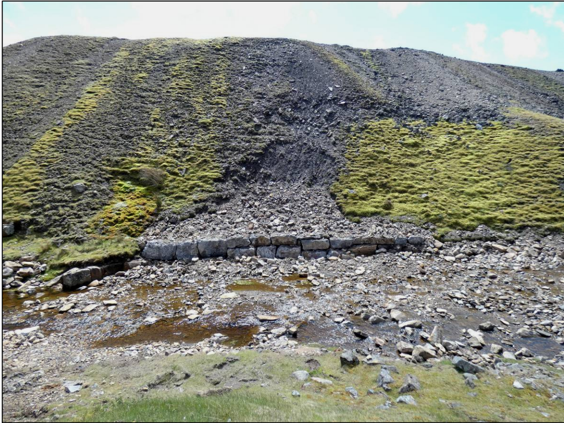
Plate 17: Area 3E, works complete and bedded-in, looking SW (photo 3/211).
