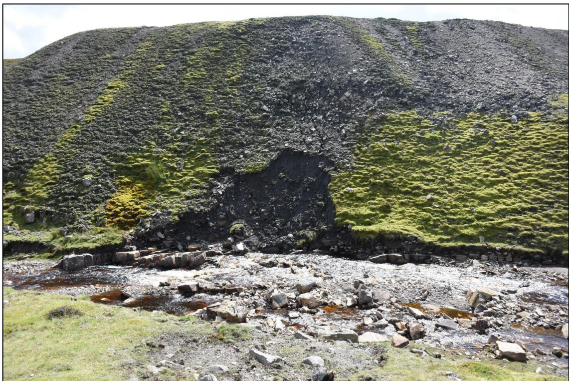
Plate 16: Area 3E, prior to start of works, looking SW (photo courtesy YDNPA).
