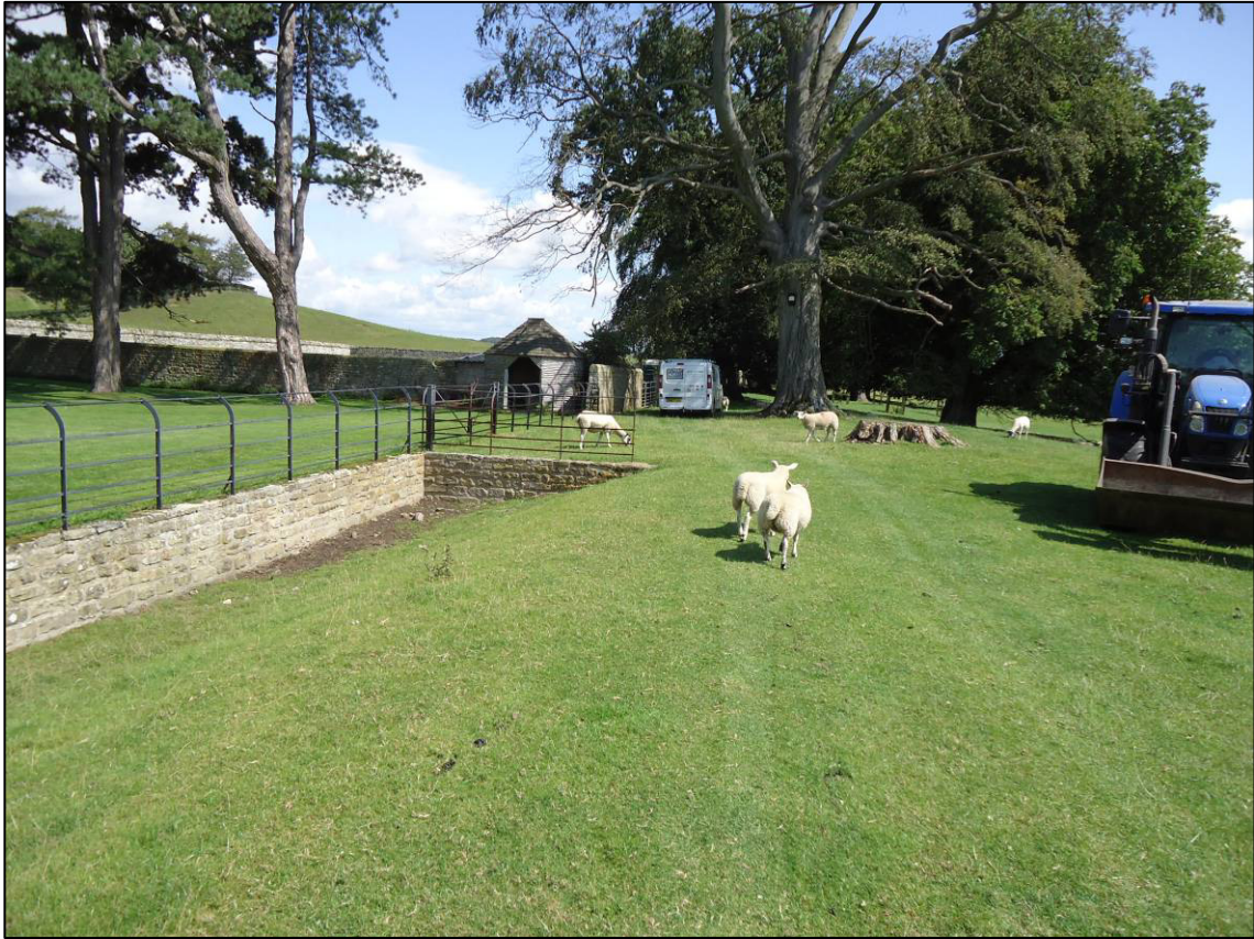
Plate 3: Existing ha-ha with gated entrance and infilled section to east, looking E (photograph courtesy Peter Pace, reproduced with permission).
