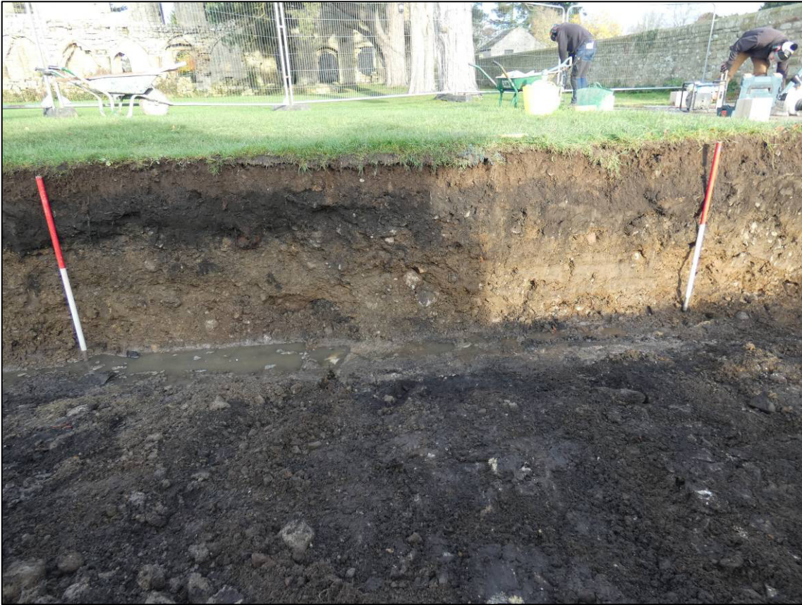
Plate 13: Ha-ha excavation, Section 3, completed excavation, looking N (photo 3/609).
