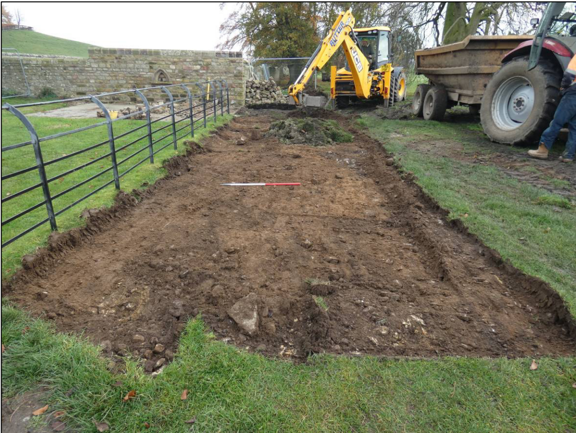
Plate 8: Topsoil stripping for ha-ha excavations, looking E (photo 2/573).
