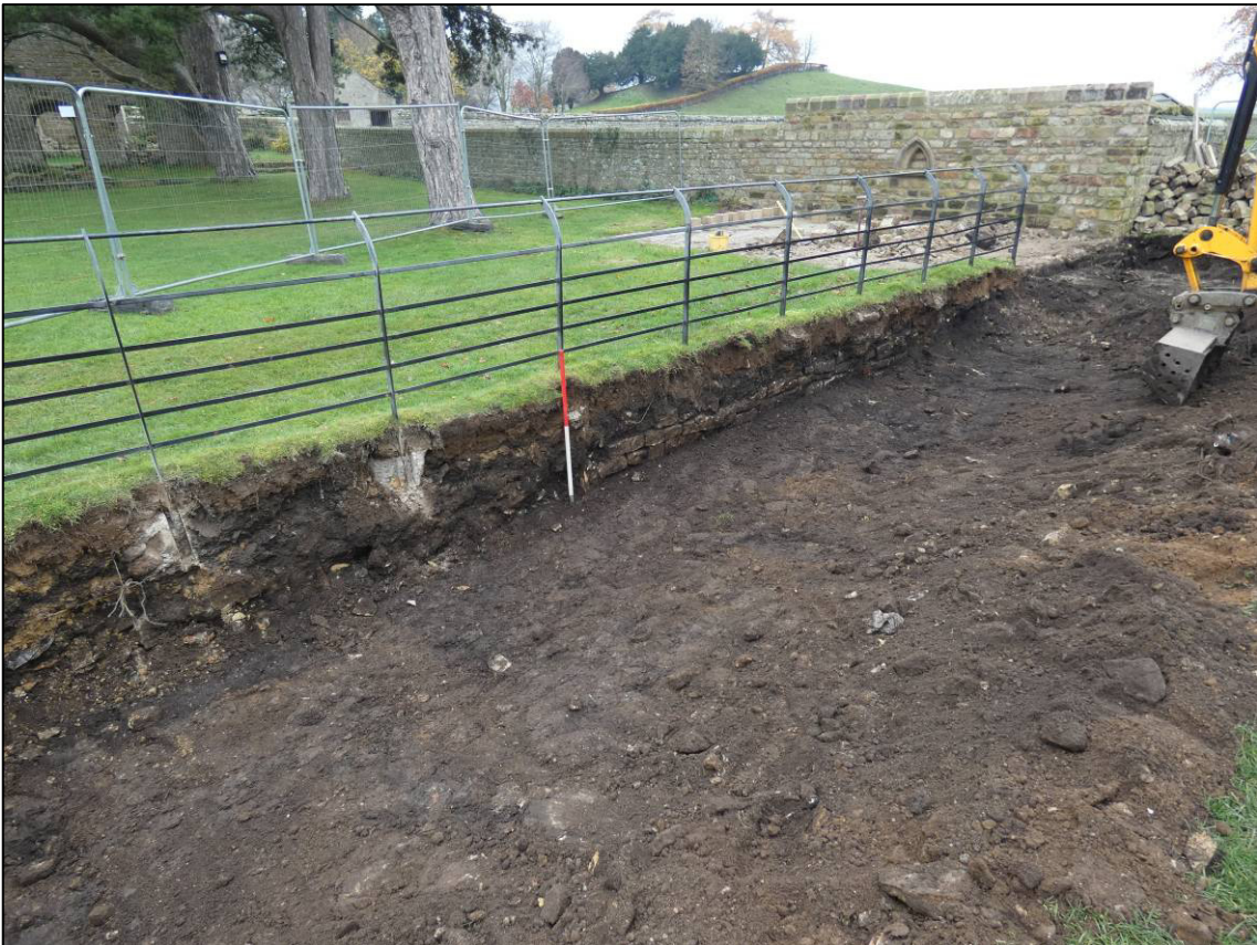
Plate 10: Ha-ha excavation, Section 2, general view, looking NE (photo 2/582).
