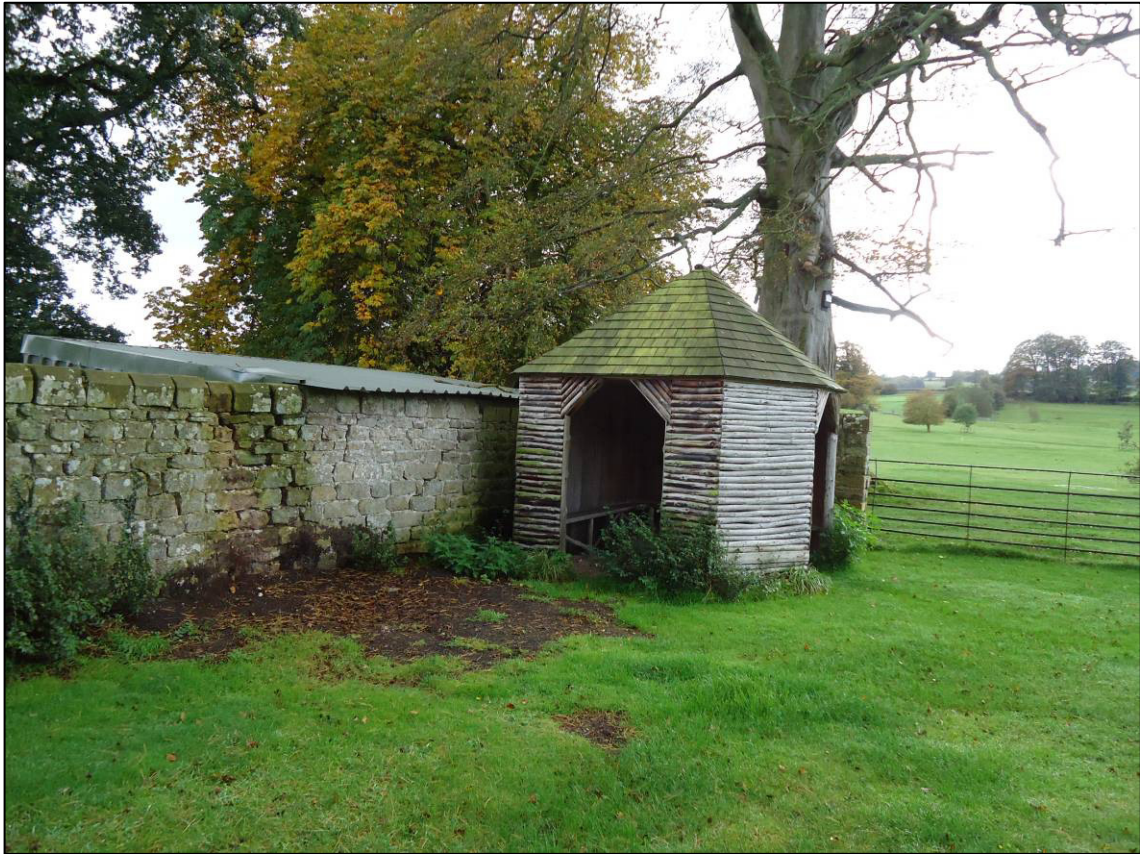
Plate 1: General view of existing shelter or gazebo, prior to demolition, looking SE (photograph courtesy Peter Pace, reproduced with permission).
