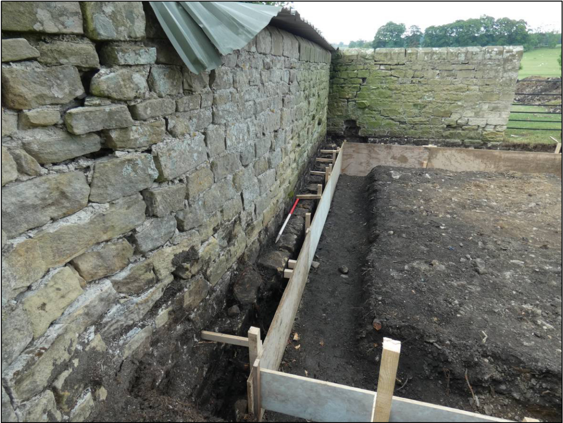
Plate 5: Footings to east boundary wall, looking S (photo 1/608).
