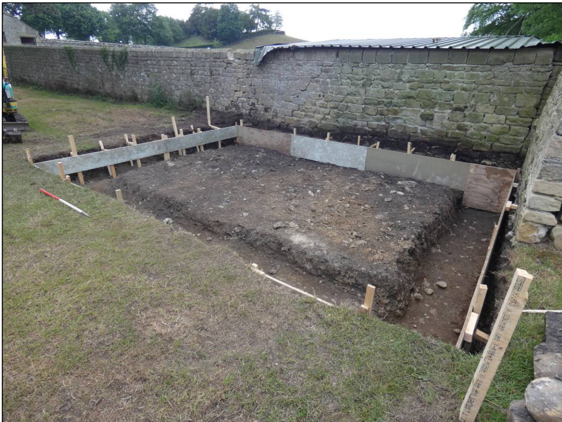
Plate 4: General view of excavations for new shelter, looking NE (photo 1/605).
