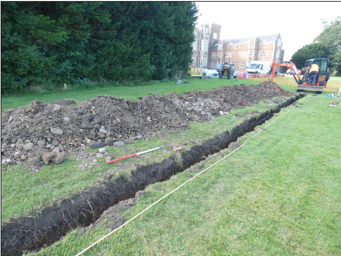
Plate 2: General view of excavations in progress, looking NW.
