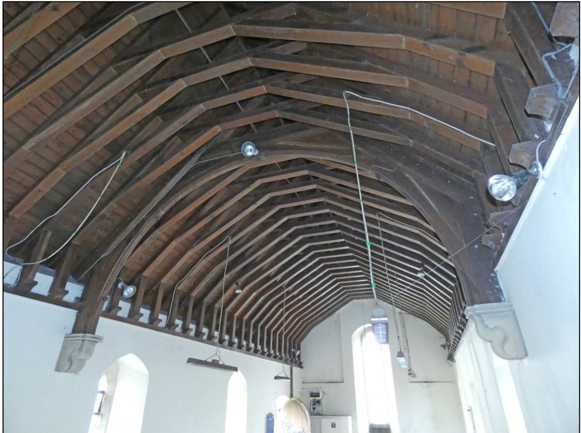
Plate 30: Internal roof structure, looking W (photo 1/003).
