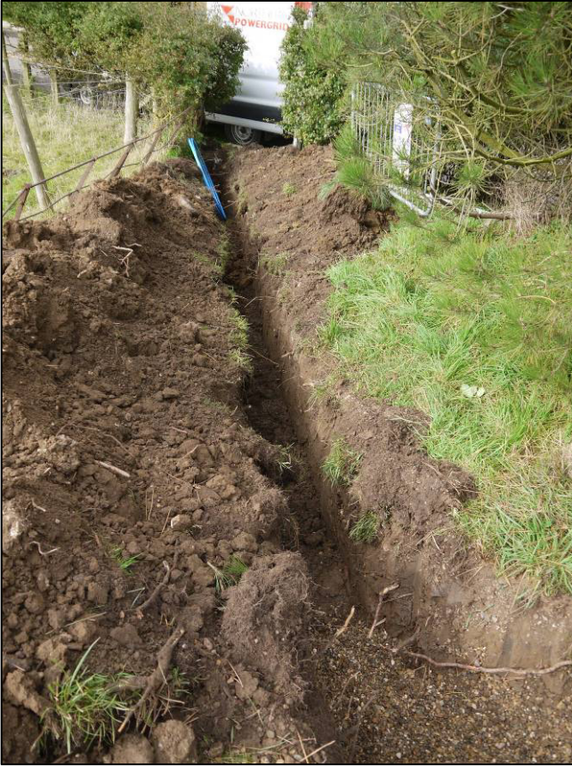
Plate 42: Trench 6, north-west end, looking NW.
