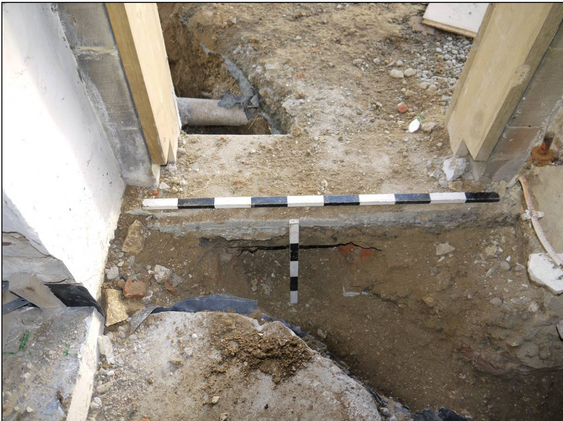
Plate 46: Trench 8, passing under step (115) of south doorway of chapel, looking S.
