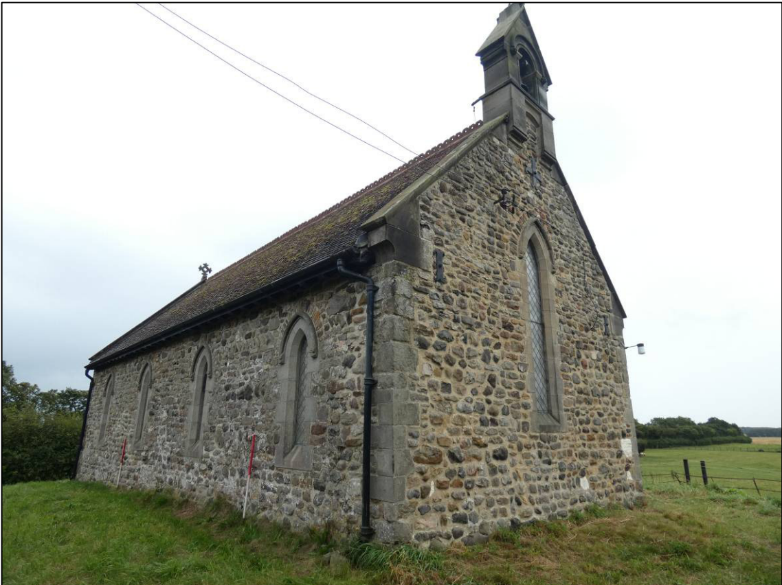
Plate 6: General view of chapel, looking SE (photo 1/960).
