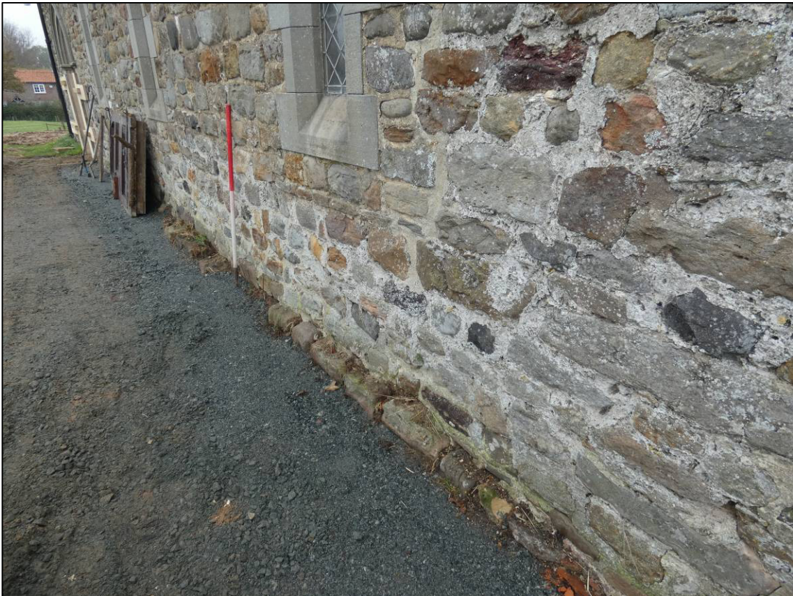
Plate 8: Plinth to central part of south elevation, looking W (photo 3/373).
