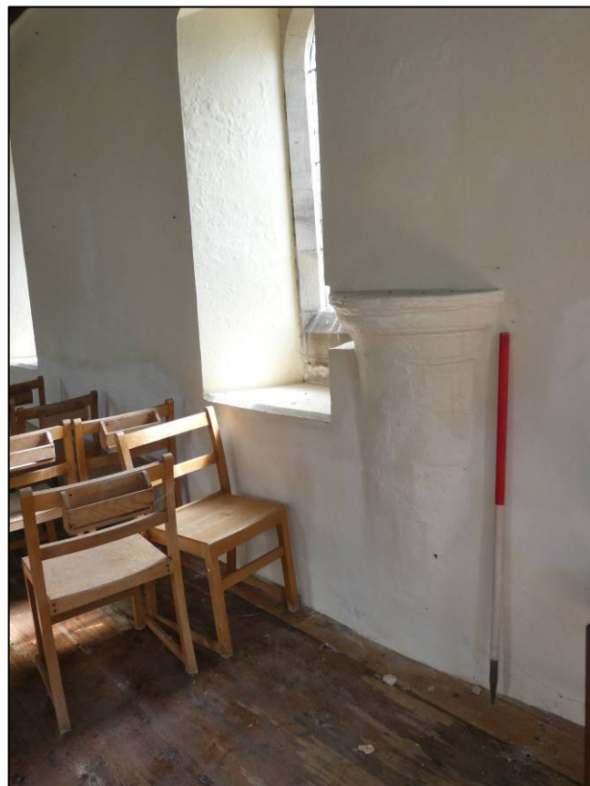
Plate 21: Internal face of south wall showing pier, looking SE (photo 1/033).
