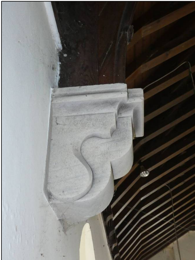
Plate 31: Internal roof structure, corbel to roof truss, looking W (photo 1/999).
