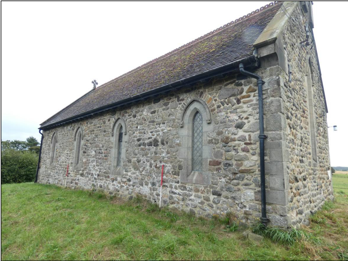
Plate 14: North elevation, looking SE (photo 1/961).
