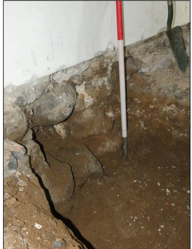
Plate 50: Internal Pit 4, showing foundations (204) on north chapel wall, looking NE.
