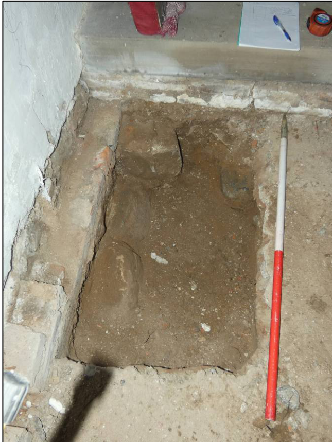
Plate 49: Internal Pit 1, showing brick sleeper wall (201) and foundations for chancel division (208), looking E.
