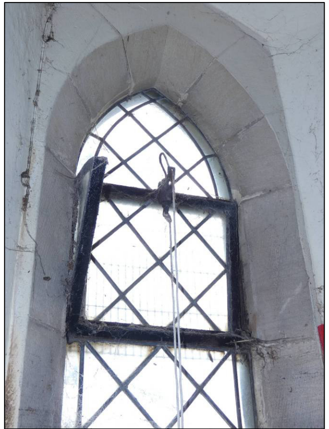
Plate 24: Central window to south wall, opening mechanism, looking SW (photo 1/013).
