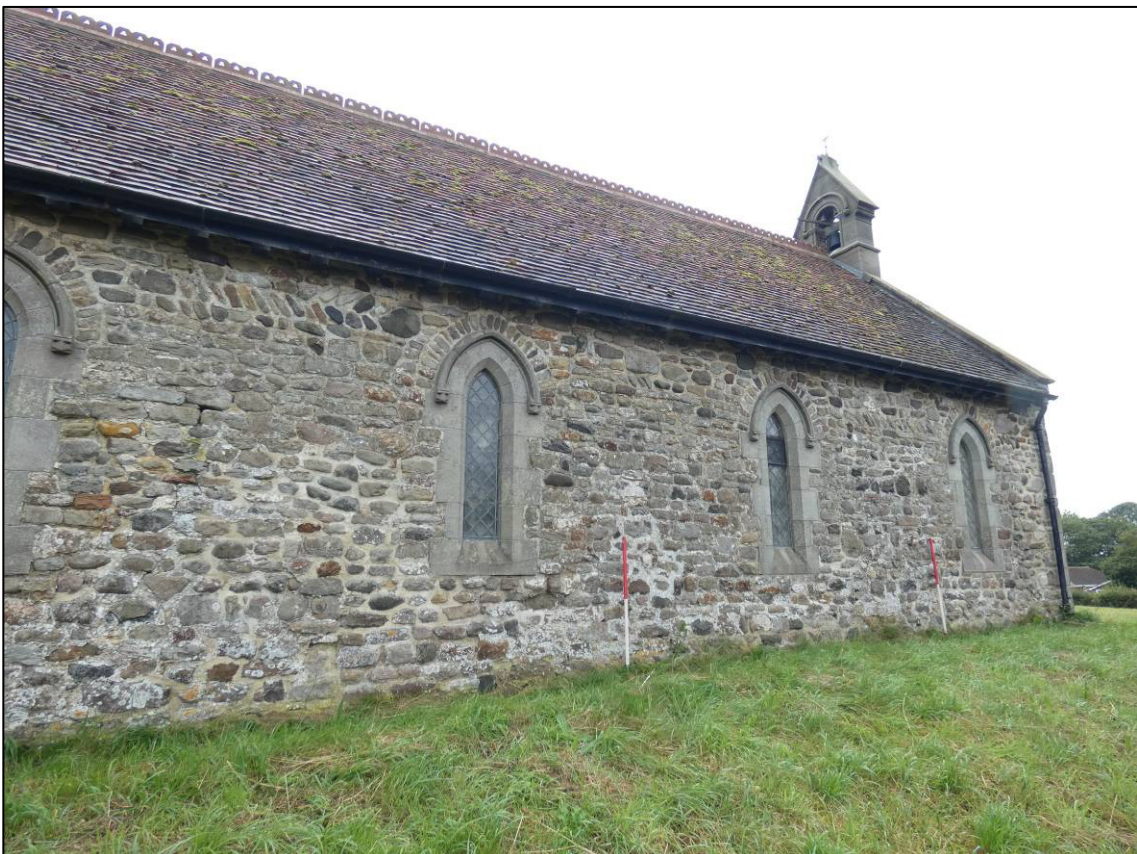
Plate 15: North elevation, looking SW (photo 1/964).
