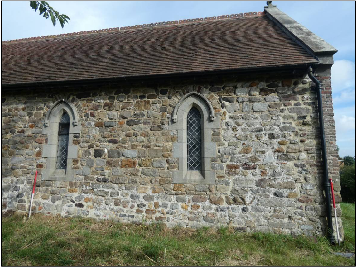
Plate 12: South elevation, east part, looking N (photo 1/943).
