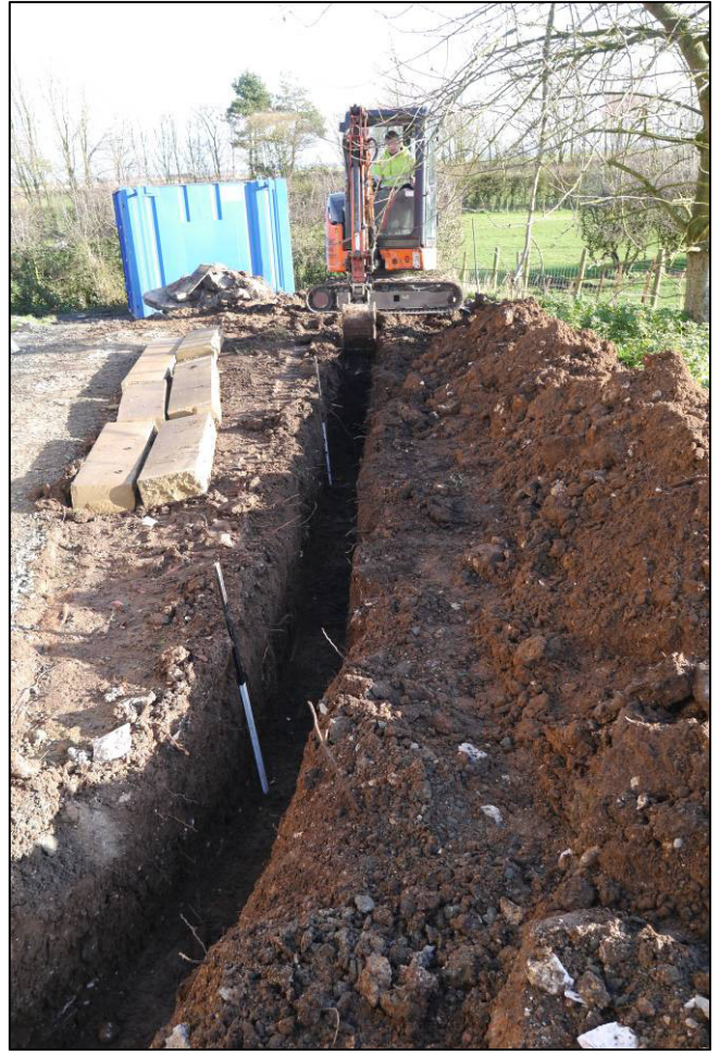
Plate 43: Trench 8, east end, looking E.
