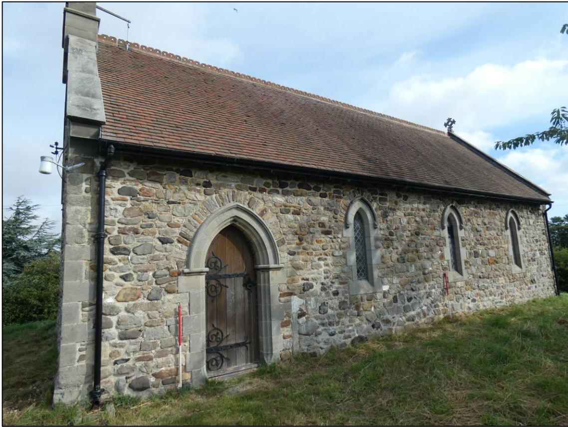
Plate 7: South elevation, looking NE (photo 1/951).
