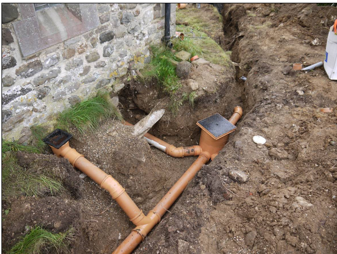
Plate 40: Trench 5, new drainage in position, showing earlier French drain (105), looking SW.
