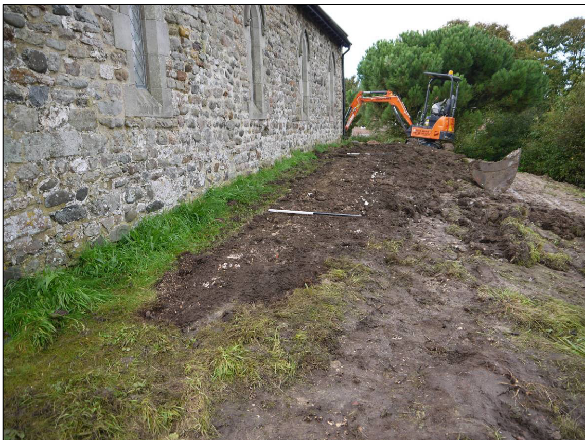
Plate 41: Levelling along north side of chapel, looking W.
