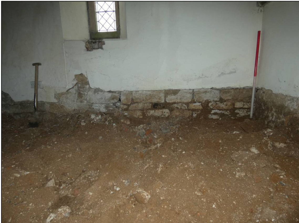
Plate 53: Exposed lower courses of north chancel wall after removal of chancel steps, looking N.
