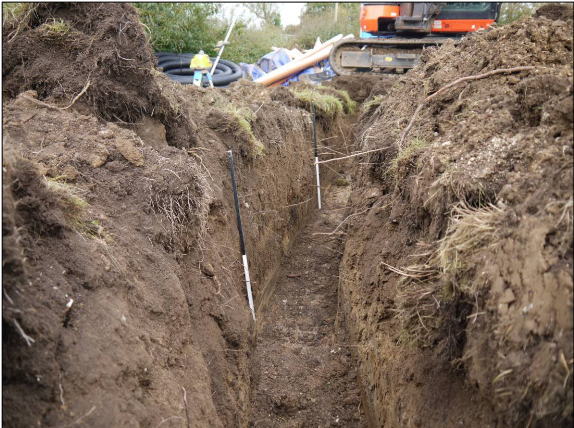
Plate 44: Trench 7, east end, looking E.
