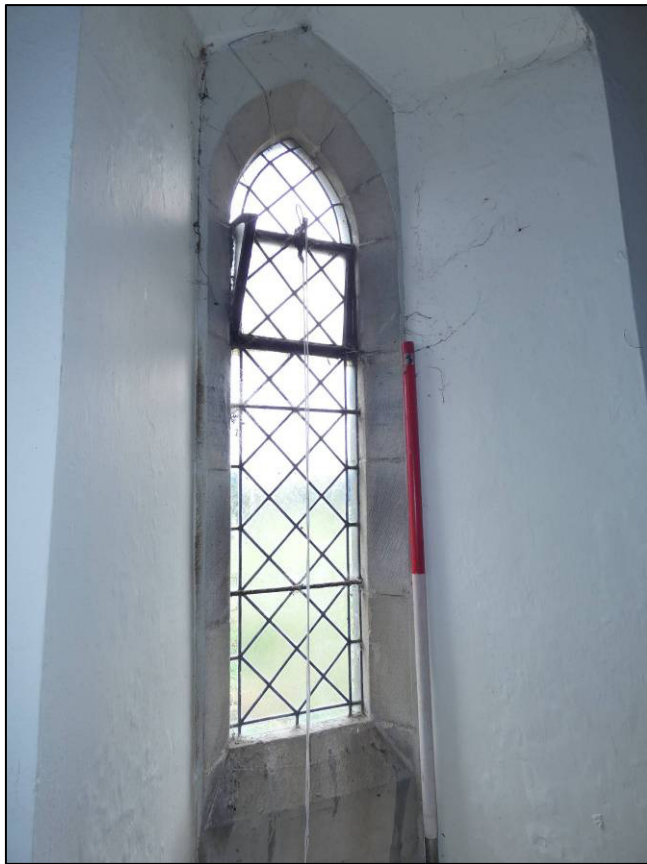
Plate 23: Central window to south wall, looking SW (photo 1/007).
