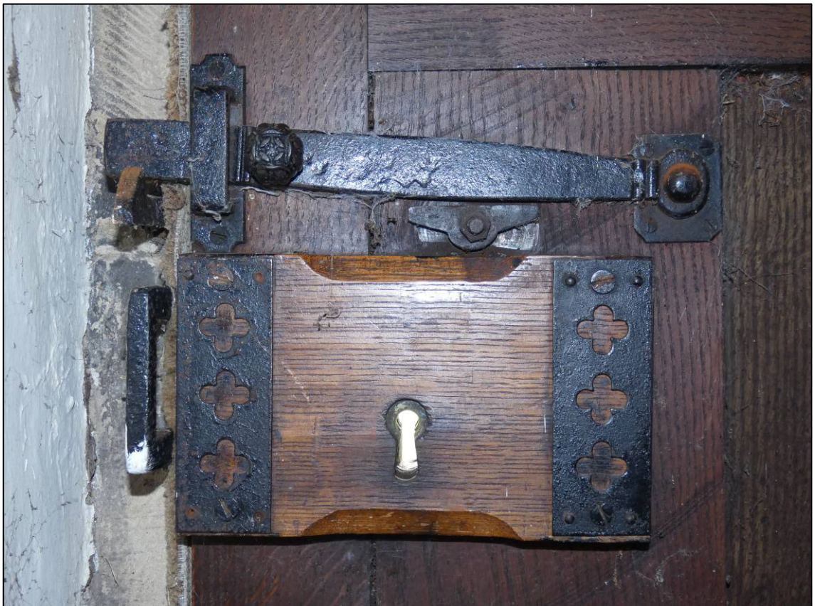
Plate 17: Lock on internal face of south doorway, looking S (photo 1/024).
