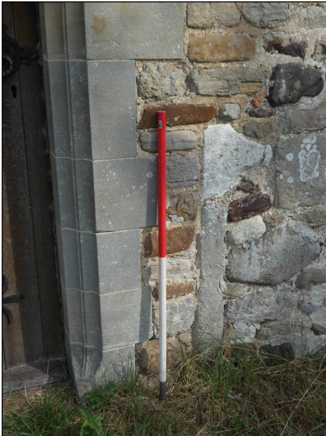
Plate 10: South elevation, earlier jamb to east of door, looking N (photo 1/953).
