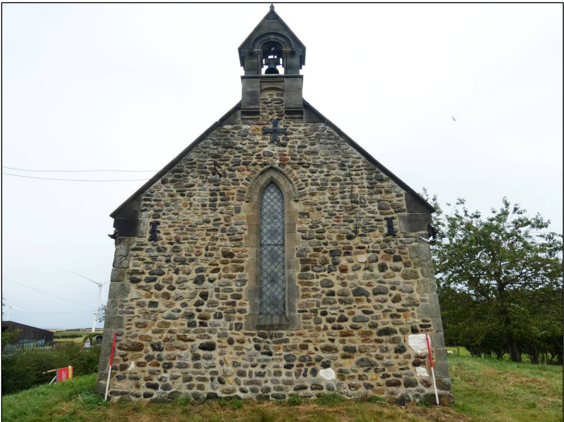
Plate 13: West gable, looking E (photo 1/956).
