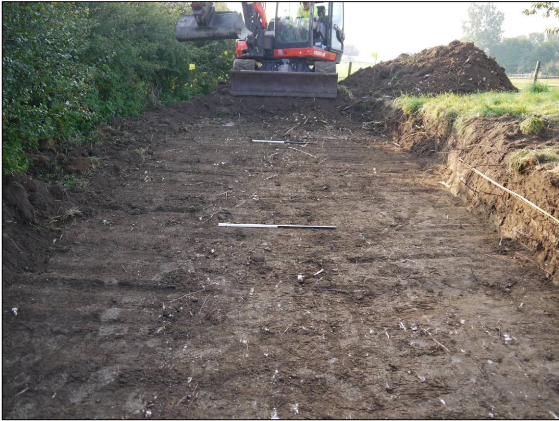
Plate 33: Trench 1, general view of central area, looking S.
