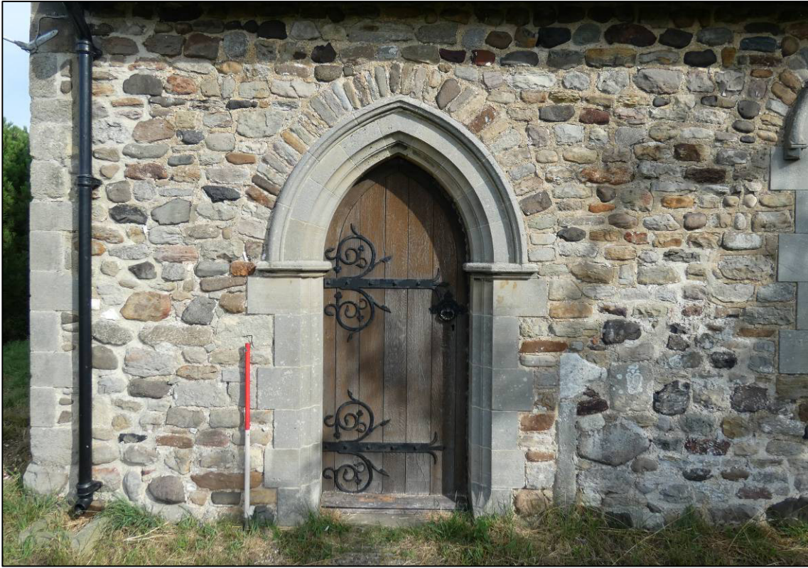
Plate 9: South elevation, south door, looking N (photo 1/952).
