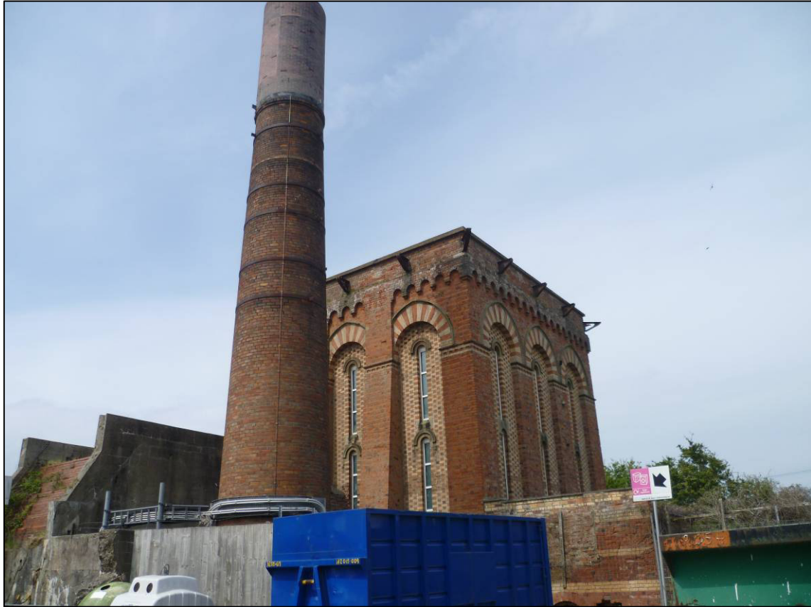
Plate 1: Former Hornsea Water Treatment Works building (rear) with incinerator and chimney to front (Site 5), looking NW.
