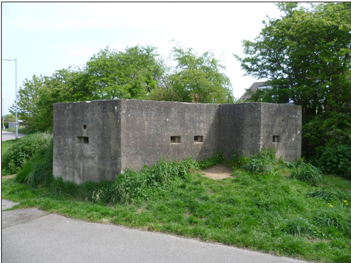
Plate 2: Lozenge-type pillbox, north of Northgate (Site 9), showing entrance blast wall to west side, looking E.
