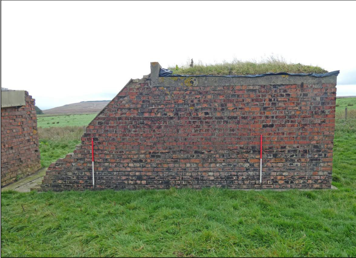
Plate 3: Shelter, south external elevation, looking NE (photo 1/069).
