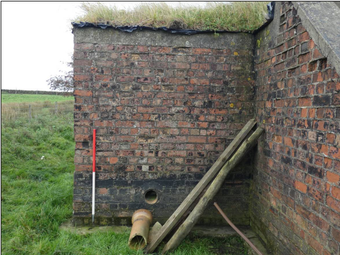
Plate 6: Shelter, return to north external elevation, looking SE (photo 1/079).
