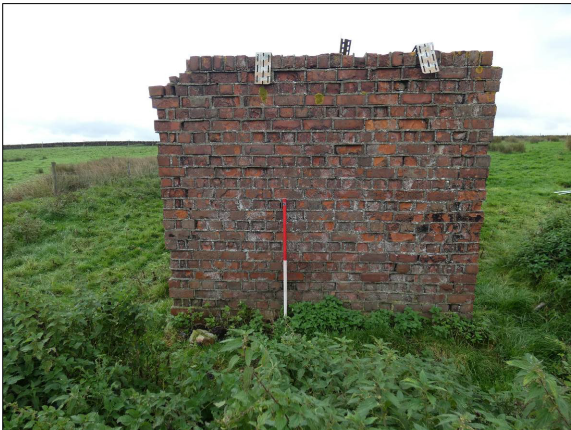
Plate 8: Shelter, west elevation of blast wall, looking SE (photo 1/068).
