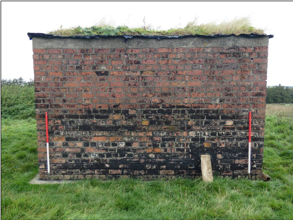
Plate 4: Shelter, east external elevation, looking NW (photo 1/075).
