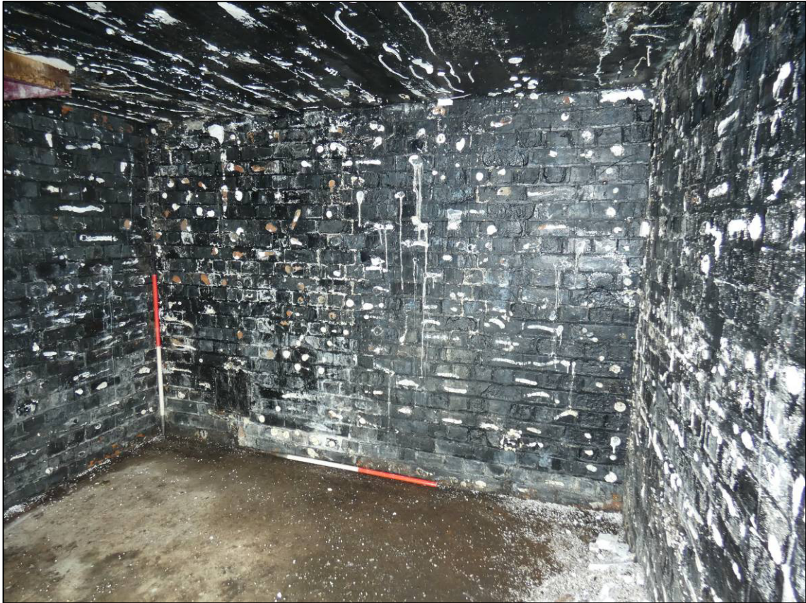
Plate 16: Shelter, east internal wall after stripping out, looking E (photo 2/401).
