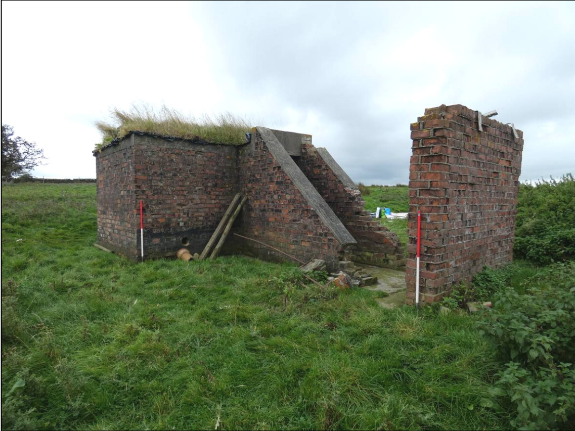
Plate 1: Shelter and blast wall, looking S (photo 1/067).
