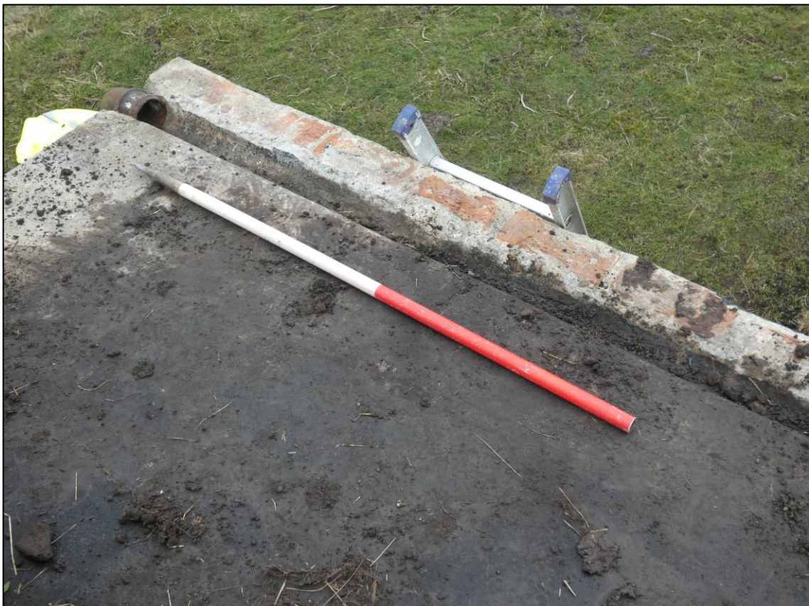
Plate 10: Shelter, roof after removal of turf showing drain to the east side, looking E (photo 2/414).
