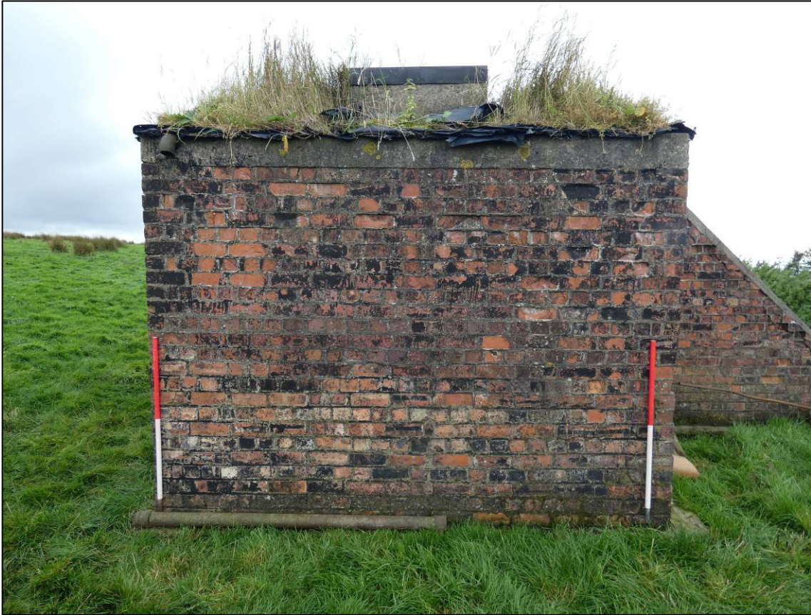
Plate 5: Shelter, north external elevation, looking SW (photo 1/076).
