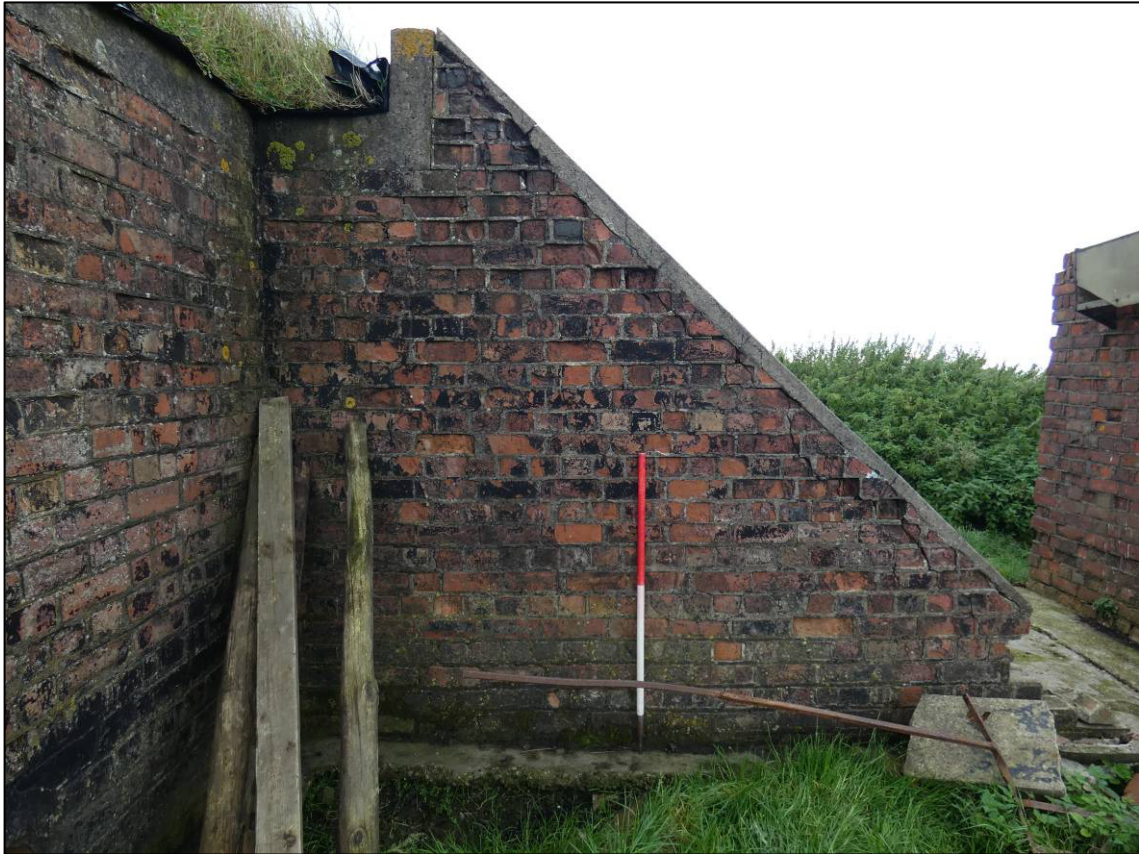
Plate 7: Shelter, north external elevation, sloping wall to entrance, looking SW (photo 1/080).
