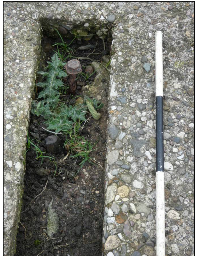
Plate 20: Hut base, slot to porch showing detail of fixings, looking SE (photo 1/099).
