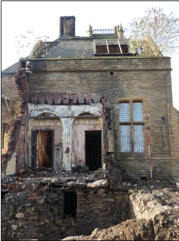
Plate 15: East elevation after demolition, looking W (photo 2/159).
