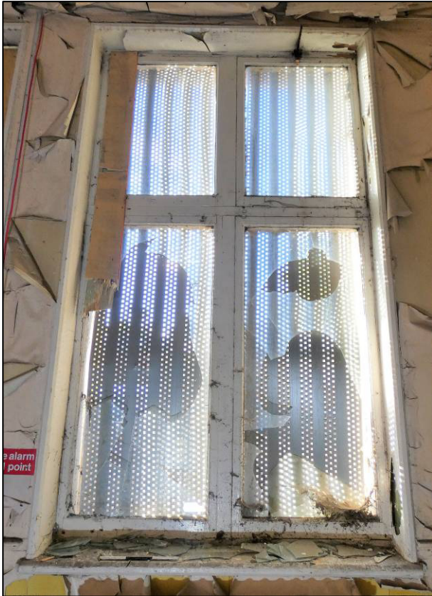
Plate 3: Ground floor corridor (G3), Type 2 window (G3/2), at east end of south side, looking S (photo 1/728).
