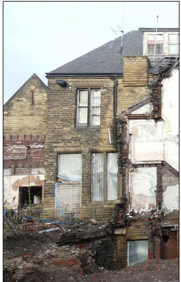
Plate 22: West end of south elevation after demolition, looking N (photo 2/195).
