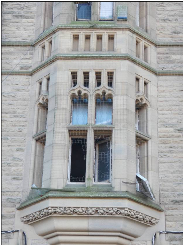
Plate 8: First floor oriel window to central tower (1F5), looking S (photo 1/752).
