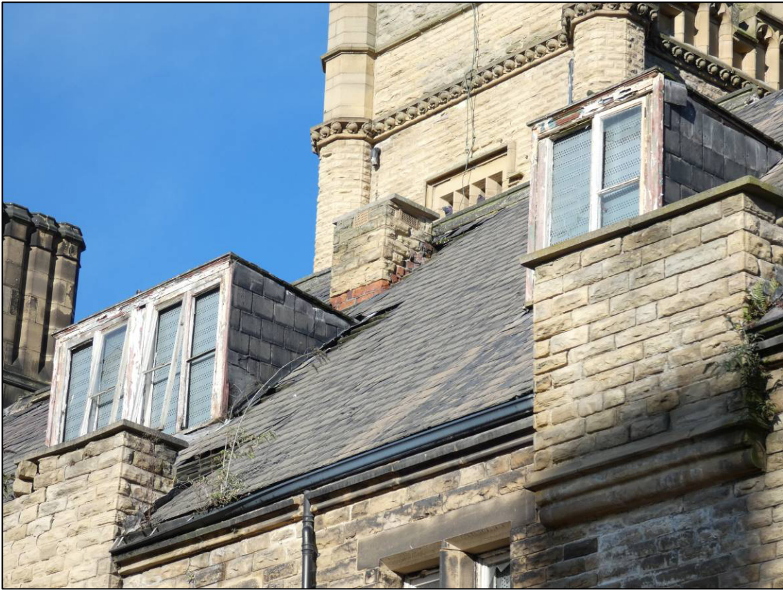
Plate 13: Second floor rooms (2F2 and 2F4), dormer windows, looking NW (photo 1/765).
