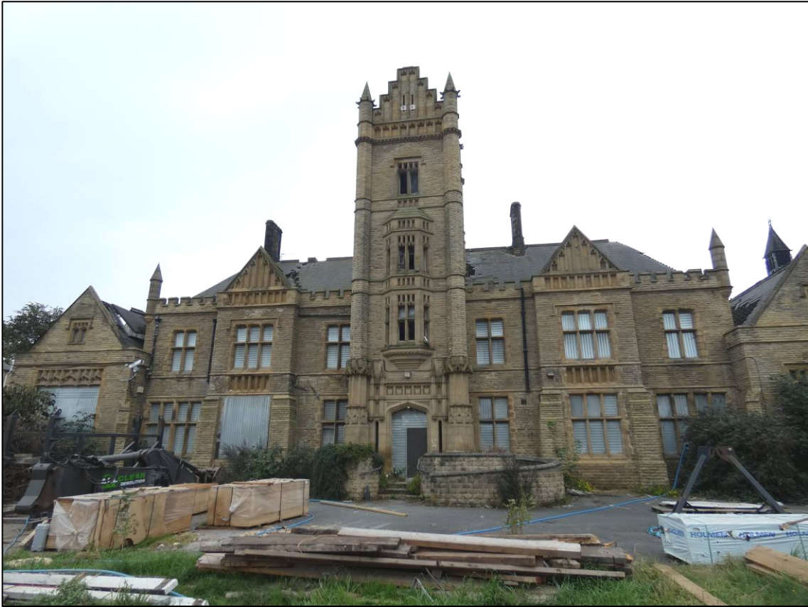
Plate 1: Front (north) elevation of retained building, looking SE.
