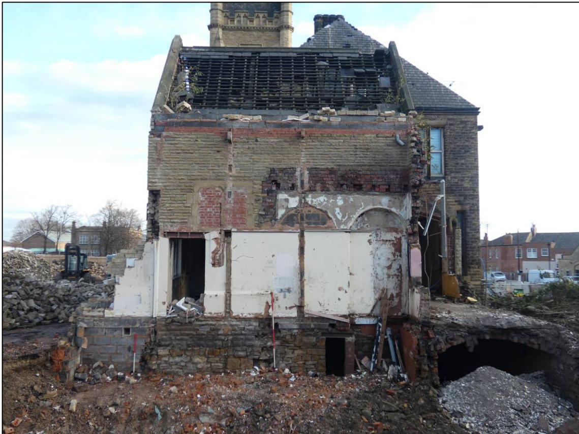
Plate 24: West elevation after demolition, looking E (photo 2/141).
