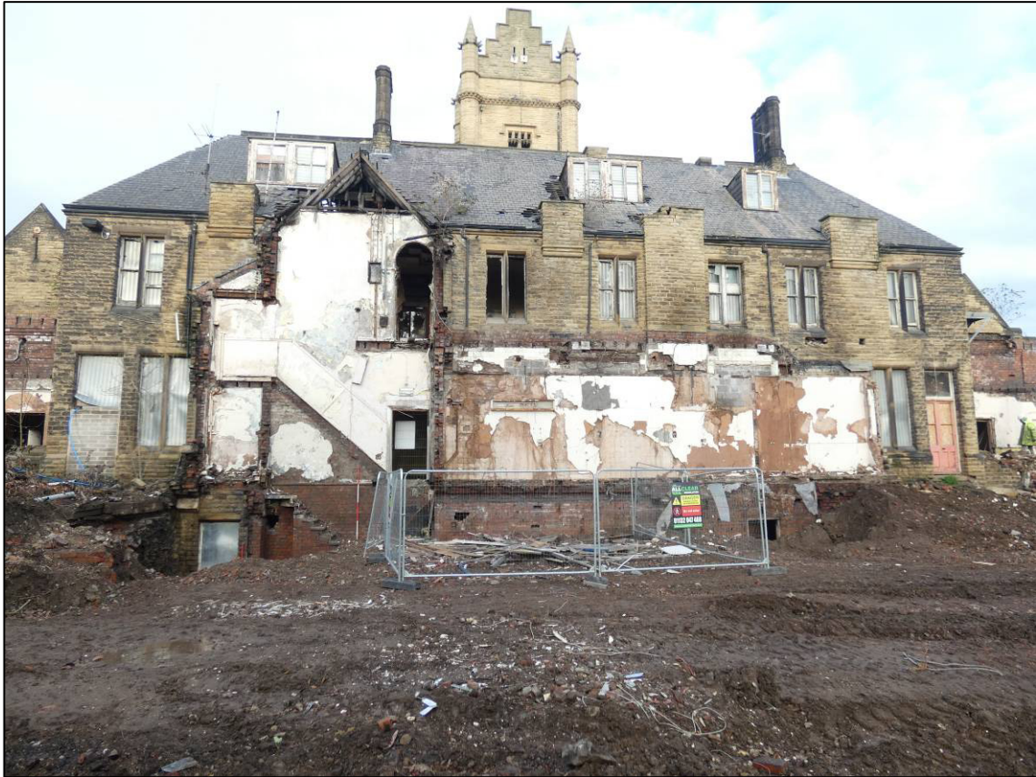
Plate 20: South elevation after demolition, looking N (photo 2/197).
