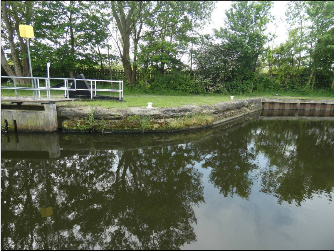
Plate 3: West approach, south wing wall to top gates, looking S (photo 1/723).
