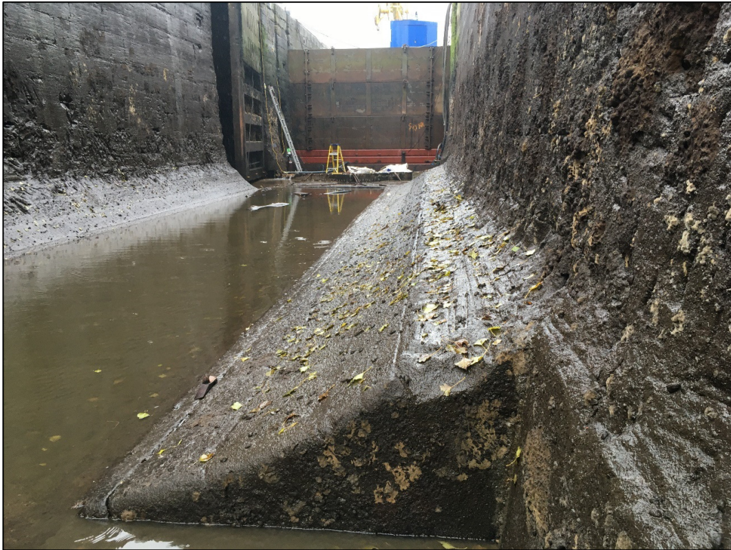
Bottom chamber, lower part, from disused gate recess showing masonry fillets.
