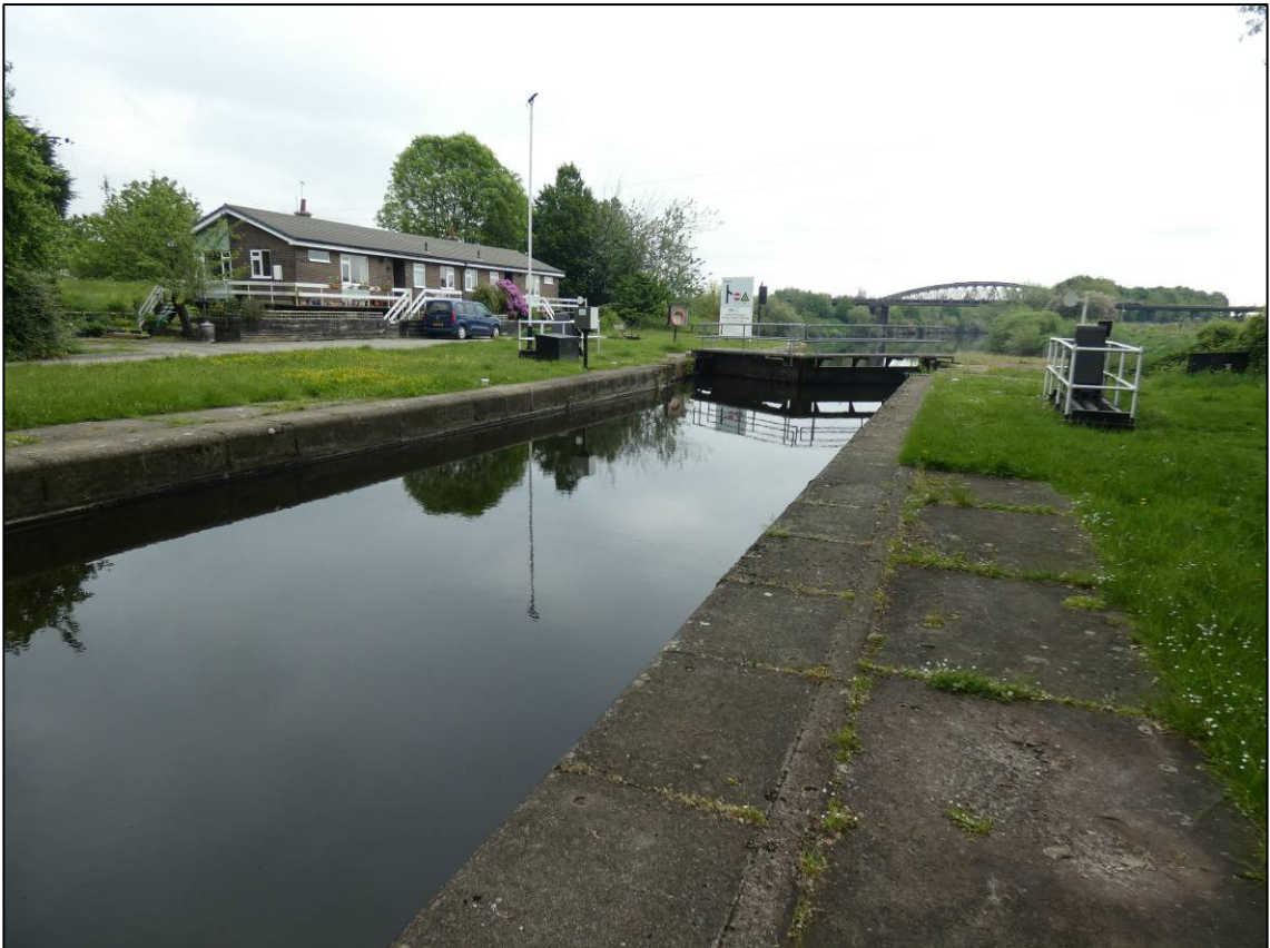
Plate 12: East end of bottom chamber, looking NE (photo 1/754).
