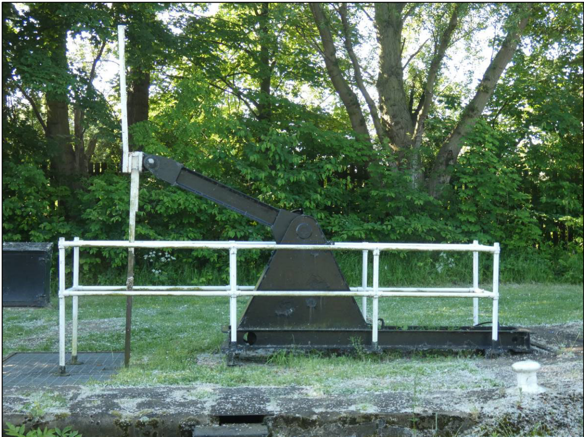
Plate 10: Sluice donkey, south side of middle gates, looking S (photo 2/768).
