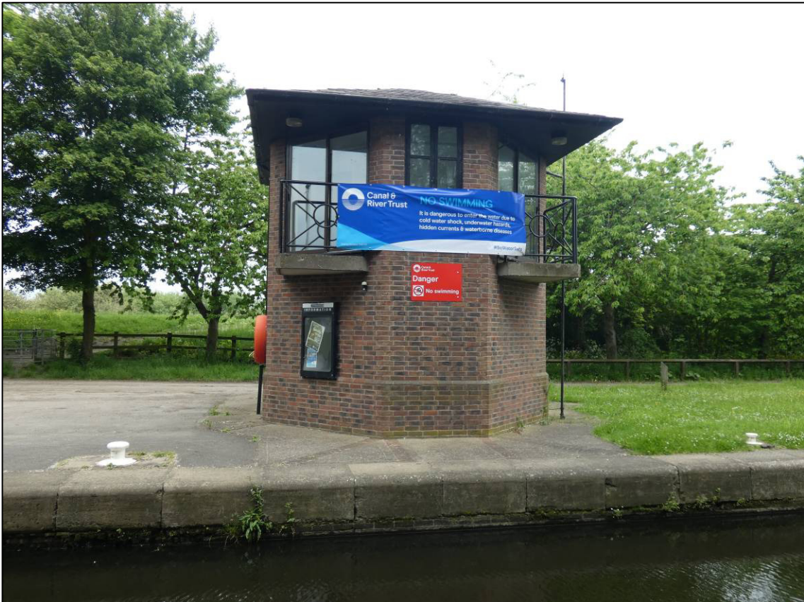
Plate 20: Lock lobby, north side of bottom chamber, looking N (photo 1/756).
