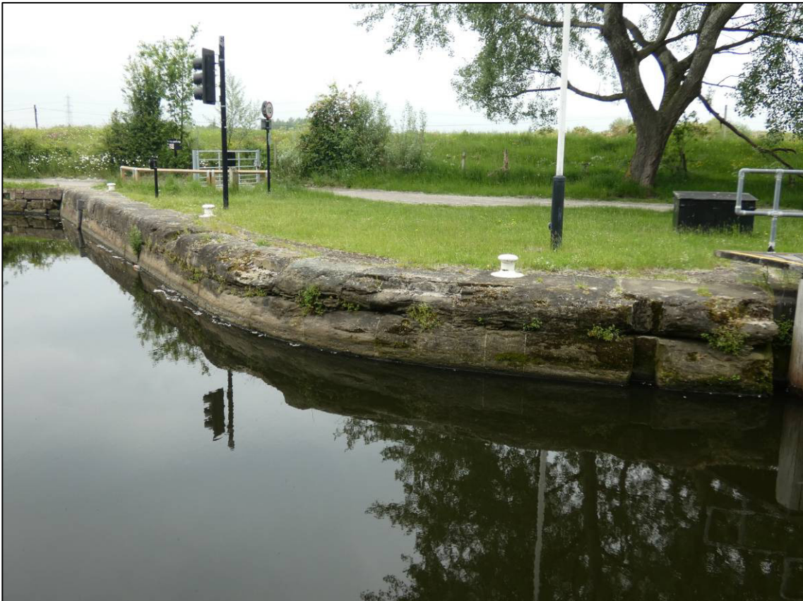
Plate 2: West approach, north wing wall to top gates, looking N (photo 1/760).
