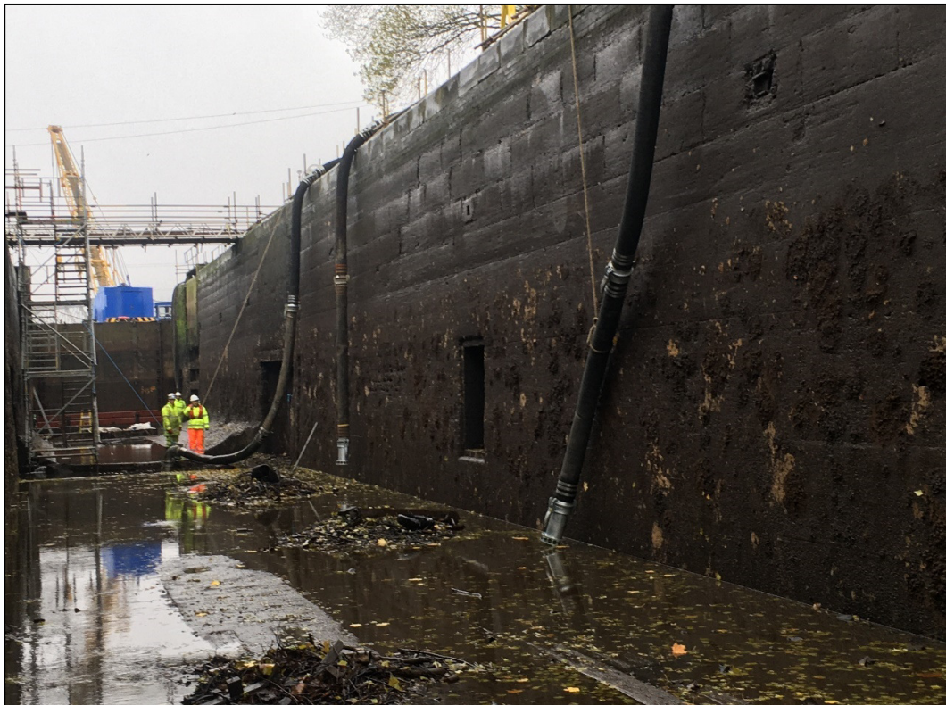
Bottom chamber, south wall showing culverts.
