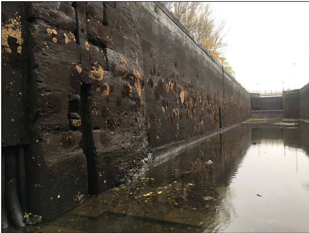
Top chamber, south wall, showing boat impact at middle gates narrows.
