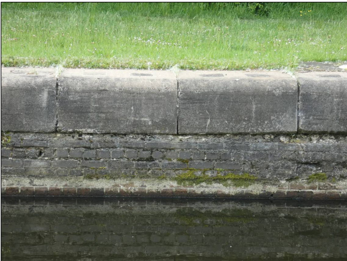
Plate 6: South wall to top chamber, looking S (photo 1/727).
