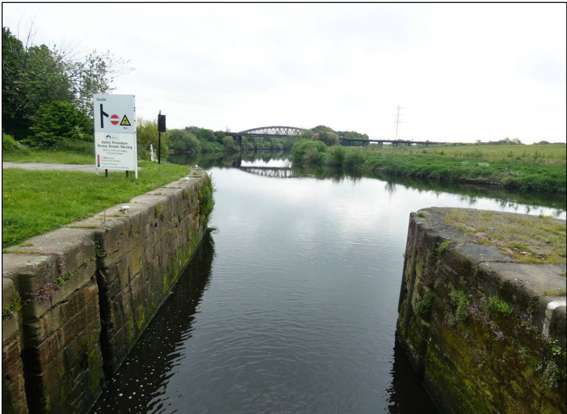
Plate 22: East approach from River Aire, showing 1878 railway bridge, looking E (photo 1/741).
