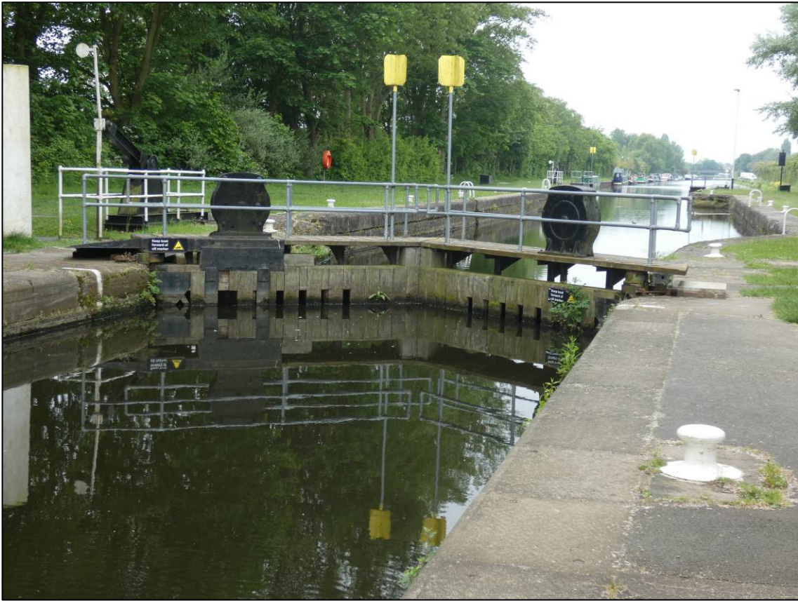
Plate 9: Middle gates (closed), looking W (photo 1/735).
