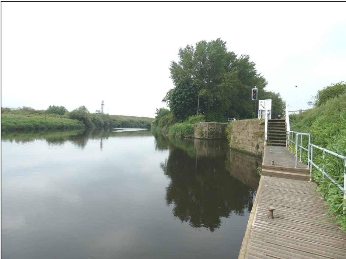
Plate 18: East approach from River Aire, showing landing to north side, looking W (photo 1/751).
