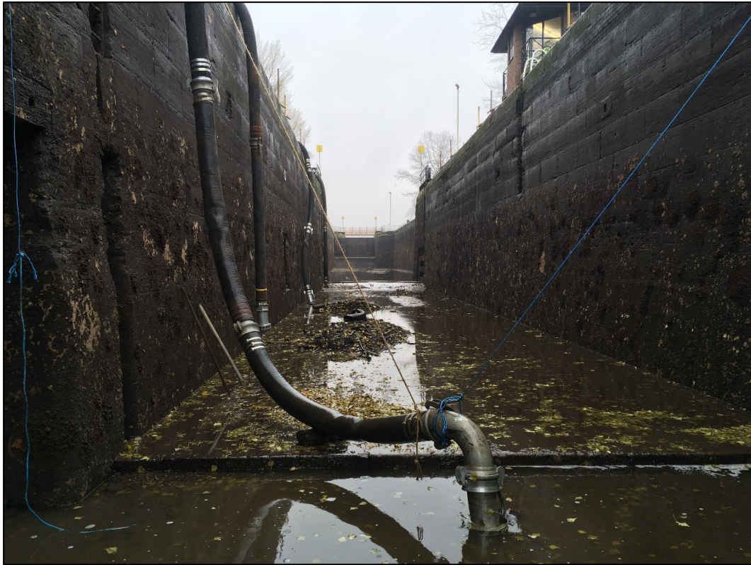
Bottom chamber, upper part, showing original timber cill from disused gates.
