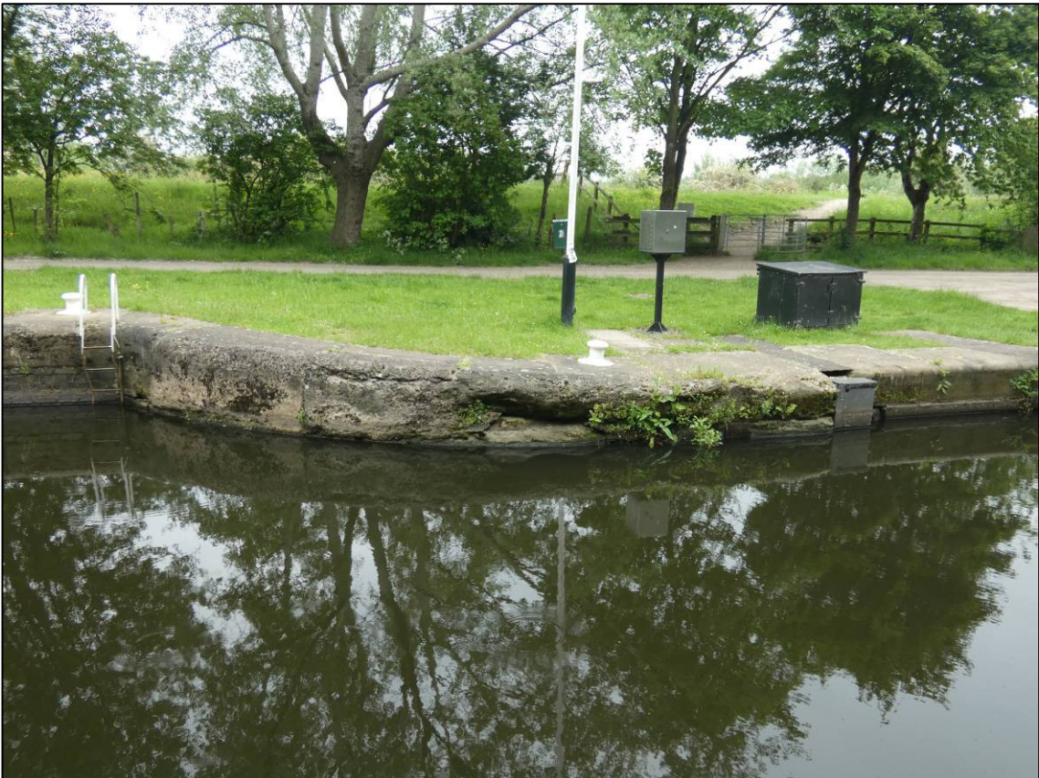
Plate 8: North wall of approach to middle gates, looking N (photo 1/758).
