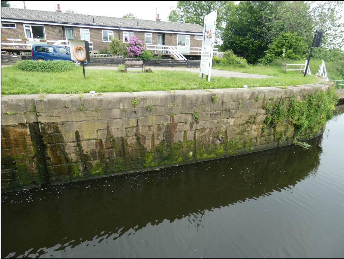
Plate 17: North wall of east approach, looking N (photo 1/749).
