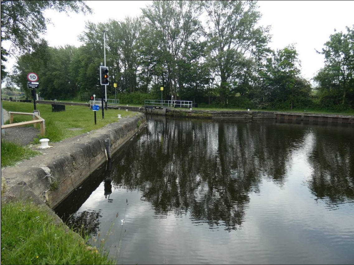
Plate 1: West approach, wing walls to top gates, looking SE (photo 1/718).
