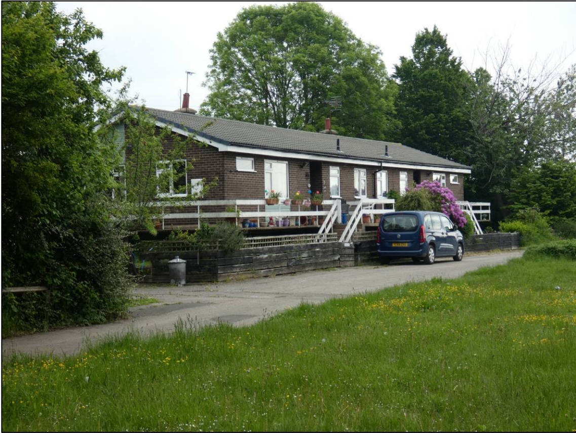
Plate 21: 1968 residential properties, north side of bottom gates, looking NE (photo 1/738).
