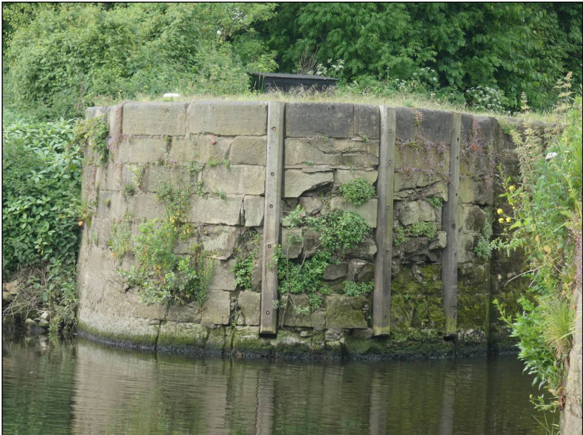
Plate 16: Bullnose end to south wall of east approach, looking SW (photo 1/753).
