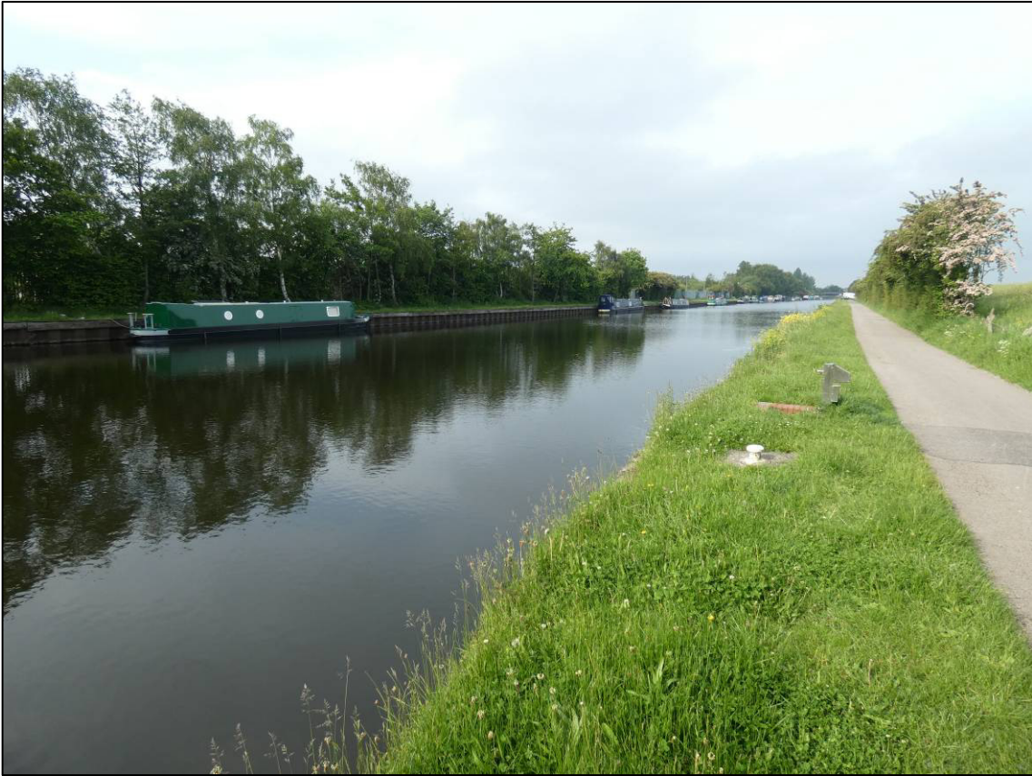
Plate 19: View down Castleford Cut from near lock, looking W (photo 1/717).
