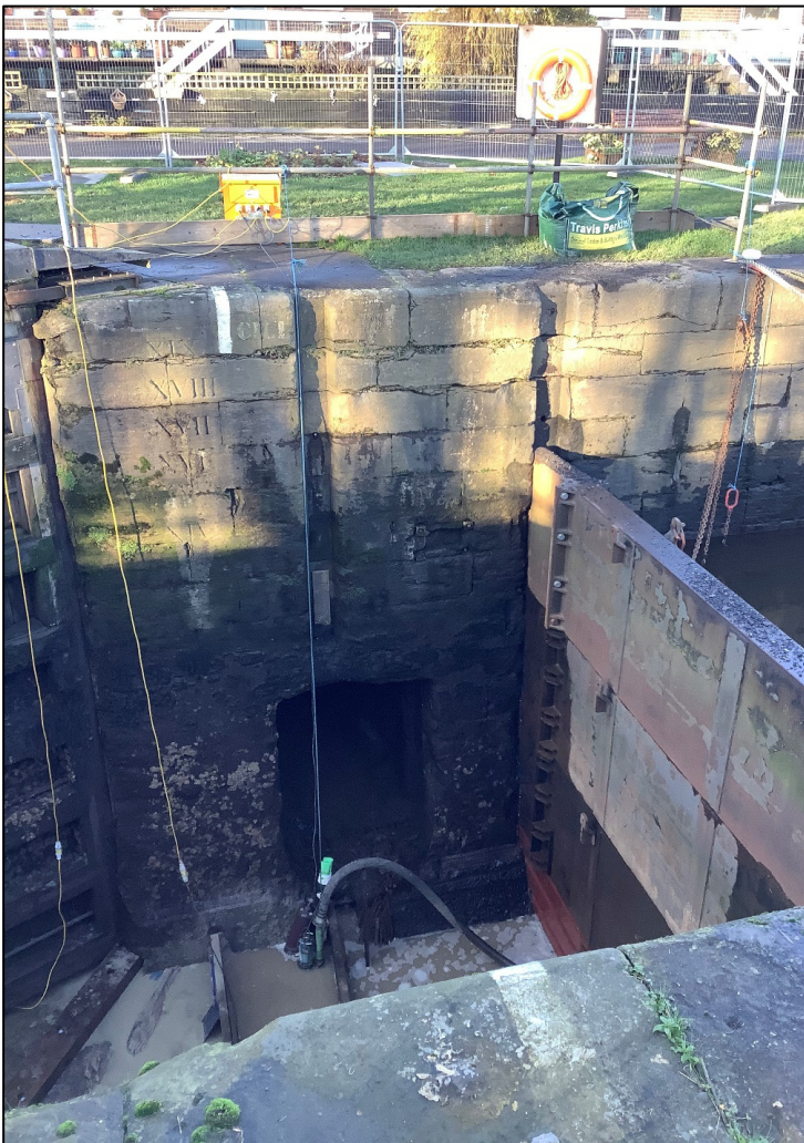
Bottom chamber, lower part, from disused gate recess showing masonry fillets.
