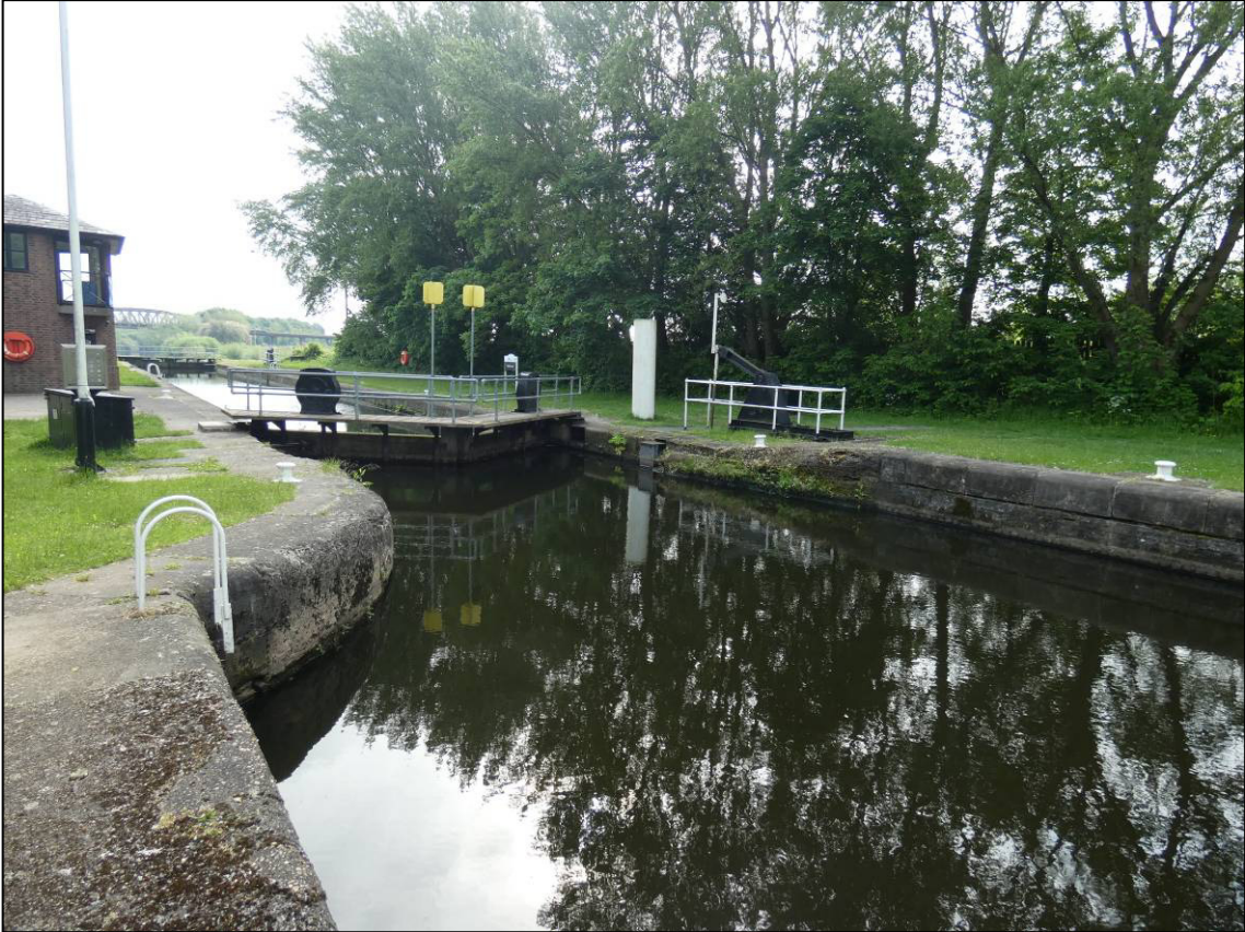
Plate 7: Approach to middle gates, looking SE (photo 1/731).
