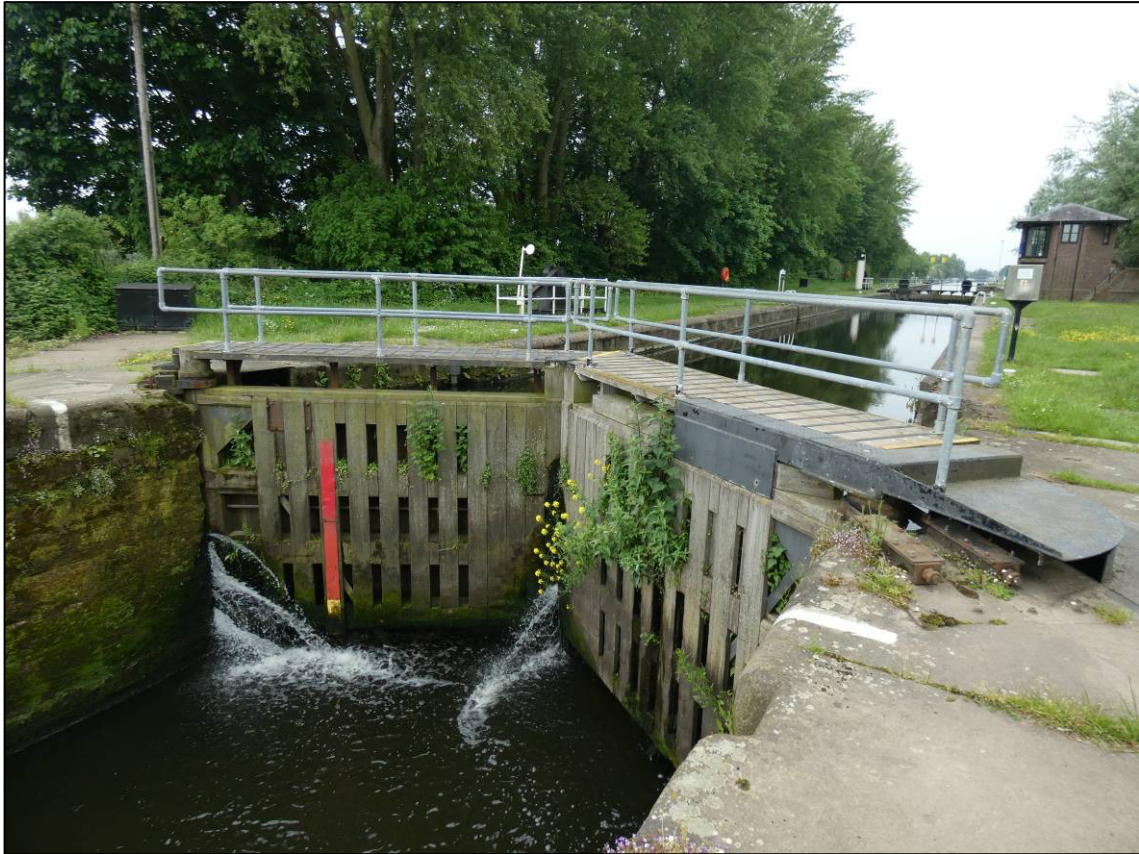
Plate 13: Bottom gates (closed), looking W (photo 1/739).
