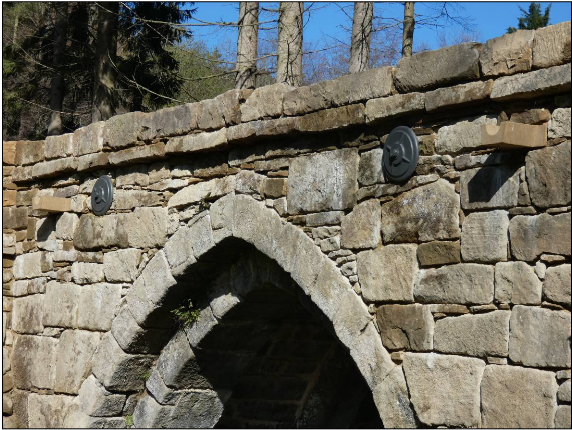
Plate 35: South elevation, details, of drains and ties, looking NW (photo 8/582).
