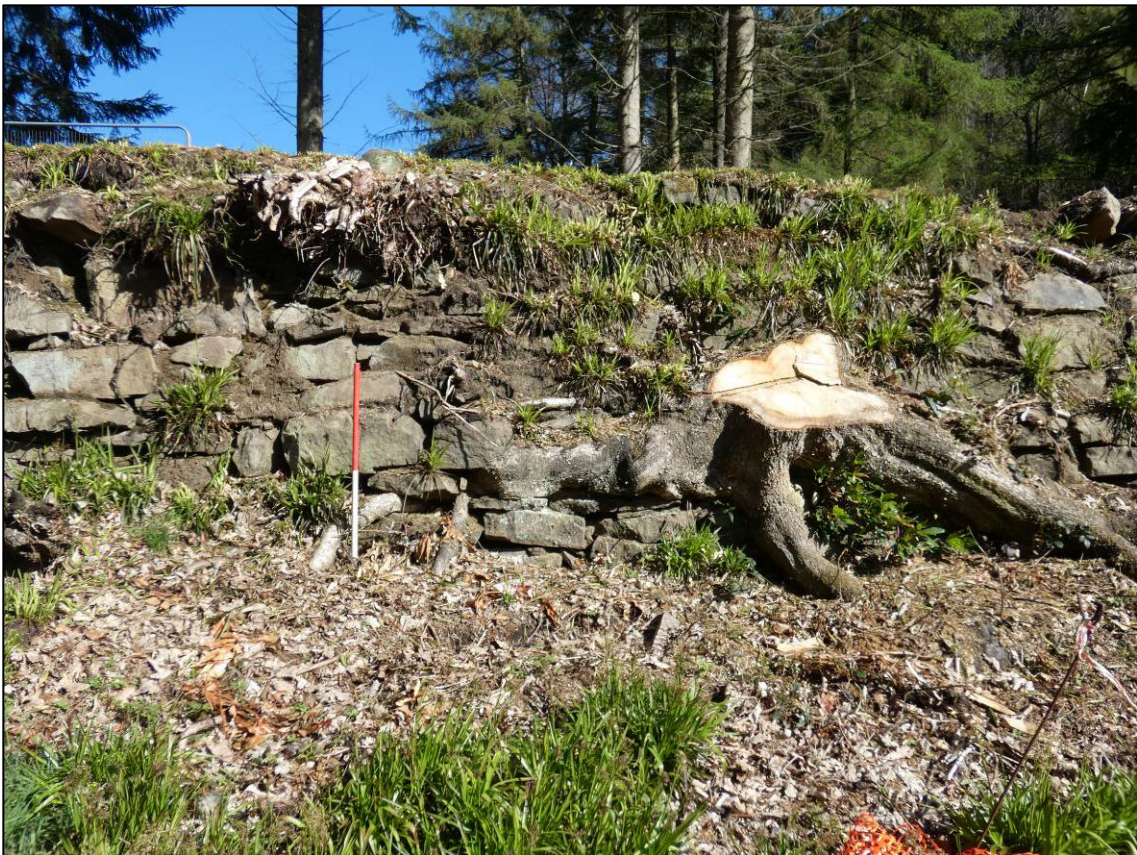
Plate 18: South elevation, section of west abutment, looking N (photo 8/574).
