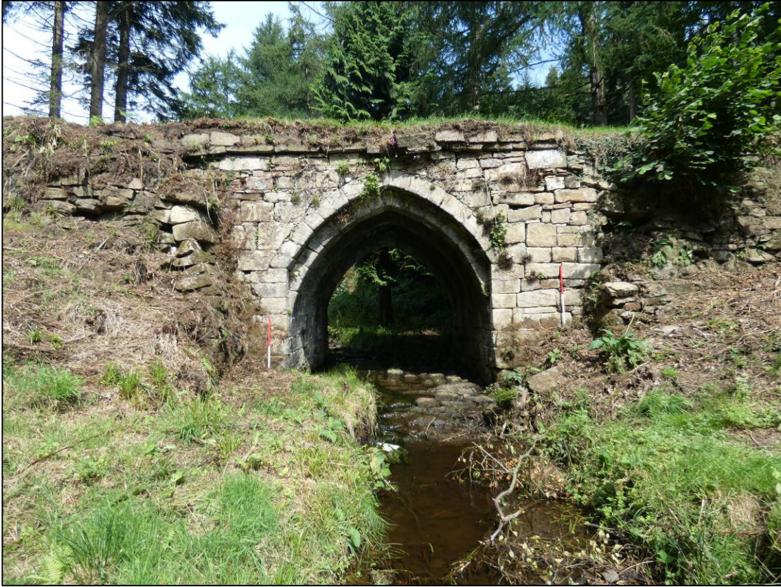
Plate 8: South elevation, prior to repairs, looking N (photo 1/883).
