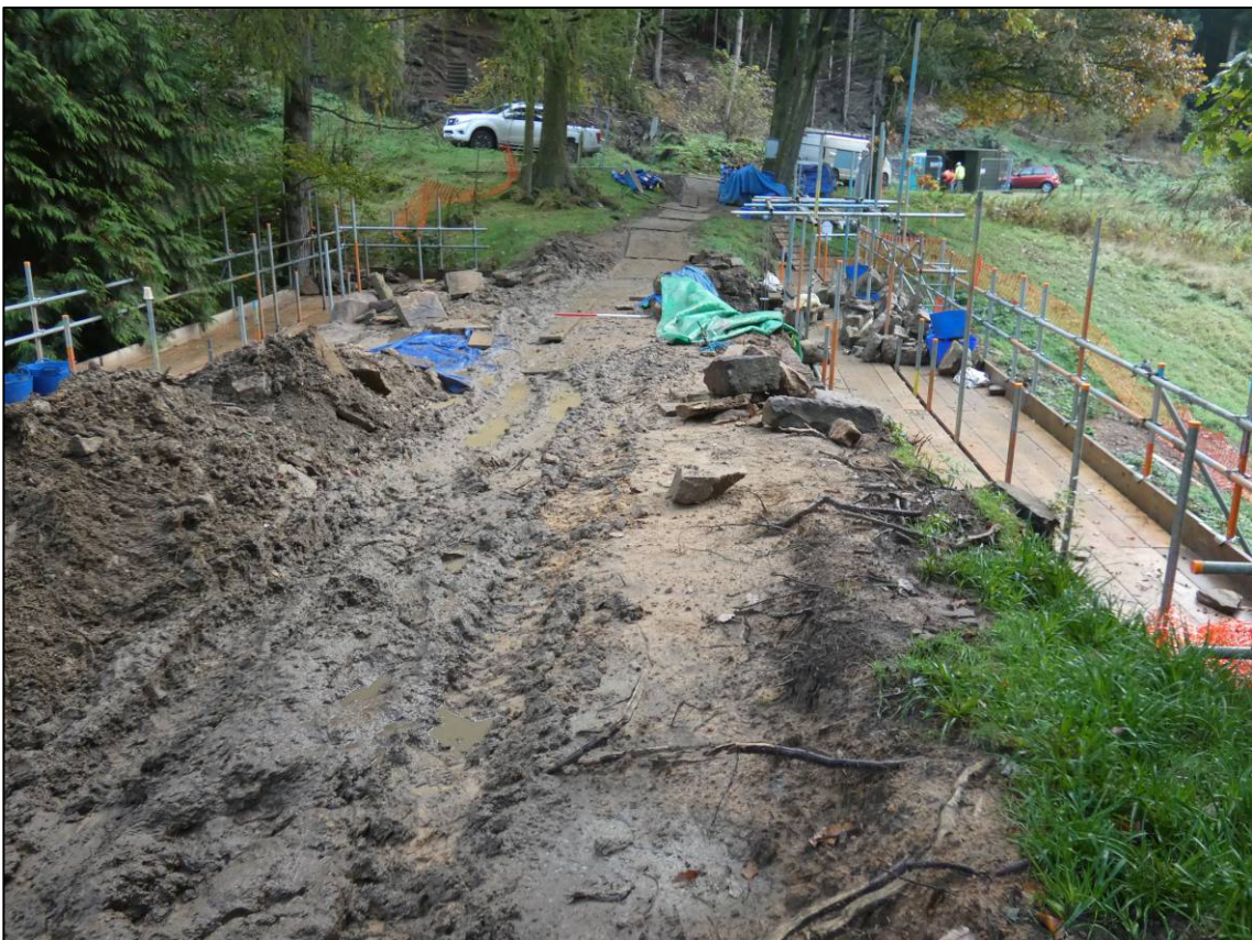
Plate 20: Surface of bridge after ground reduction, looking E (photo 3/287).
