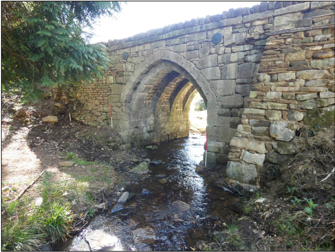
Plate 33: North elevation, repairs complete, looking SE (photo 8/593).
