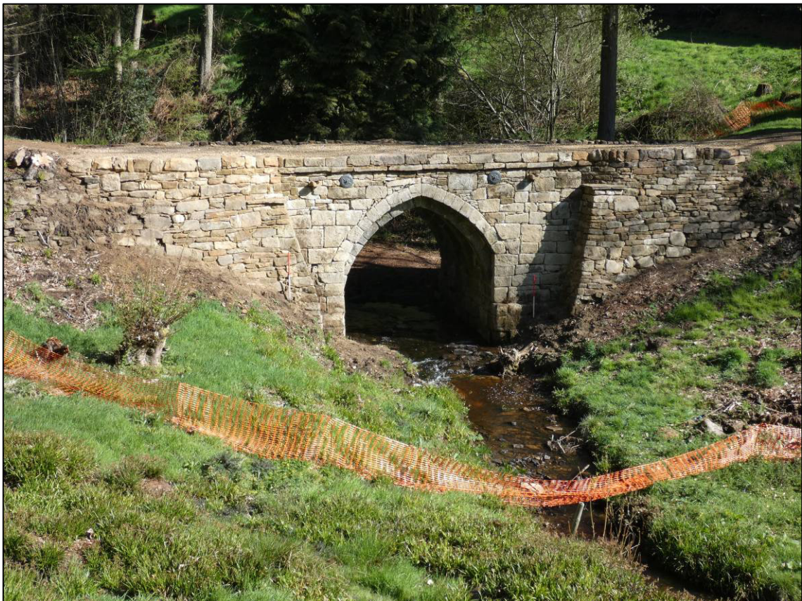
Plate 34: South elevation, repairs complete, looking N (photo 8/566).
