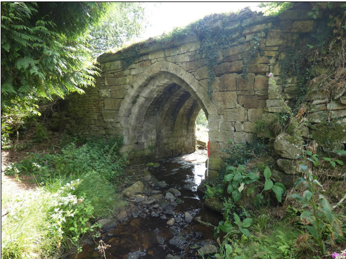
Plate 9: North elevation, prior to repairs, looking SE (photo 1/907).
