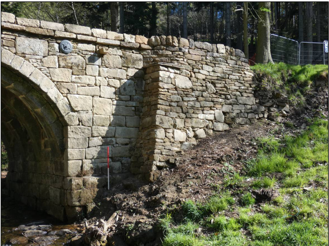
Plate 28: South elevation, east abutment and buttress/return, repairs complete, looking NE (photo 8/572).
