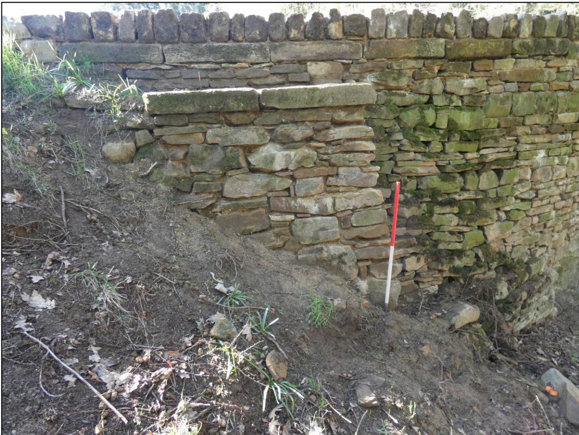
Plate 24: North elevation, east buttress/return after repairs, looking S (photo 8/587).
