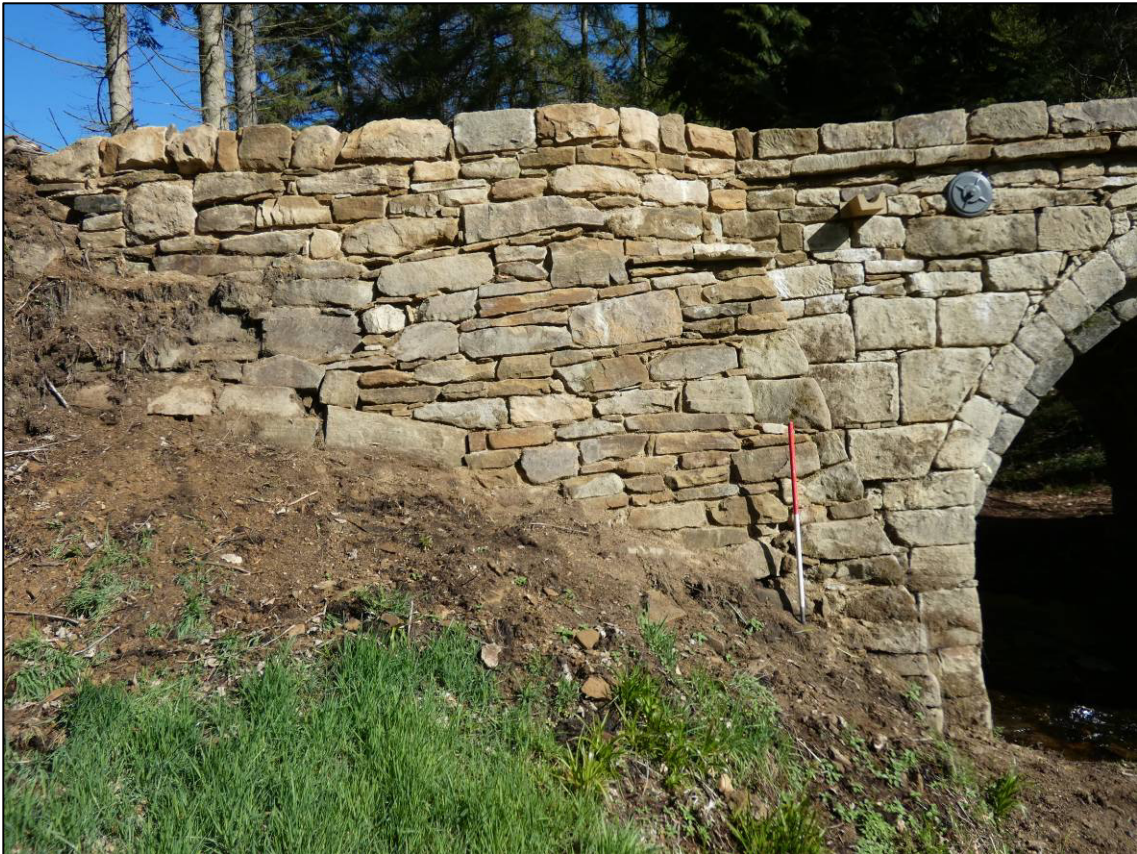
Plate 29: South elevation, west abutment and buttress/return, repairs complete, looking N (photo 8/570).
