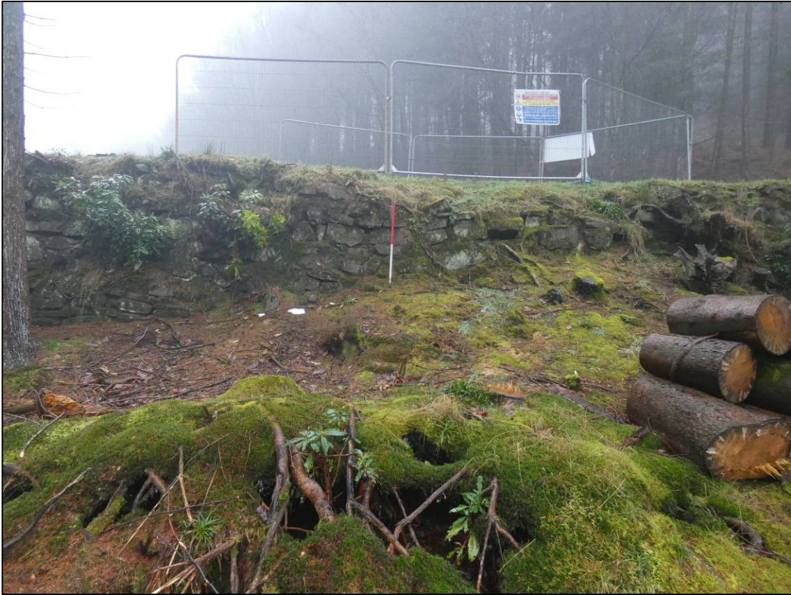
Plate 12: North elevation, west abutment, looking S (photo 7/064).
