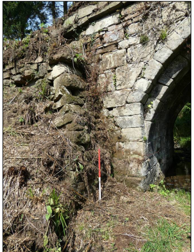
Plate 16: South elevation, west buttress/return, prior to repair, looking NW (photo 1/898).
