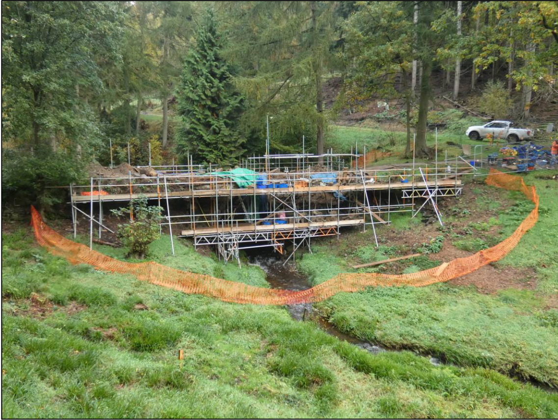
Plate 19: South elevation undergoing repair, looking NE (photo 3/316).
