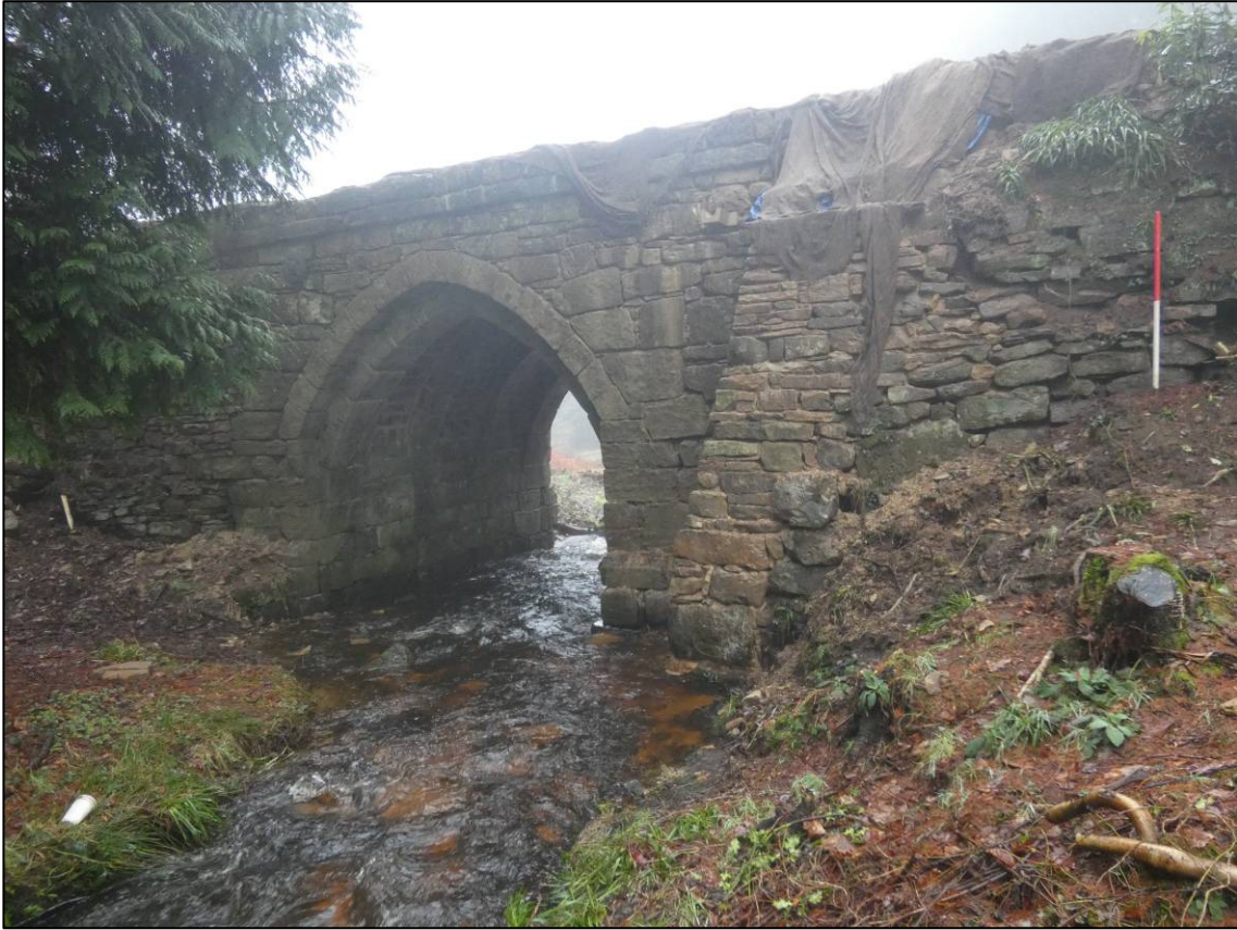
Plate 23: North elevation after repairs, showing rebuilt west buttress/return, looking SE (photo 7/068).
