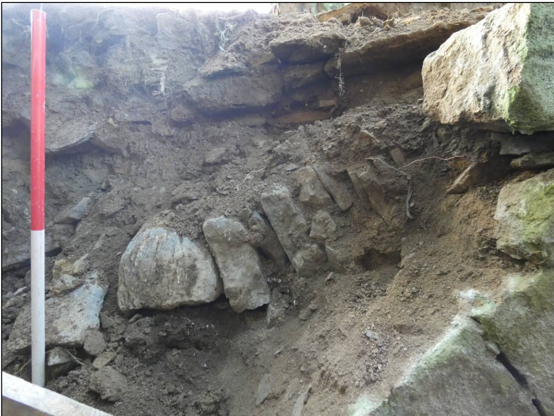
Plate 22: North elevation, area east of arch during clearance, showing section of relieving arch in section, looking S (photo 2/118).
