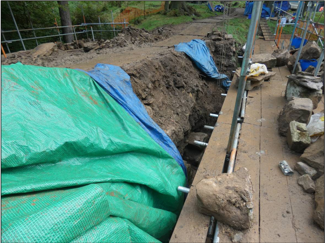
Plate 27: South elevation, under repair, looking E (photo 3/288).
