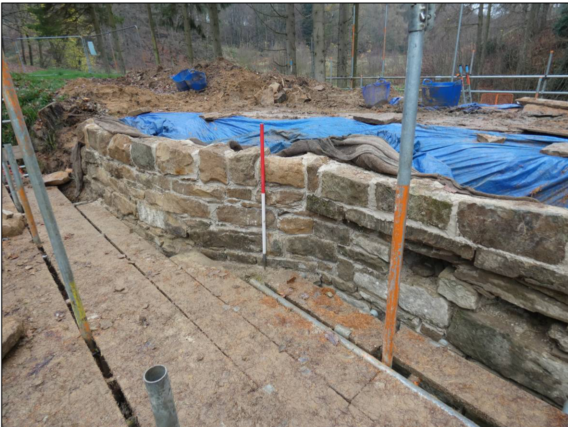
Plate 30 South elevation, rebuilt parapet to west of arch, looking NW (photo 5/633).
