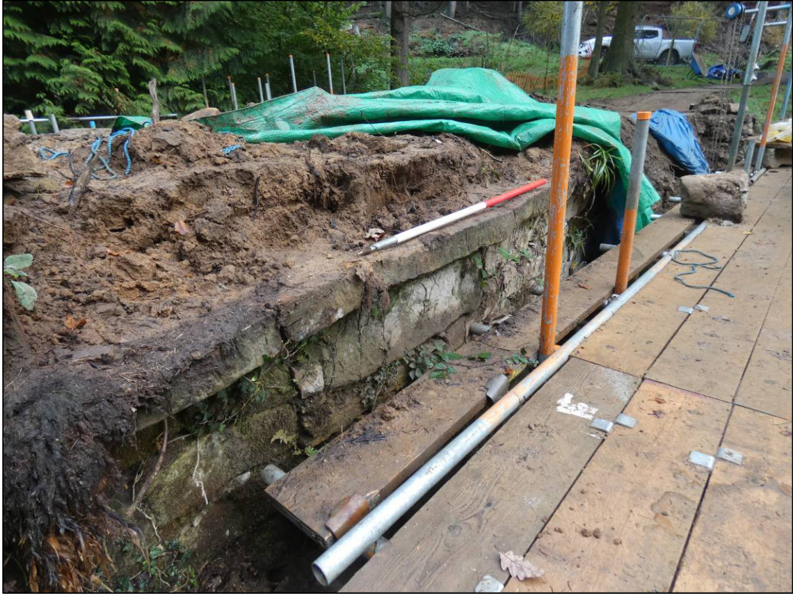
Plate 14: South elevation under repair, showing exposed stringcourse, looking NE (photo 3/290).
