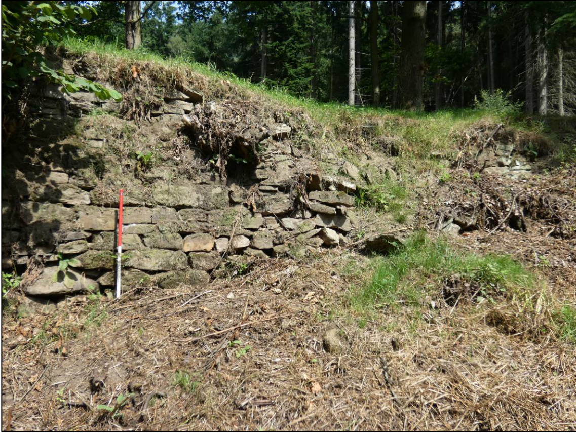
Plate 17: South elevation, east abutment, looking E (photo 1/905).
