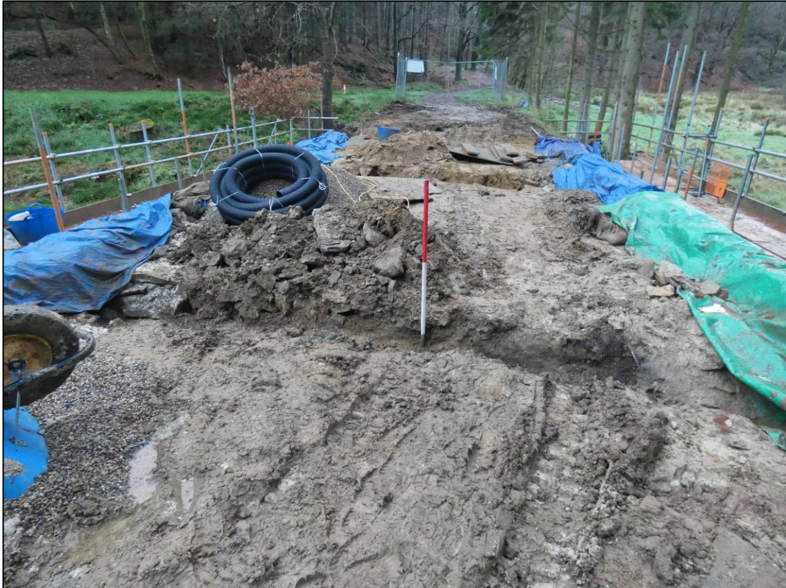
Plate 31: Excavated east trench (Trench A) across bridge top, looking W (photo 6/780).
