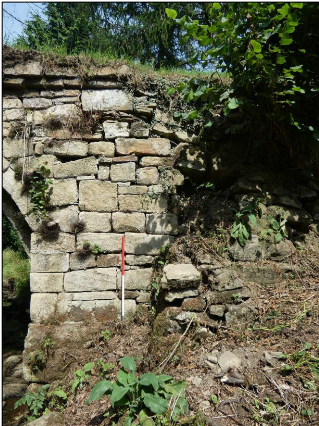
Plate 15: South elevation, east buttress/return, prior to repair, looking N (photo 1/903).
