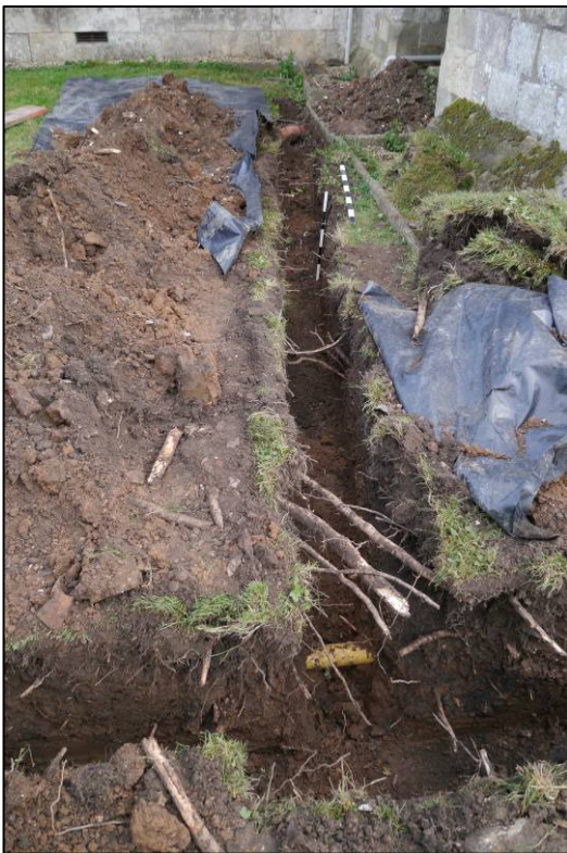
Plate 14: Trench 3 under excavation, looking E.
