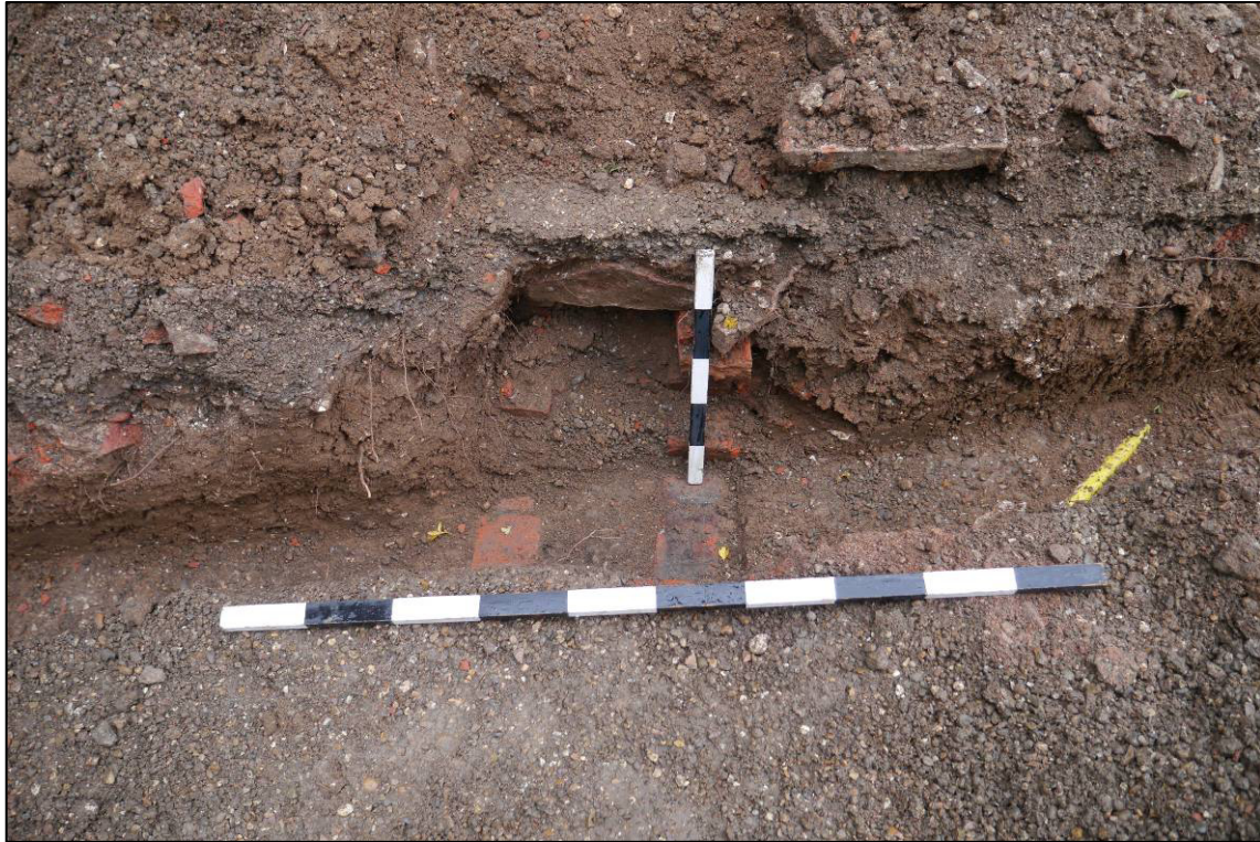
Plate 5: Brick culvert (113) in central section of Trench 1, looking NE.
