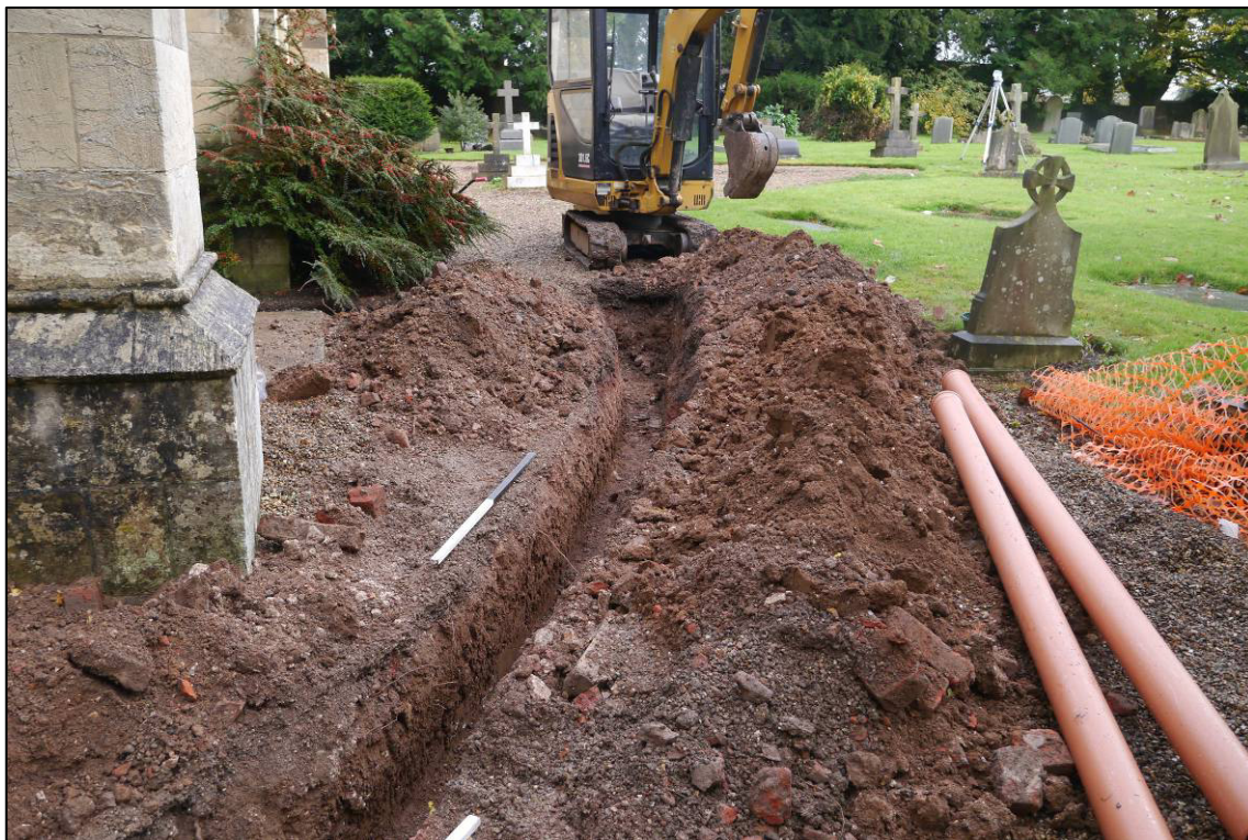
Plate 3: Trench 1 around south-west corner of tower under excavation, looking SE.
