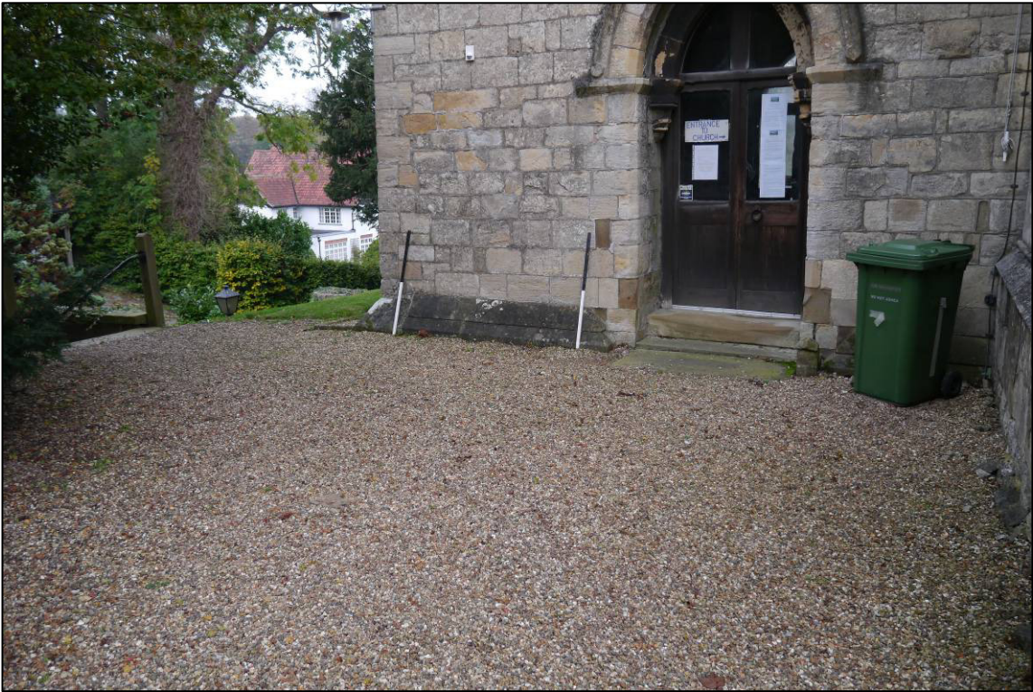
Plate 1: Area to south of the tower, prior to works commencing, looking NW.
