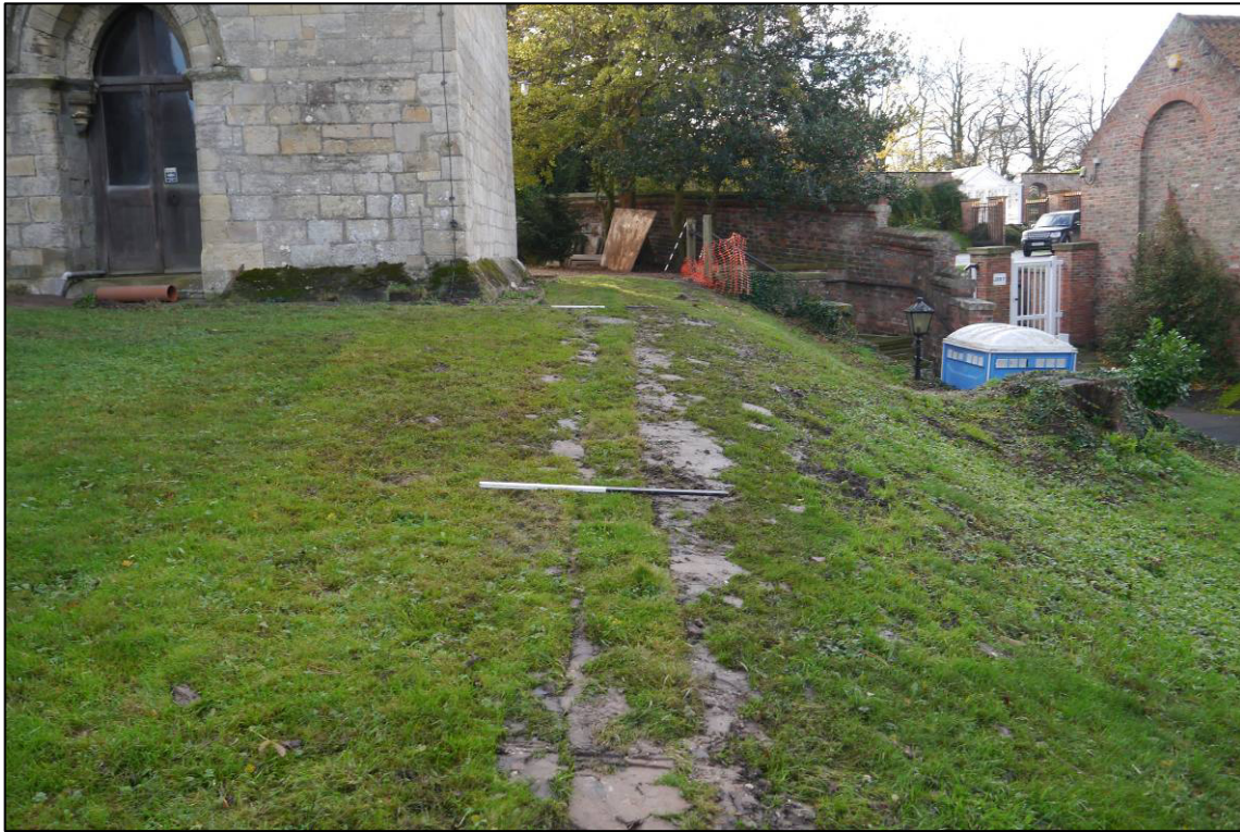
Plate 13: South end of Trench 2 after re-instatement, looking S.
