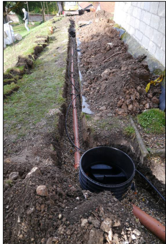
Plate 12: South end of Trench 2, prior to backfilling, looking N.
