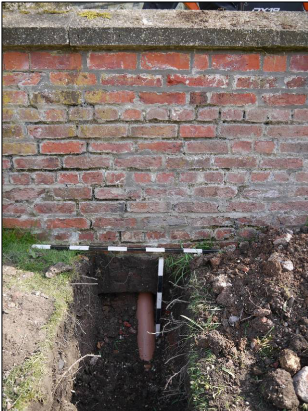
Plate 11: Drainage pipe emerging through north churchyard wall (115), looking S.
