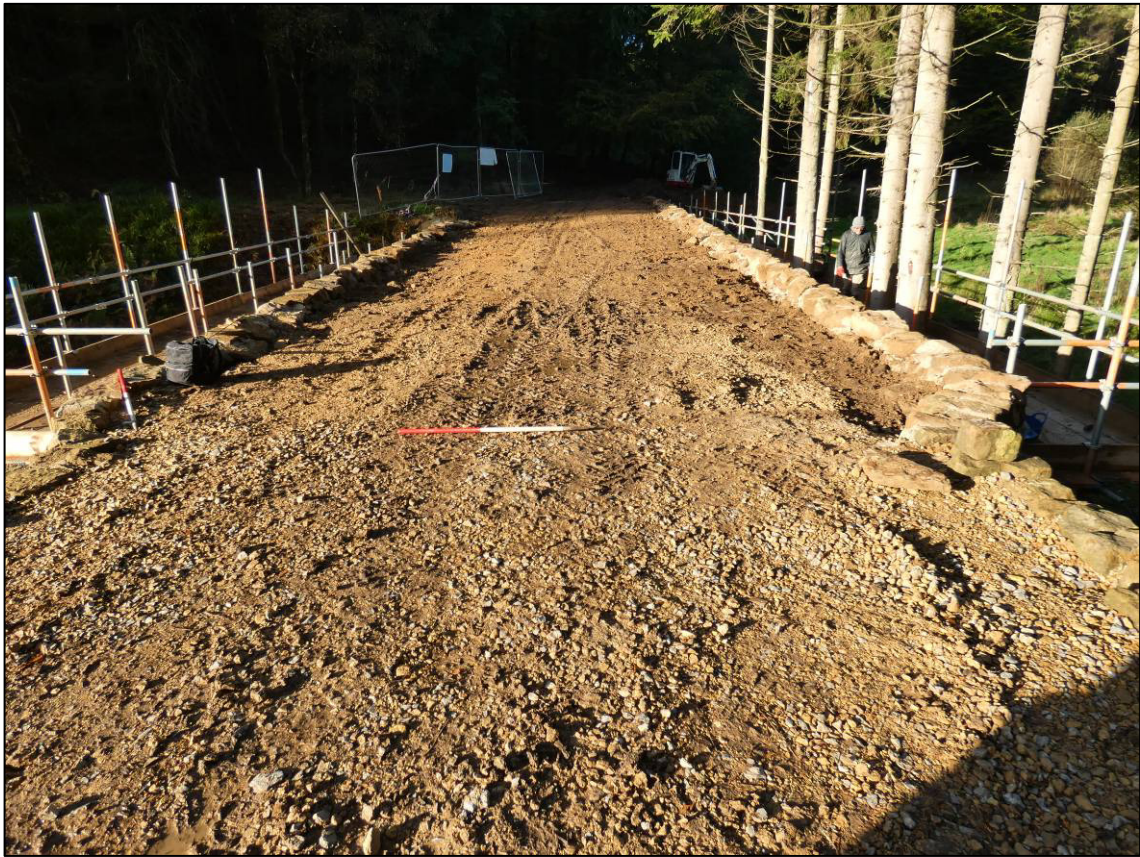
Plate 11: Abutments and bridge top surface after repair, looking SW (photo 5/772).
