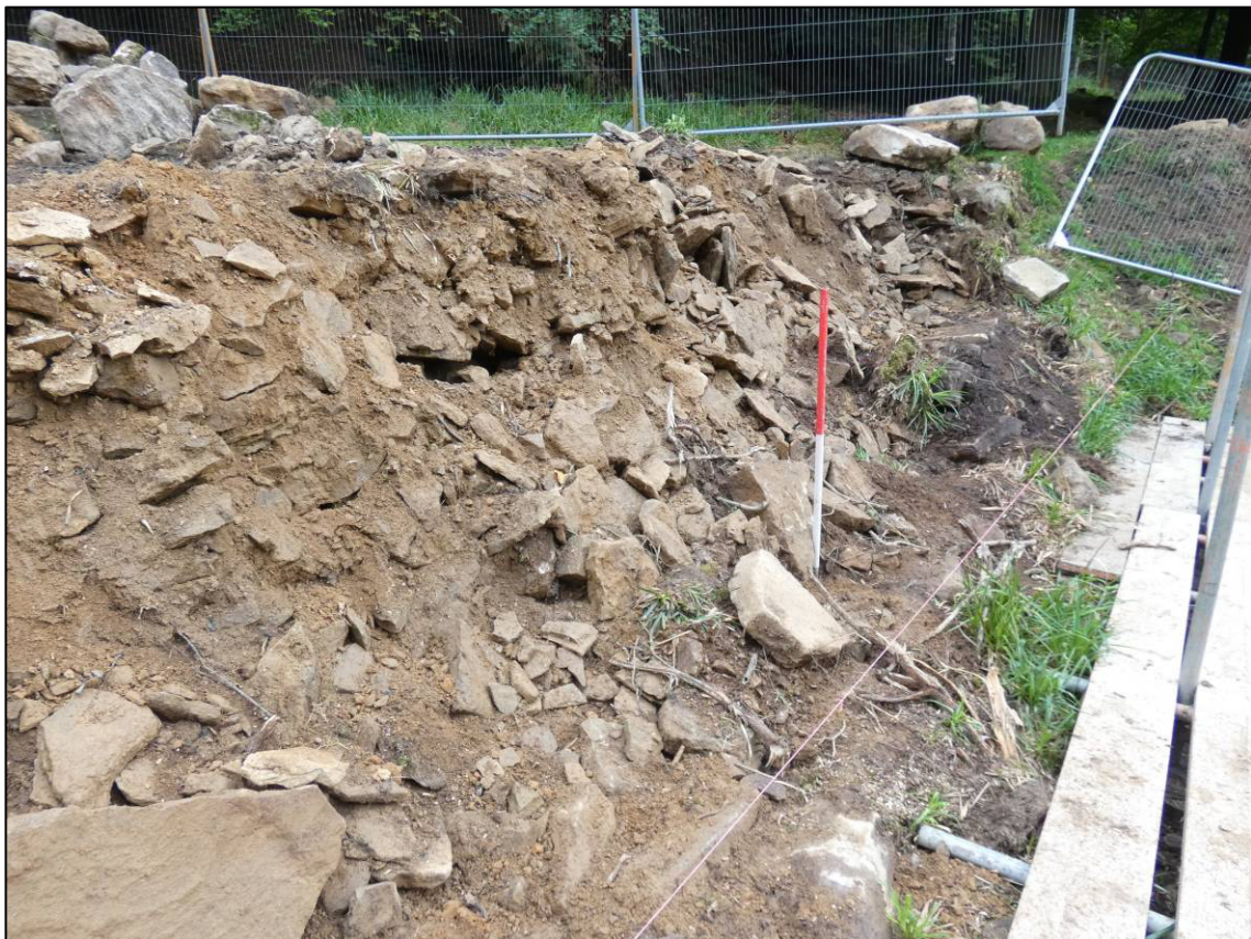
Plate 10: West abutment, north elevation, west section, during repair, looking SW (photo 4/639).
