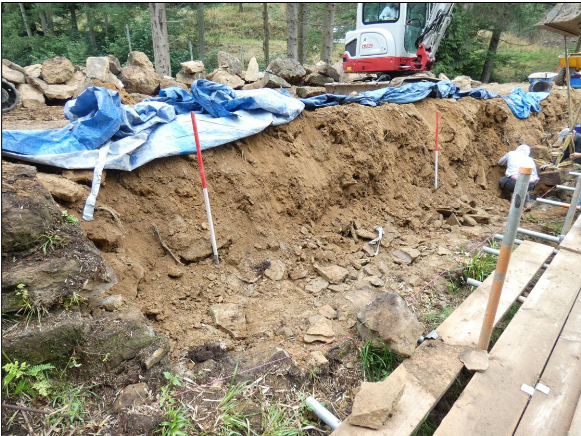
Plate 8: West abutment, south elevation, during repair, looking NE (photo 3/461).
