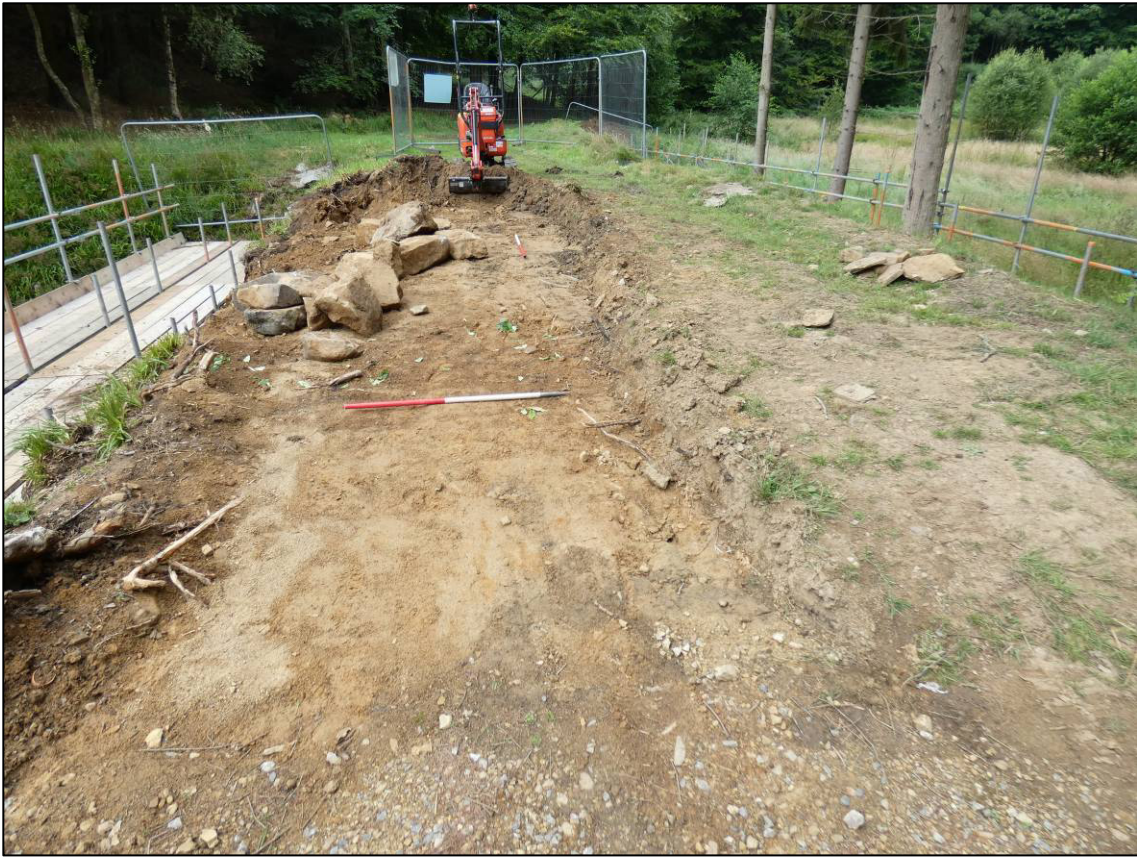
Plate 7: West abutment surface, reduction in ground level, looking SW (photo 2/331).
