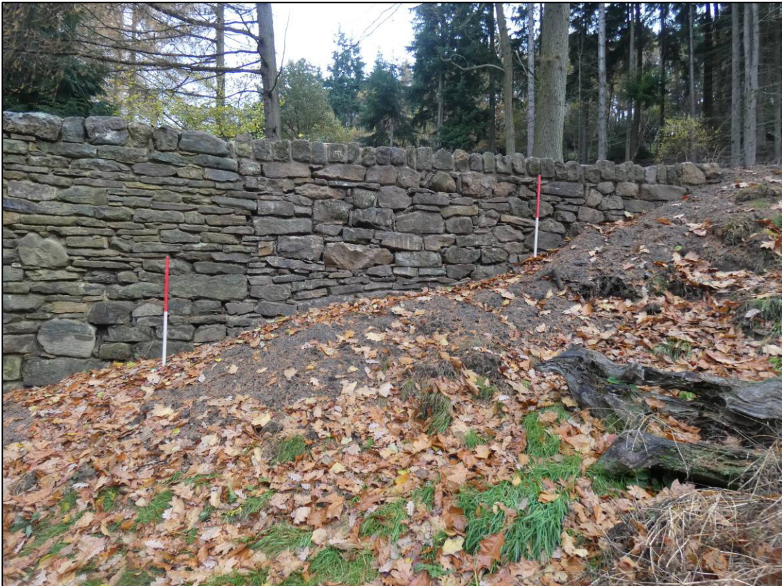
Plate 14: East abutment, south elevation after repair, looking NW (photo 6/019).
