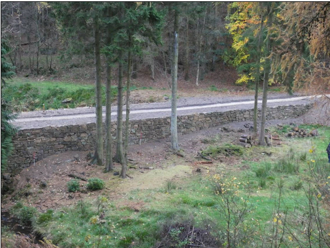
Plate 16: West abutment, north elevation after repair, looking S (photo 6/028).
