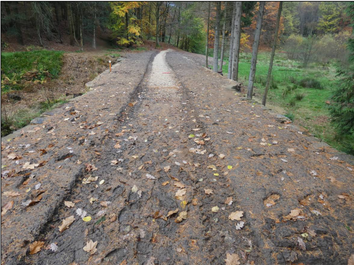
Plate 18: Bridge and abutment surfaces after resurfacing, looking SW (photo 6/044).
