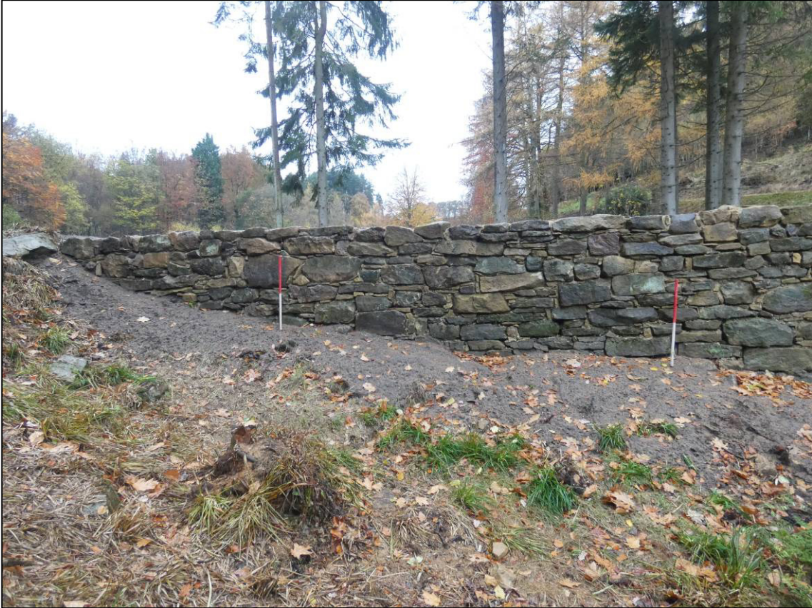
Plate 13: West abutment, south elevation, west section, after repair, looking NW (photo 6/025).
