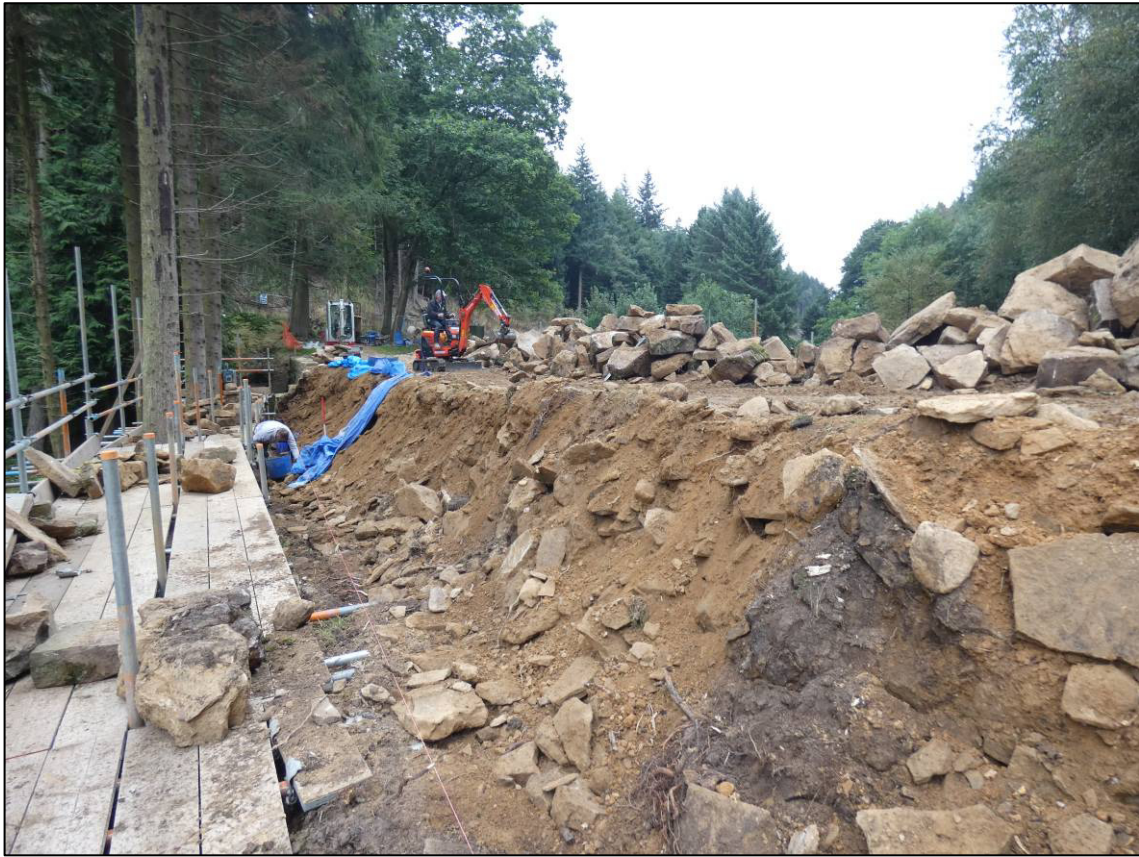
Plate 9: West abutment, north elevation, during repair, looking E (photo 4/634).
