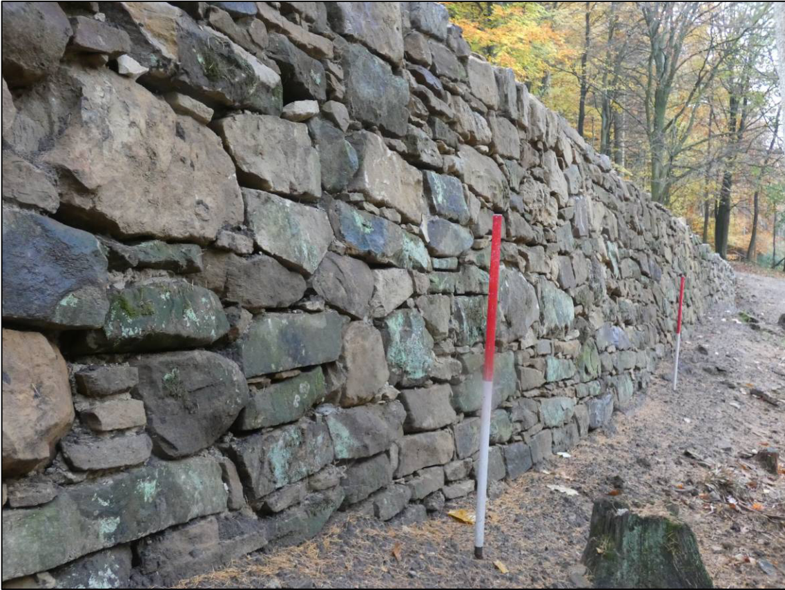
Plate 17: West abutment, north elevation after repair, looking SW (photo 6/032).
