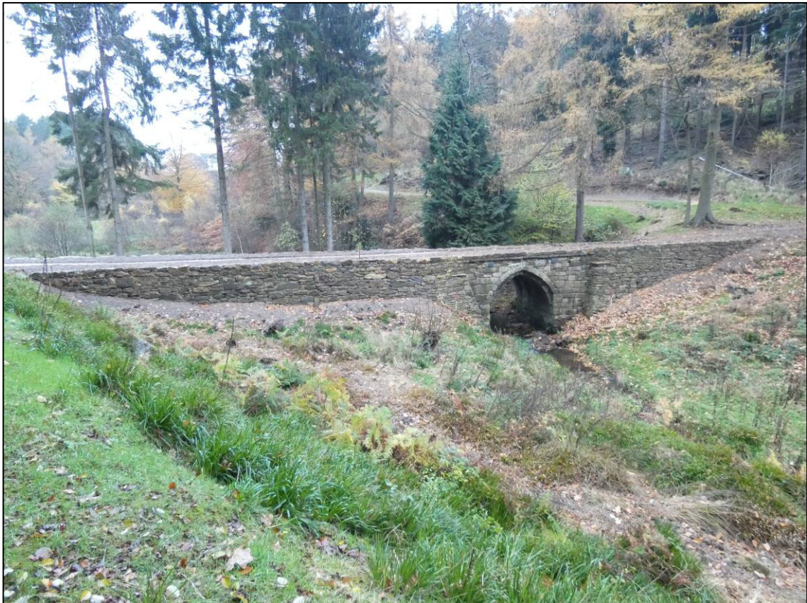
Plate 12: South elevation after repair, looking N (photo 6/007).
