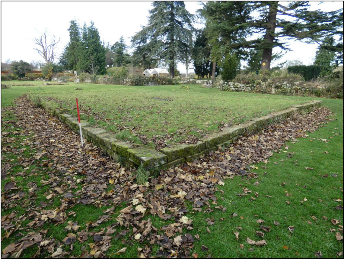
Plate 61: Area 19: Abbey church, central crossing platform, after repair, looking NW (photo 7/613).
