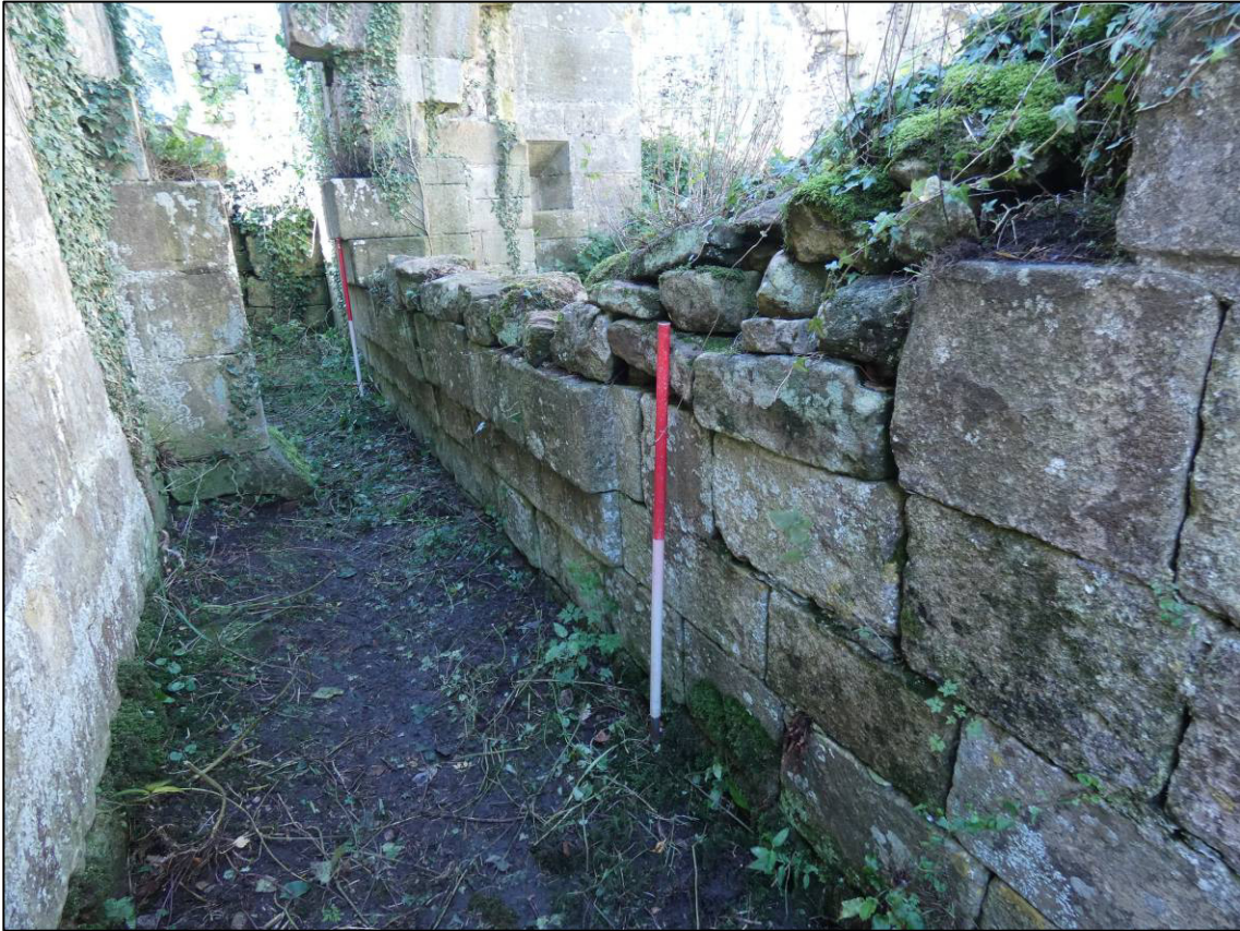
Plate 38: Area 13: Meat kitchen, south external elevation of south wall, showing corbelling for fireplace, looking W (photo 4/179).
