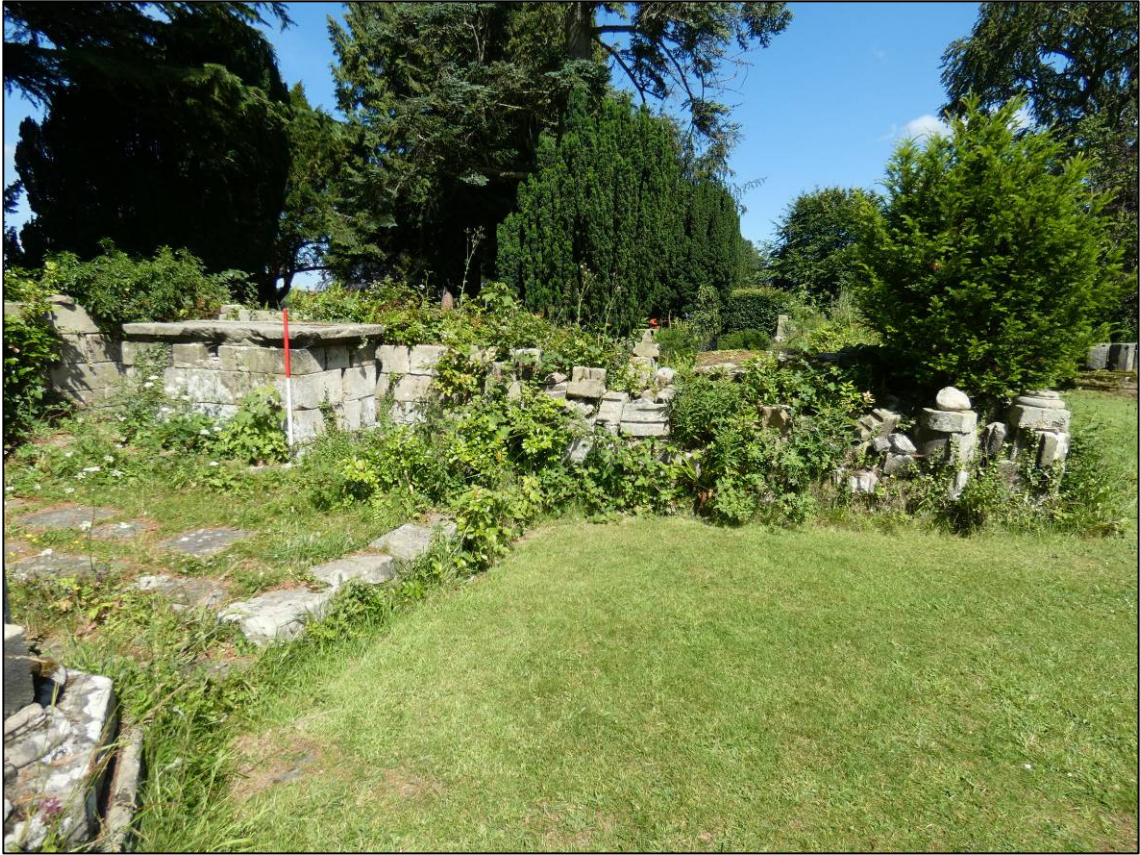
Plate 59: Area 19: Abbey church, north transept, west internal elevation of east wall, looking E (photo 1/394).
