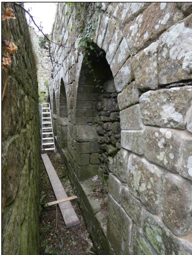
Plate 44: Area 14: Monks' rere-dorter, south internal elevation of drain, looking E (photo 3/567).
