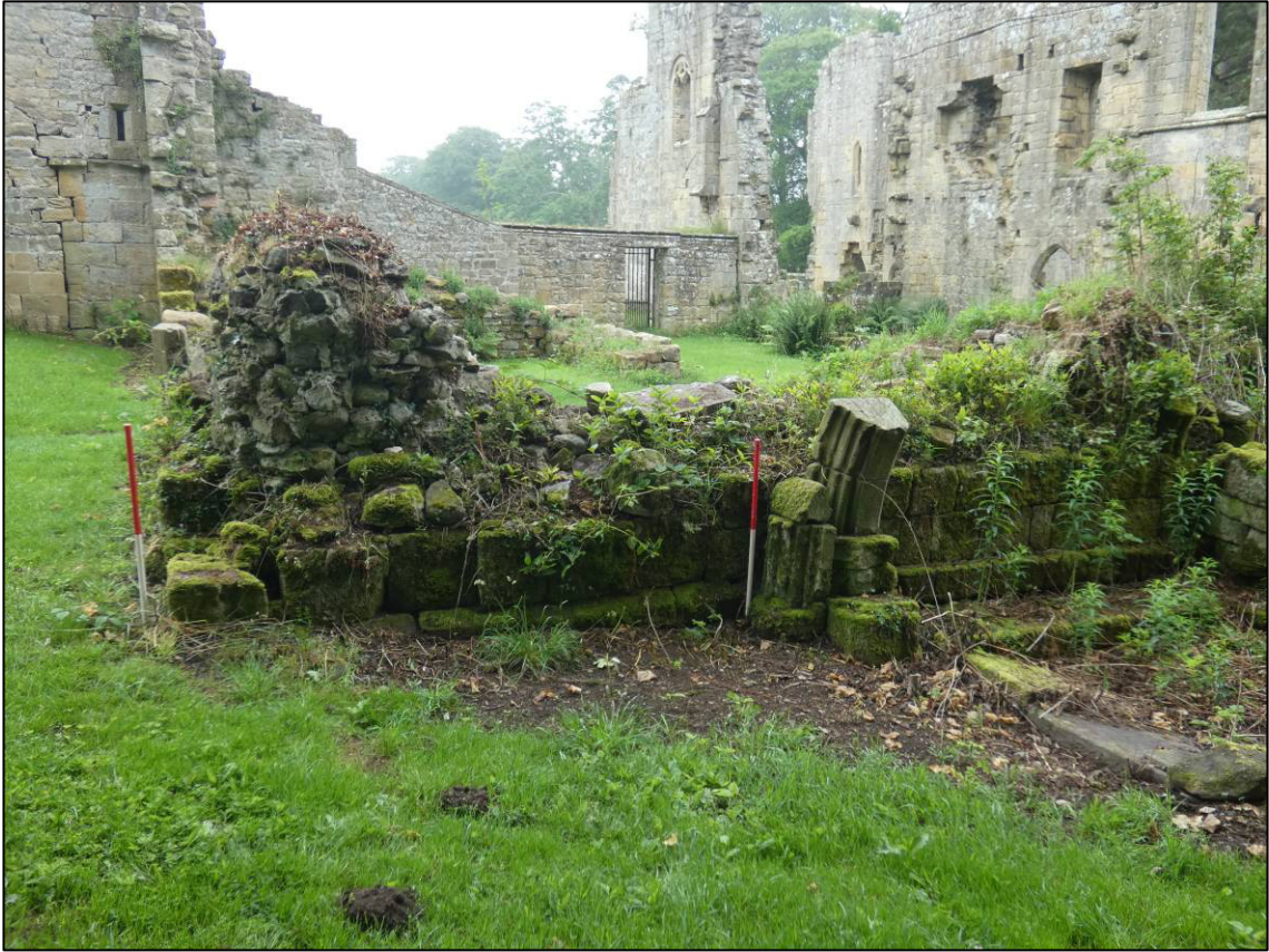
Plate 47: Area 15: Infirmary's lodging, west external elevation of west wall, before clearance, looking E (photo 6/642).
