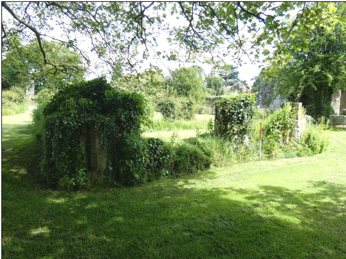
Plate 3: Area 2: Lay brothers' rear-dorter, south external elevation of south wall, before clearance, looking NE (photo 1/257).
