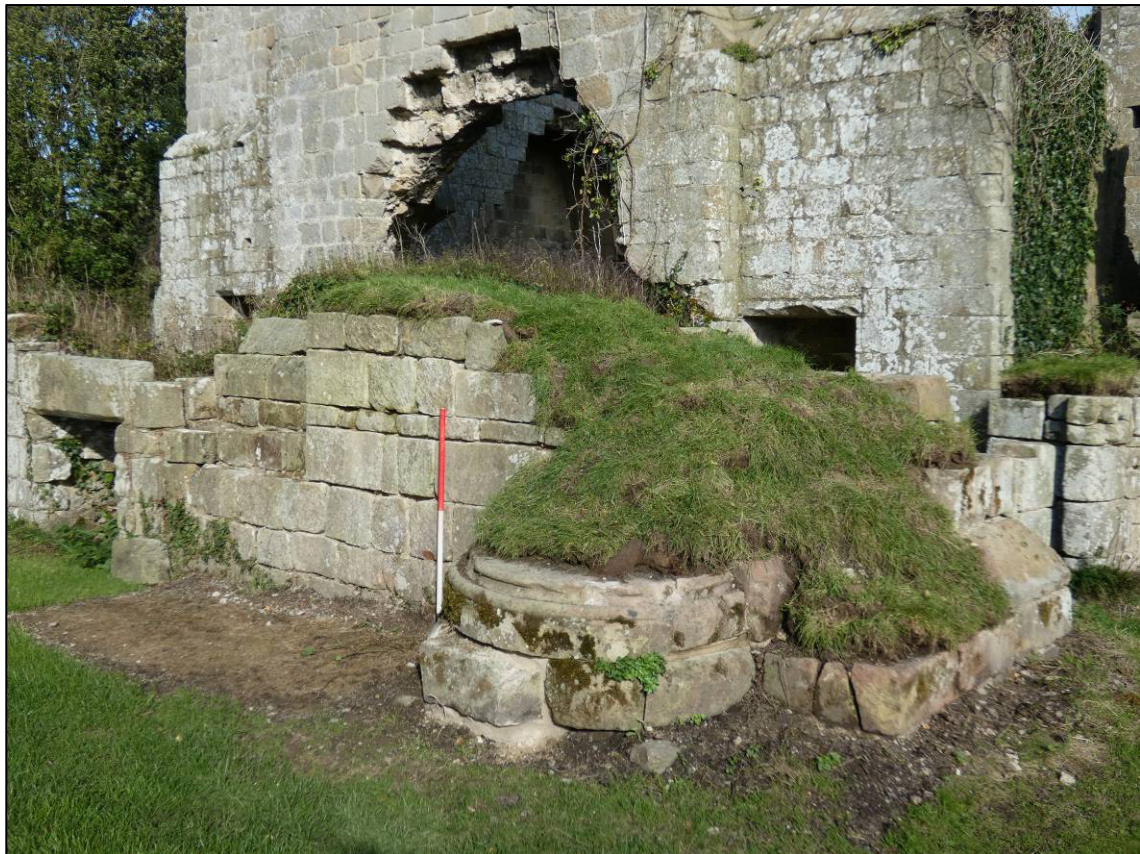
Plate 27: Area 9: Monks' dorter, pier base and west internal elevation of east wall (south end), after repair, looking NE (photo 4/185).
