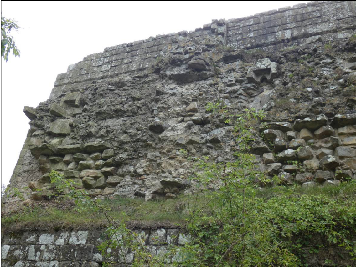
Plate 42: Area 14: Monks' rere-dorter, north internal elevation of south wall (upper level), after clearance, showing possible lancet windows either side of chimney and cut line of former rere-dorter roof, looking S (photo 3/563).
