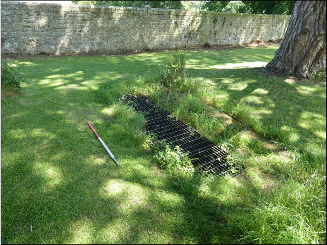
Plate 67: Area 15: Monks' infirmary, grills over open culvert of east-west drain, looking SE (photo 1/364).
