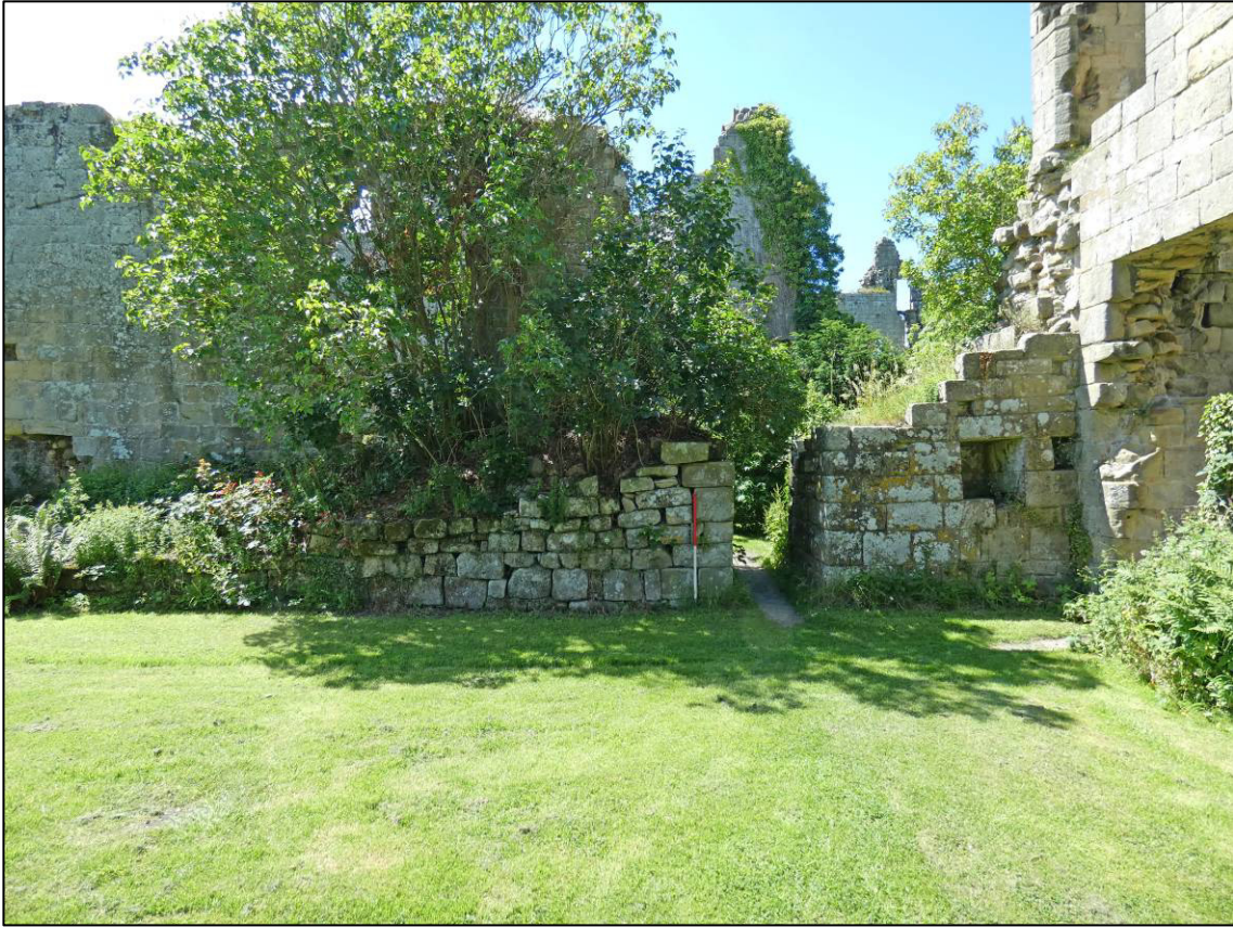
Plate 32: Area 11: Abbots' lodging, east internal elevation of west wall (north end), showing doorway into garderobe, looking W (photo 1/342).
