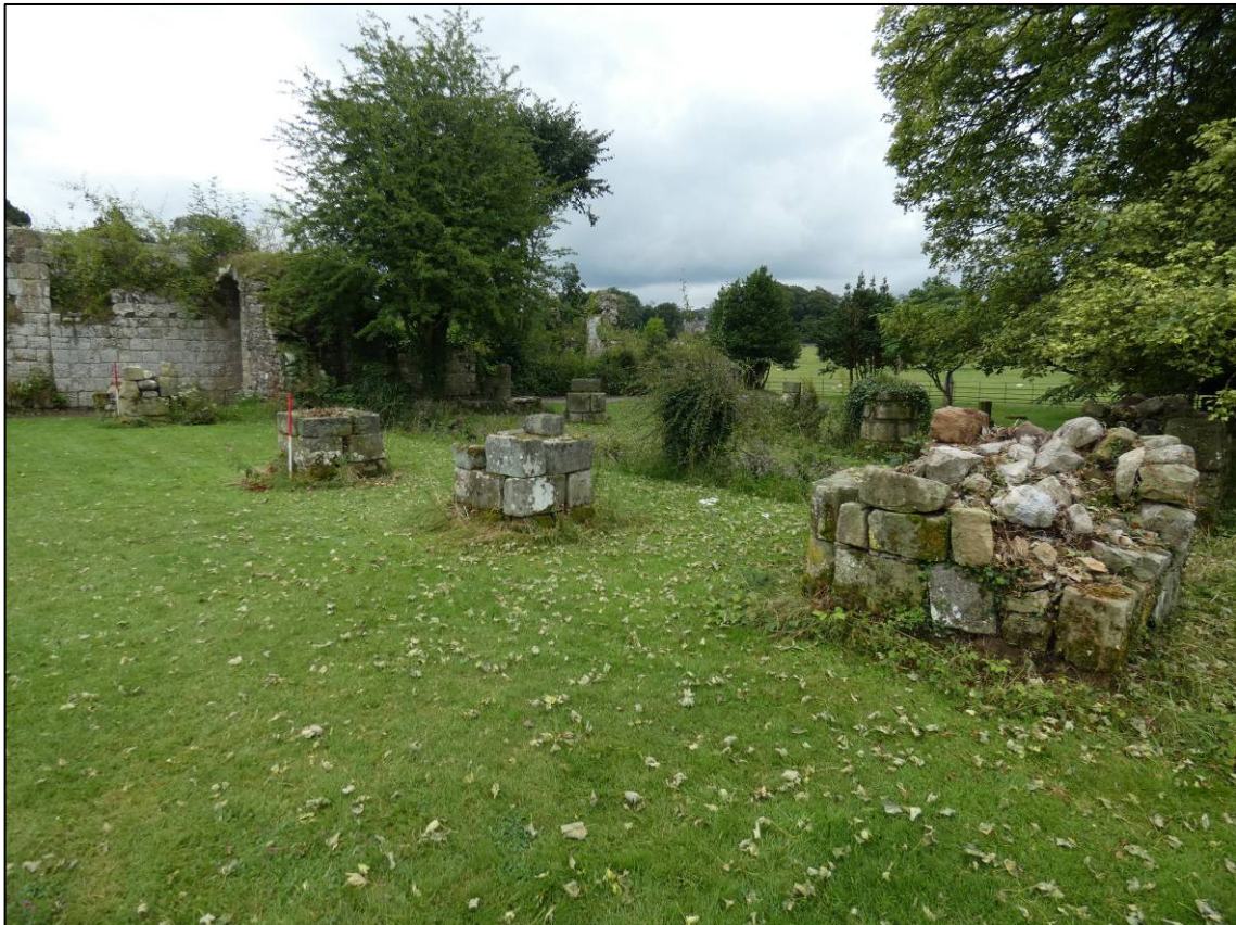
Plate 5: Area 2: Lay brothers' rear-dorter, north external elevation, piers and east return of west wall, looking SE (photo 2/465).
