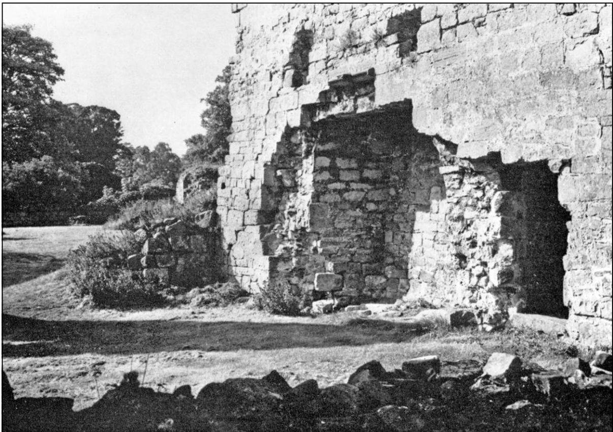
Area 6: Monks' frater, showing surviving section of east elevation of east wall, against north wall of the misericord (Area 8), looking NW.
