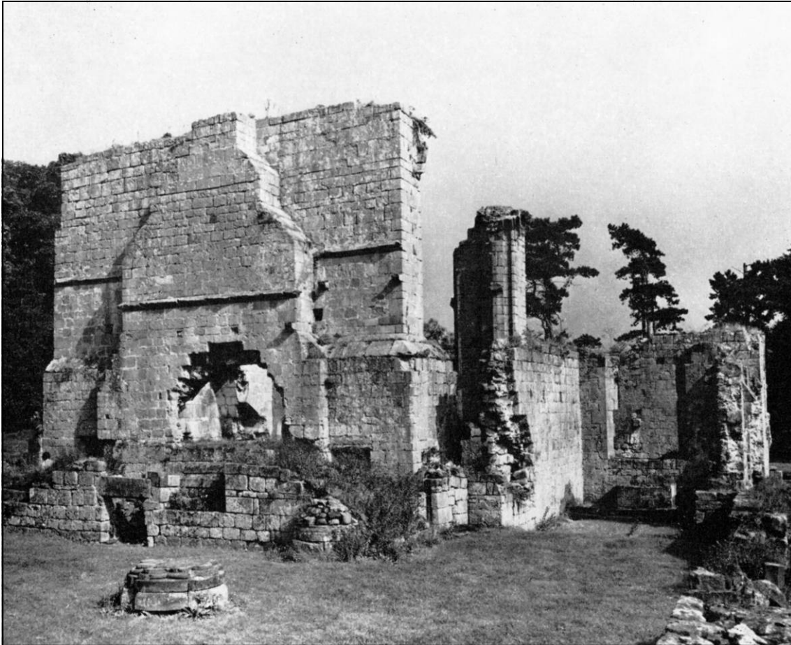
Area 9: Monks' dorter, showing fireplace, window and pier base in west internal elevation of east wall (south part), with west wall of meat kitchen (Area 13) behind and chapel (Area 10) to right, looking NE.
