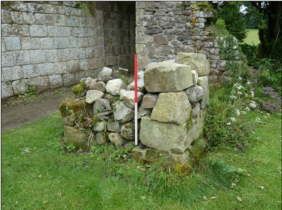
Plate 7: Area 2: Lay brothers' rear-dorter, east end of north wall, after clearance, looking E (photo 2/463).
