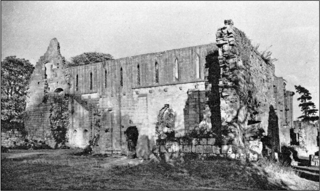
Area 6: Monks' frater, showing surviving section of west elevation of east wall, against north wall of the misericord (Area 8), looking NE.
