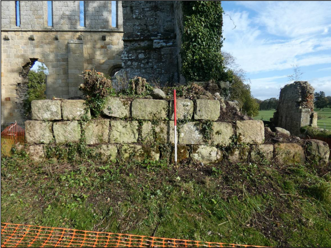
Plate 14: Area 6: Monks' frater, west internal elevation of east wall (south end), after clearance, looking E (photo 4/191).
