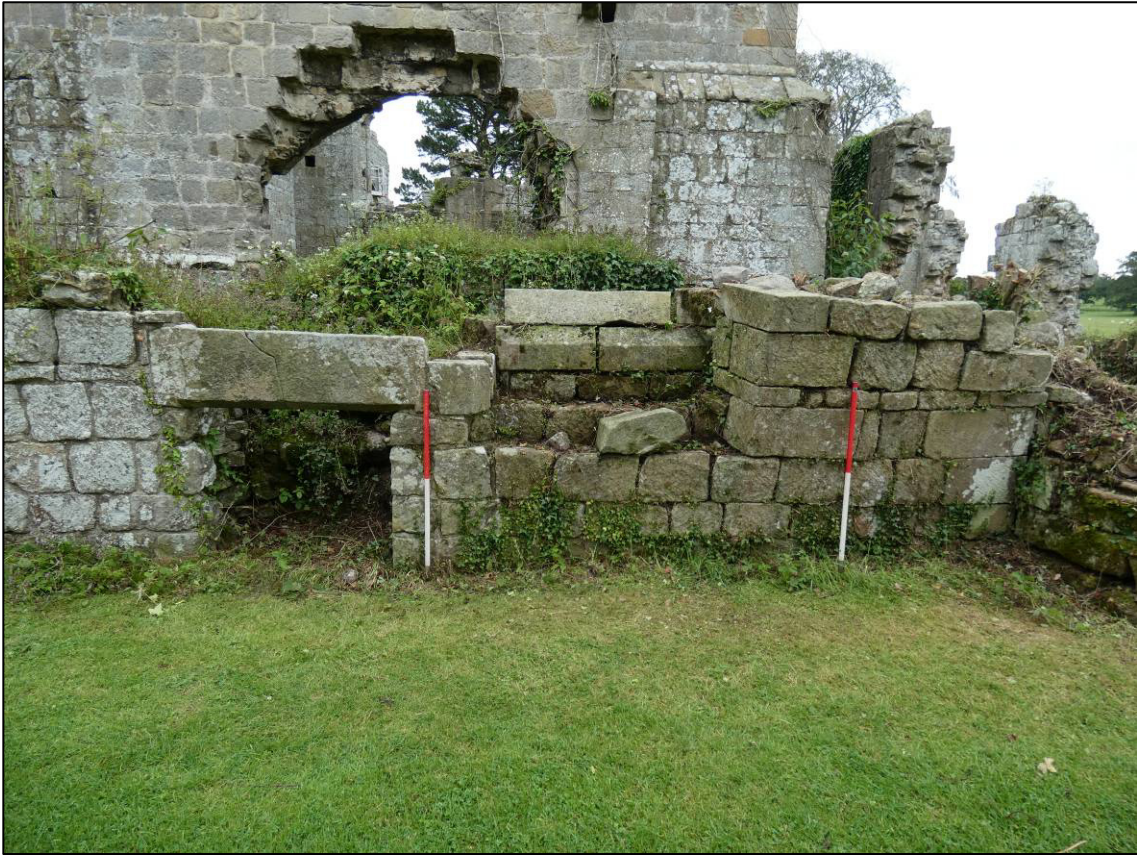
Plate 22: Area 9: Monks' dorter, fireplace and window in west internal elevation of east wall (south part), after clearance, looking E (photo 2/477).
