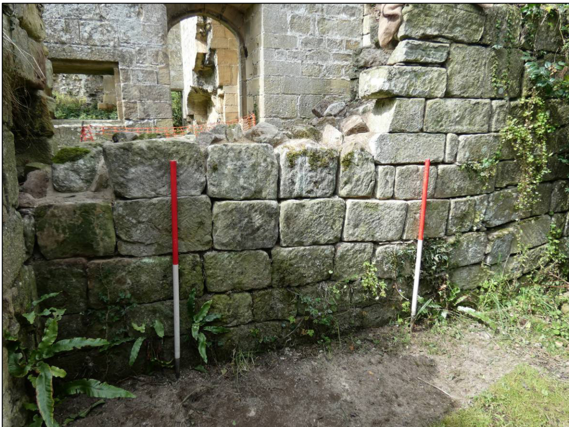
Plate 35: Area 12: Staircase between abbots' lodging and monks' rere-dorter, east elevation of wall to the east, after repair, looking W (photo 3/562).
