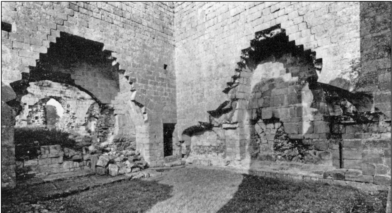
Area 13: Meat kitchen, showing fireplaces in north and west internal walls, looking NW.
