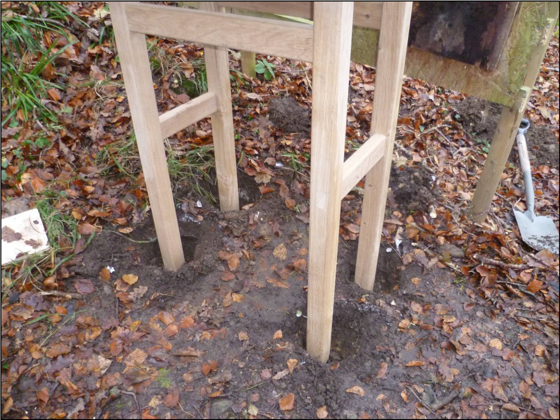
Plate 5: Excavated holes for leg supports, Foss Castle interpretation board, looking NE.
