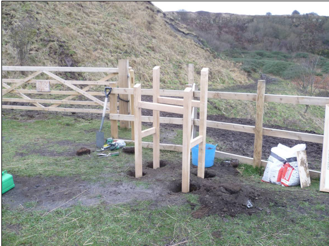
Plate 1: Installation of Deep Grove quarry interpretation board, looking SW.
