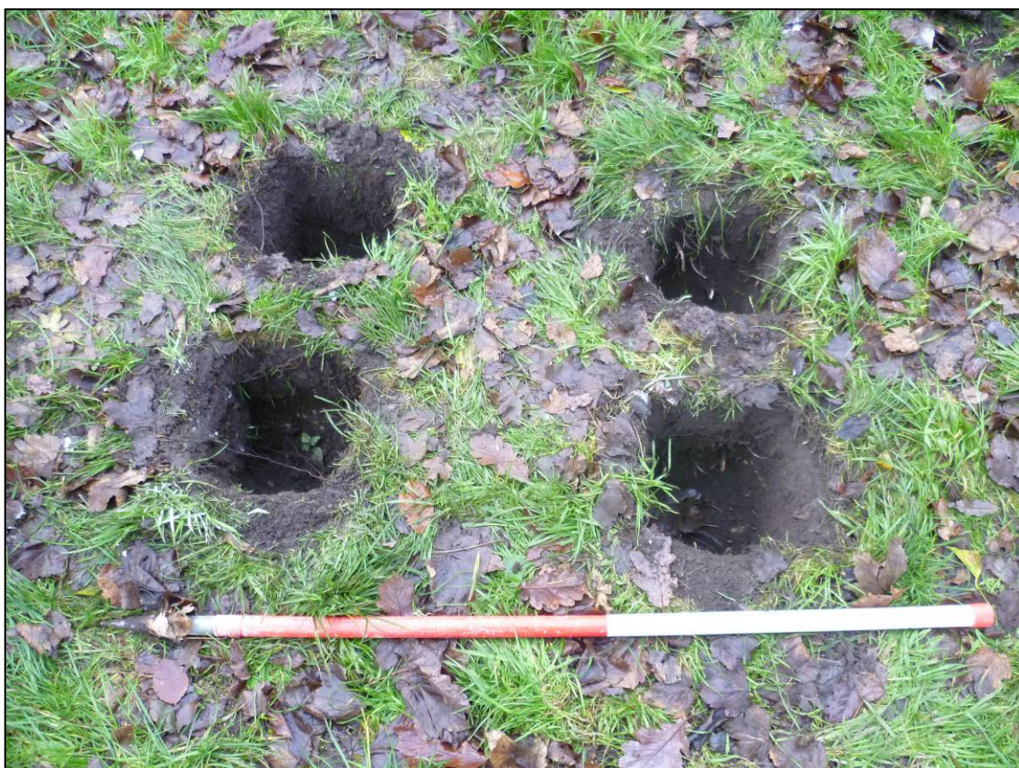
Plate 7: Excavated holes for leg supports, Old Mulgrave Castle interpretation board, looking E.
