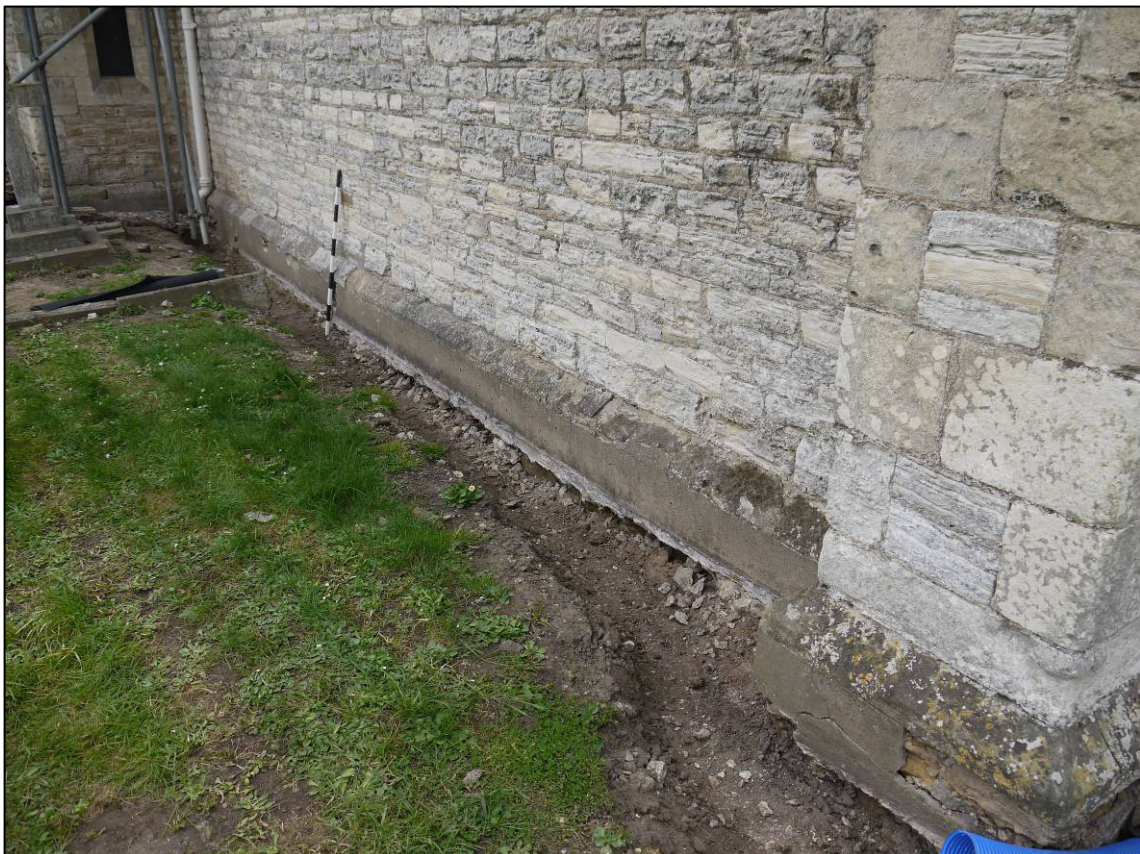
Plate 15: Excavated drainage channel (Trench 3) along south side of chancel, looking NW.
