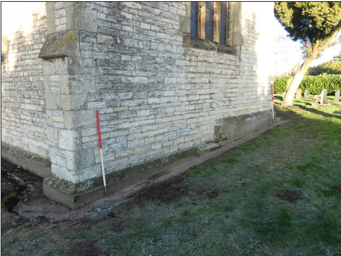
Plate 13: Existing drainage channel along east side of chancel, looking NW.
