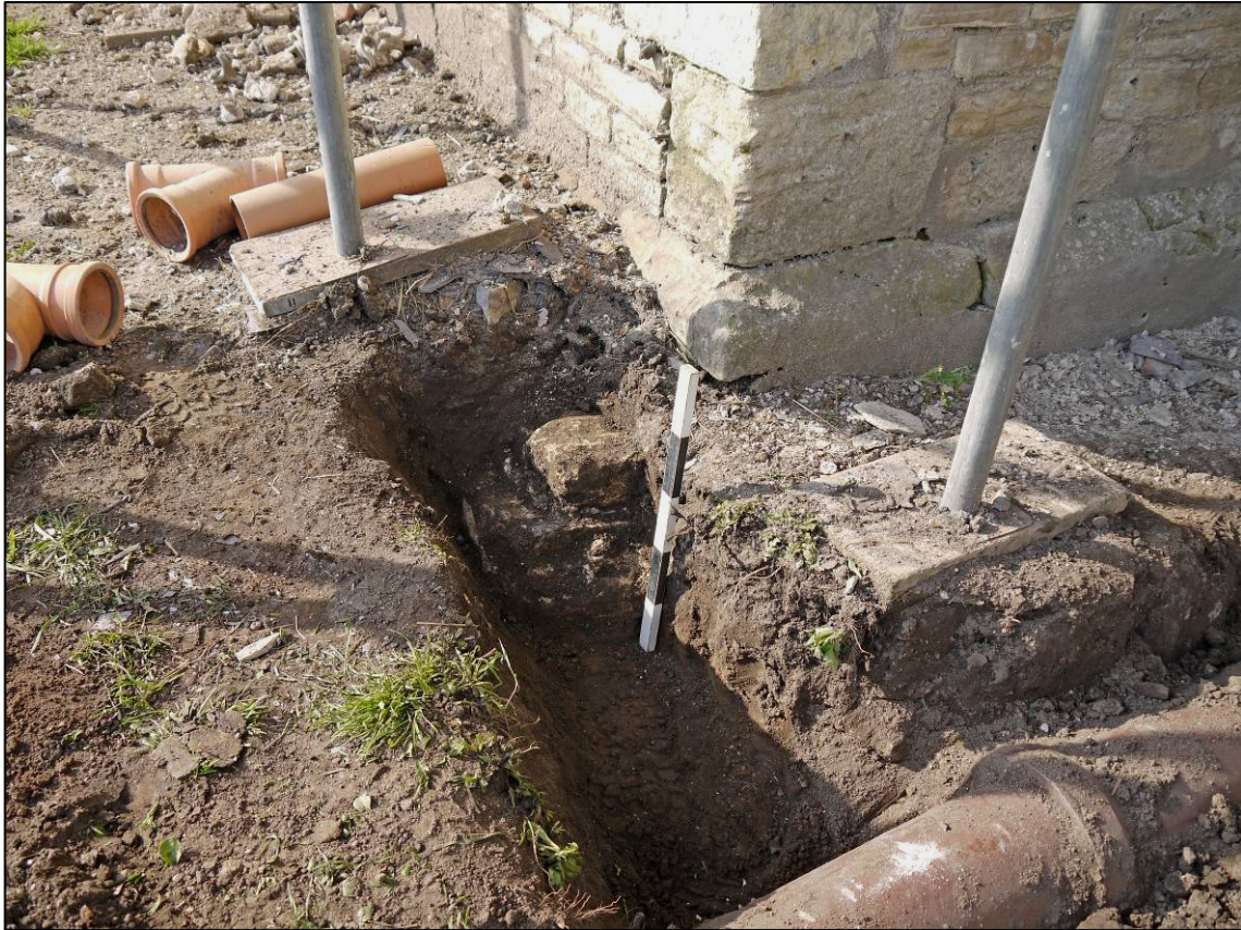
Plate 16: West end of Trench 3, showing projecting footings of south-east corner of nave (106), looking W.
