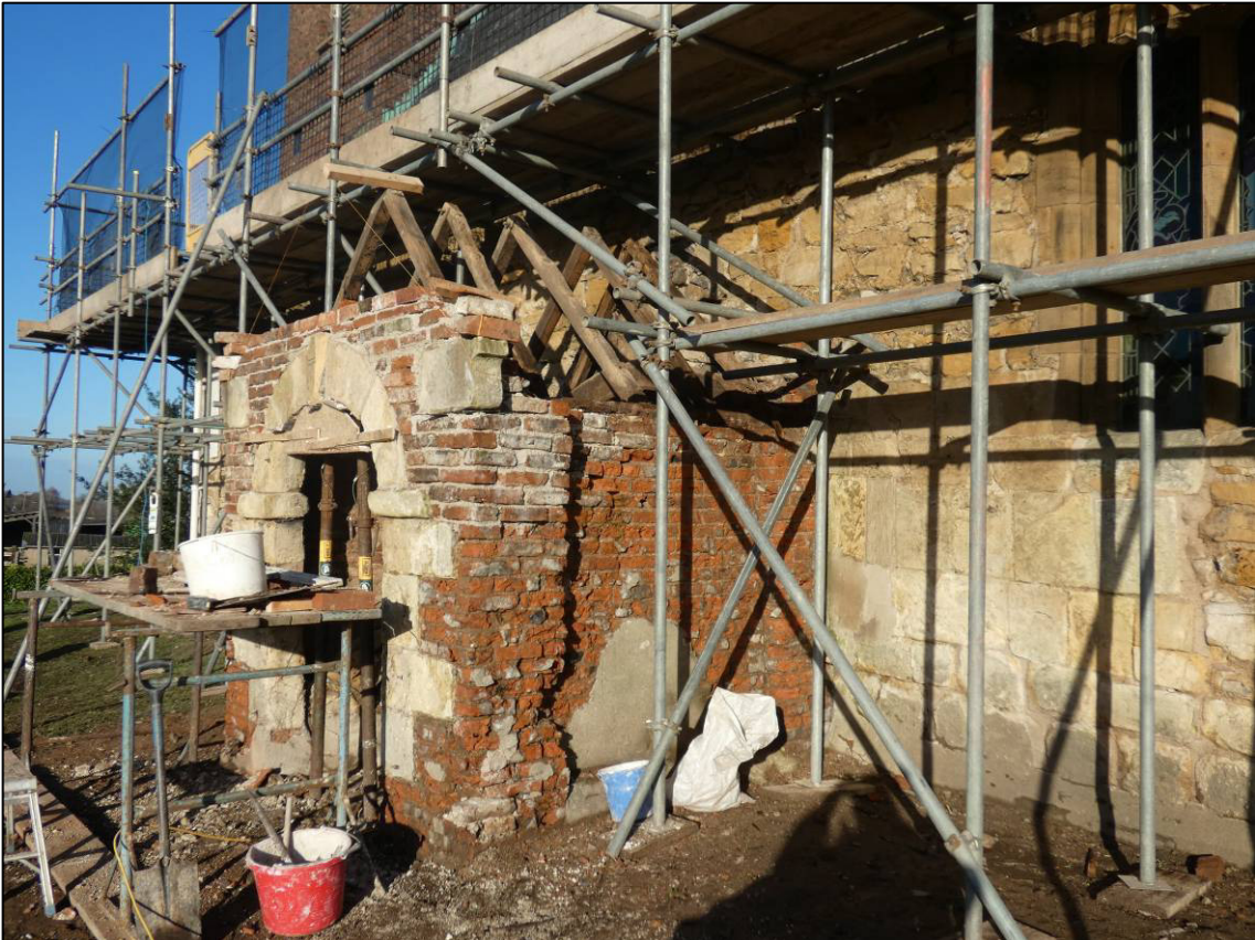
Plate 9: South porch, with stucco removed and undergoing repair, looking NW.
