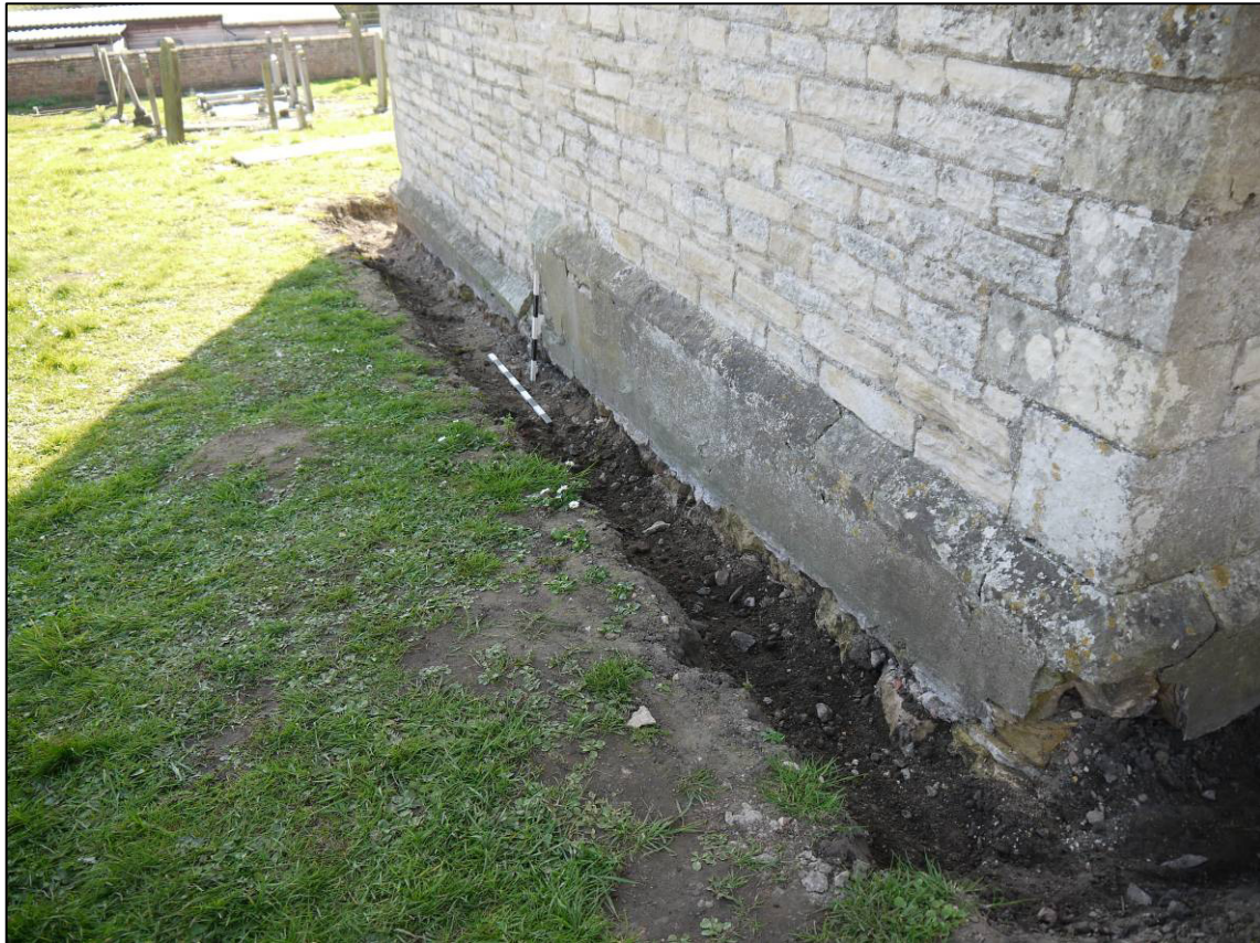
Plate 14: Excavated drainage channel (Trench 2) along east side of chancel, looking SW.
