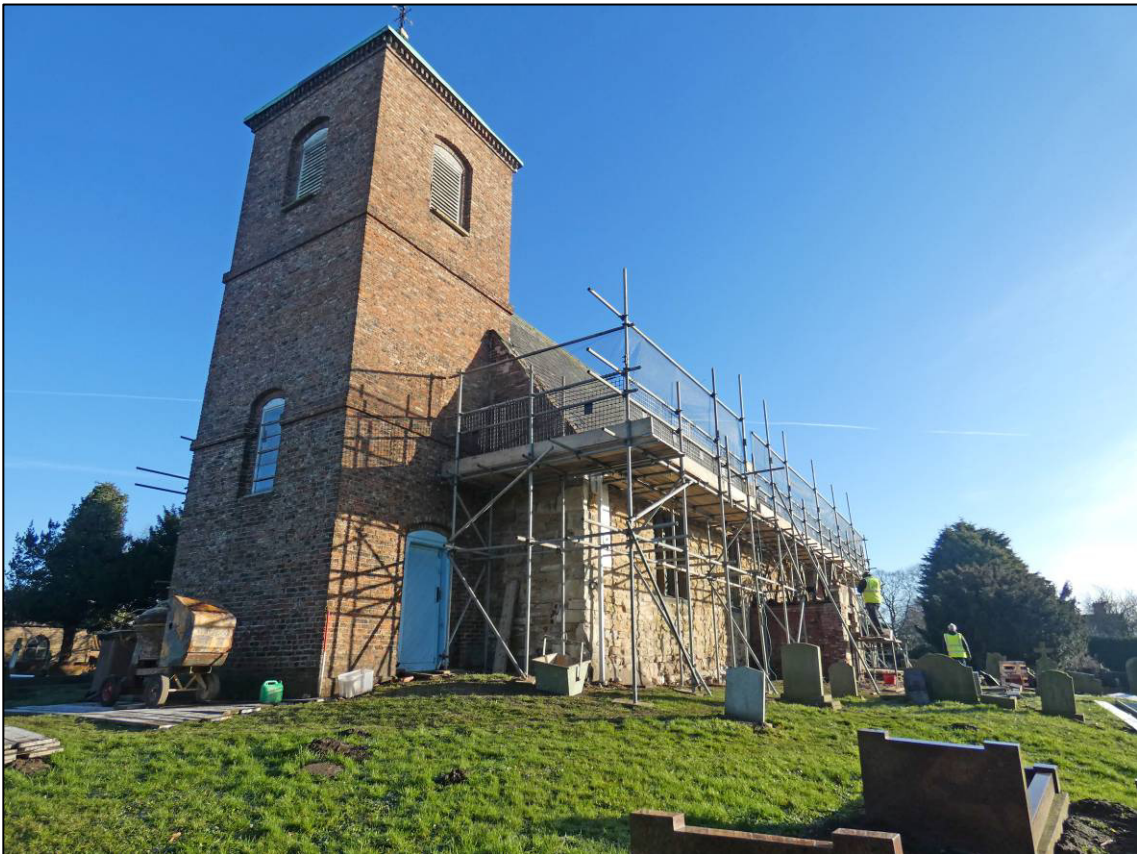
Plate 2: St Helen's Church, showing 18th century brick tower, looking NE.
