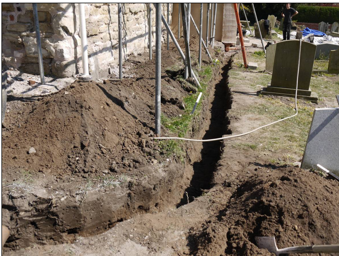
Plate 19: Excavated Trench 6, running west from south porch, looking E.
