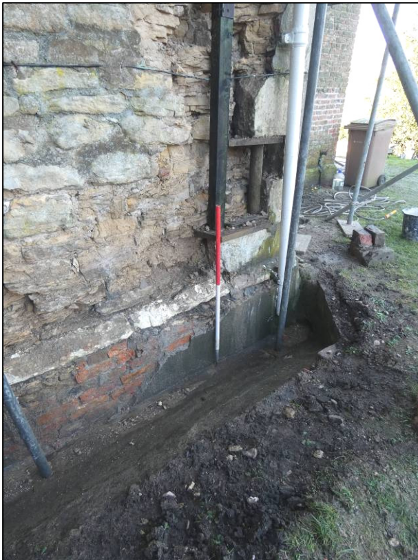
Plate 6: Brick plinth at west end of nave, looking SW.
