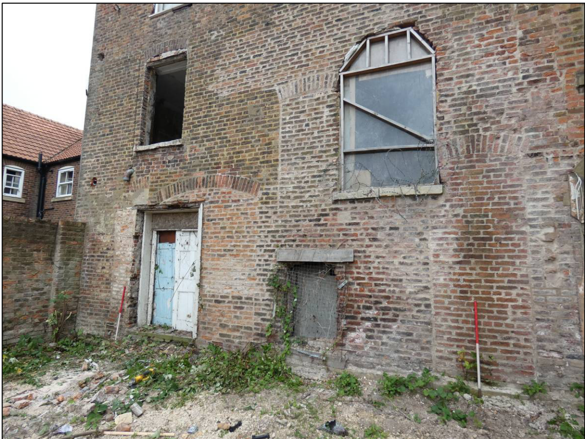
Plate 9: East elevation, south end, showing blocked openings, looking SW (photo 1/035).
