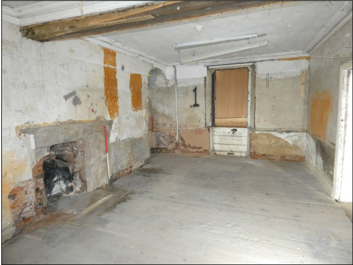
Plate 29: Ground floor south room (GF3), looking W (photo 2/163).
