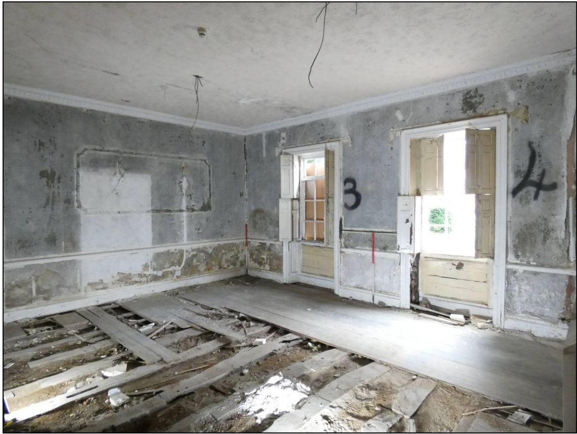
Plate 21: Ground floor north room (GF1), looking SW (photo 1/090).
