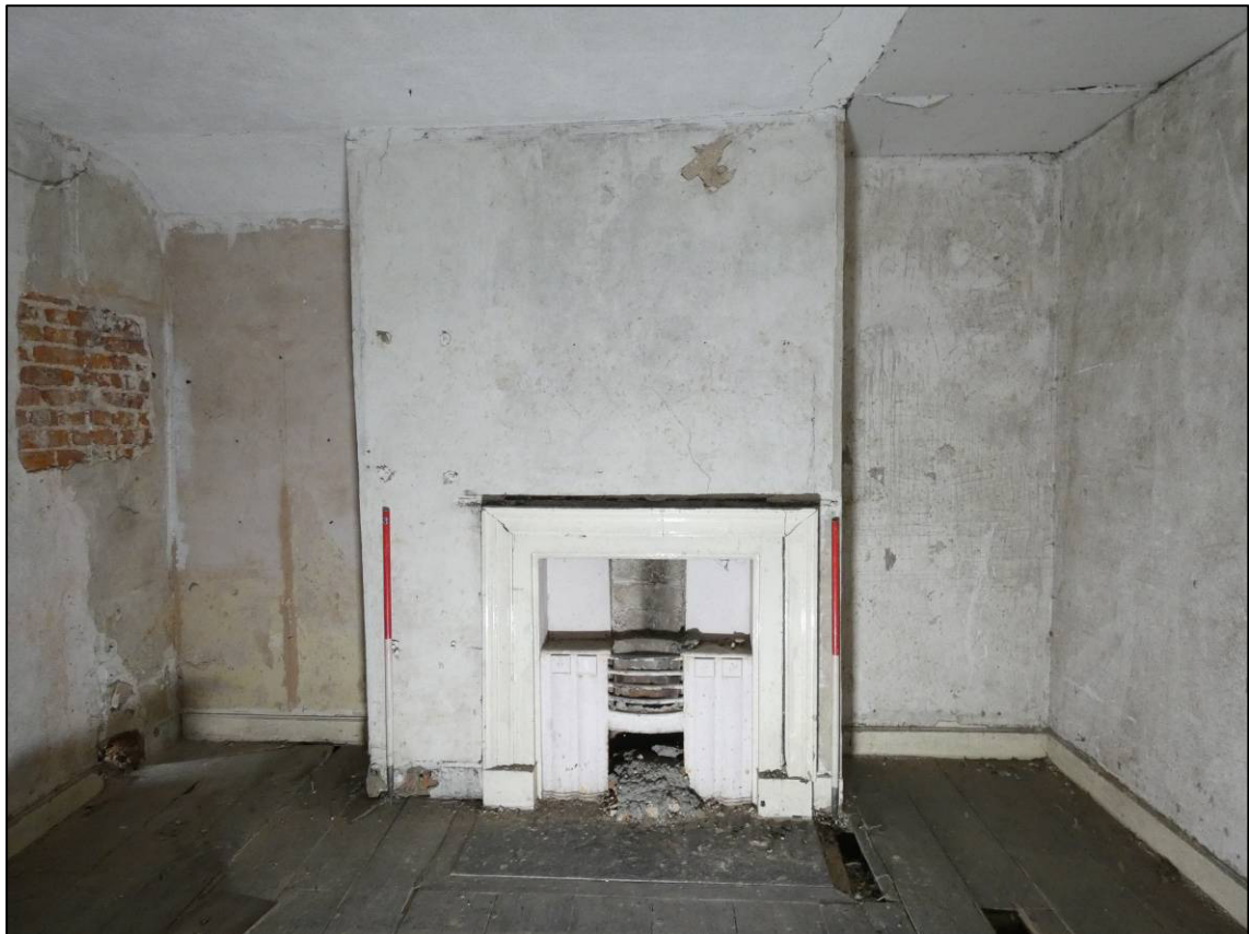
Plate 49: First floor south-west room (1F3), south wall, looking S (photo 2/275).
