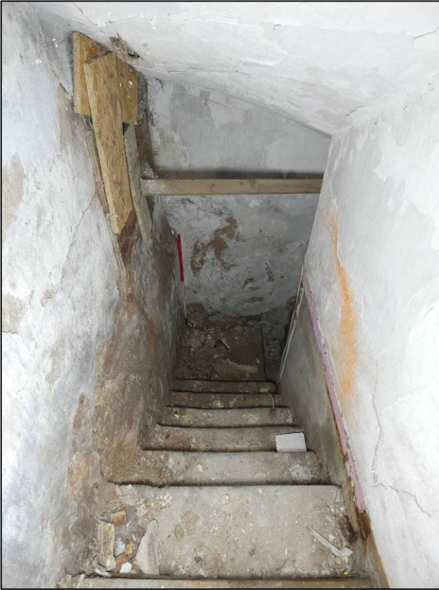
Plate 12: Stairs to cellar room C1, looking S (photo 2/103).
