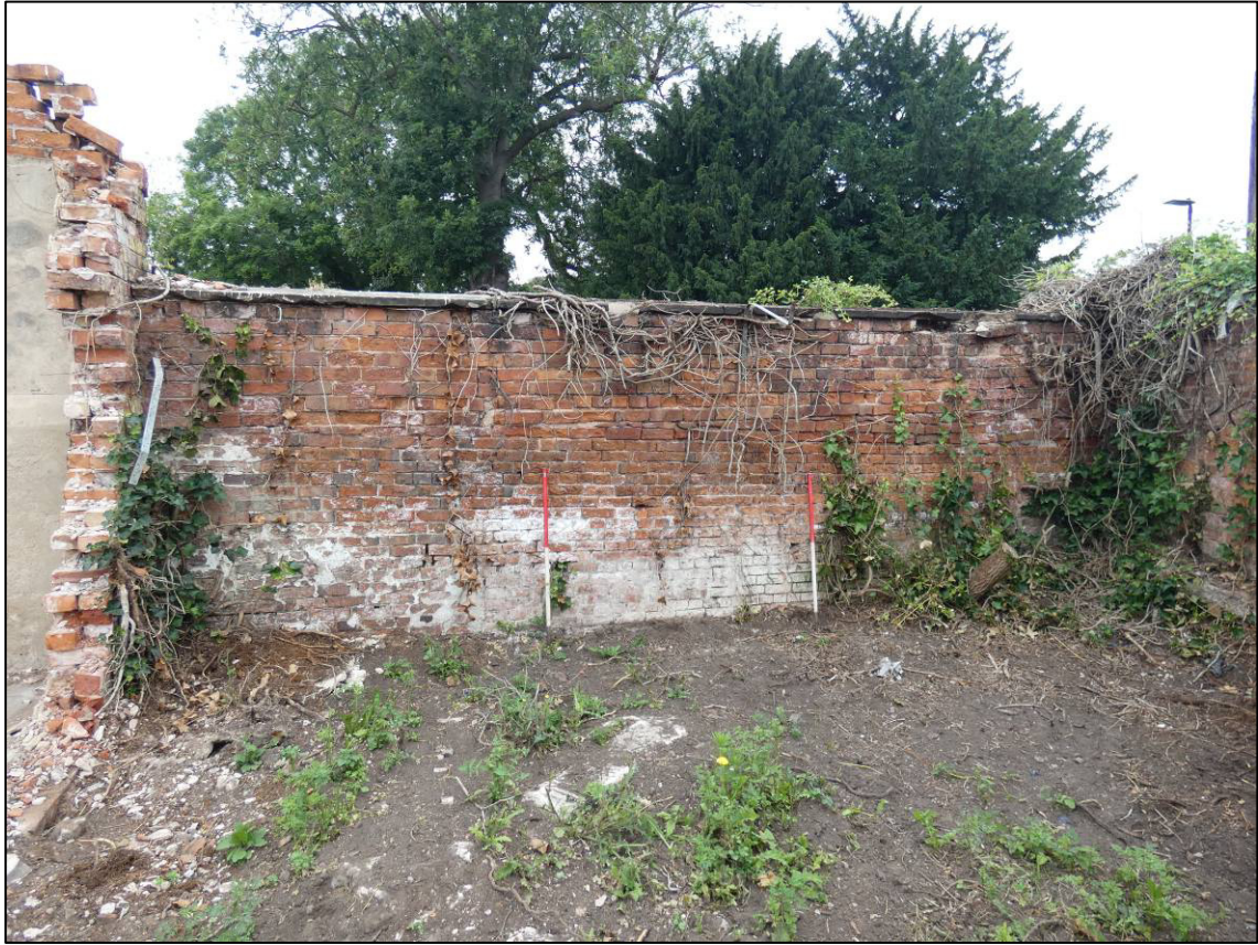
Plate 72: Rear yard, east end of north boundary wall, looking N (photo 1/958).
