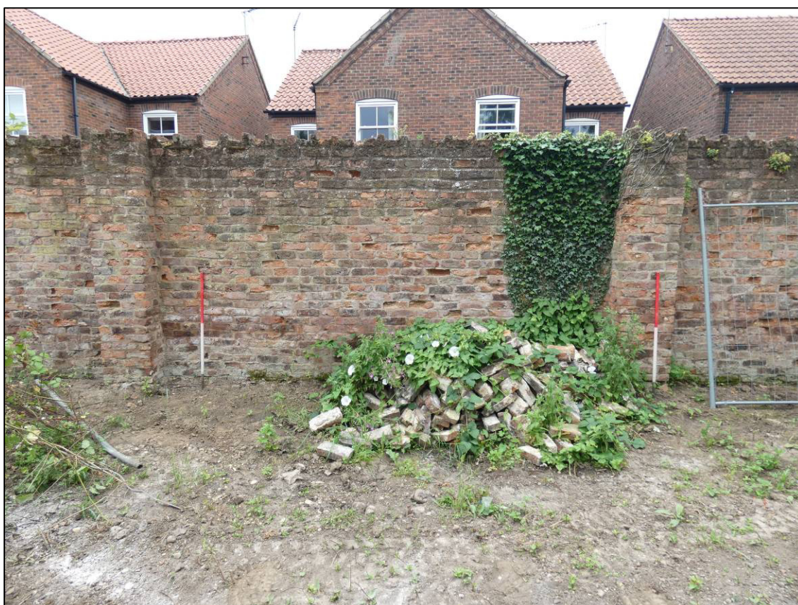
Plate 75: Rear yard, central part of south boundary wall, looking S (photo 1/971).
