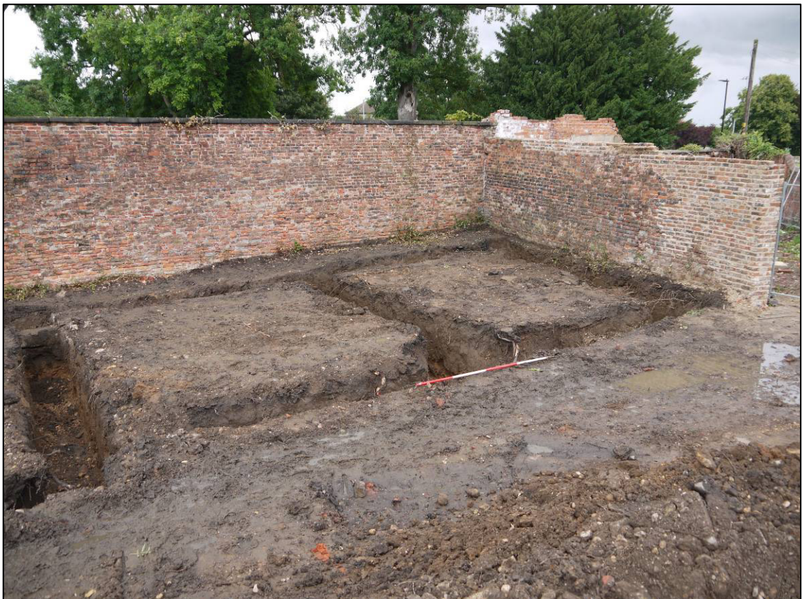
Plate 80: Excavated trenches for east end of new building, looking NE.
