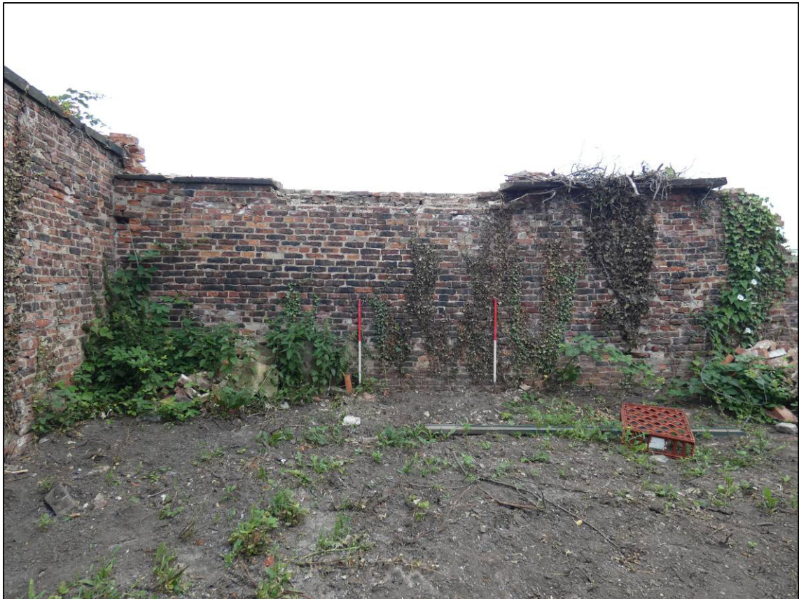
Plate 71: Rear yard, north end of east cross wall, looking E (photo 1/961).
