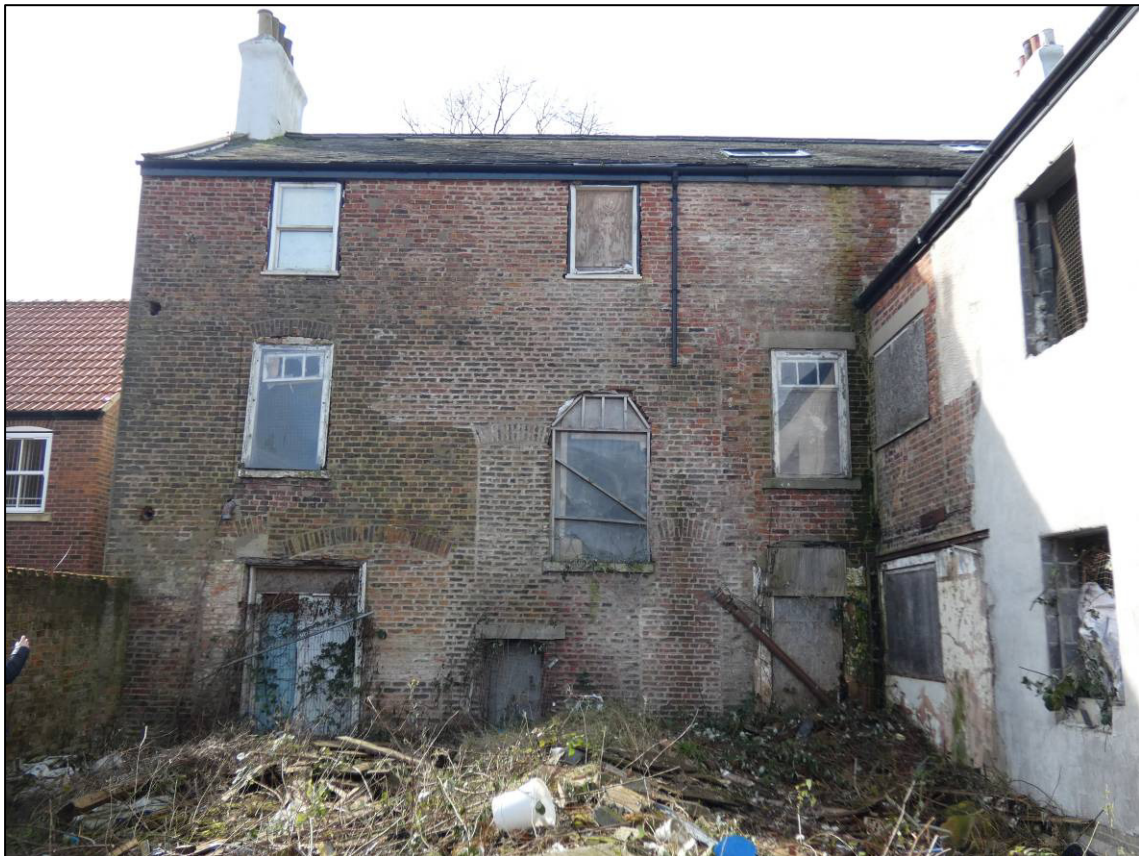
Plate 2: East (rear) elevation, looking W.
