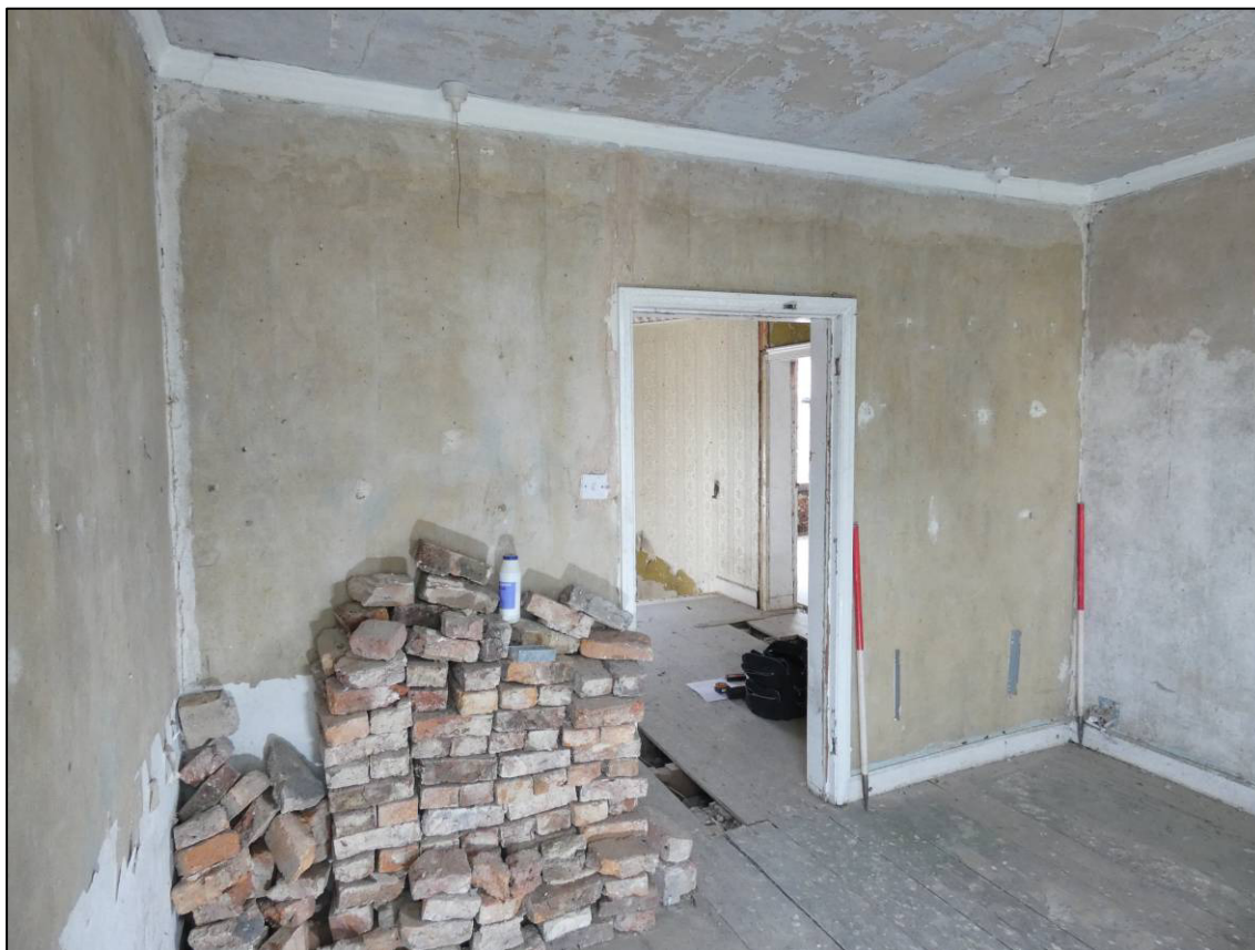
Plate 52: First floor front west room (1F4), east wall, looking E (photo 2/291).
