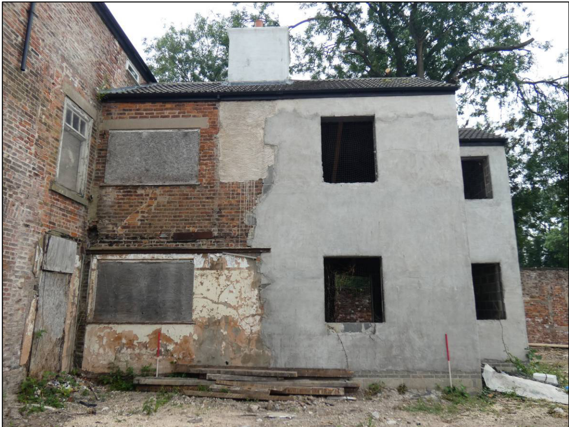
Plate 11: Rear wing, south elevation, showing 2017 extension, looking N (photo 1/037).
