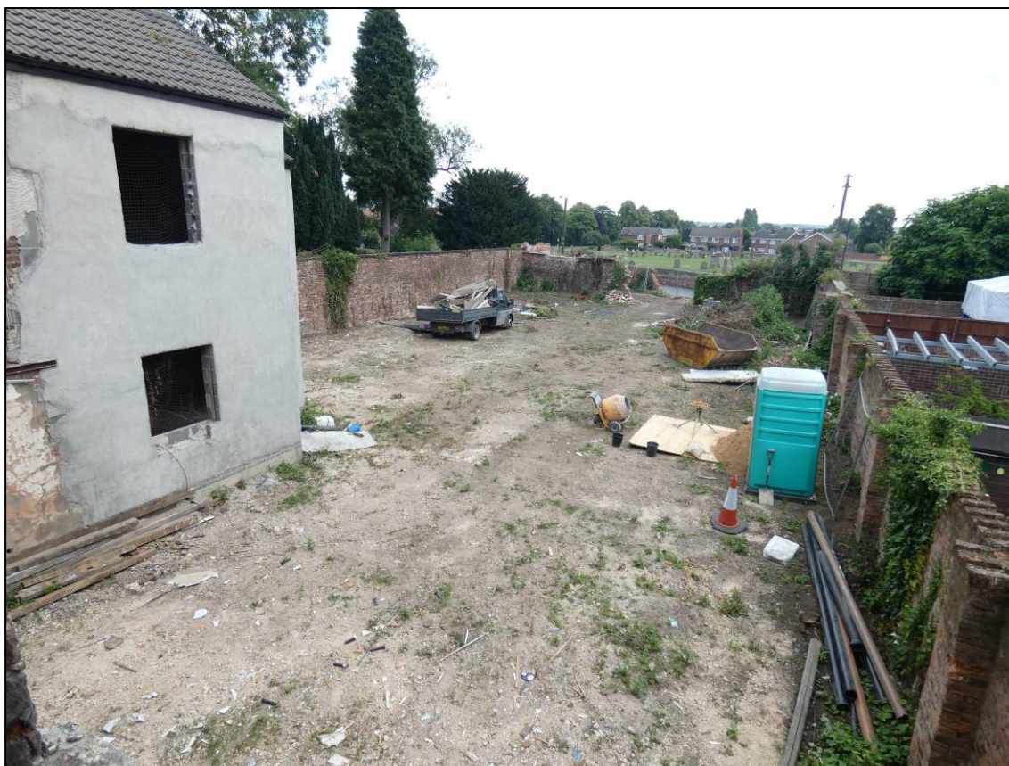
Plate 66: General view of the rear yard, looking NE (photo 2/251).
