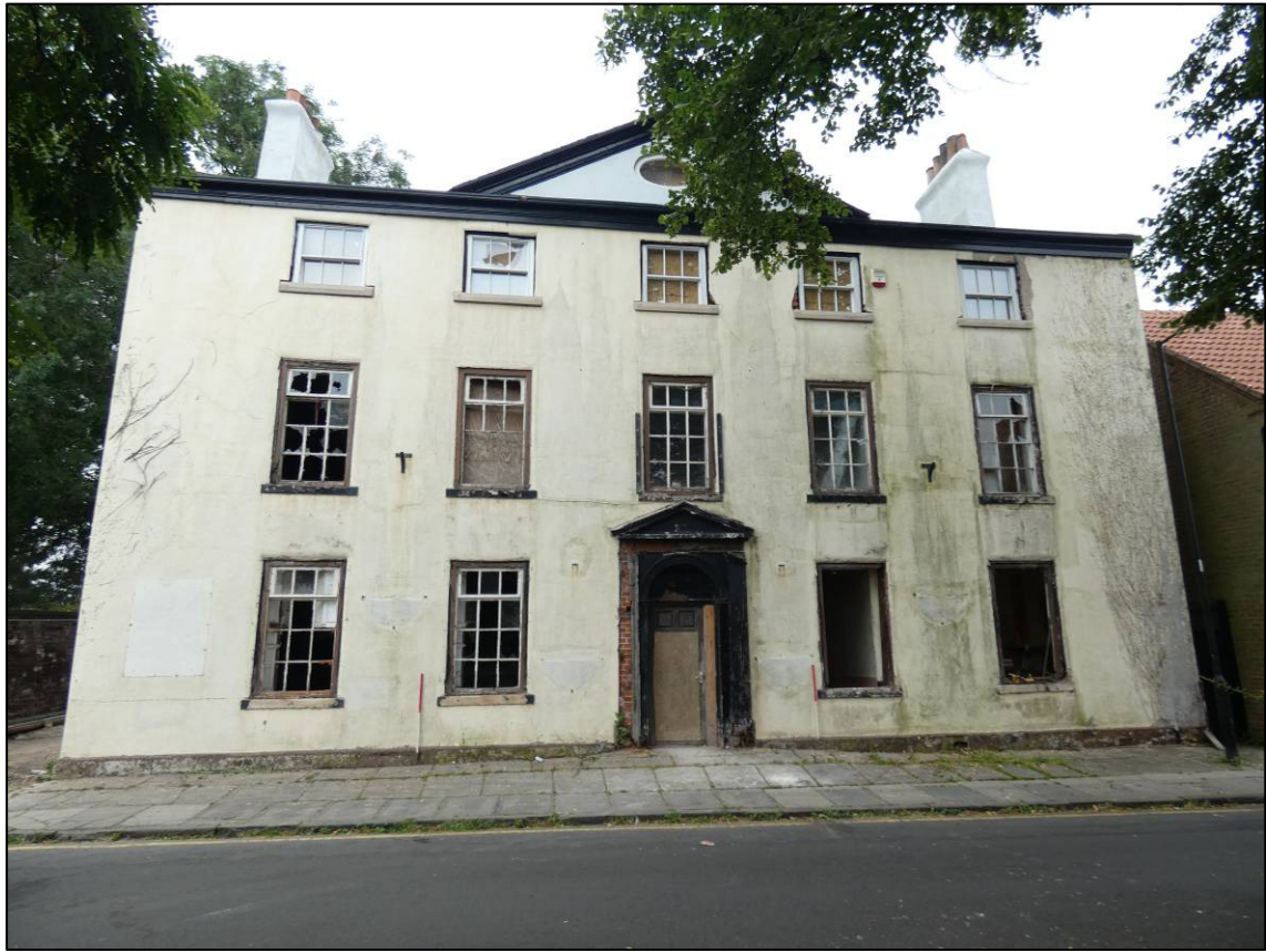
Plate 3: West elevation to Stonegate, looking E (photo 1/975).
