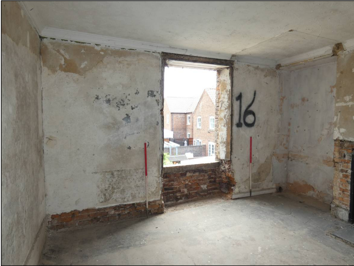
Plate 46: First floor south-east room (1F2), east wall, looking SE (photo 2/253).
