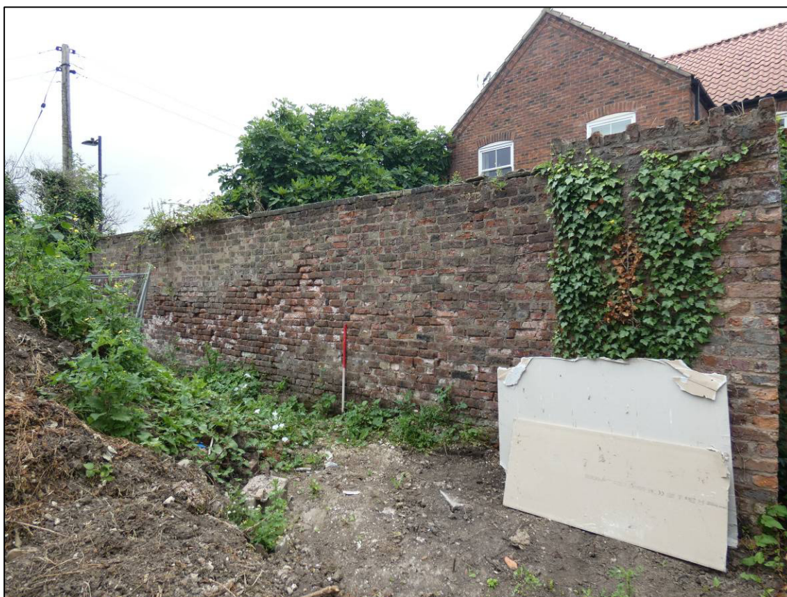
Plate 74: Rear yard, east part of south boundary wall, looking SE (photo 1/969).
