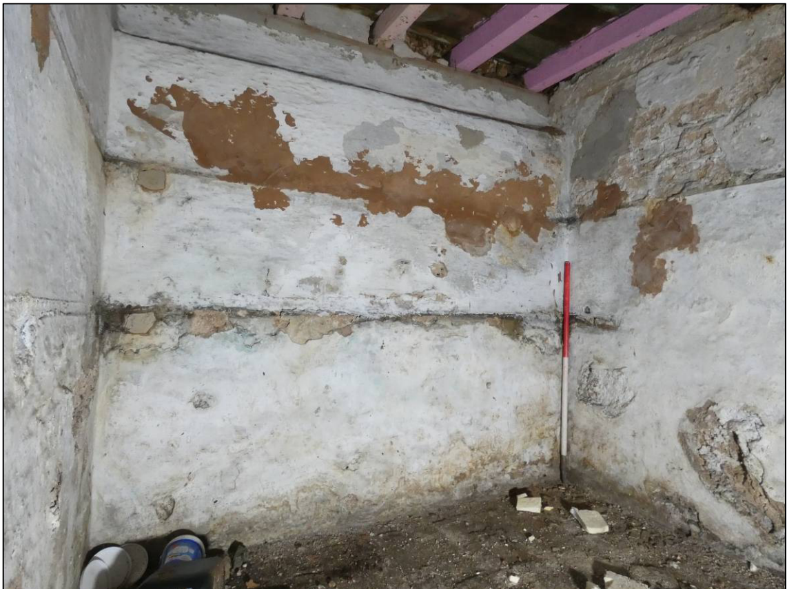
Plate 14: Cellar room C1, west wall, looking W (photo 1/099).
