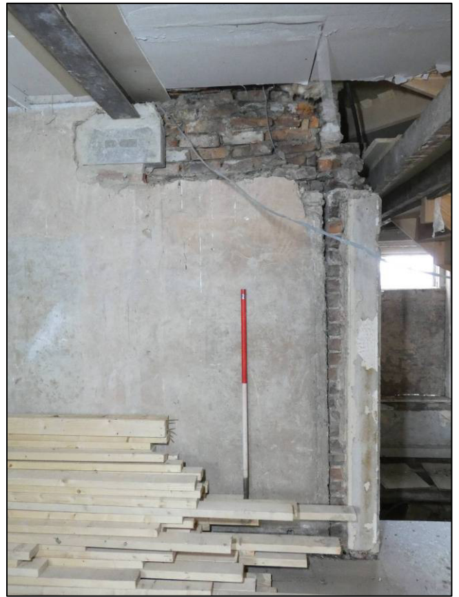
Plate 55: First floor front north room (1F5), butt joint to east wall, looking E (photo 2/303).
