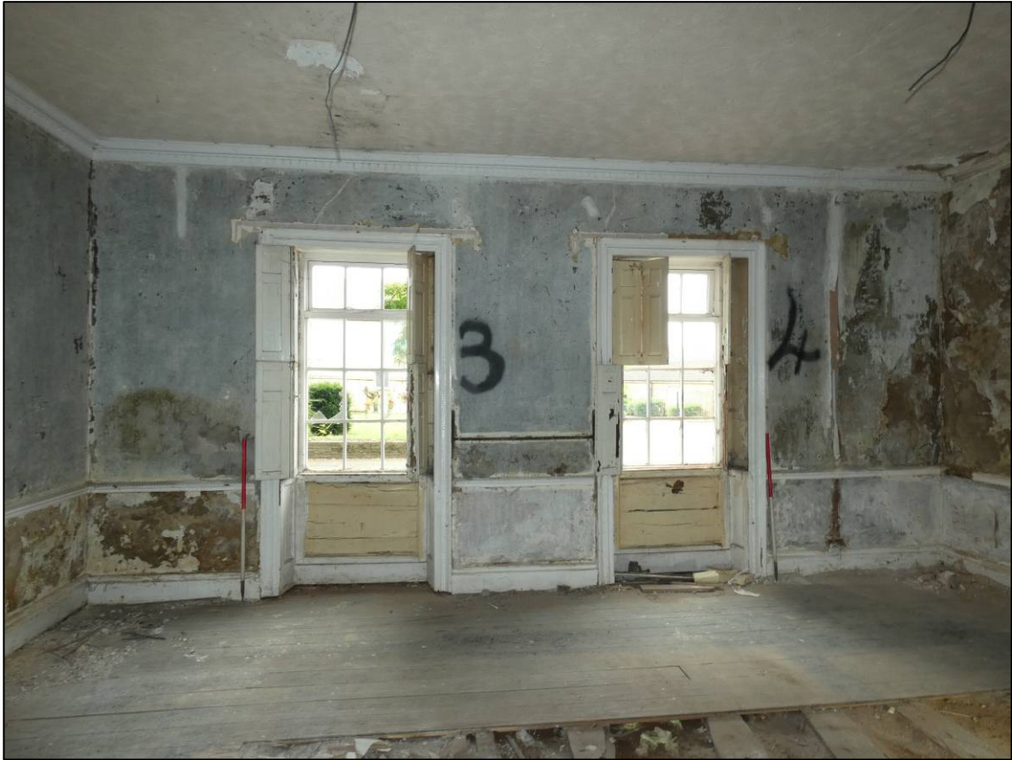
Plate 26: Ground floor north room (GF1), west wall, looking W (photo 1/064).
