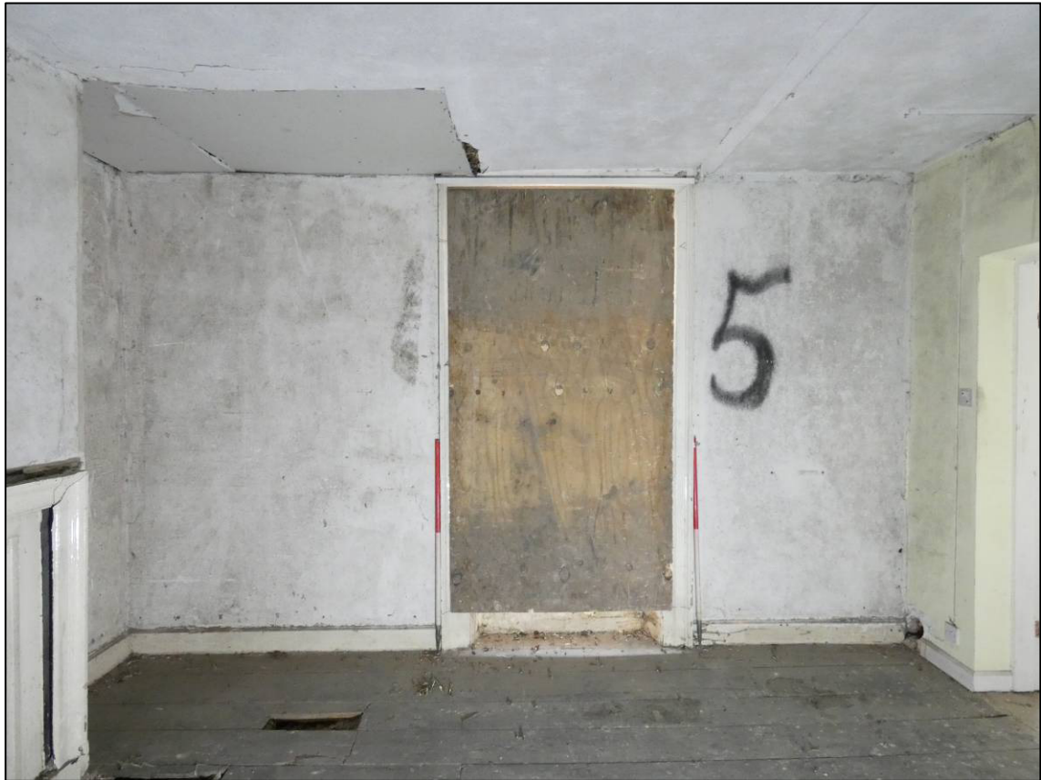
Plate 50: First floor south-west room (1F3), west wall, looking W (photo 2/281).
