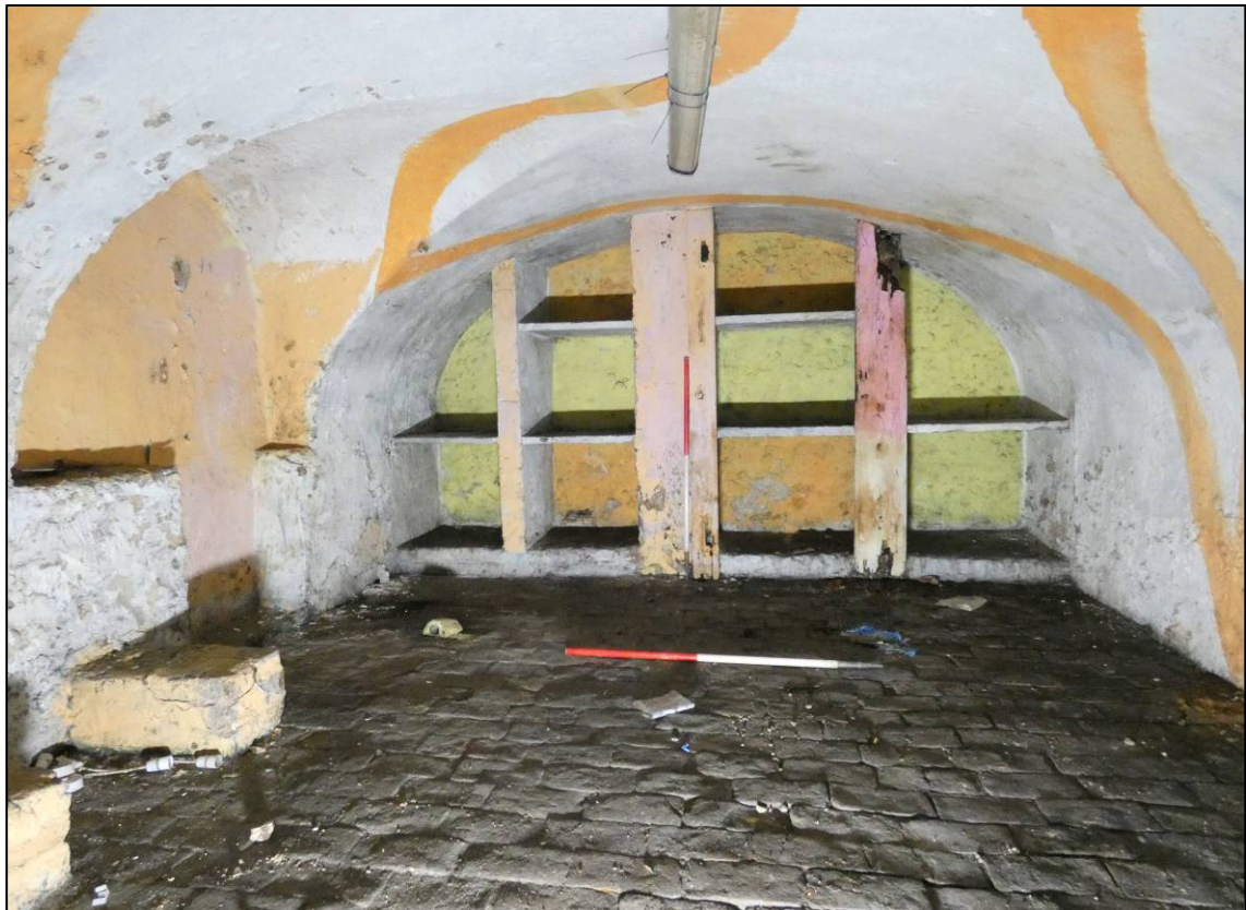
Plate 16: Cellar room C1, shelves to south wall, looking S (photo 1/093).
