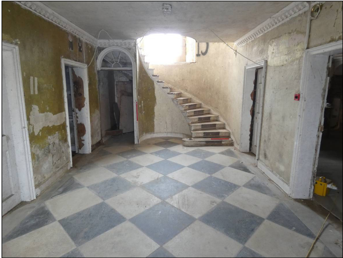
Plate 17: Ground floor entrance hall (GF2), looking E (photo 2/206).
