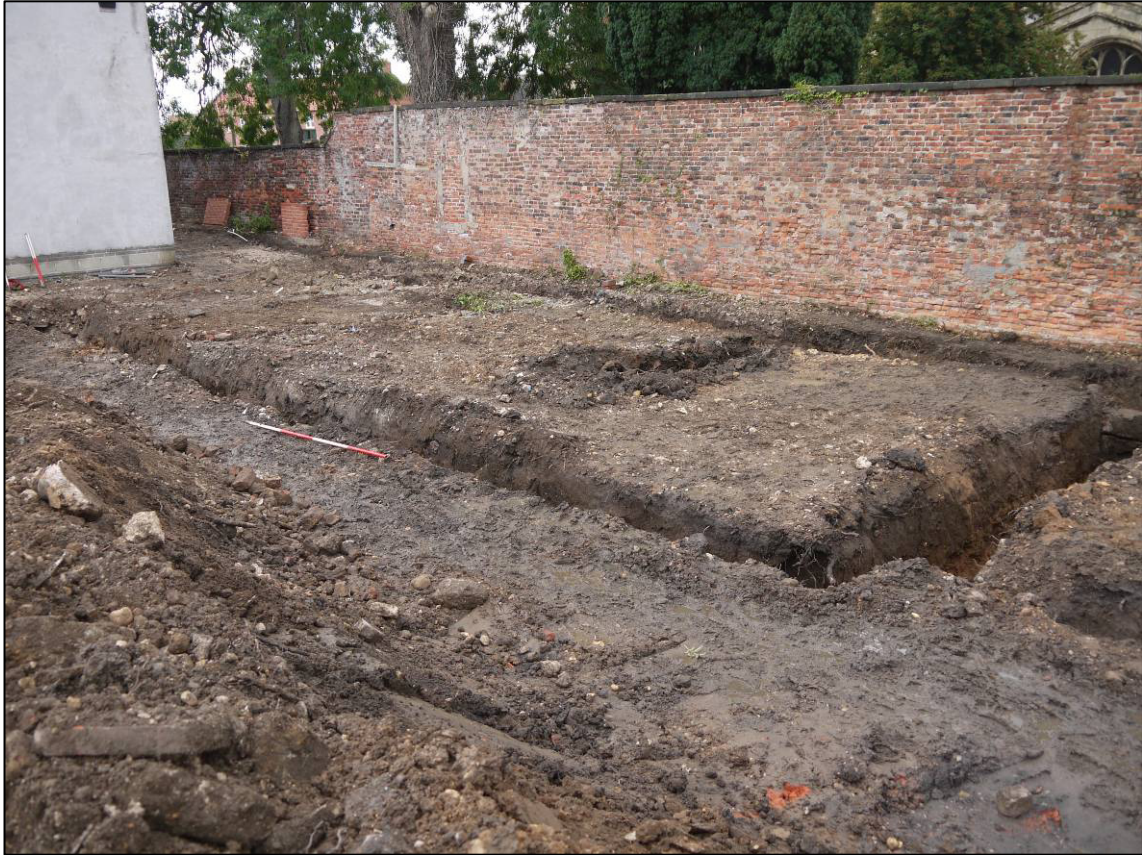
Plate 81: Trenches undergoing excavation for west end of new building, looking NW.
