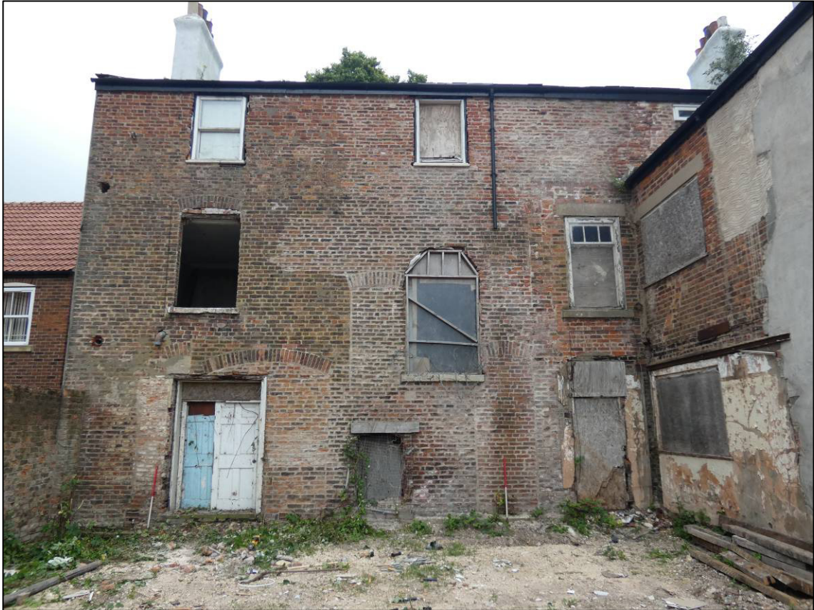
Plate 8: East elevation, looking W (photo 1/028).
