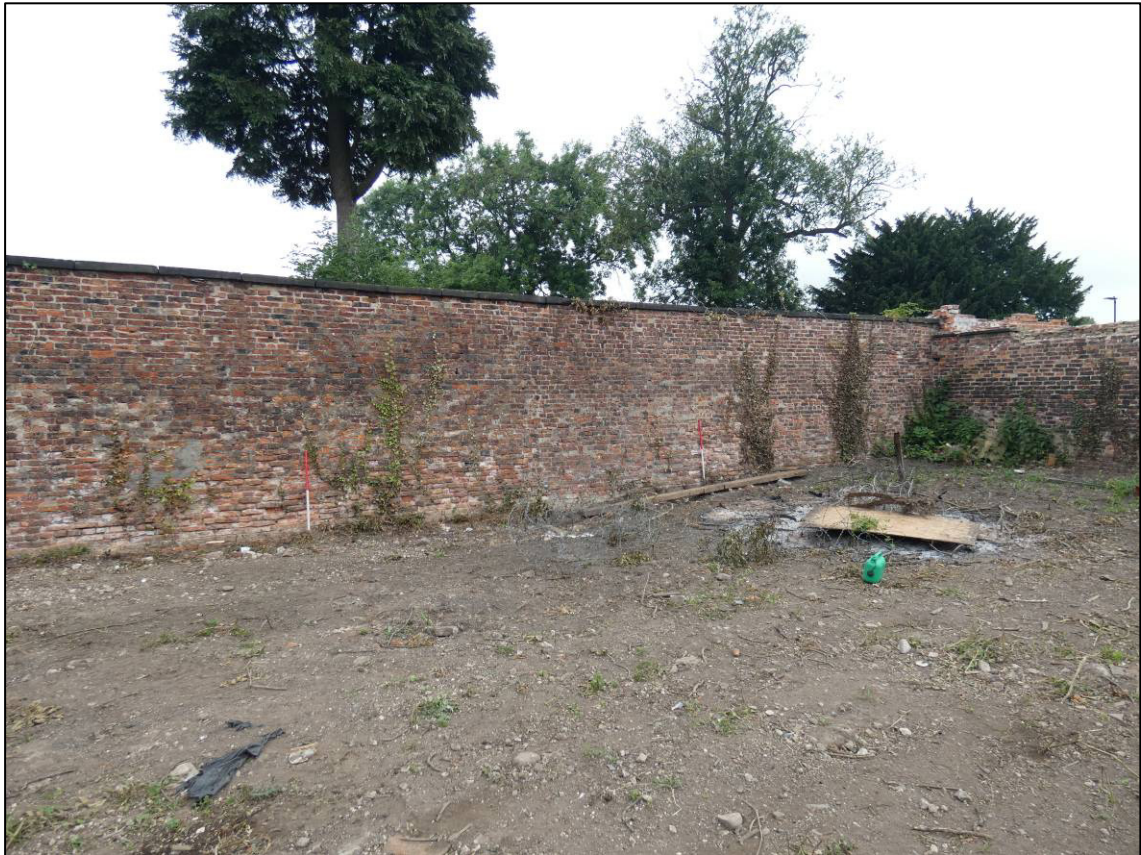
Plate 69: Rear yard, east end of north boundary wall, looking NE (photo 1/962).
