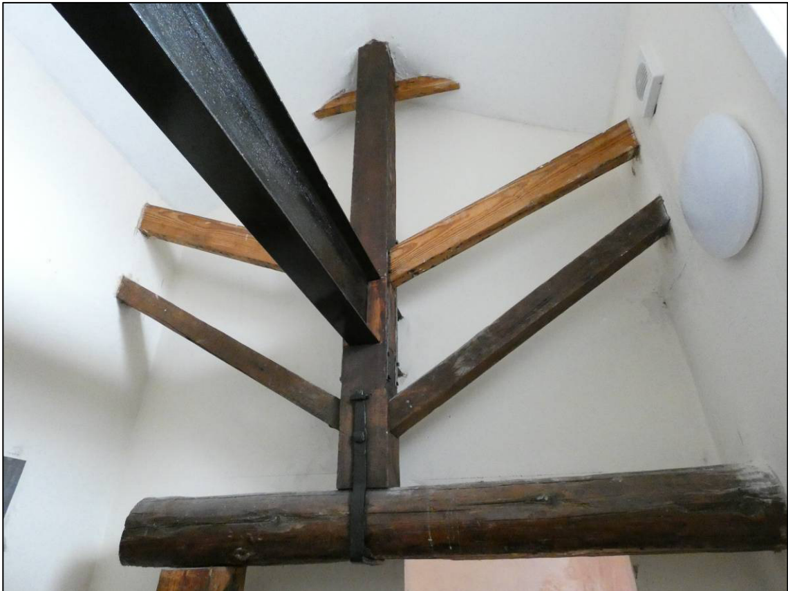
Plate 63: Second floor, east room (2F3), roof truss, looking N (photo 2/318).
