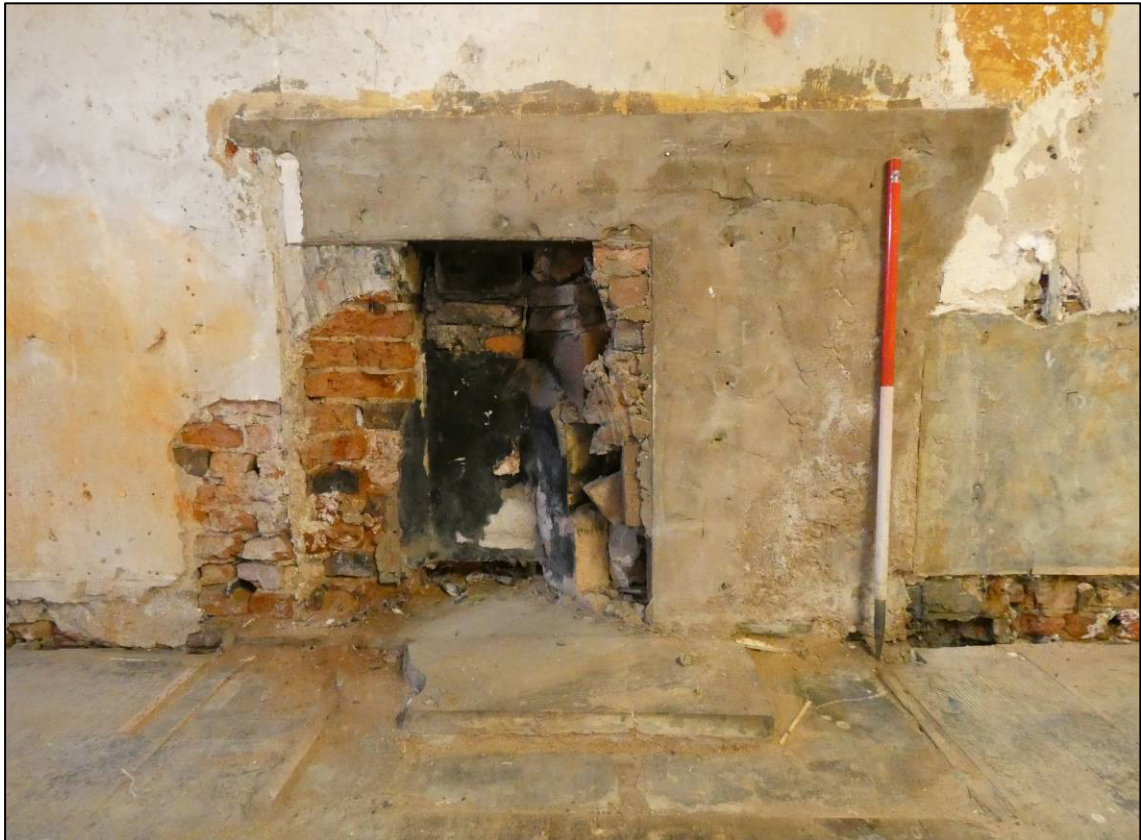
Plate 32: Ground floor south room (GF3), fireplace to south wall, looking S (photo 2/159).
