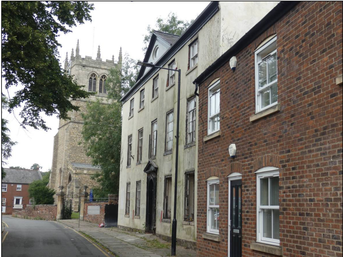
Plate 1: West elevation to Stonegate, looking N (photo 1/986).
