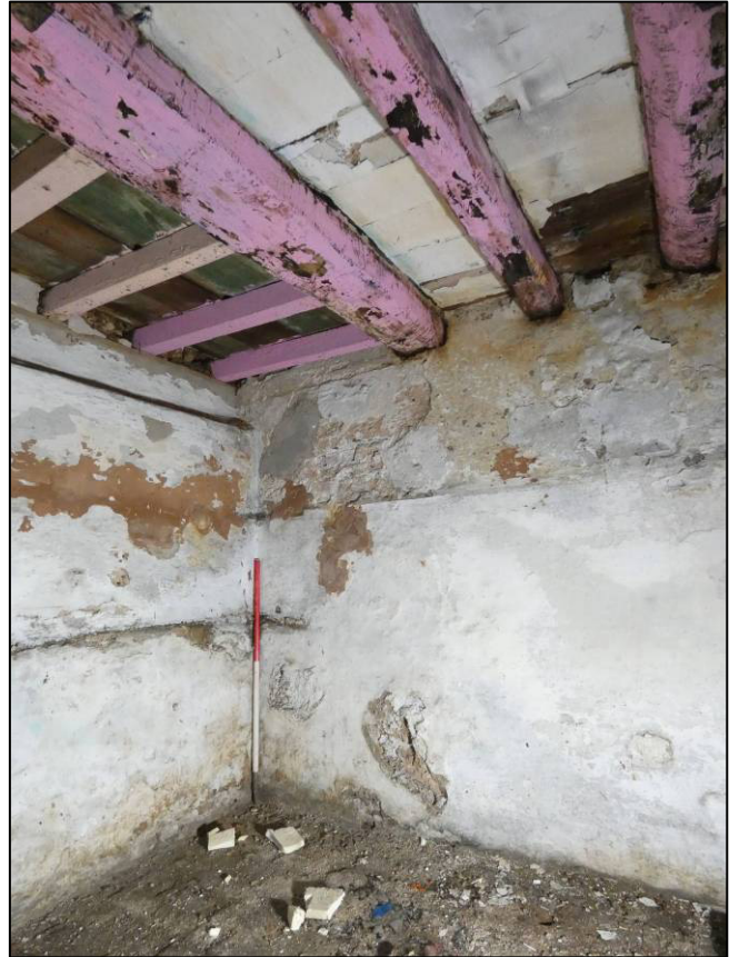
Plate 13: Cellar room C1, looking NW (photo 1/098).
