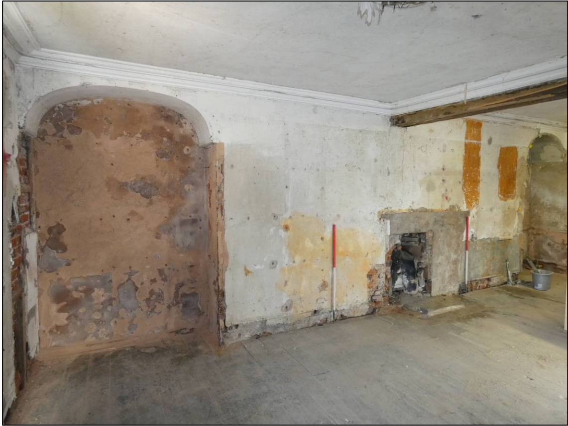
Plate 31: Ground floor south room (GF3), south wall, looking SW (photo 2/144).
