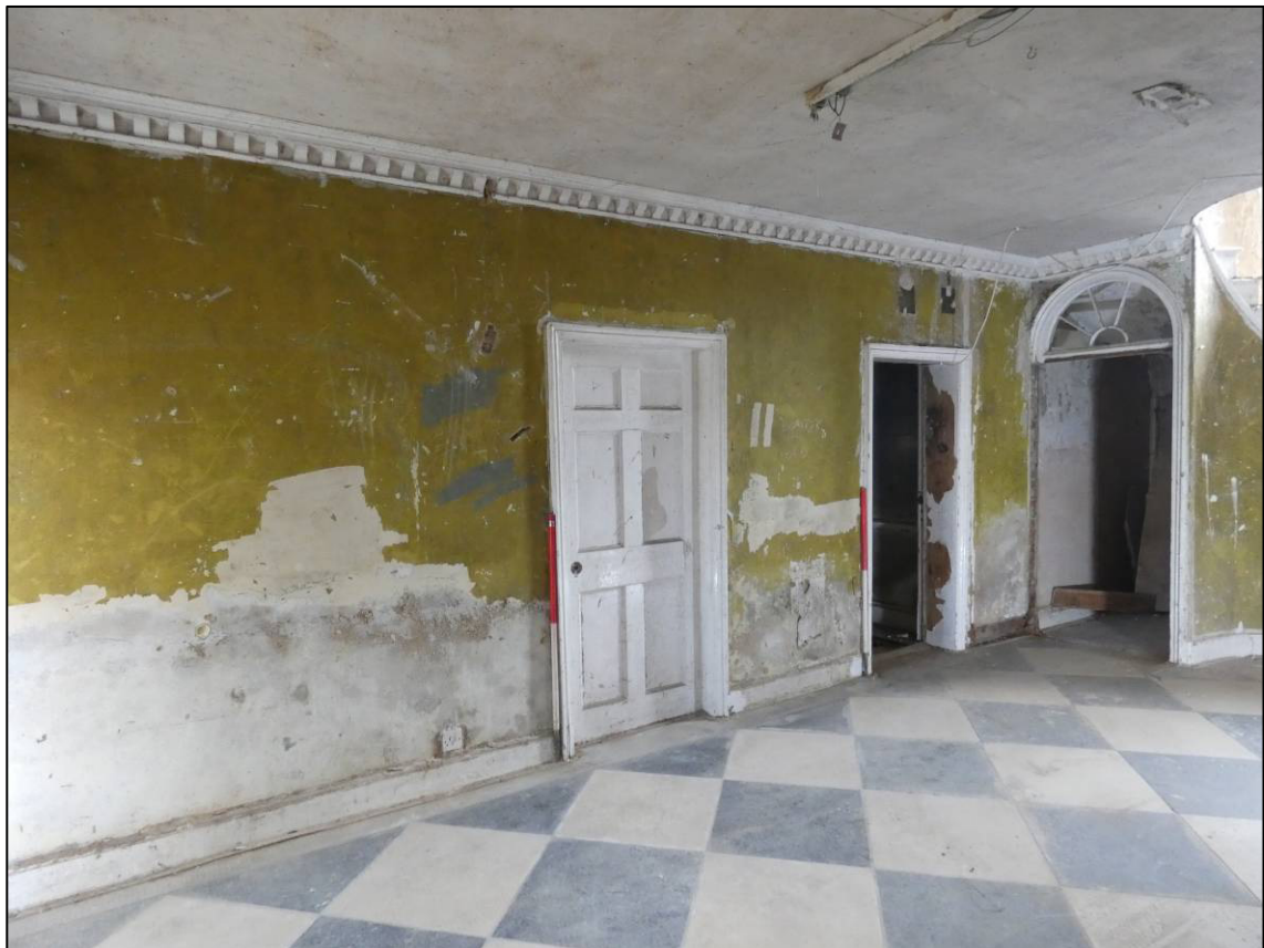
Plate 18: Ground floor entrance hall (GF2), north wall, looking NE (photo 2/190).
