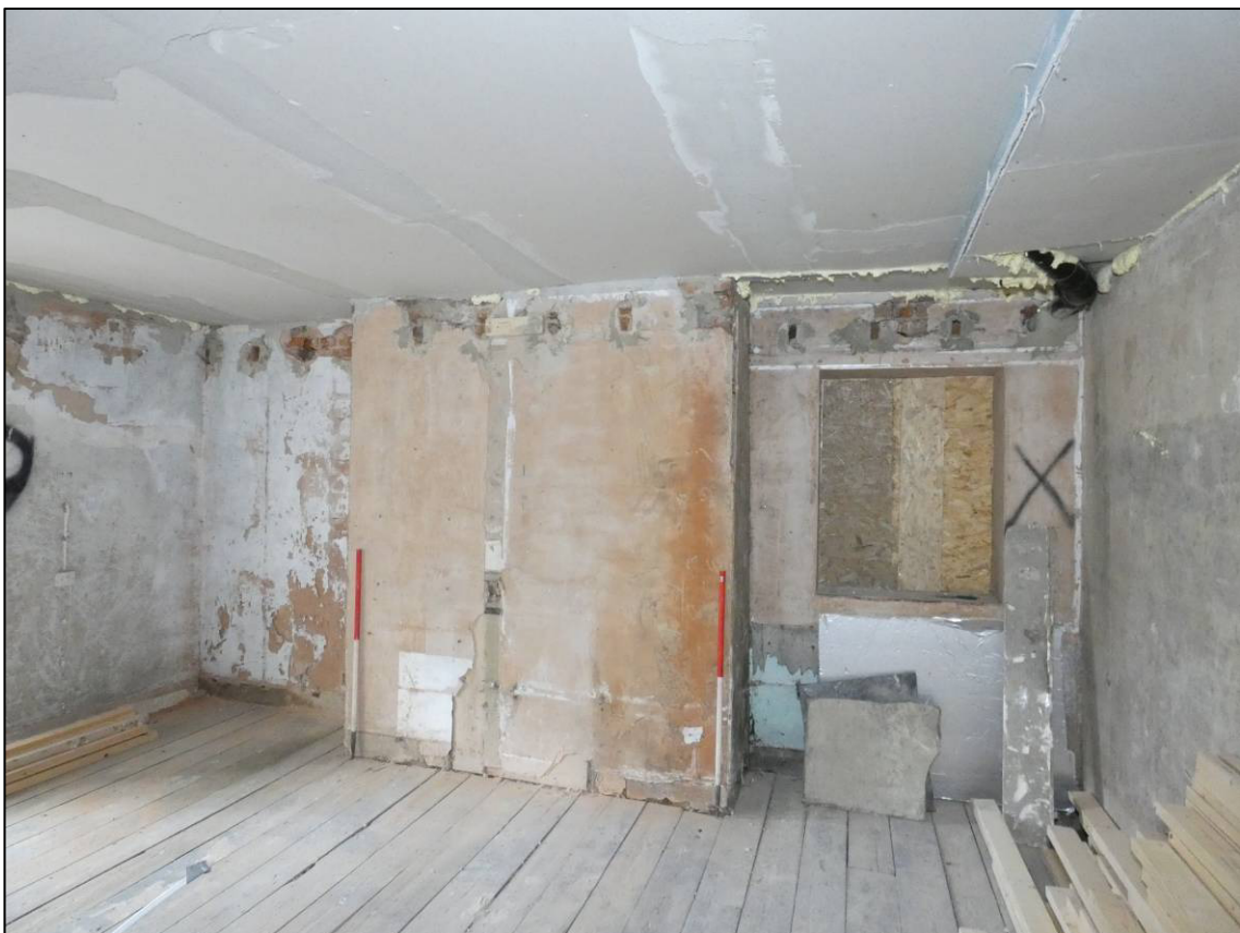
Plate 56: First floor front north room (1F5), north wall, looking NW (photo 2/301).
