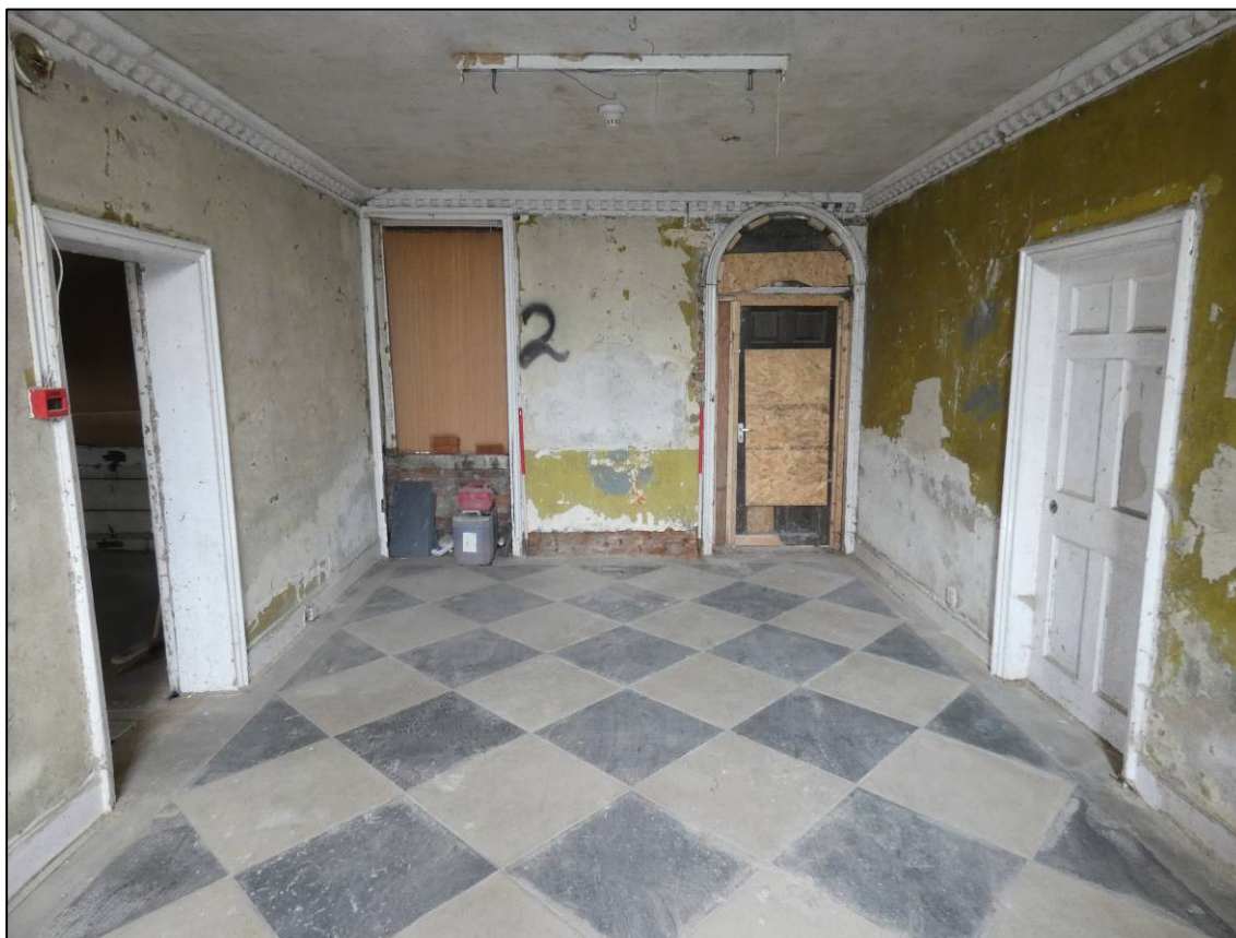
Plate 19: Ground floor entrance hall (GF2), west wall, looking W (photo 2/176).
