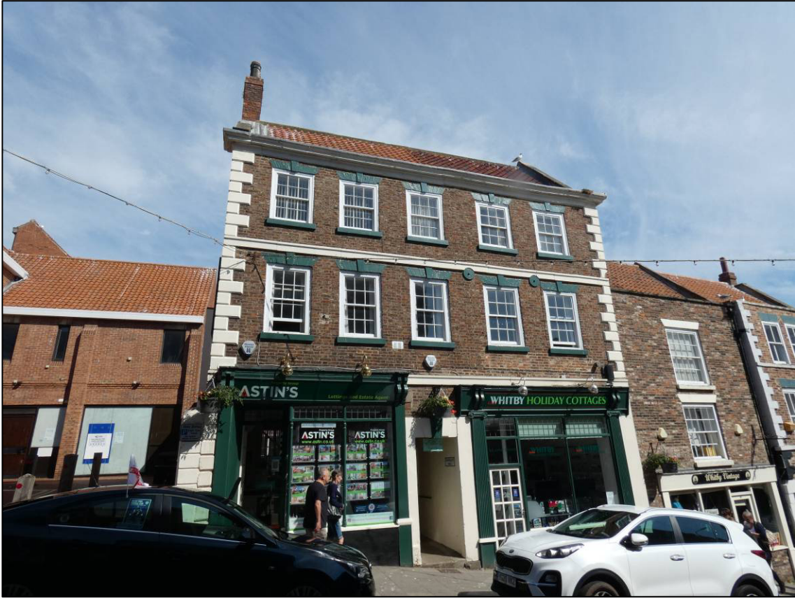
Plate 1: No. 47 Flowergate, south elevation, looking N.
