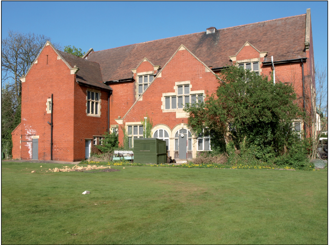
Plate 3: West elevation, viewed from bowling green, looking NE (photo 6/66).
