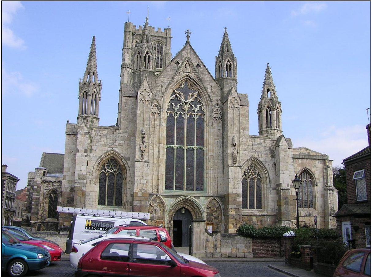
Plate 4: West front prior to restoration.
