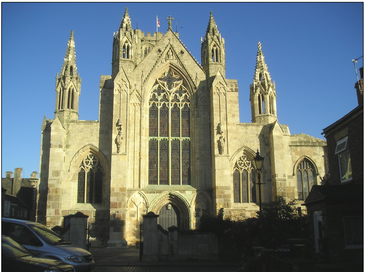
Plate 5: West front after restoration.
