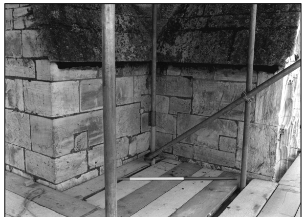
Photo 2/10: Possible putlog holes, north nave buttress, looking S.
