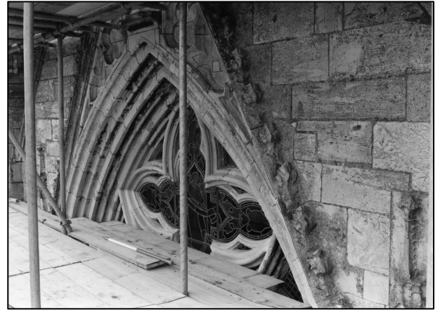
Photo 2/6: Crocketed gable to west window, looking NE.
