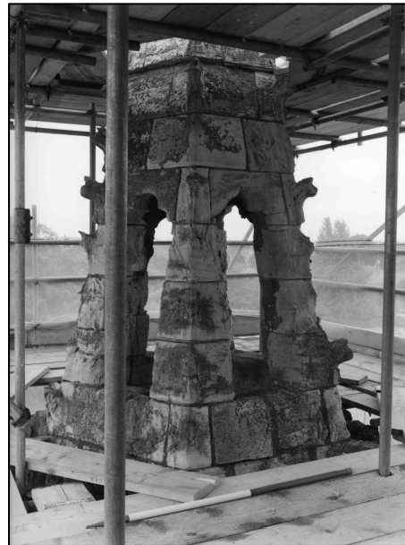
Photo 2/7: Spirelet of north aisle turret, looking NW.
