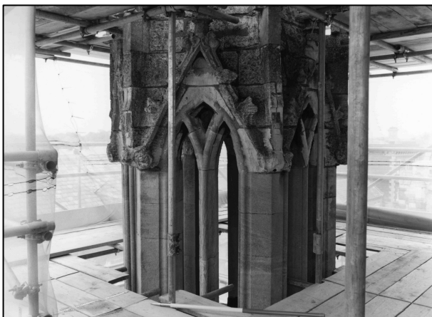
Photo 2/8: North aisle turret, looking NW.
