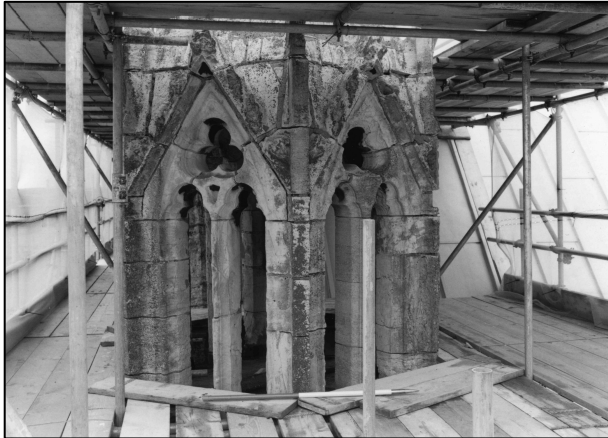
Photo 1/16: South nave turret, looking S.
