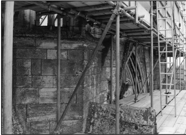
Photo 2/4: North nave turret base, looking S.
