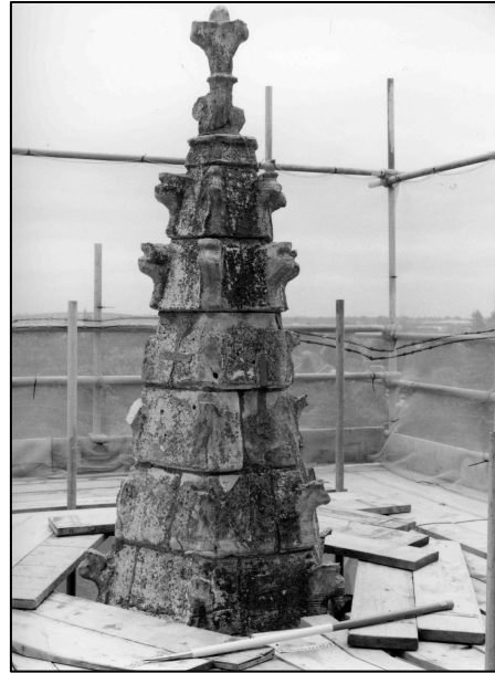
Photo 1/17: Top of spirelet of north aisle turret, looking NW.
