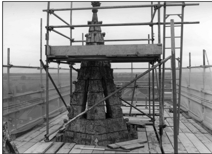
Photo 1/4: Spirelet of north nave turret, looking N.
