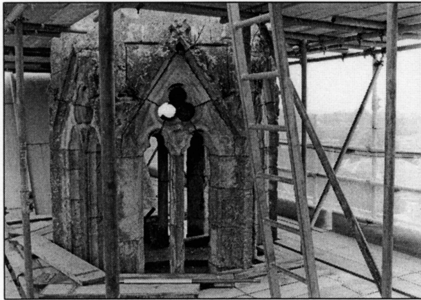
Photo 1/10: South nave turret, looking S.
