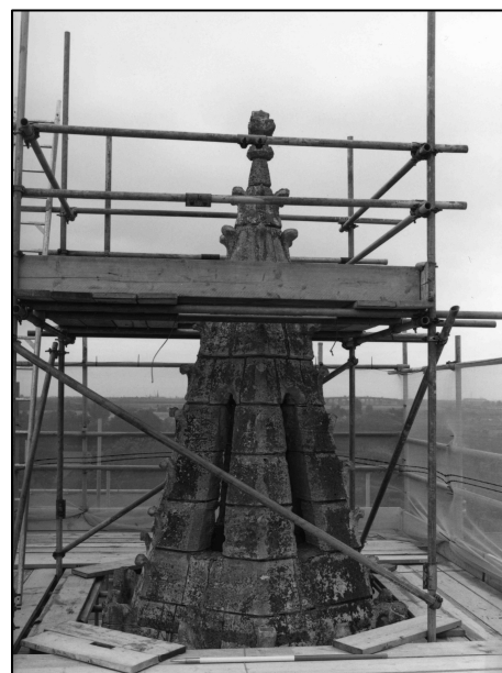
Photo 1/6: Spirelet of south nave turret, looking S.
