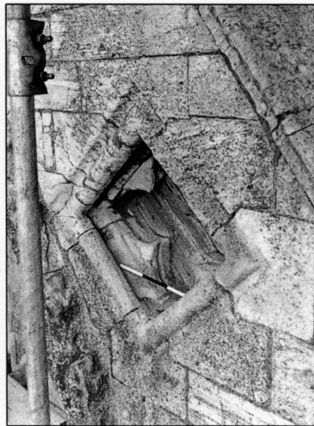
Photo 1/13: South quatrefoil flanking Majestas, looking N.
