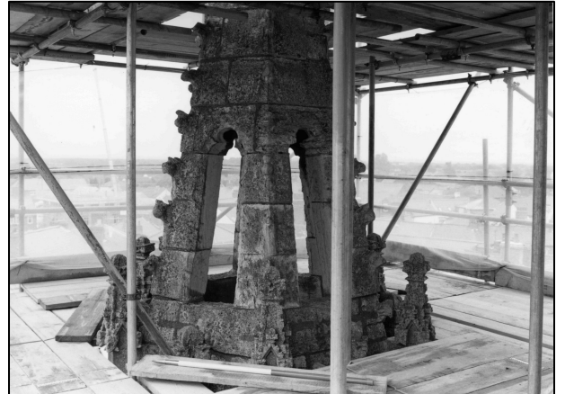
Photo 1/18: Spirelet of north aisle turret, looking NW.
