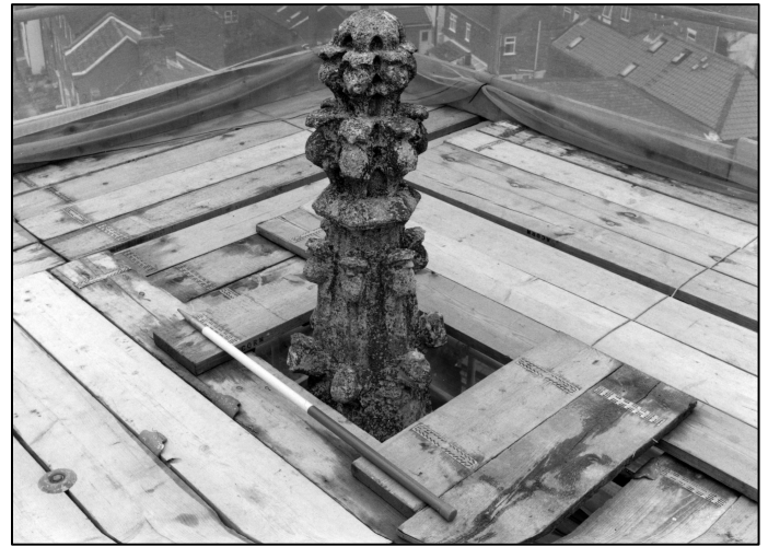
Photo 1/2: Apex of spirelet of north nave turret, looking NW.
