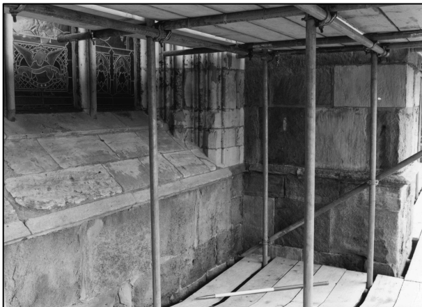
Photo 4/11: Sill and south jamb of south aisle window, looking S.
