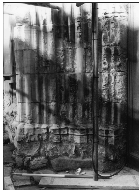
Photo 5/3: North jamb of west door.
