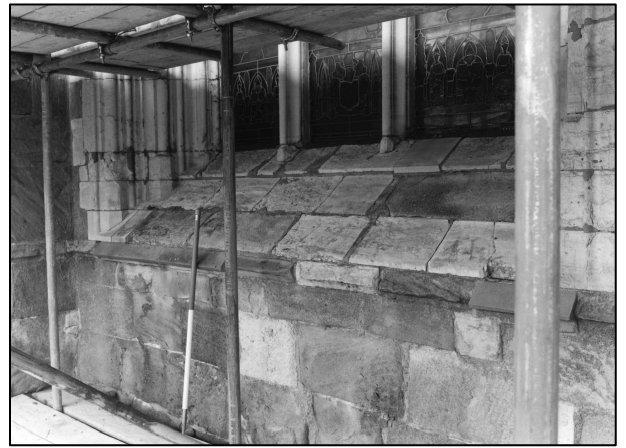
Photo 4/17: Sill of south aisle window, looking NE.
