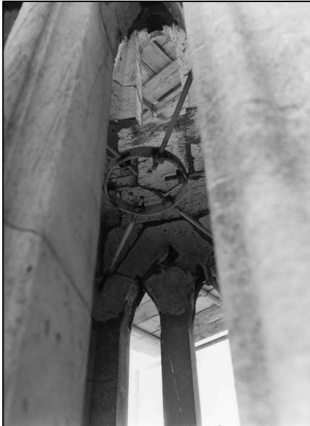
Photo 3/7: North aisle turret, central ring.
