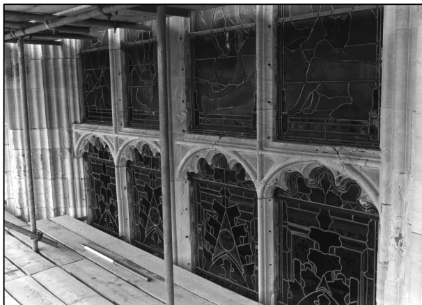
Photo 3/14: Perpendicular transom, west window, looking NE.
