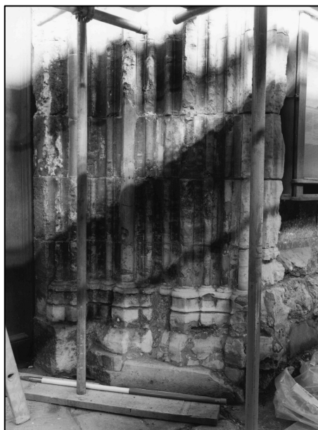
Photo 5/1: South jamb of west door.
