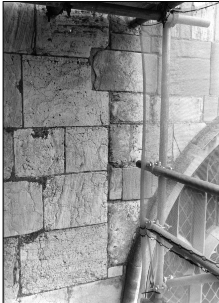
Photo 4/7: Joint between south aisle and grammar school, looking SE.
