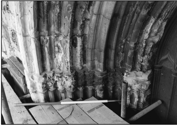
Photo 4/14: Detail of moulding to north side of west door, looking NE.
