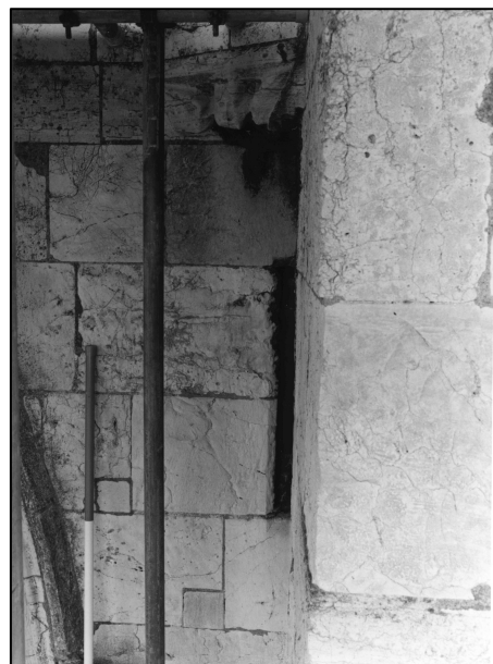
Photo 4/6: Putlogs and winged figure corbel to south aisle turret, looking E.
