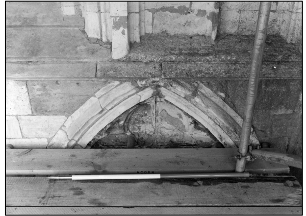
Photo 4/10: Blind arcading on south side of west door, looking E.
