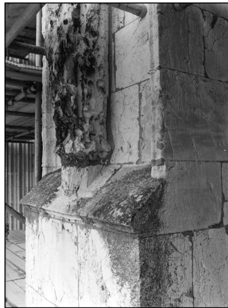
Photo 4/4: Base of figure, south nave buttress, looking N.
