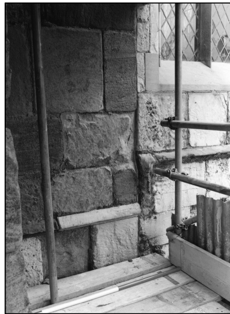
Photo 4/18: Joint between south aisle and grammar school, looking SE.
