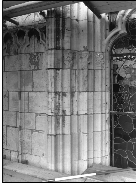
Photo 3/6: North jamb of west window, looking NE.
