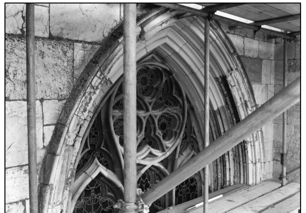
Photo 3/17: North aisle window head, looking SE.
