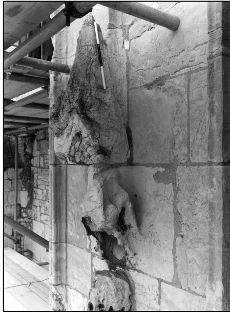
Photo 3/11: Canopy over figure, north nave buttress, looking N.
