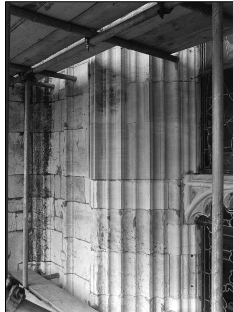
Photo 3/15: North jamb of west window, looking N.
