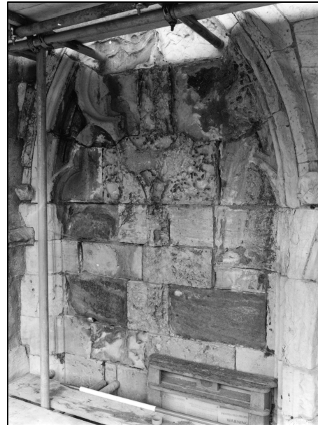
Photo 4/13: Blind arcading on north side of west door, looking NE.
