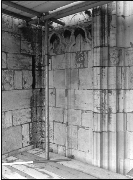
Photo 3/5: Blind arcading, north side of west window, looking NE.
