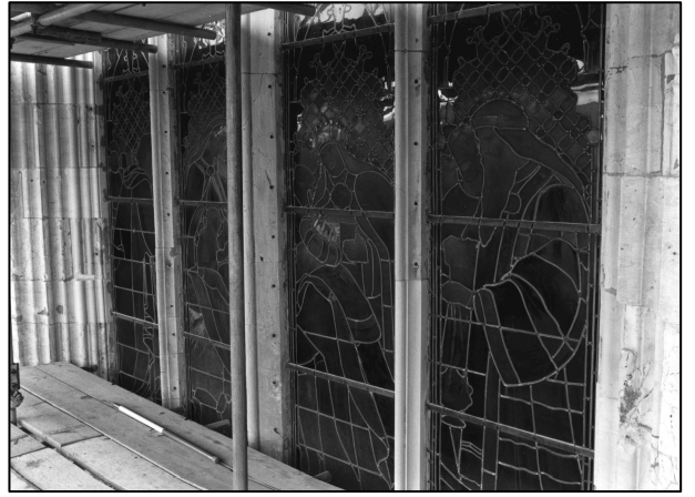
Photo 4/2: Lower part of west window, looking NE.
