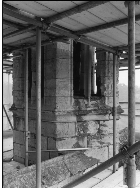
Photo 3/8: South aisle turret, looking S.
