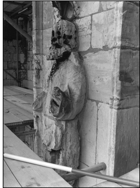
Photo 3/12: Figure, north nave buttress, looking N.
