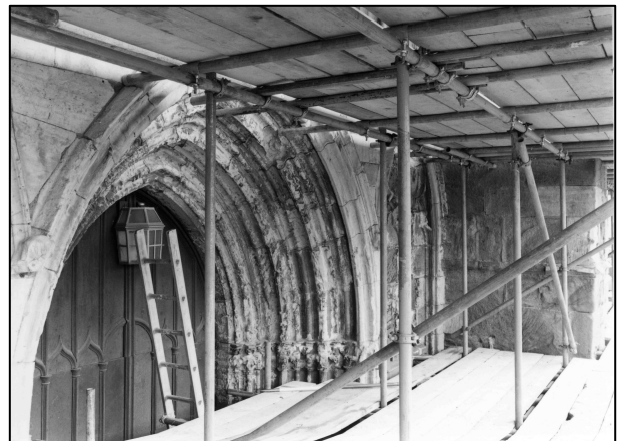
Photo 4/12: Head of west door, looking S.
