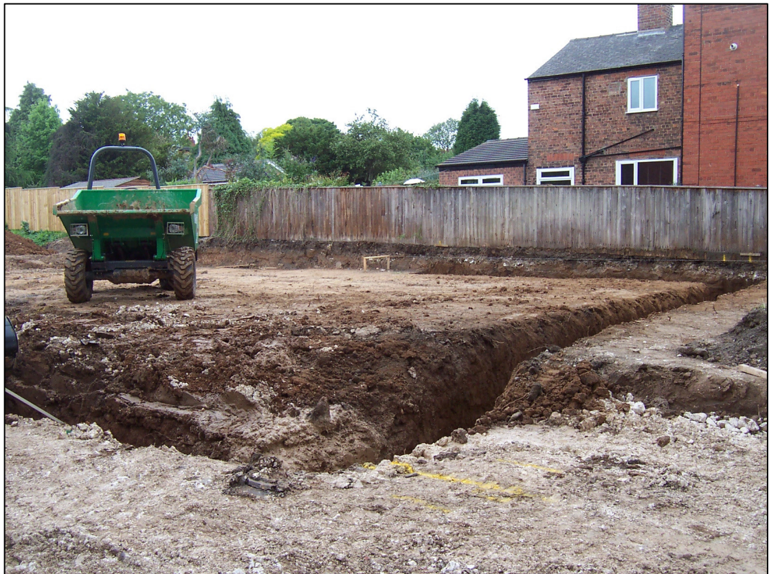
Plate 2: Excavated foundation trenches, looking NW.
