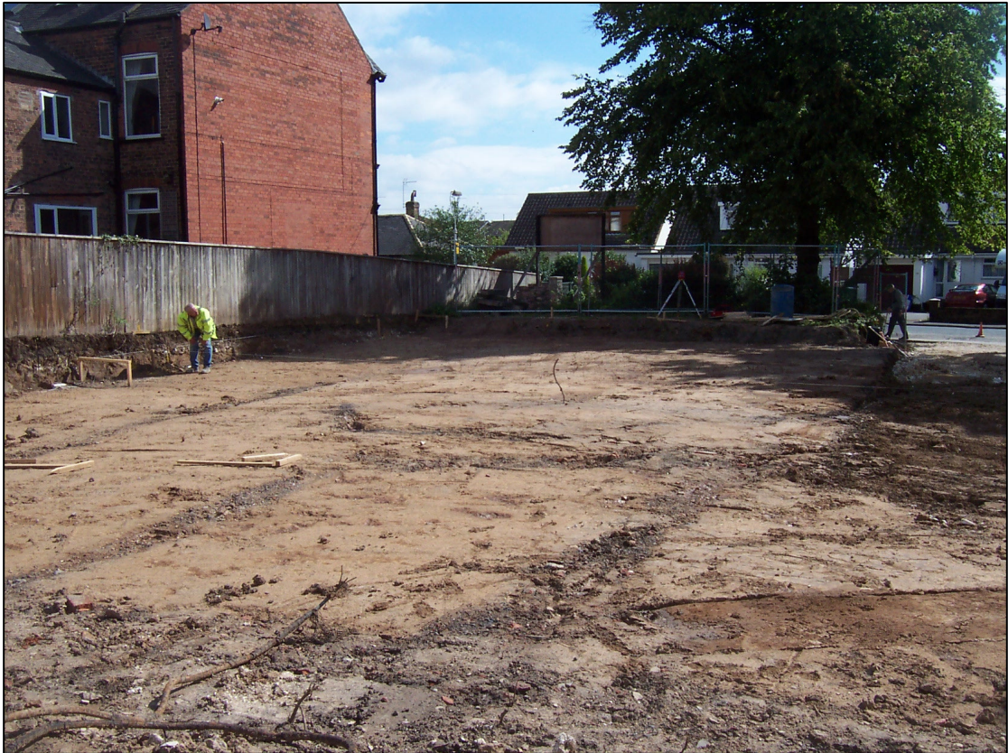
Plate 1: General view of stripped site, looking NE.
