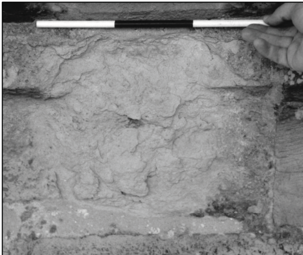
Plate 26: Corbel S8 - eroded original and replacement
