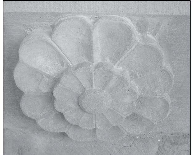
Plate 25: Corbel S5 - eroded original and replacement.
