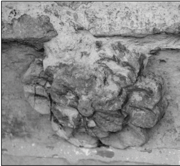
Plate 25: Corbel S5 - eroded original and replacement.
