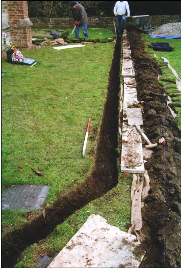
Plate 7: General view of Trench 2 under excavation, looking east.
