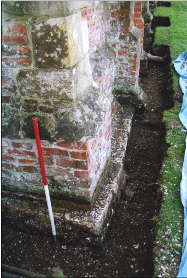
Plate 4: Footings around butress F, looking west.
