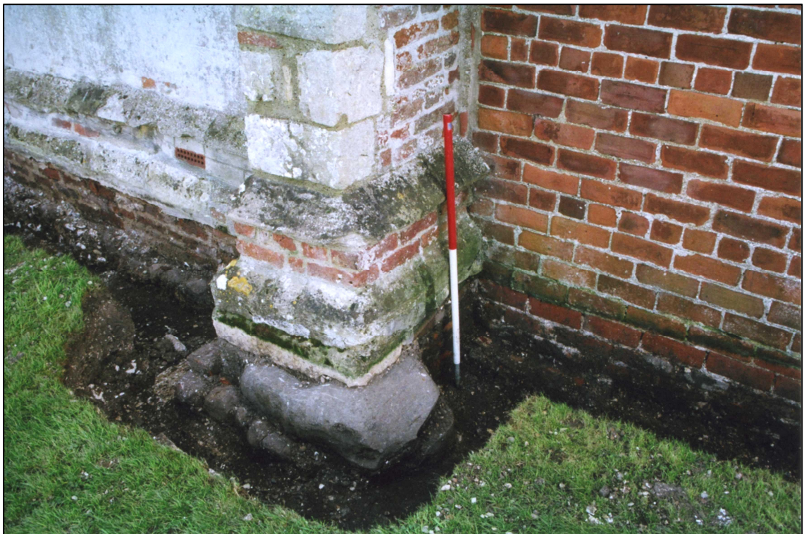
Plate 6: Footings to butress A on north aisle, looking south-east.
