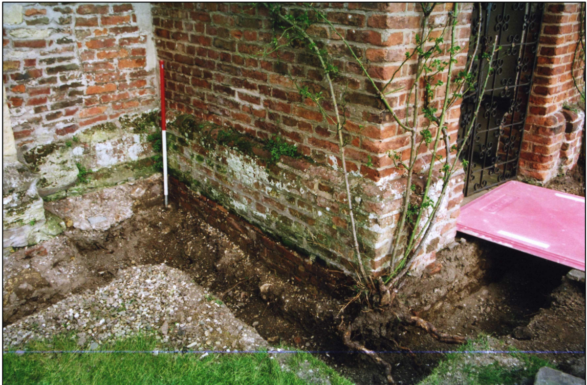
Plate 9: Footings of south porch, looking north-east.
