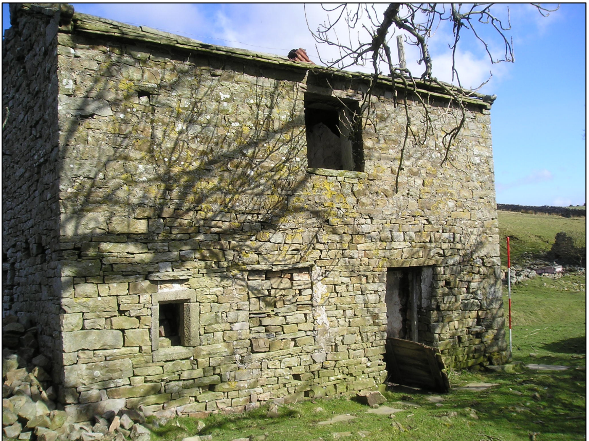
Plate 2: South elevation, looking NE (photo 1/2).
