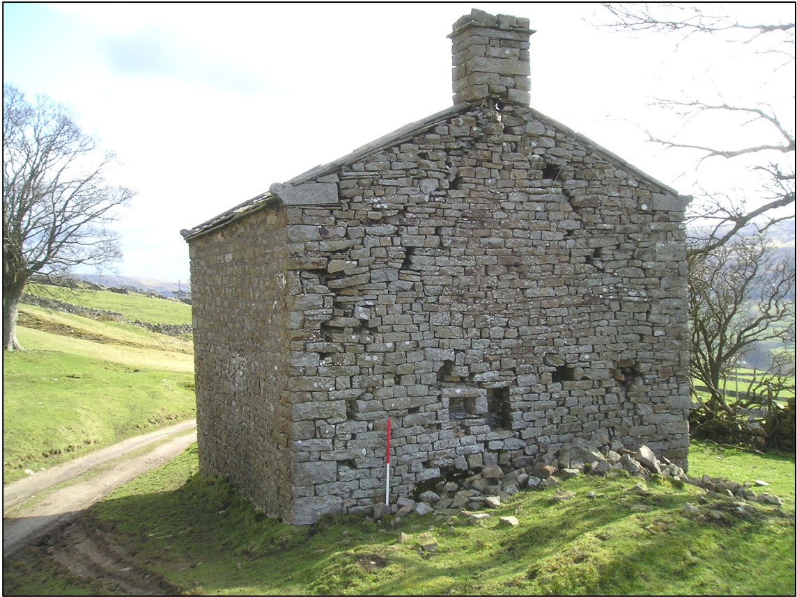
Plate 3: West gable, looking E (photo 1/11).
