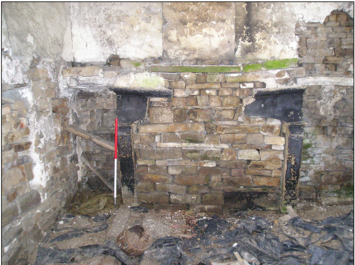
Plate 4: Blocked fireplace, internal west wall, looking W (photo 1/15).
